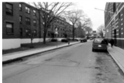
The Charlestown Development (show above) will be undergoing several changes in the coming months
