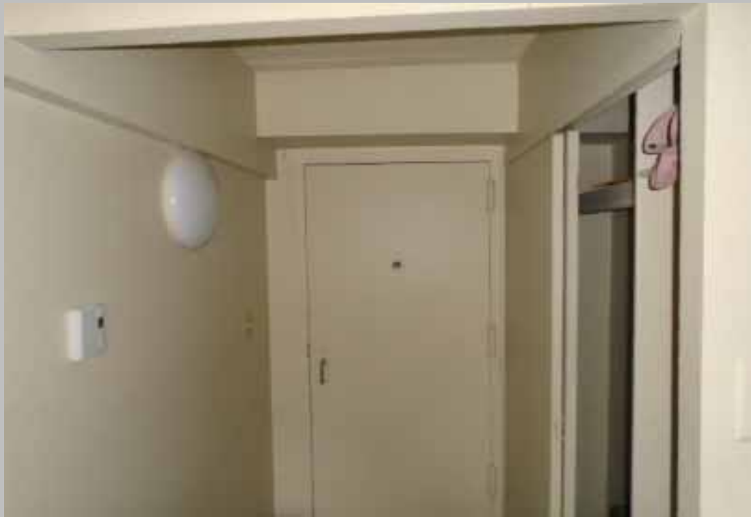
Install Automatic Door Openers at the Ten (10) Designated Handicapped Dwelling Units (Critical Repair)
