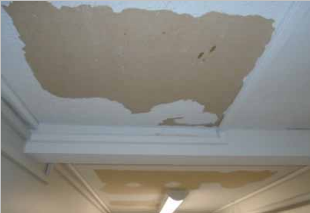
Paint Common Hallway Ceiling on the 7 th Floor (Non-Critical Repair)
