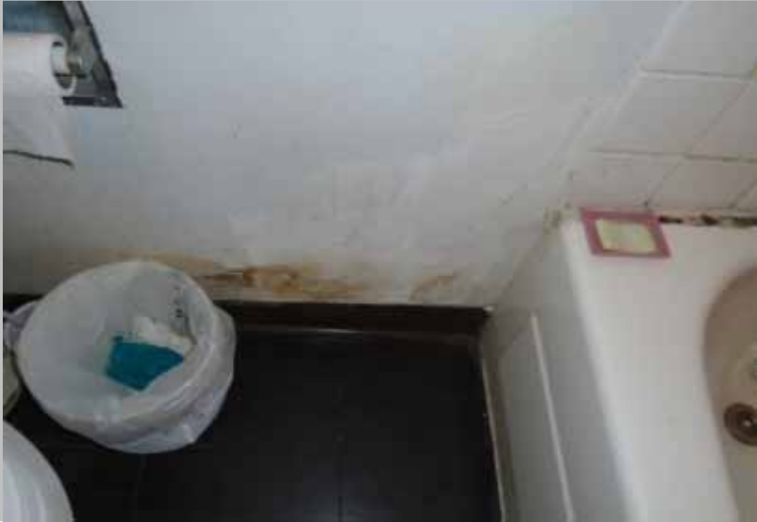
Fix Bathroom Wall in Unit 1703 (Non-Critical Repair)
