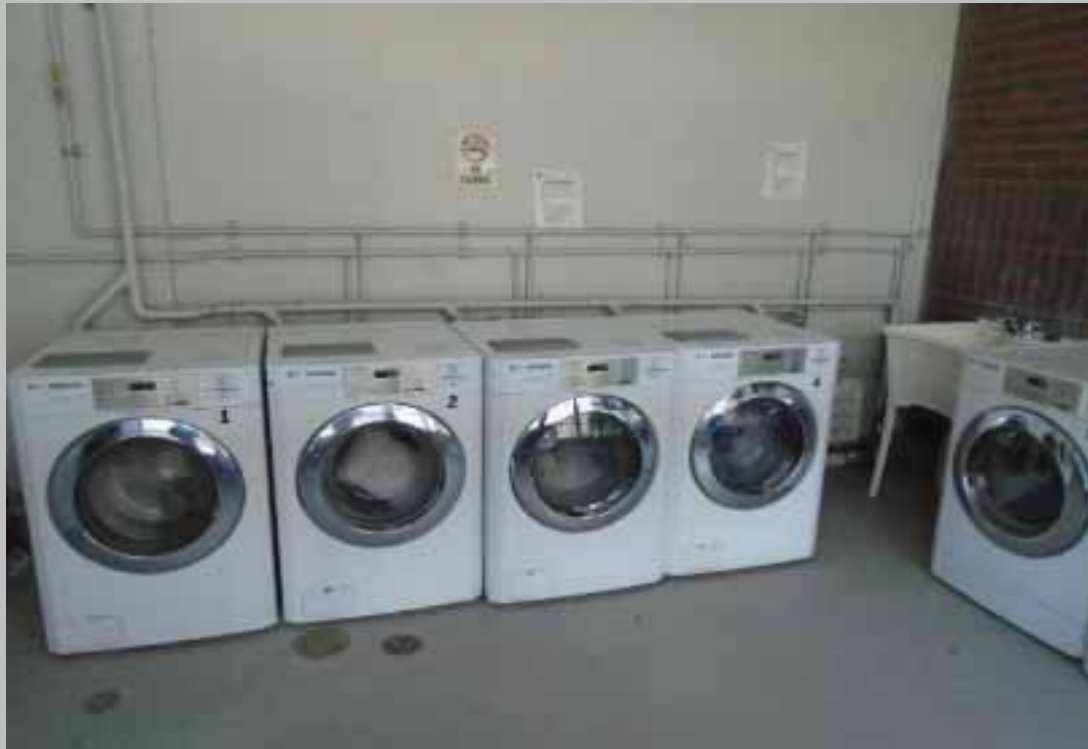
Common Laundry Room
