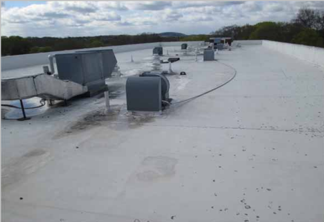
View of the building roof surface
