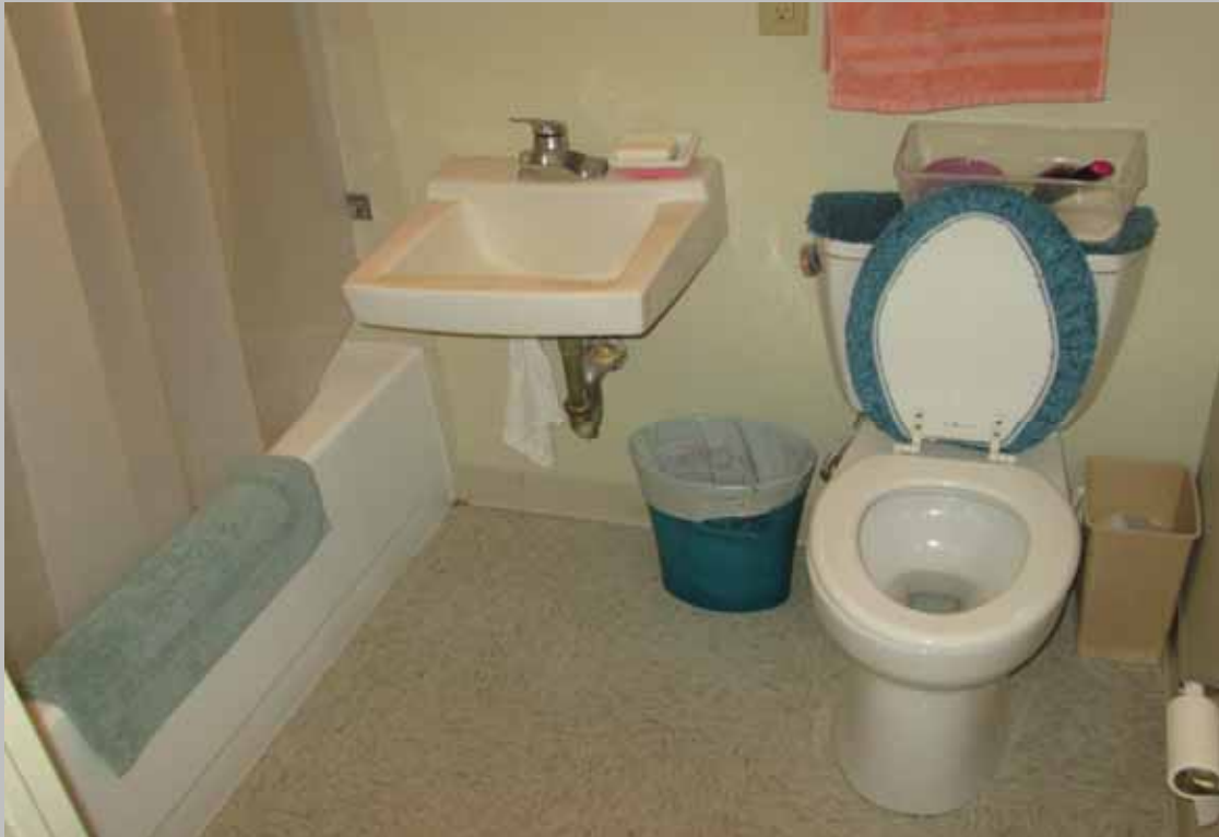
View of bathroom at Unit 217
