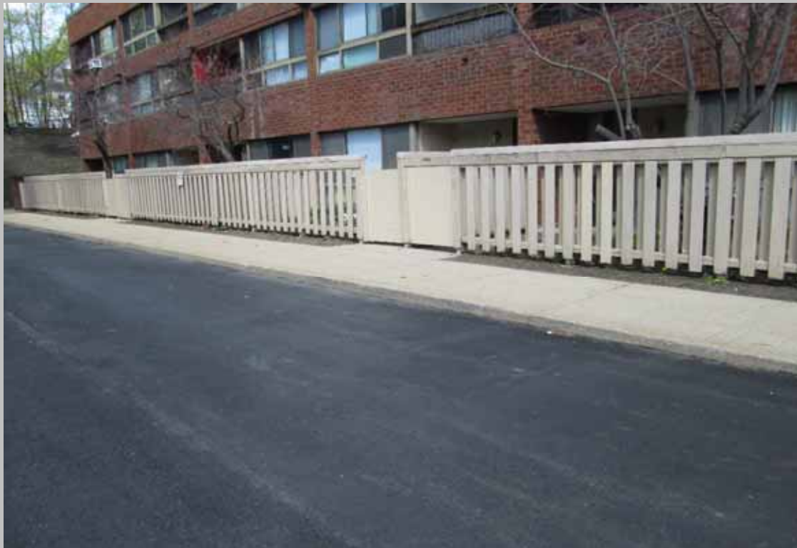
View of concrete sidewalk
