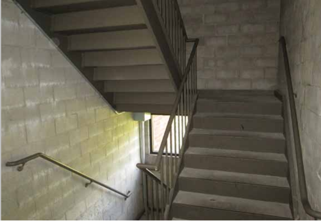
View of common interior stairwell
