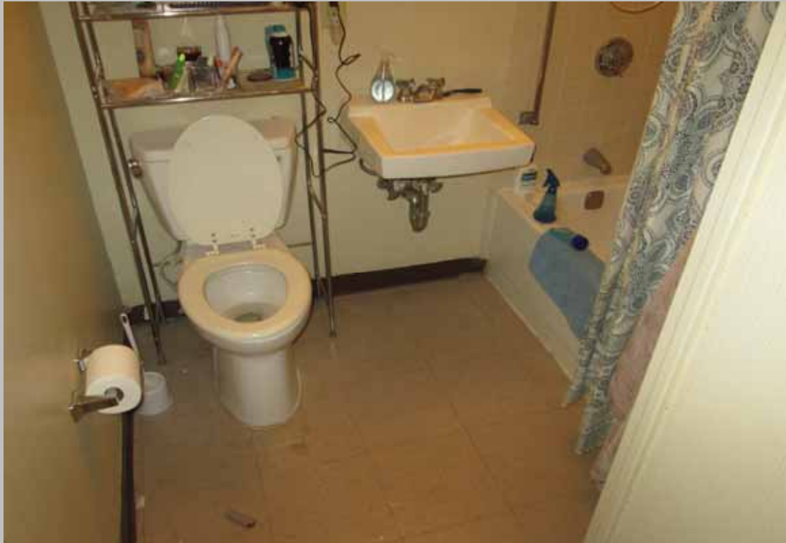
View of bathroom at Unit 106
