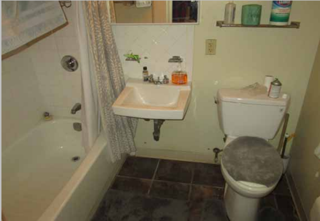
View of bathroom at Unit 109
