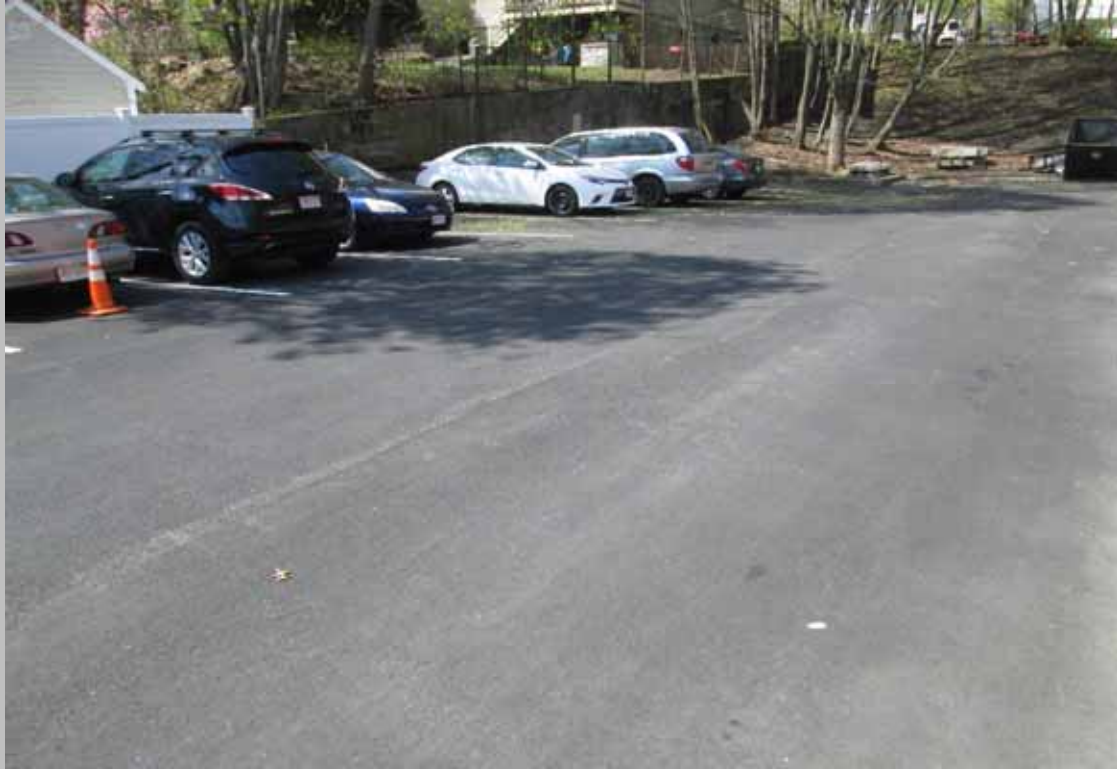
View of asphalt parking surface
