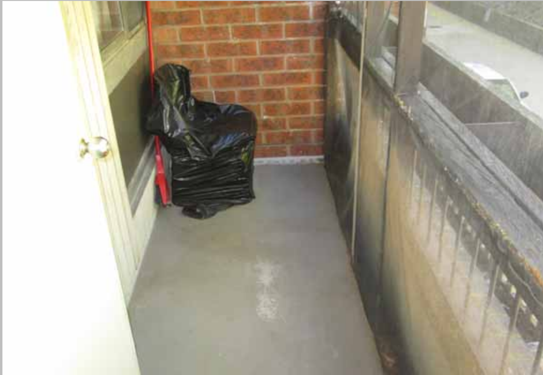
View of balcony at Unit 217
