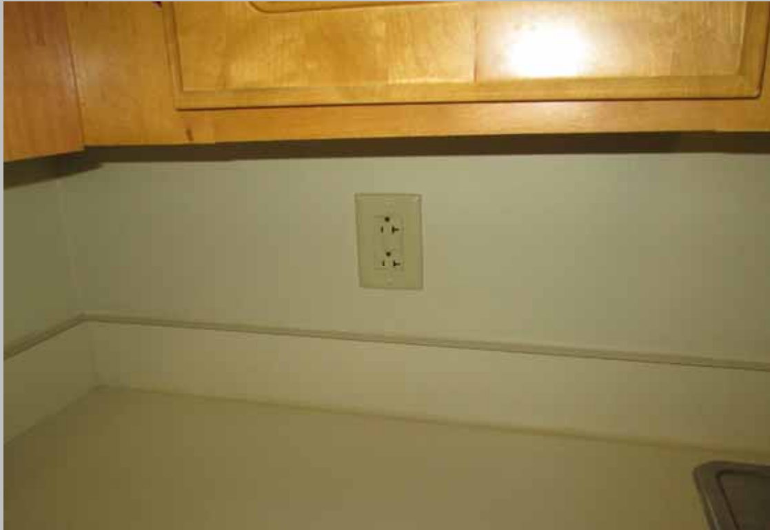
View of GFCI electrical outlet – dwelling unit
