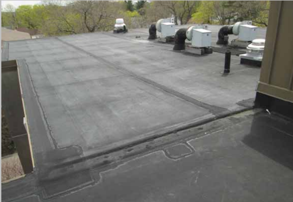
View of building roof
