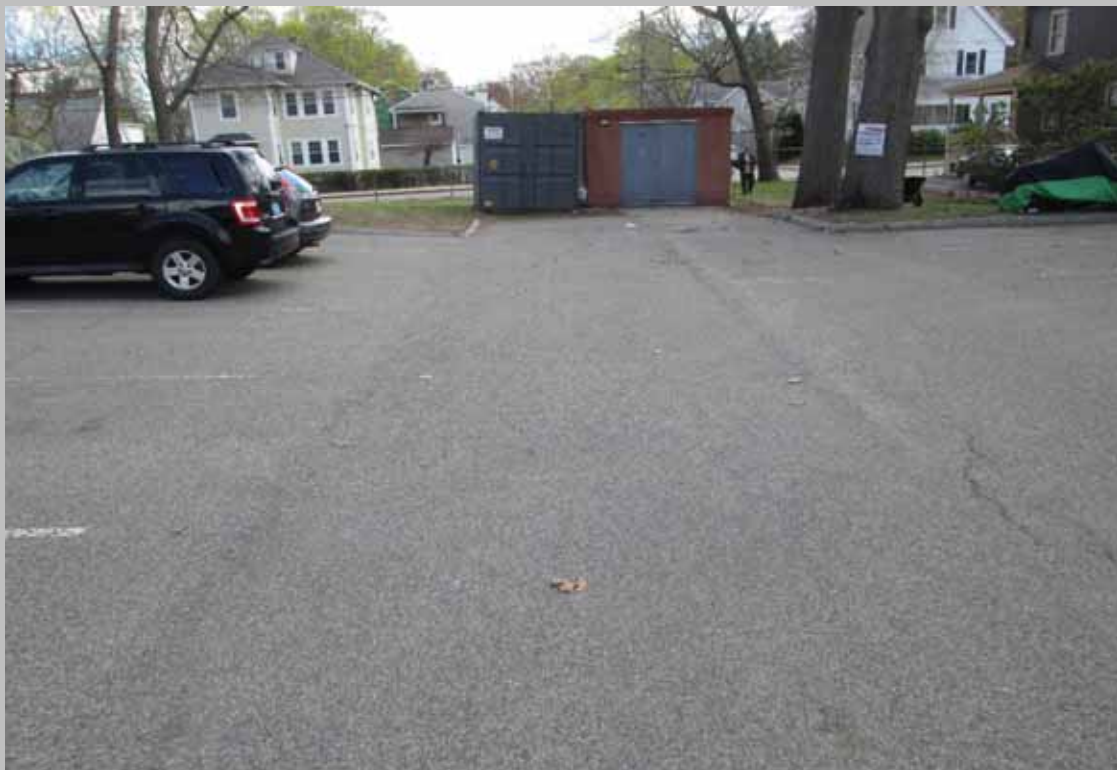
View of asphalt parking surface condition
