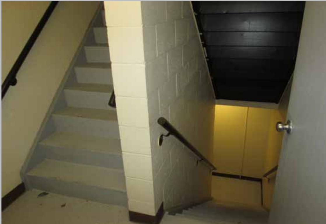
View of common interior stairwell
