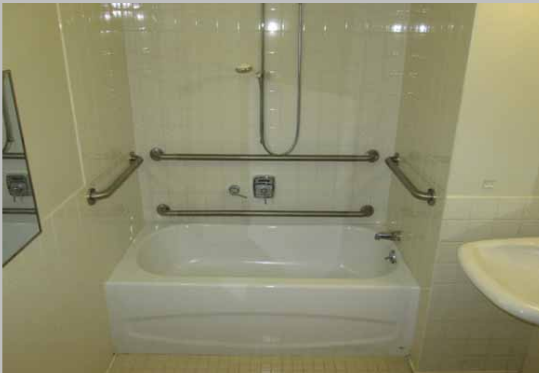
View of the shower within designated handicapped Unit 17 featuring compliant grab bars and a 60-inch shower hose
