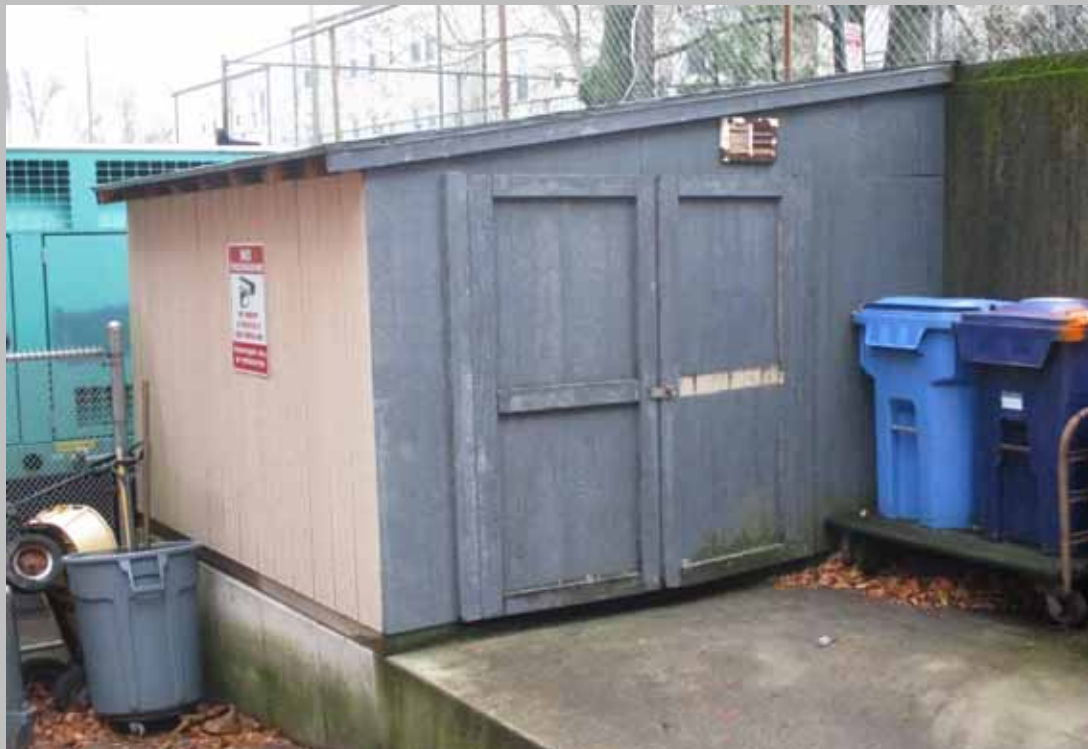
Wooden storage shed.
