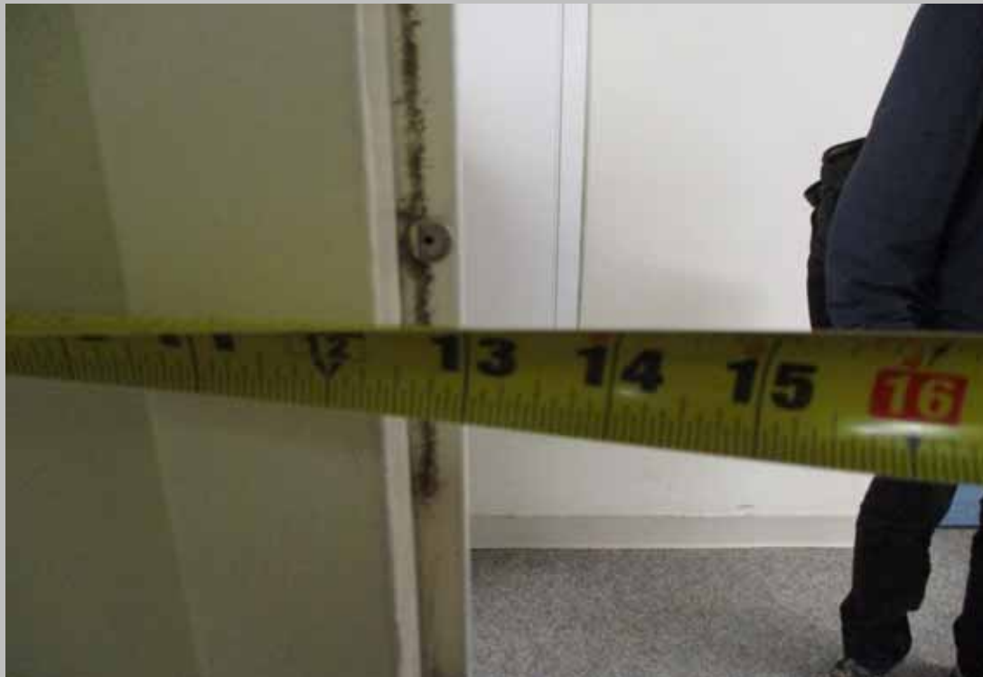
Only 12" at latch side of door.
