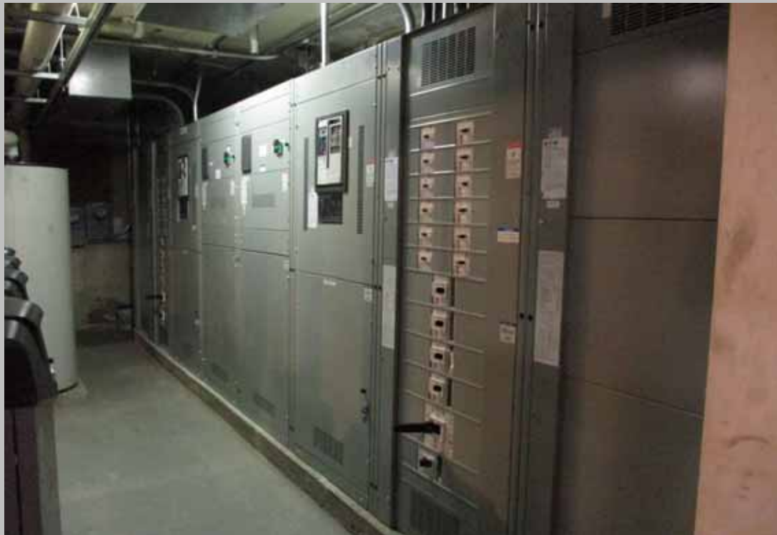
New switchgear.
