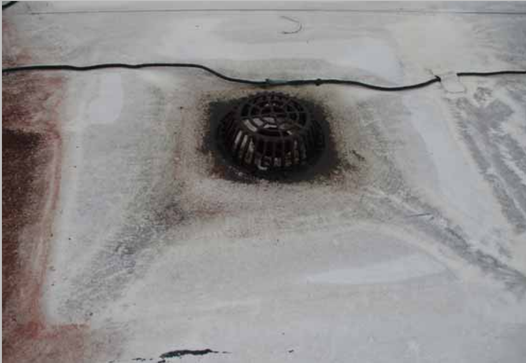
Typical roof drain.
