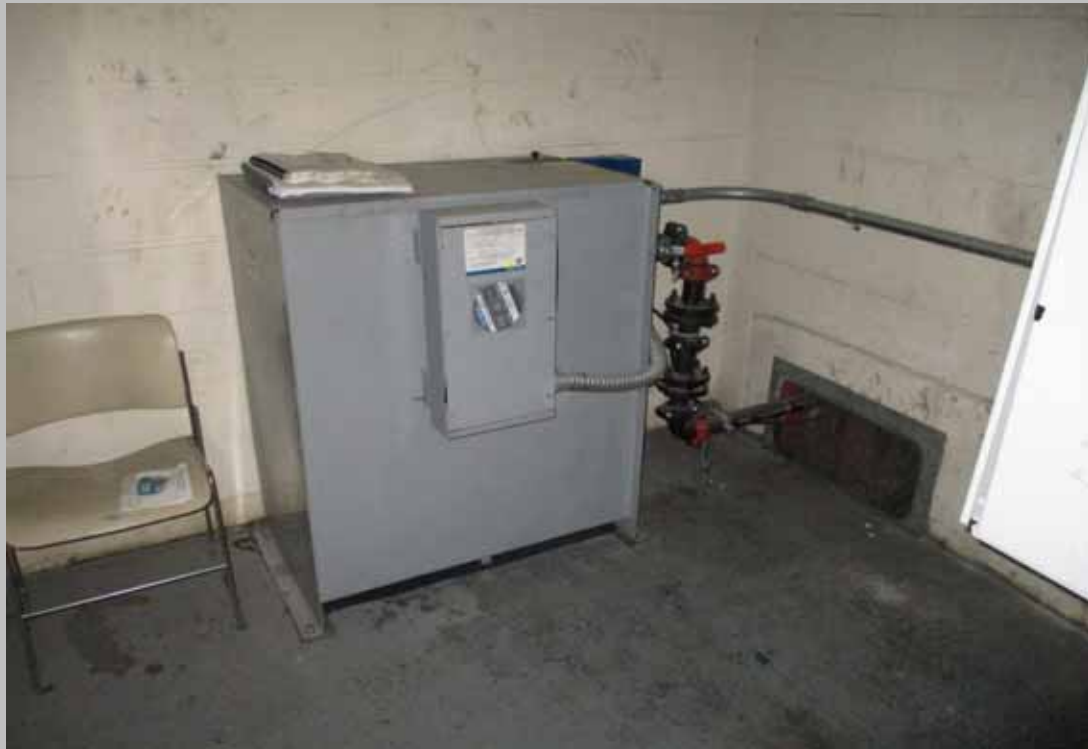
Hydraulic elevator control machinery.
