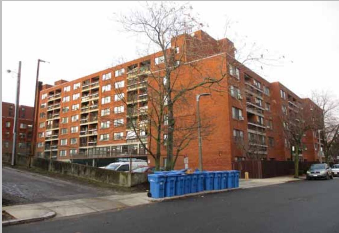
Southern and southeastern facades off Corey Road.
