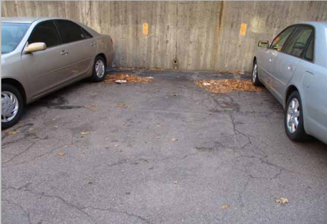
Example of faded striping.
