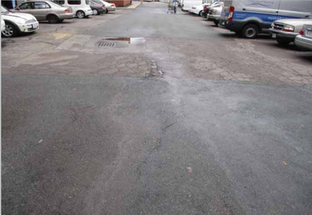
Close up of parking lot drive lane.
