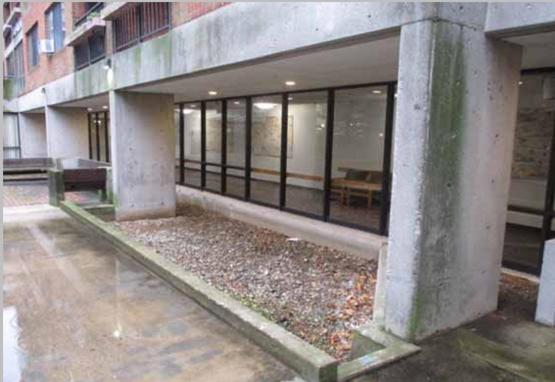
Concrete support pillars.
