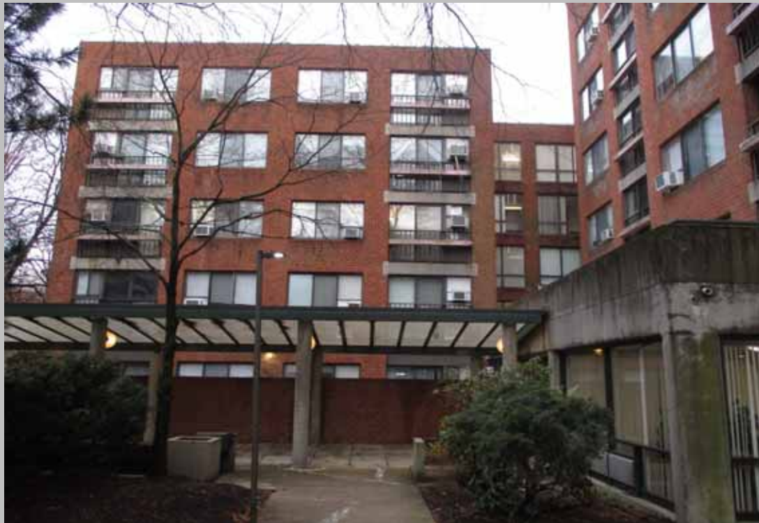
Inside portion of Corey Road portion of building.
