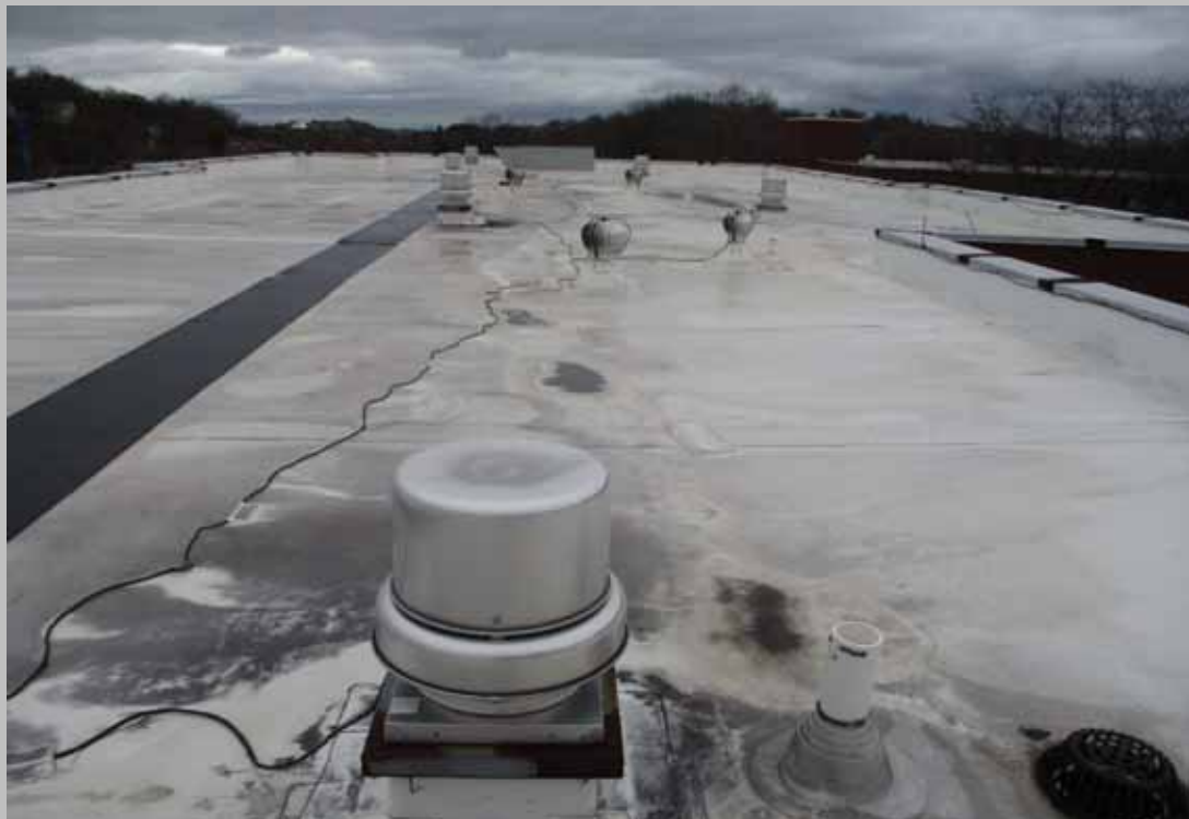
Another portion of roof.
