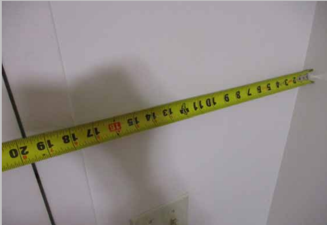
Correct latch side spacing in Unit 227.
