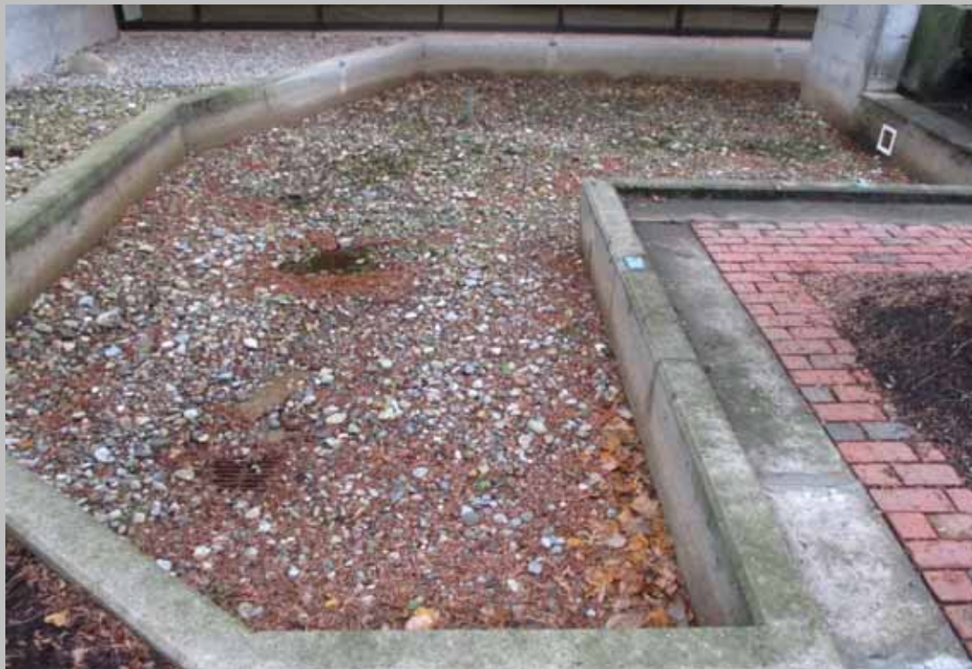
Concrete forms in courtyard.
