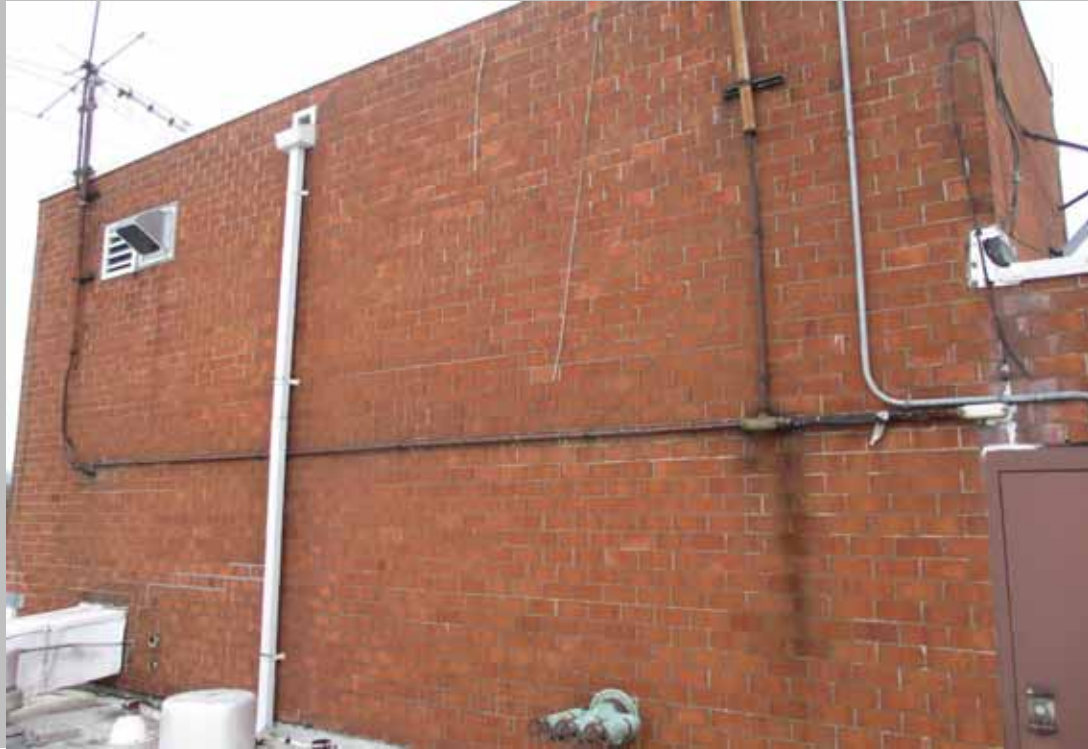
A side wall and elevator tower on roof between building sections.
