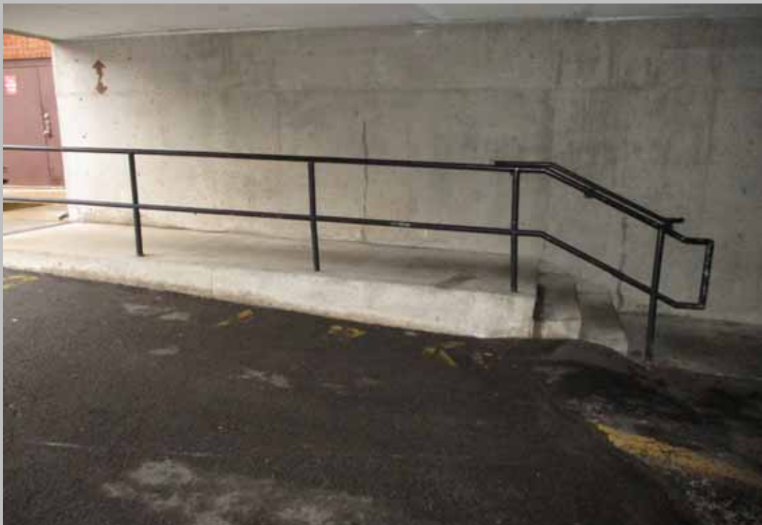
Stairs under carport leading to boiler room.
