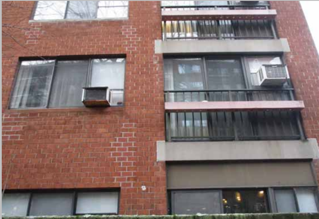
Close up of brick facades and balconies.
