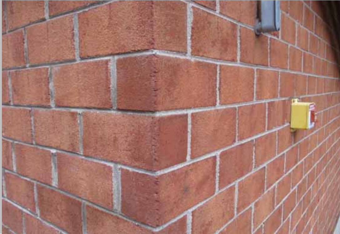
A close-up of brick façade.
