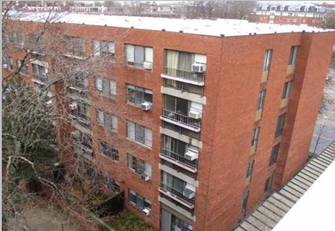
Inside portion of Washington Street portion of building.
