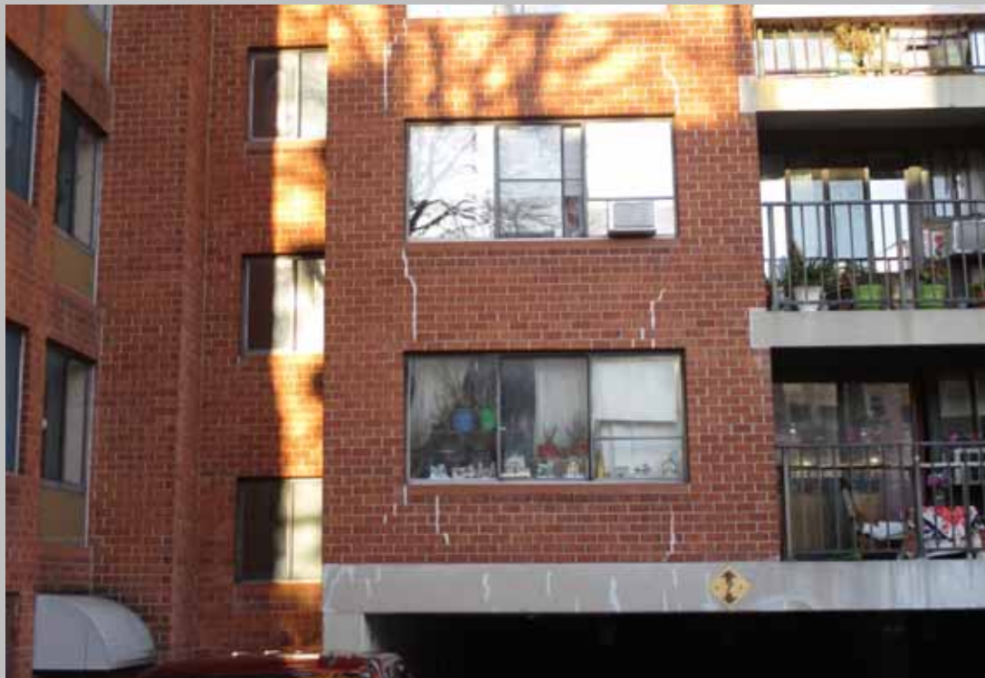
Repaired cracks in southern façade.
