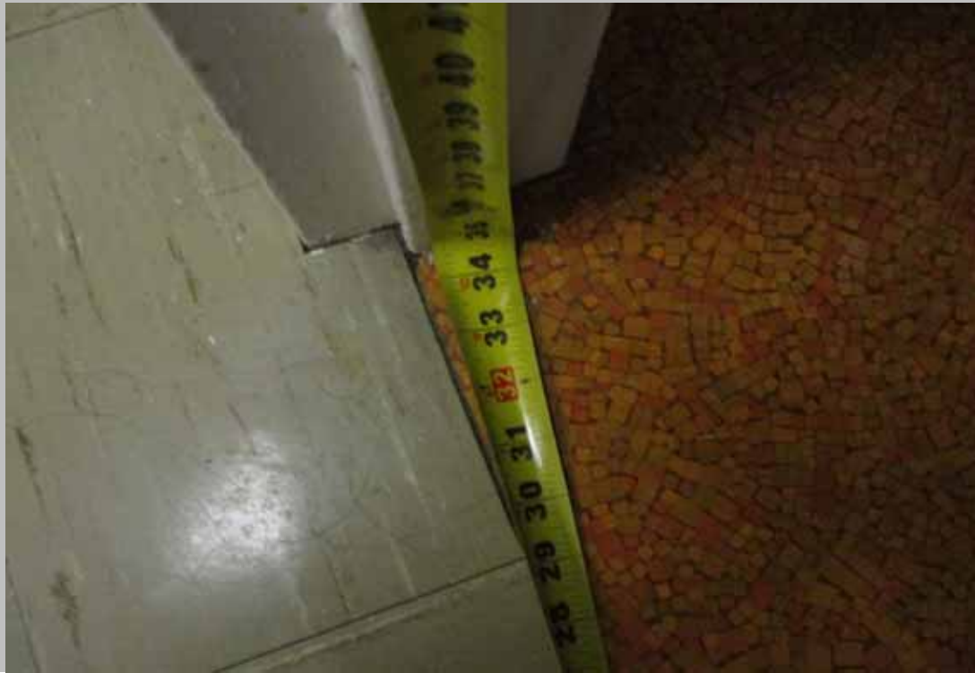
Door width into bathroom.
