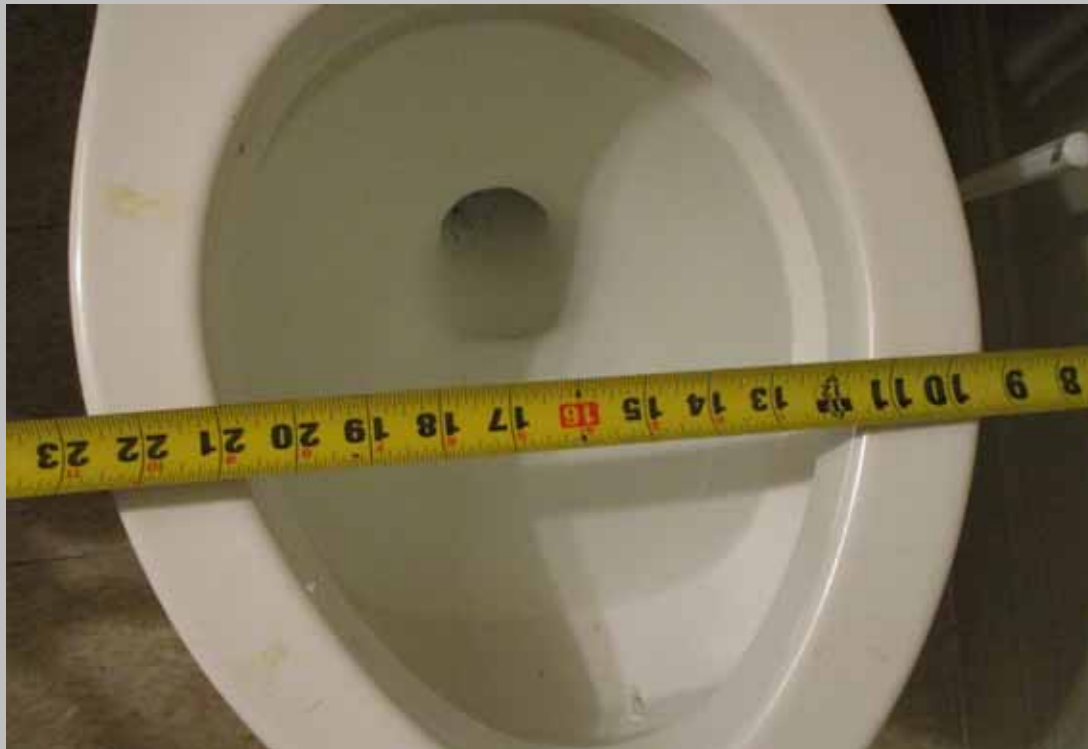
Typical toilet centering in UFAS units.
