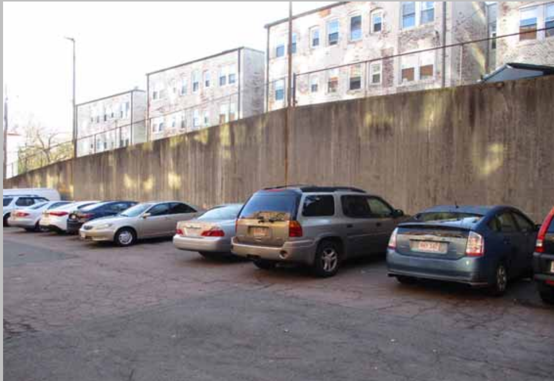
Retaining wall along parking area.
