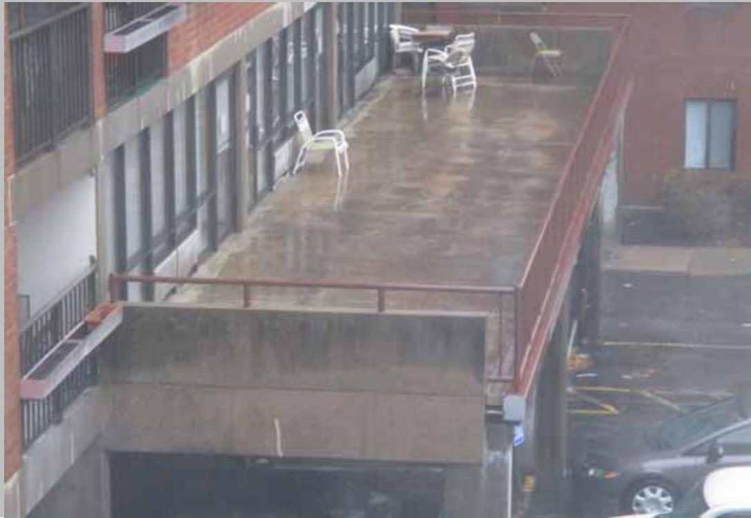
Roof deck outside community room.
