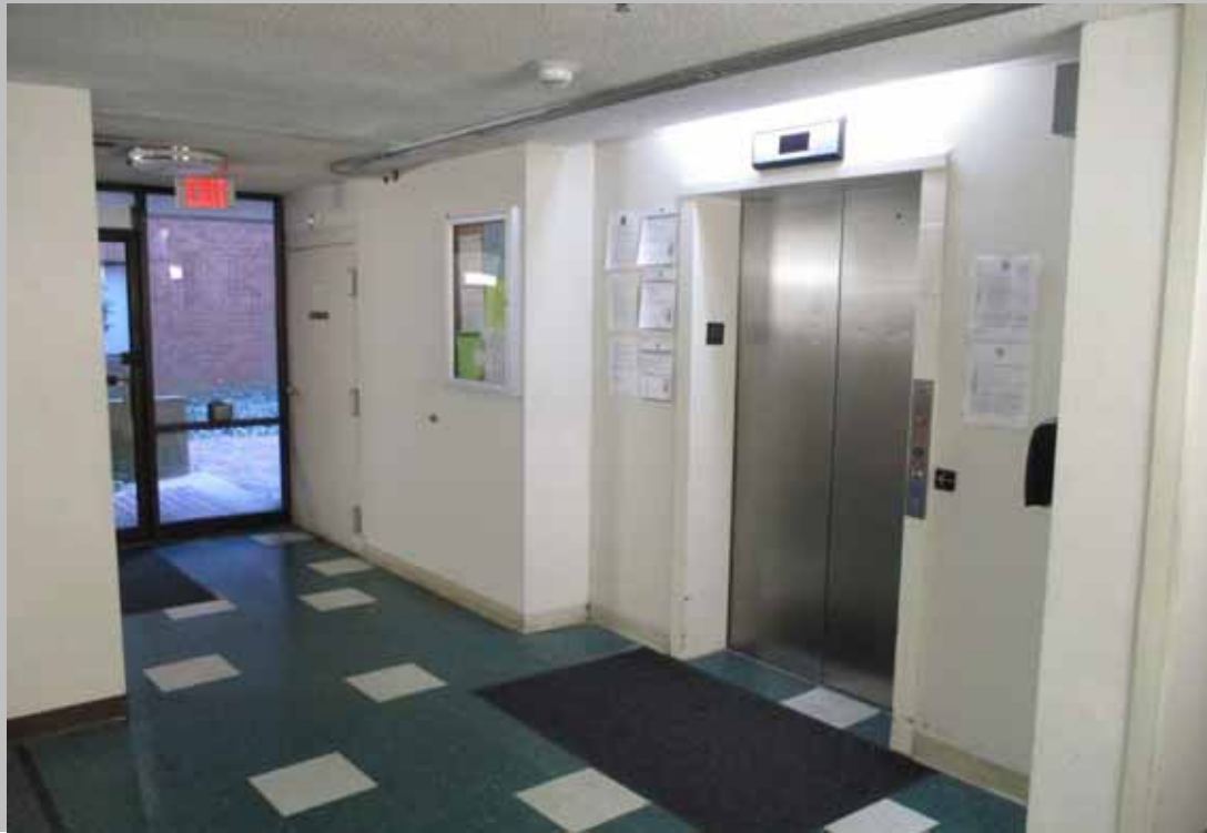
Typical elevator lobby.
