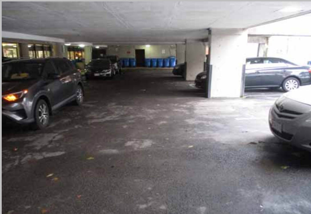
Another view under carport.
