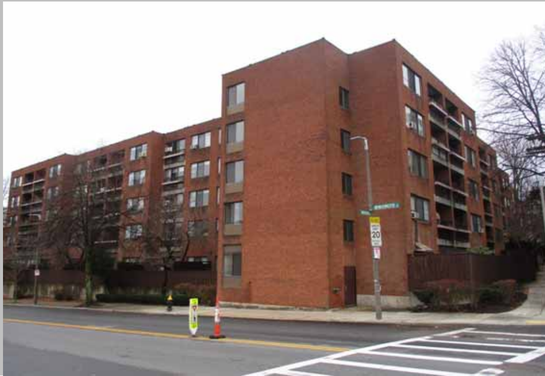
Northern façade on Washington Street.
