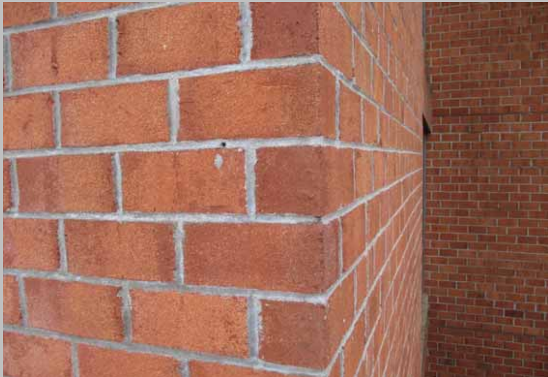
Another close-up of brick façade.
