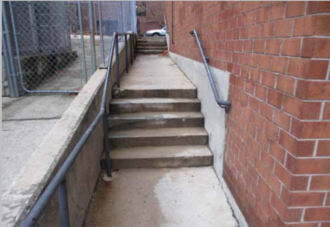
Stairs from parking lot up to Egremont Road.
