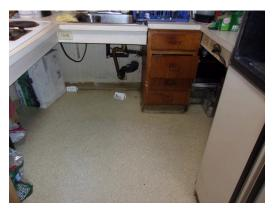
Handicapped Accessible Unit Lacking Scald And Abrasion Protection On Under Sink Piping
