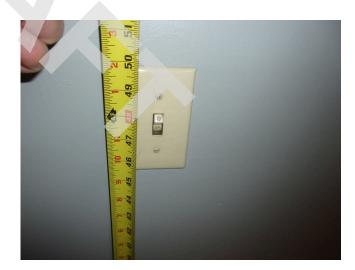
12. Community Building Restroom Light Switch Measurement From Finished Floor
