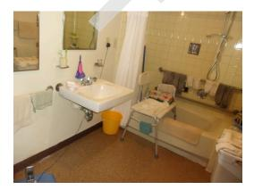
Handicapped Accessible Unit Lacking Scald And Abrasion Protection On Under Sink Piping
