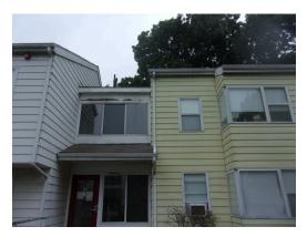
Damaged Fascia (Non-Critical Repair)
