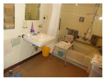
78. Handicapped Accessible Unit Lacking Scald And Abrasion Protection On Under Sink Piping
