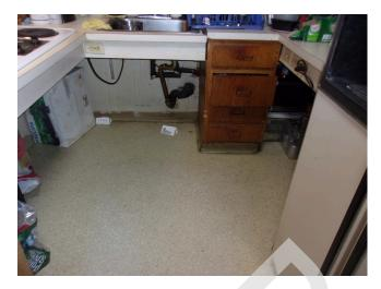
81. Handicapped Accessible Unit Lacking Scald And Abrasion Protection On Under Sink Piping
