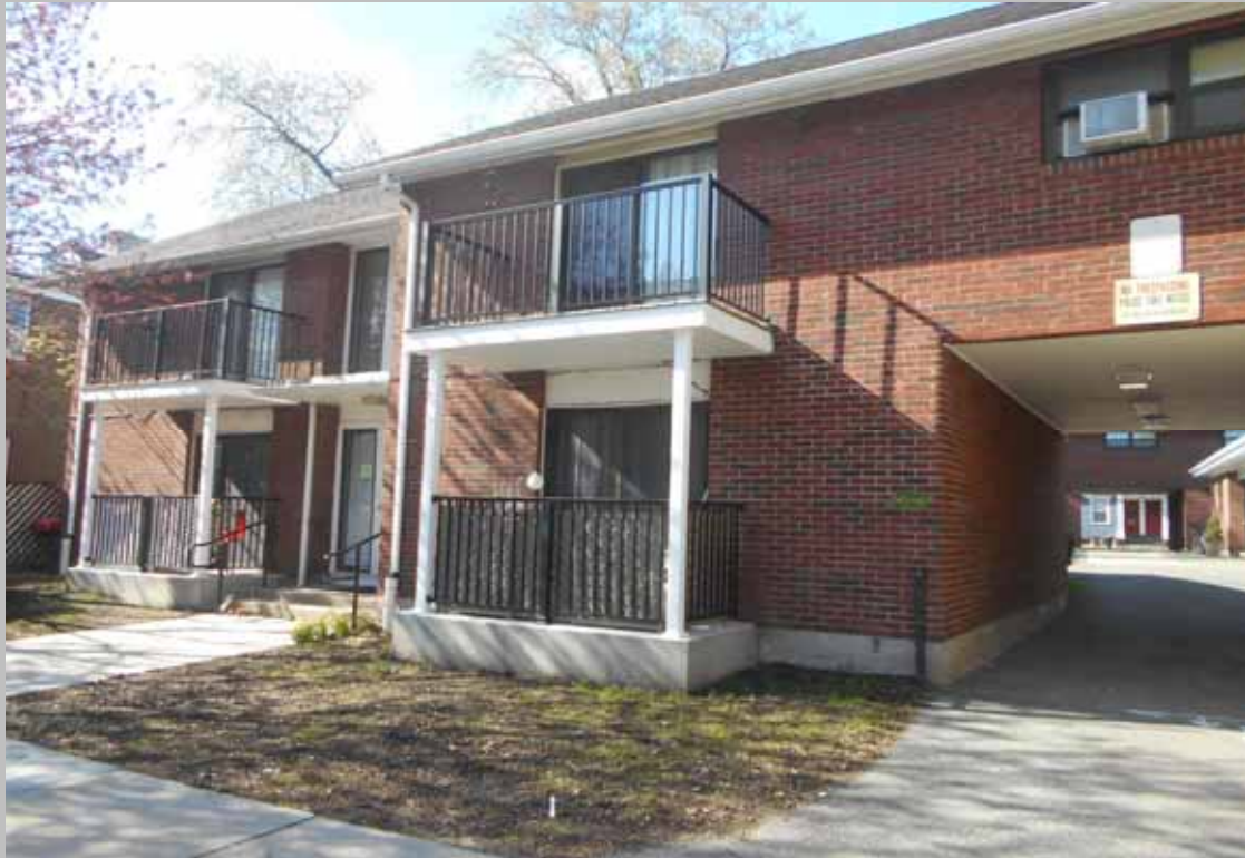
Building exterior - typical front elevation
