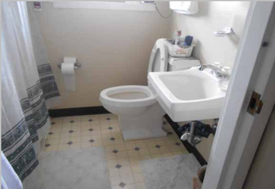
1-bedroom dwelling unit – typical bathroom
