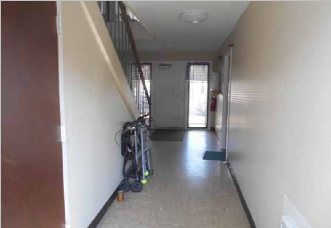
Typical common hallway (apartment buildings)
