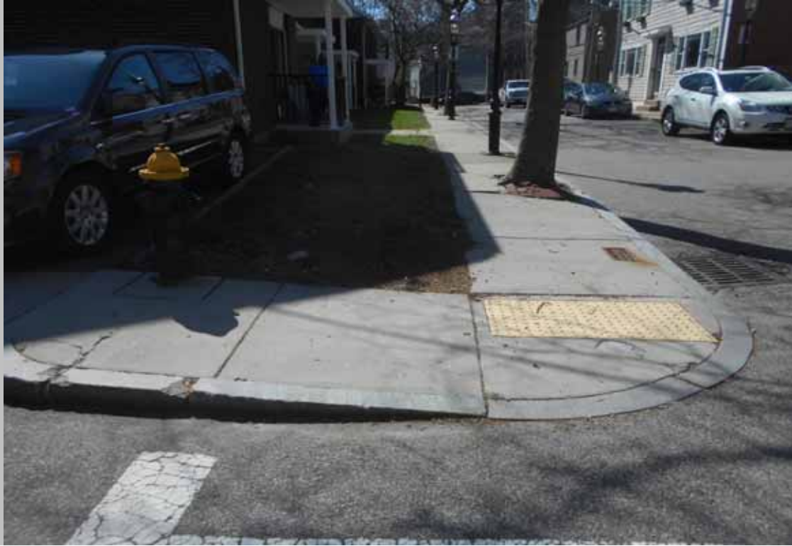
Typical municipal sidewalk
