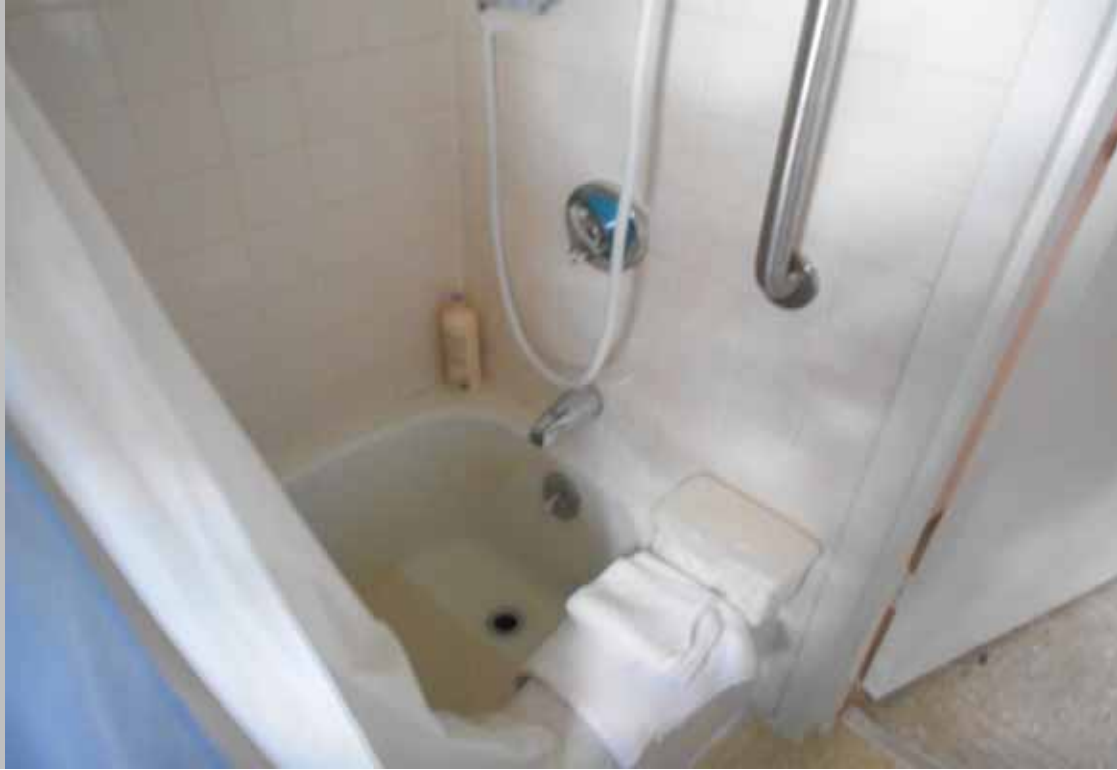
2-bedroom dwelling unit – typical bathtub/shower
