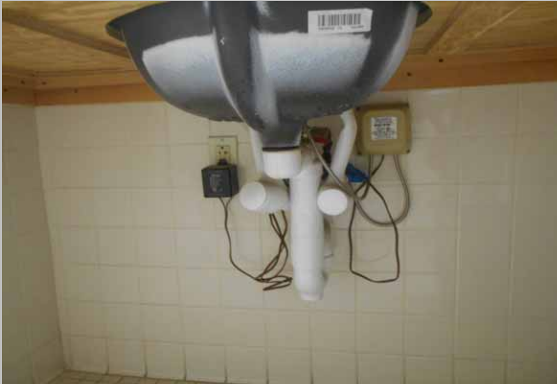
Roll-under sink with scald and abrasion protection – common area public unisex restroom (Compliant, UFAS)
