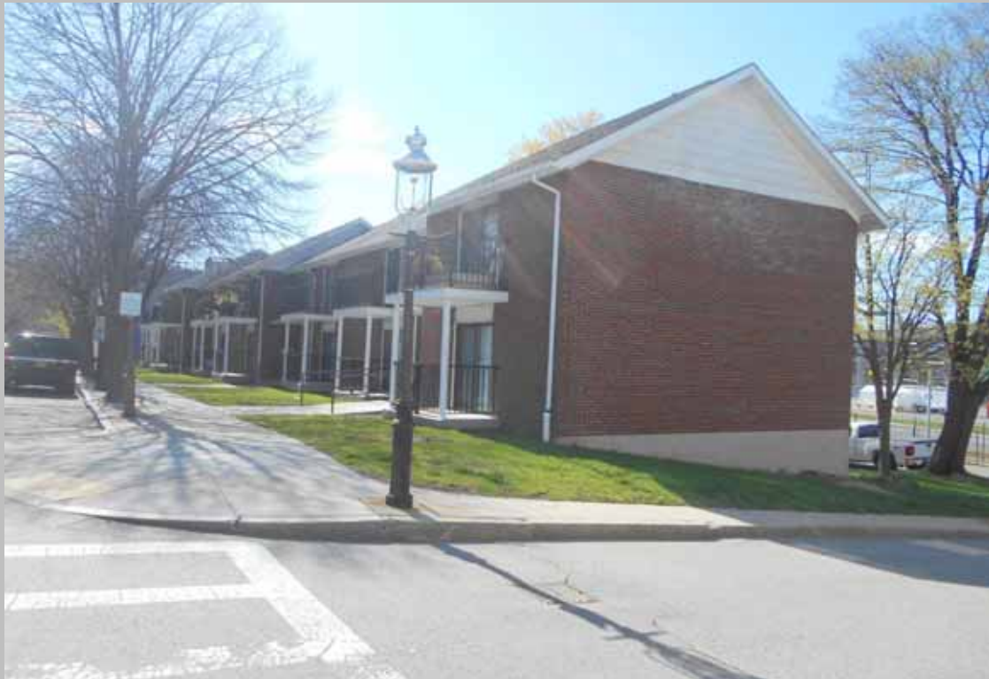
Building exterior (with crawl space) – front elevation
