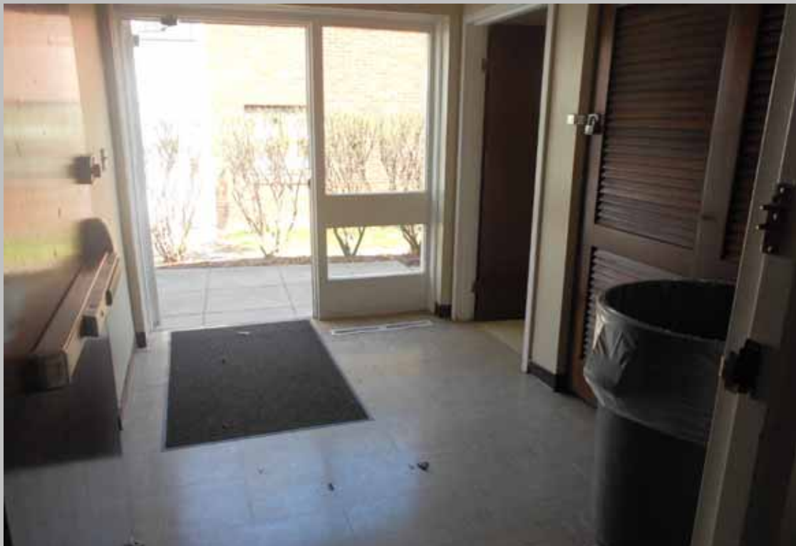
Accessible route at Community Building 1 entrance (Compliant, UFAS)
