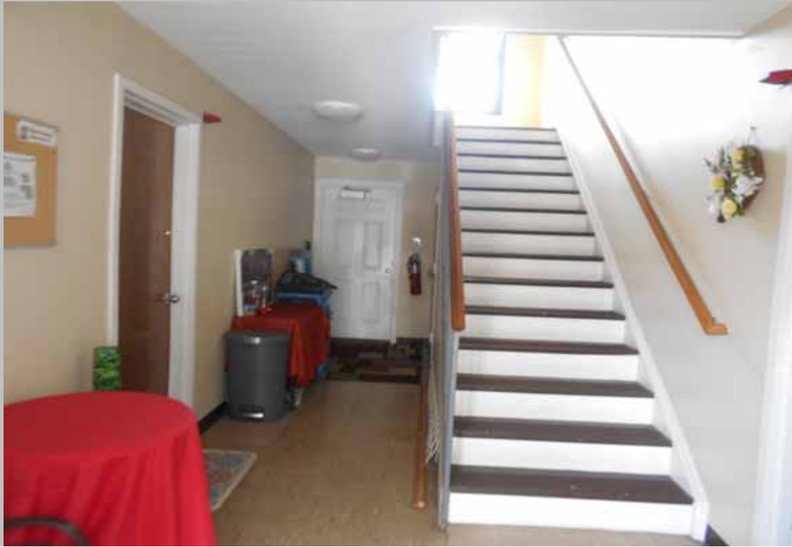
Common interior stairwell (apartment buildings)
