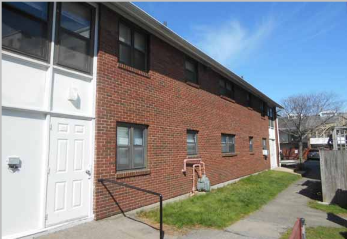
Typical asphalt sidewalks
