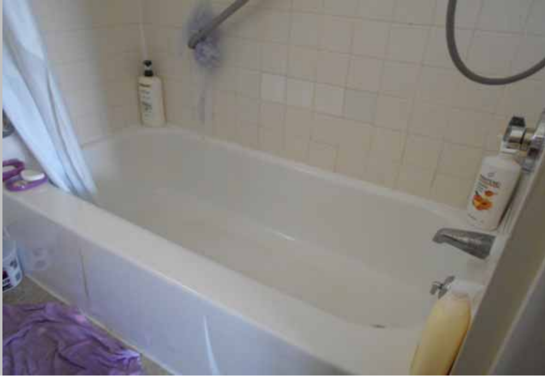
1-bedroom dwelling unit – typical bathtub/shower
