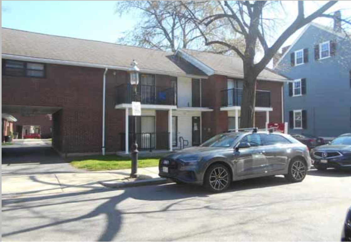
Leasing/Management Office primary entrance (47 Washington Street)
