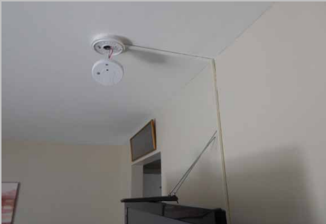
Typical hardwired smoke alarm (dwelling units)
