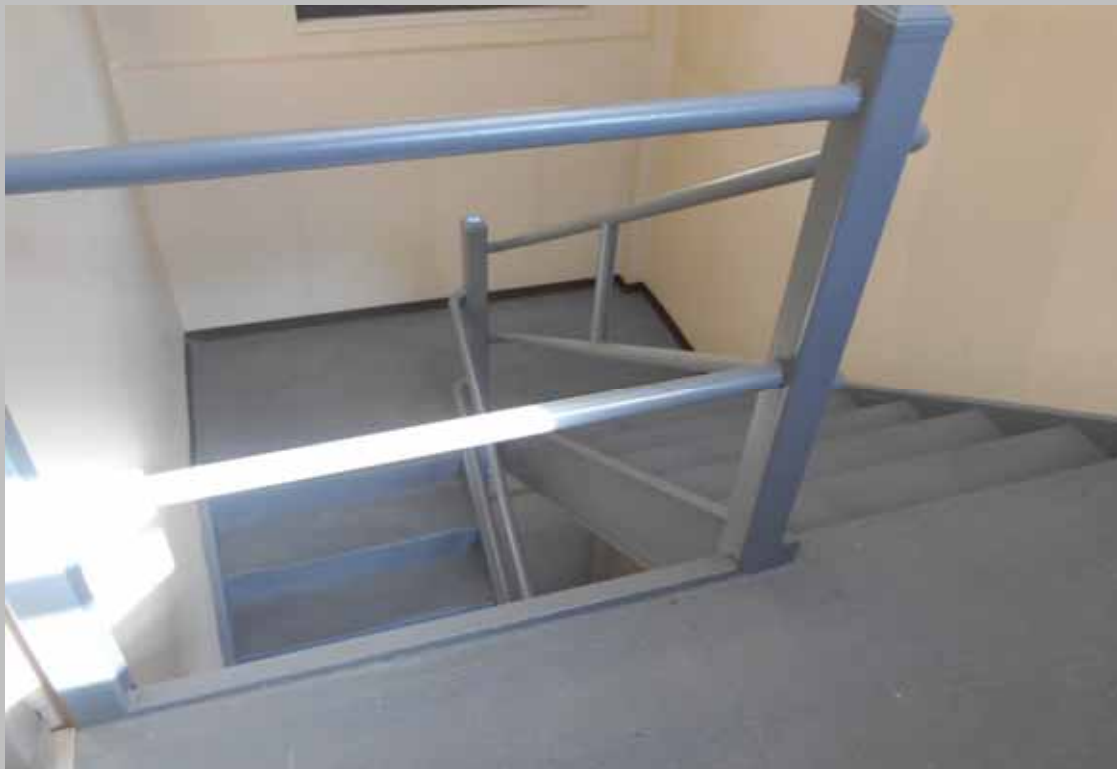
View of interior stairwell leading to the roof access
