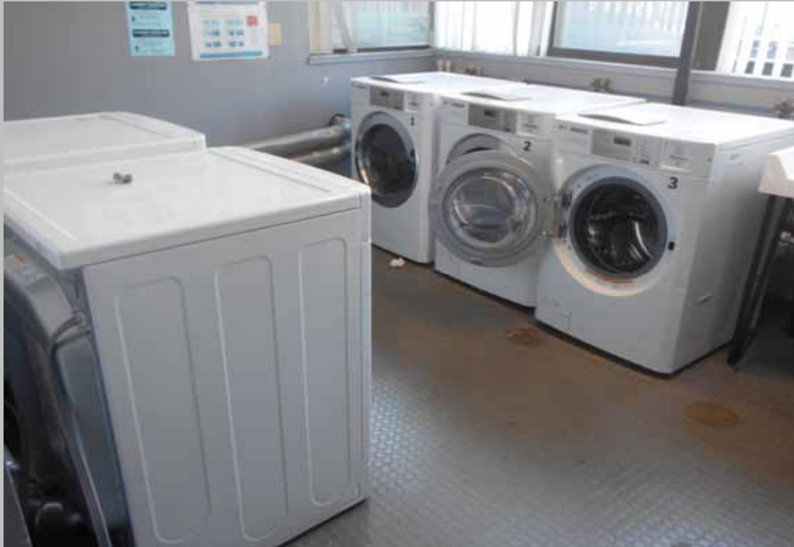
View of the laundry room
