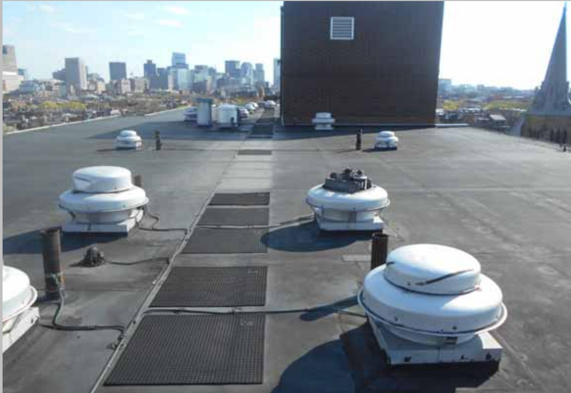
View of building roof
