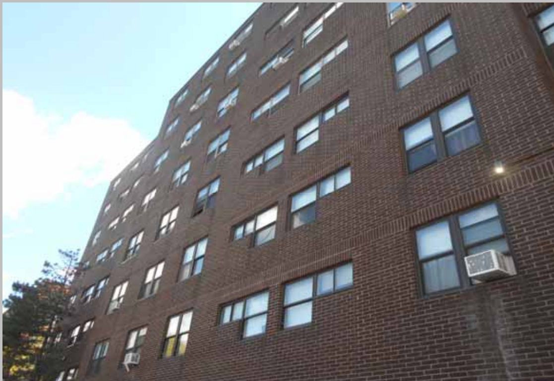
View of building exterior
