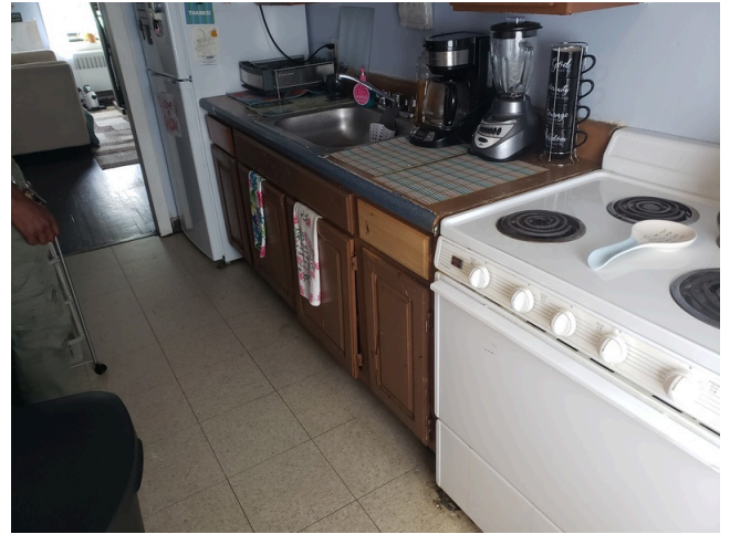
106. Dwelling Unit Interior Elements: Typical vinyl flooring and sheetrock finish found in dwelling units throughout the site.
