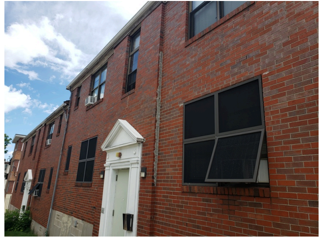
58. Sidewall System: Building 1 west facade.
