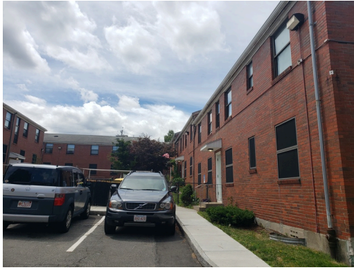
Stormwater Drainage: Typical downspout found throughout site.
