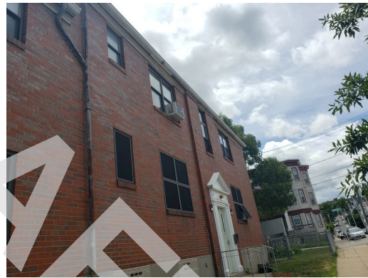
Roofing Finish: Typical gutters and downspouts found throughout the site.
