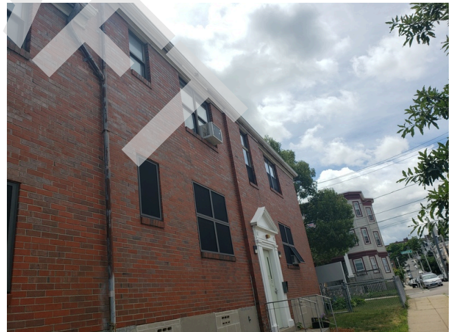
72. Roofing Finish: Typical gutters and downspouts found throughout the site.
