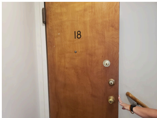
Exterior Doors & Entry Systems: Typical unit door found throughout the site.
