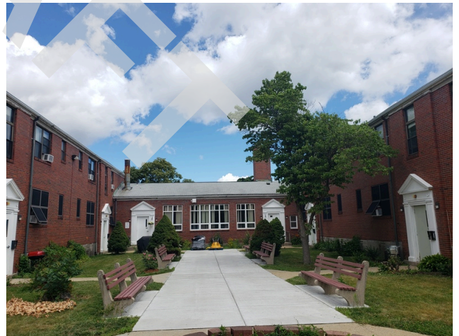
16. Flatwork (Walks, Plazas, Terraces, Patios): Typical concrete sidewalks found at the property.
