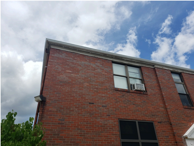
23. Landscaping & Appurtenances: Typical parking area lighting found throughout the property.
