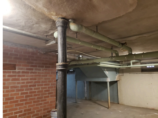
Foundation: Typical basement found throughout the site.
