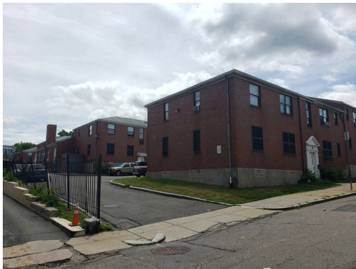
Sidewall System: Building 1 northwest corner facade.
