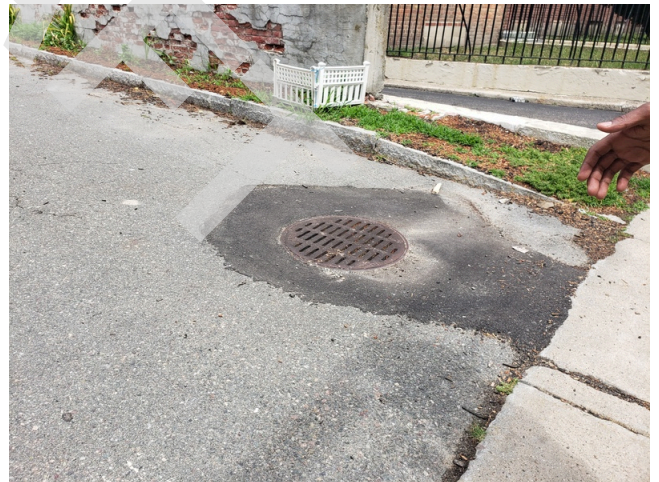
4. Stormwater Drainage: Typical paving drainage found throughout site.
