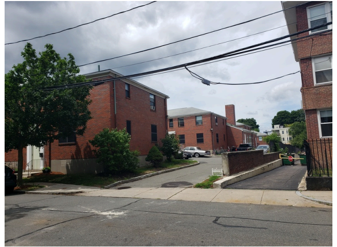
50. Sidewall System: Building 2 northeast corner facade.
