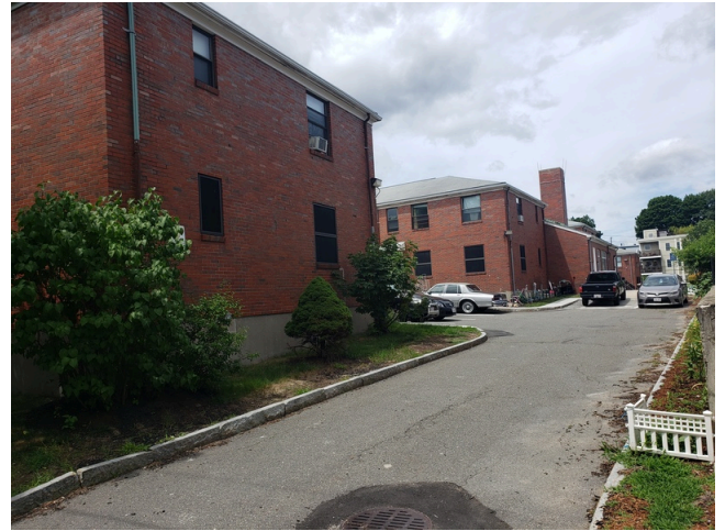
10. Paving, Curbing, & Parking: Typical concrete curbing found throughout the site.
