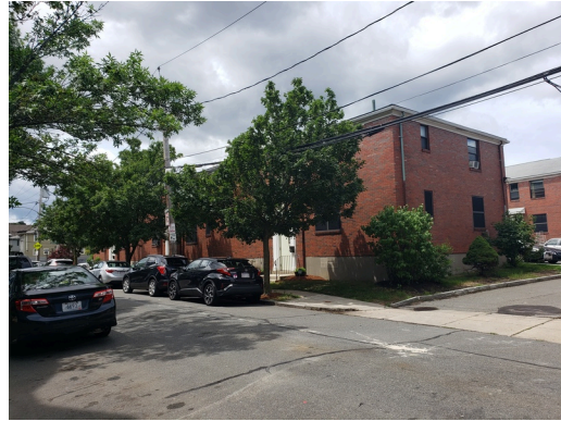
Sidewall System: Building 2 east facade.
