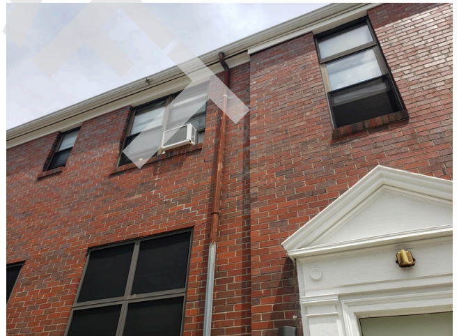
44. Sidewall System: Typical sidewall unpainted brick found throughout the site.
