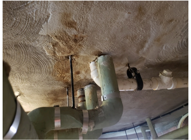
74. Plumbing: Typical cast iron and PVC waste pipes found throughout the property.
