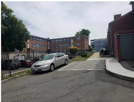
Paving, Curbing, & Parking: Typical accessible parking spaces found throughout the property.
