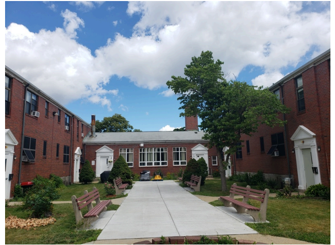
70. Roofing Finish: Typical asphalt shingle roofing found throughout the site.
