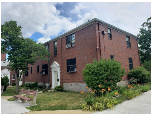
Sidewall System: Building 3 northwest corner facade.
