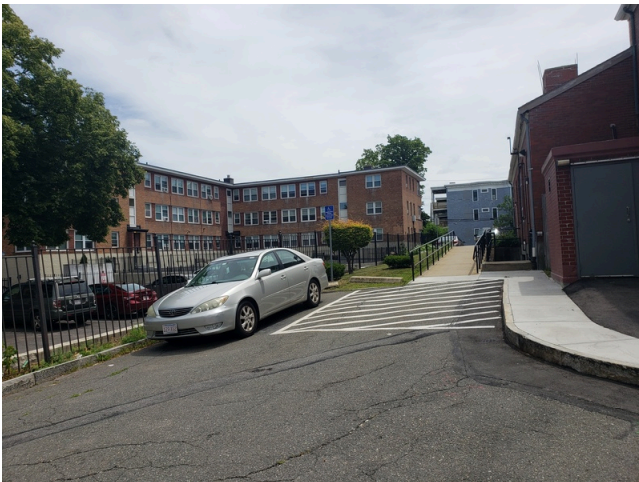
11. Paving, Curbing, & Parking: Typical accessible parking spaces found throughout the property.
