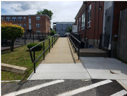
Flatwork (Walks, Plazas, Terraces, Patios): Poured in place concrete ramp and sidewalks found at the property.
