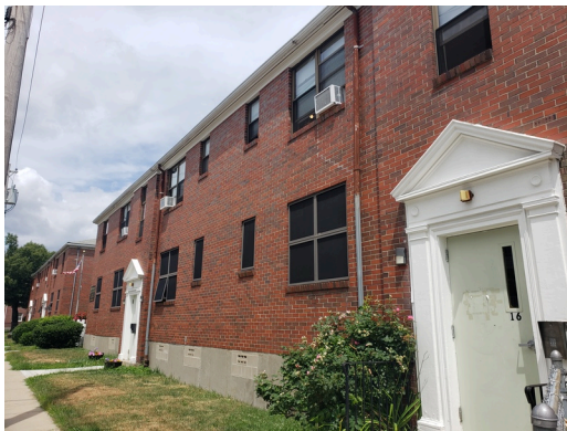
Sidewall System: Typical sidewall unpainted brick found throughout the site.
