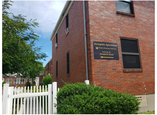
54. Sidewall System: Building 2 southwest corner facade.
