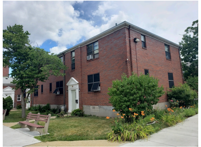
66. Sidewall System: Building 3 northwest corner facade.
