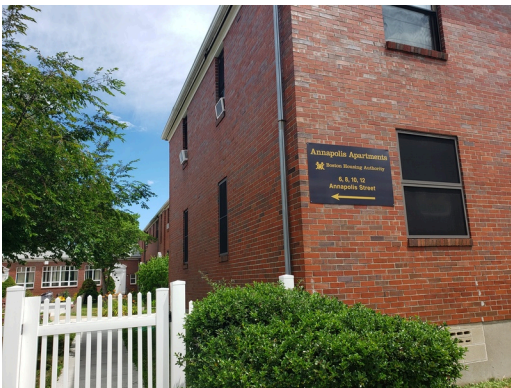
Sidewall System: Building 2 southwest corner facade.
