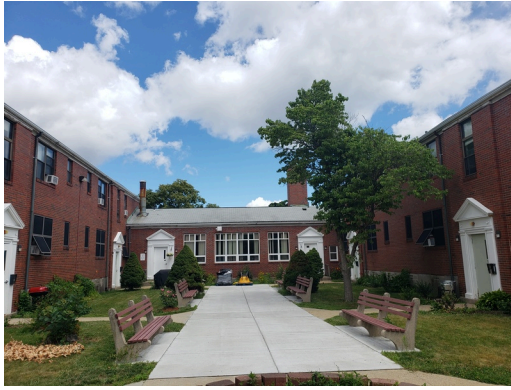
Flatwork (Walks, Plazas, Terraces, Patios): Typical concrete sidewalks found at the property.
