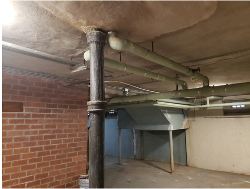
Foundation: Typical basement found throughout the site.
