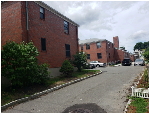
Access & Egress: West access drive to the property.
