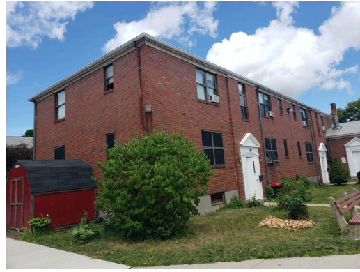
Sidewall System: Building 3 southwest corner facade.
