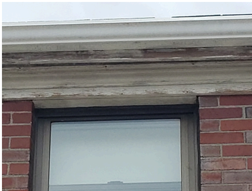
Attics & Eaves: Typical perforated eaves vents found throughout the site (Non-Critical Repair)
