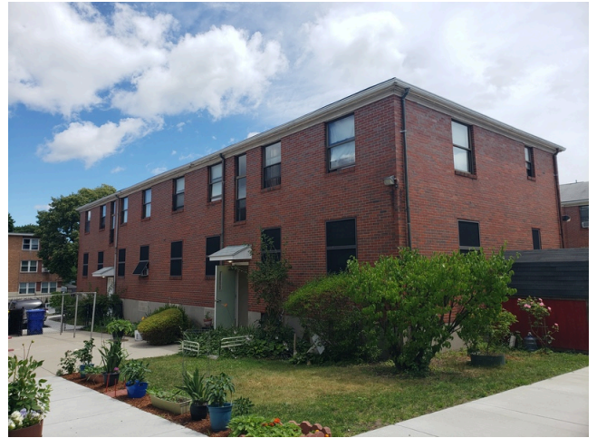
62. Sidewall System: Building 3 southwest corner facade.
