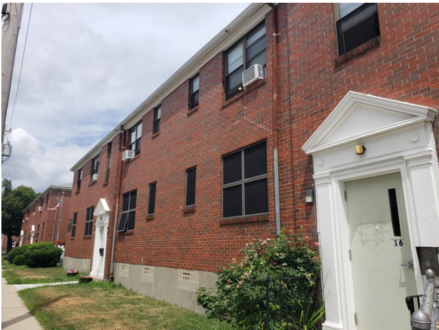
43. Sidewall System: Typical sidewall unpainted brick found throughout the site.
