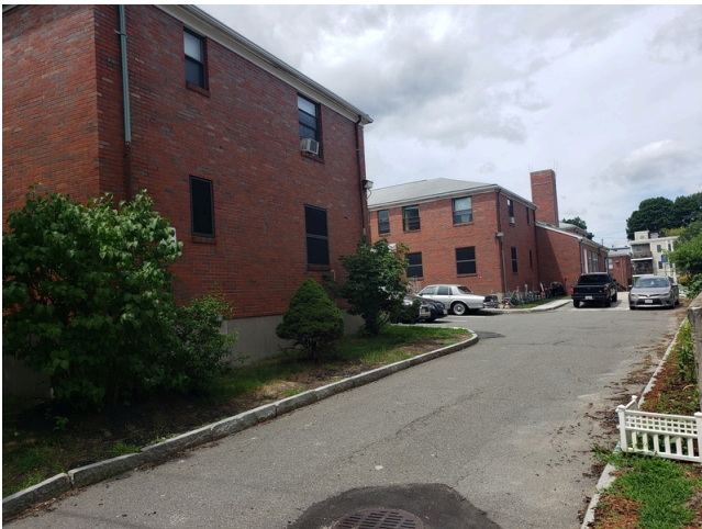
7. Access & Egress: West access drive to the property.
