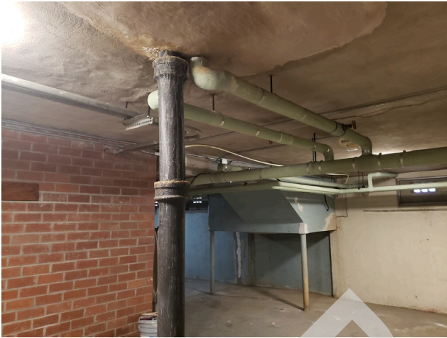
73. Plumbing: Typical cast iron and PVC waste pipes found throughout the property.
