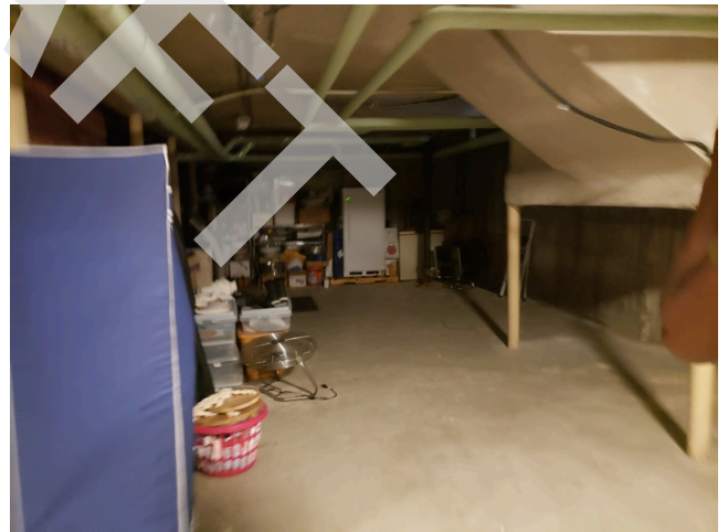
32. Foundation: Typical basement found throughout the site.
