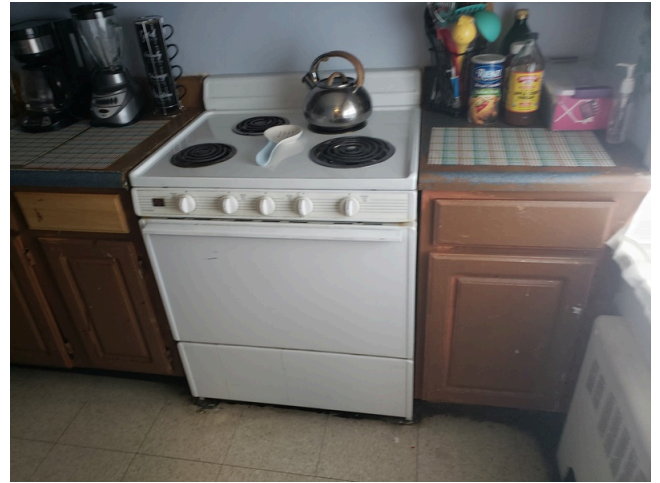
122. Appliances: Typical range found throughout the site.
