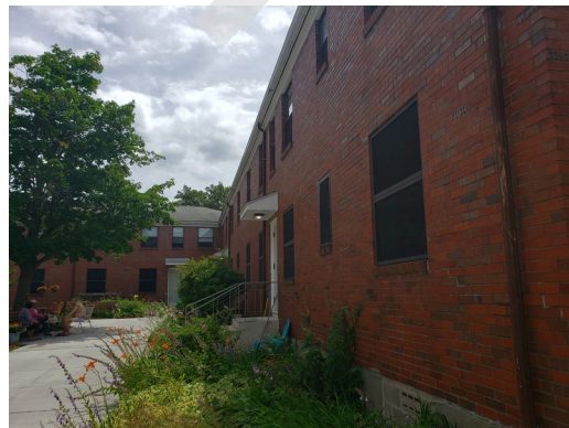
Sidewall System: Building 2 west internal facade.
