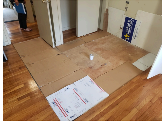
Dwelling Unit Interior Elements: Removed flooring and finishes due to decomposing body removal. (Critical Repair)
