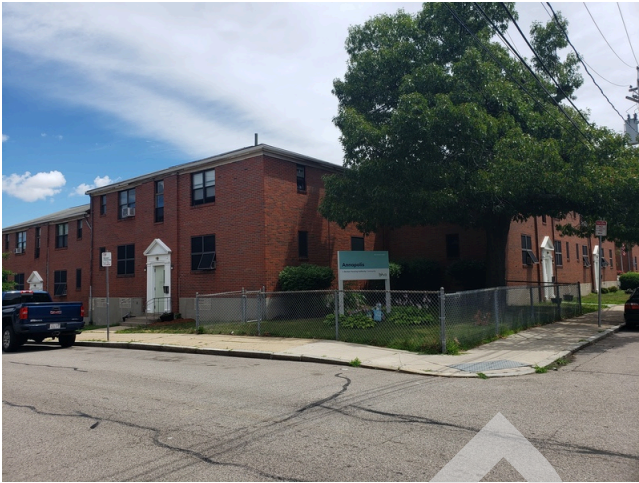
57. Sidewall System: Building 1 southwest corner facade.
