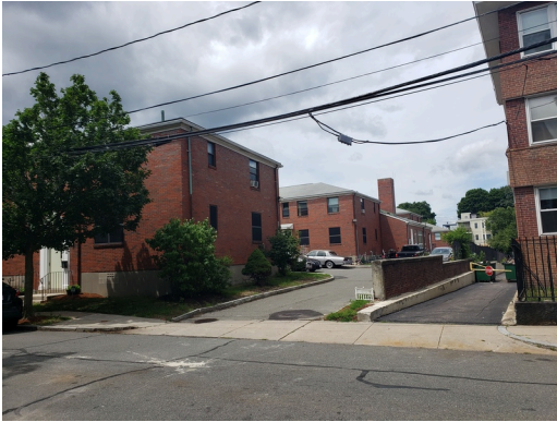
Sidewall System: Building 2 northeast corner facade.
