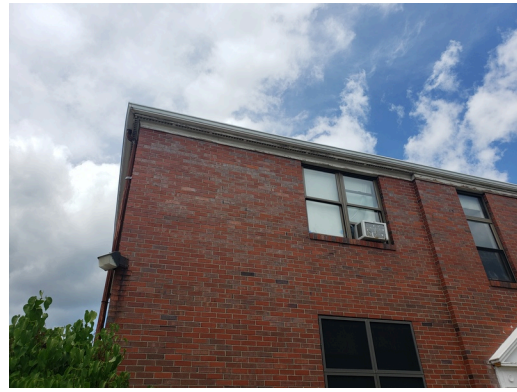
Landscaping & Appurtenances: Typical parking area lighting found throughout the property.
