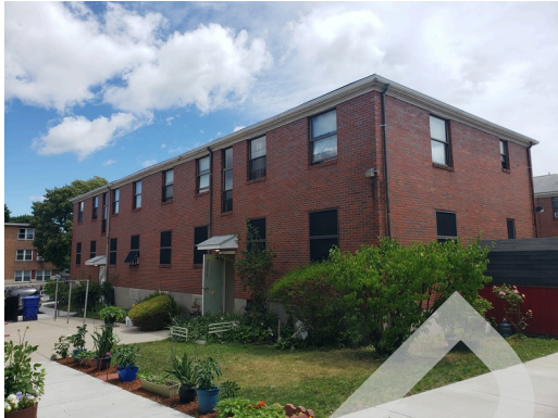
Windows: Typical single-hung style double-pane aluminum windows found throughout the site.
