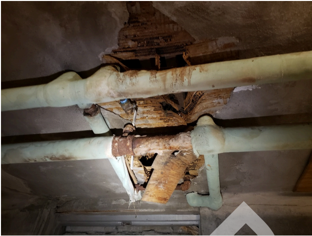
29. Foundation: Typical cracks on basement walls and ceilings found throughout the site. (Critical Repair)
