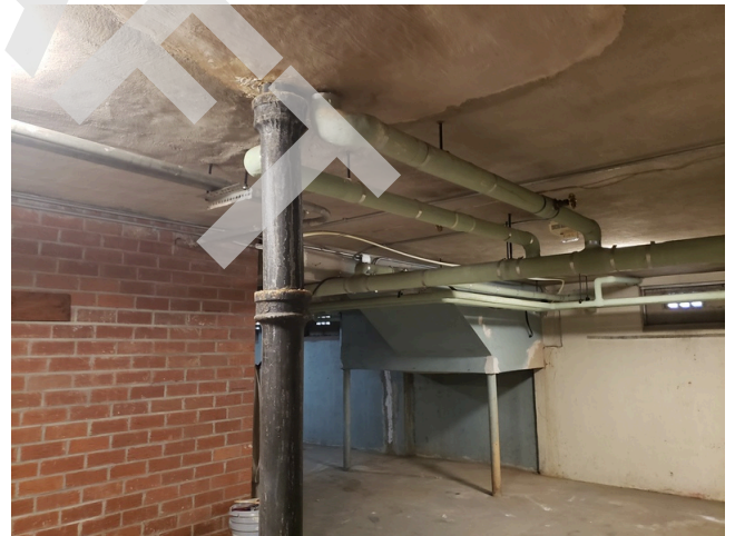
28. Foundation: Typical basement found throughout the site.
