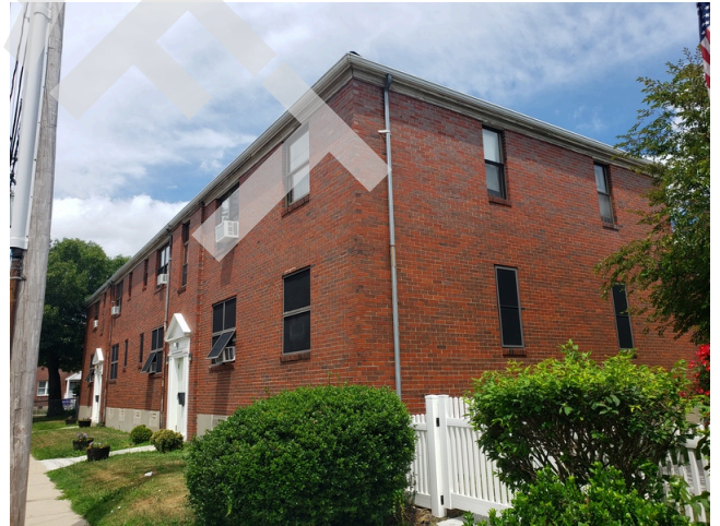
56. Sidewall System: Building 1 southeast corner facade.
