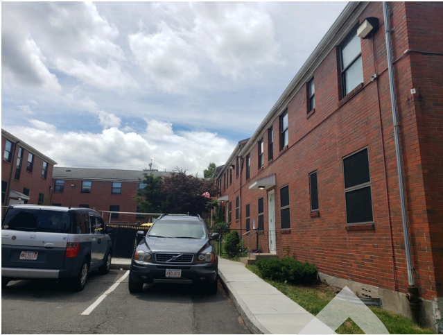
61. Sidewall System: Building 1 northeast internal corner facade.
