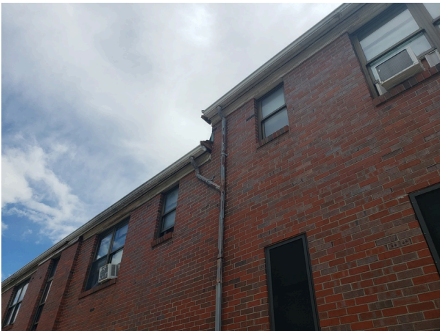
71. Roofing Finish: Typical gutters and downspouts found throughout the site.
