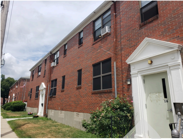
53. Sidewall System: Building 2 south facade.
