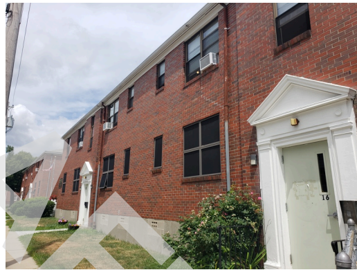
Sidewall System: Building 2 south facade.
