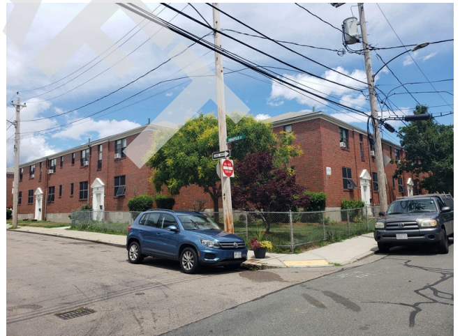
52. Sidewall System: Building 2 southeast corner facade.
