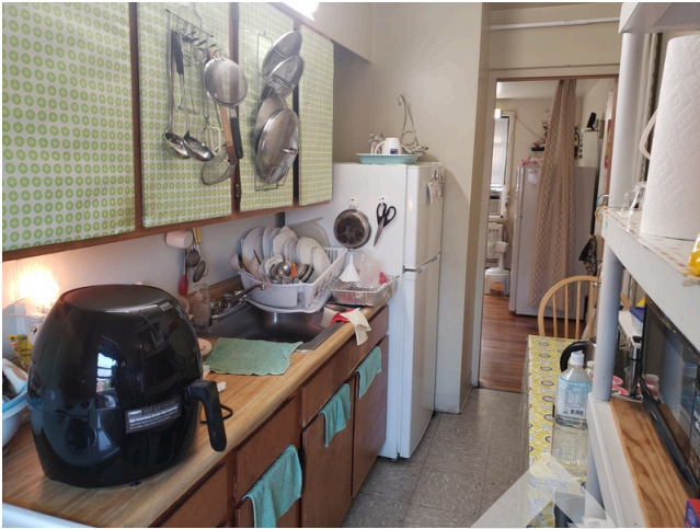
125. Cabinets & Fixtures: Typical dwelling unit kitchen sink, countertop, and wood cabinets found throughout the site.
