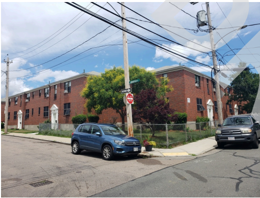
Sidewall System: Building 2 southeast corner facade.
