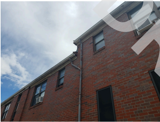
Roofing Finish: Typical gutters and downspouts found throughout the site.
