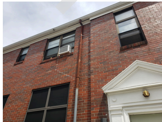
Sidewall System: Typical sidewall unpainted brick found throughout the site.
