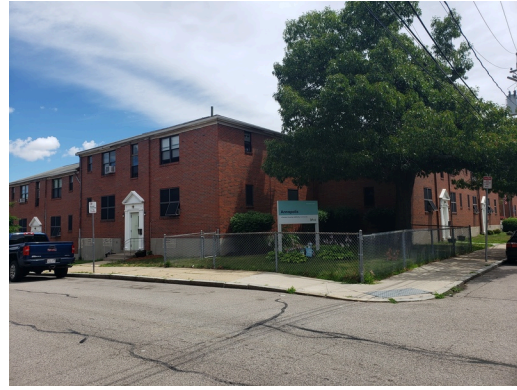
Sidewall System: Building 1 southwest corner facade.
