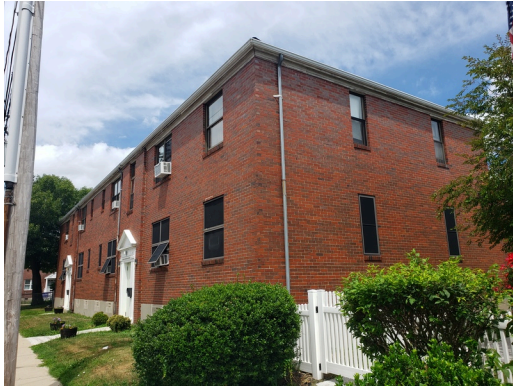
Sidewall System: Building 1 southeast corner facade.
