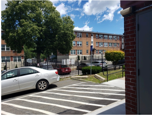
Paving, Curbing, & Parking: Typical striping found throughout the property.
