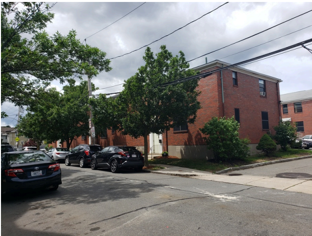
51. Sidewall System: Building 2 east facade.
