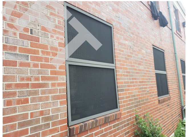
68. Windows: Typical single-hung style double-pane aluminum windows found throughout the site.
