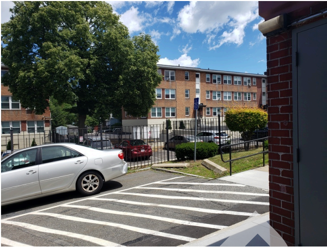
13. Paving, Curbing, & Parking: Typical striping found throughout the property.
