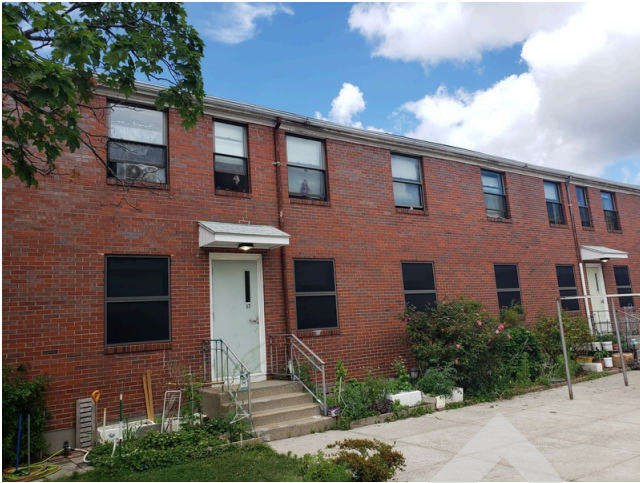
41. Sidewall System: Typical sidewall unpainted brick found throughout the site.
