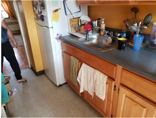
Cabinets & Fixtures: Typical dwelling unit kitchen sink, countertop, and wood cabinets found throughout the site.
