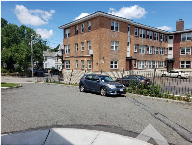
9. Paving, Curbing, & Parking: Typical asphalt pavement found throughout the site.
