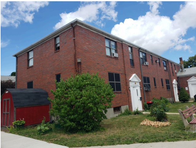
63. Sidewall System: Building 3 southwest corner facade.
