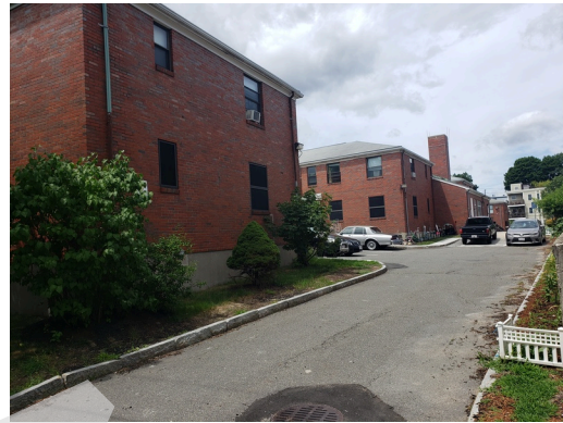
Paving, Curbing, & Parking: Typical concrete curving found throughout the site.
