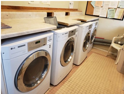
Common Area Interior Elements: Common laundry room.
