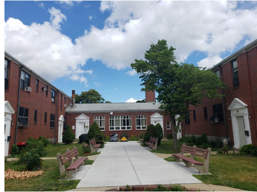
Landscaping & Appurtenances: Typical landscaping found throughout at the property.
