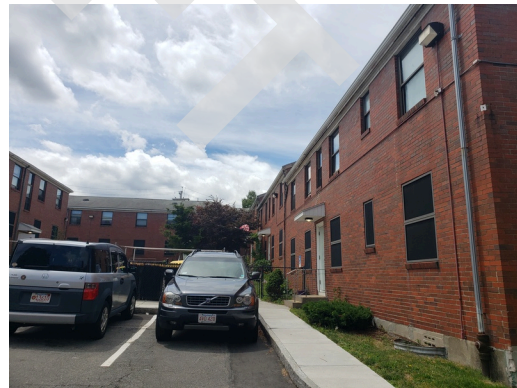
Sidewall System: Building 1 northeast internal corner facade.
