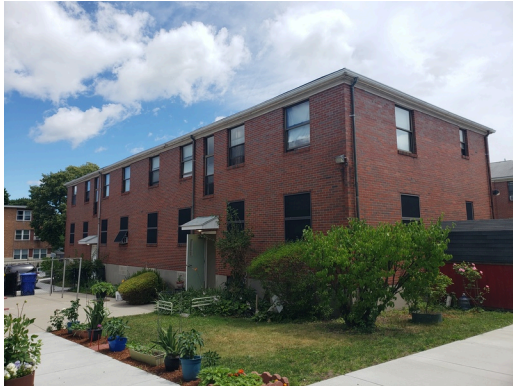
Sidewall System: Building 3 southwest corner facade.
