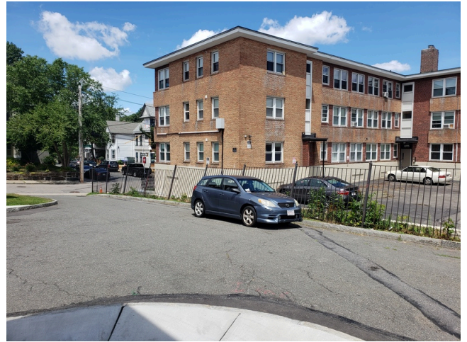
2. Stormwater Drainage: Typical adjoining property found around the site.
