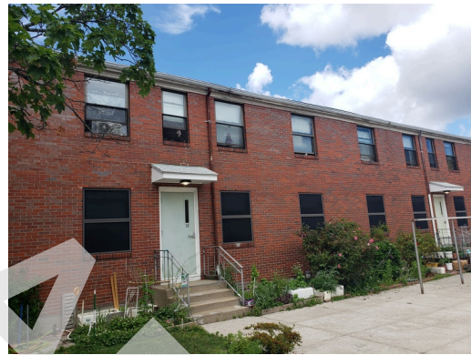
Sidewall System: Building 3 west facade.
