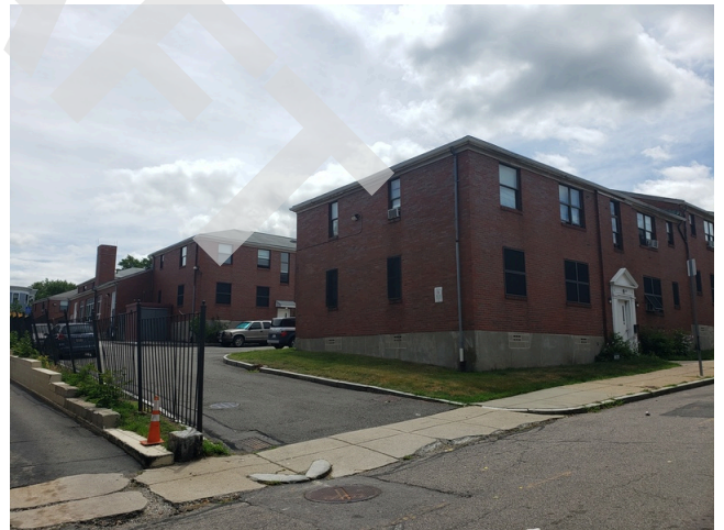
60. Sidewall System: Building 1 northwest corner facade.
