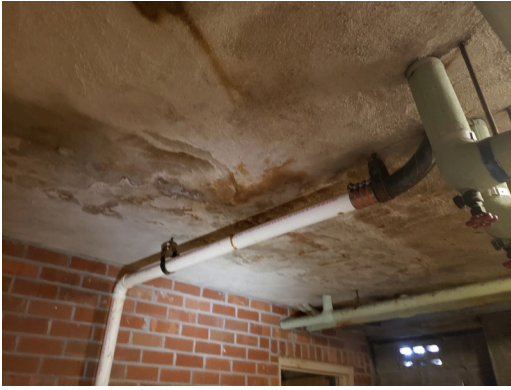
Plumbing: Typical cast iron and PVC waste pipes found throughout the property.
