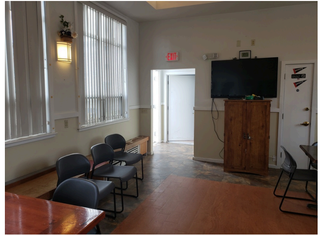
94. Life & Fire Safety: Typical illuminated exit sign found throughout the site.
