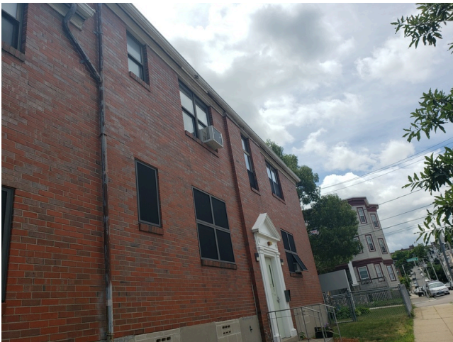
59. Sidewall System: Building 1 west facade.
