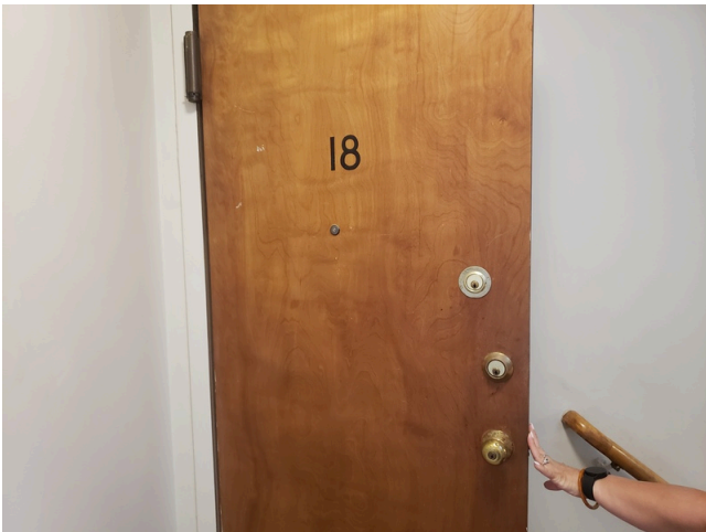
39. Exterior Doors & Entry Systems: Typical unit door found throughout the site.
