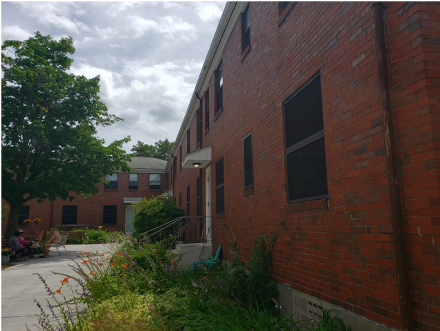
55. Sidewall System: Building 2 west internal facade.
