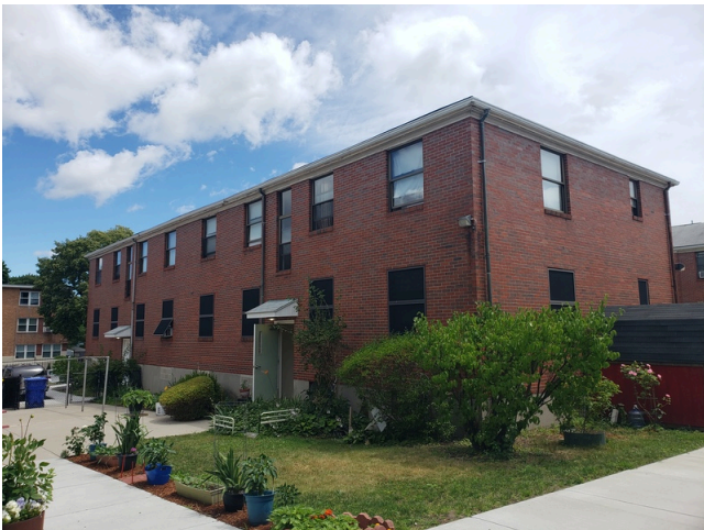
67. Windows: Typical single-hung style double-pane aluminum windows found throughout the site.
