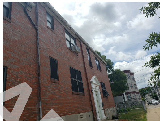
Sidewall System: Building 1 west facade.
