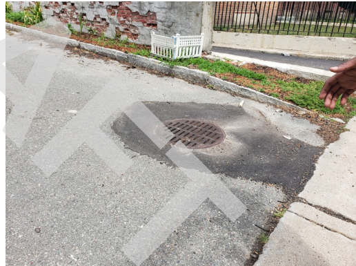
Stormwater Drainage: Typical paving drainage found throughout site.
