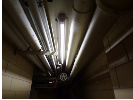
Maintenance Shop Lighting
