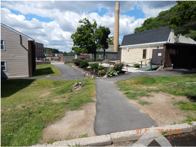
1. Stormwater Drainage: Typical topography found throughout the site.
