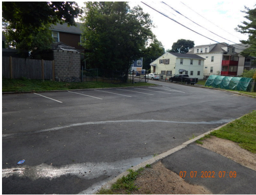
Access & Egress: North access drive to the property.
