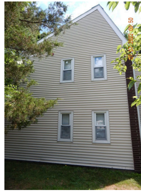
Sidewall System: Typical sidewall vinyl siding found throughout the site.
