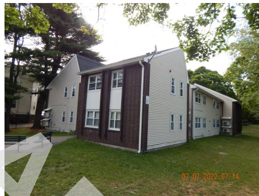
Stormwater Drainage: Typical downspout found throughout site.
