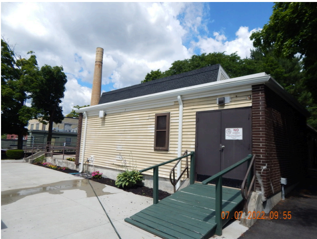
59. Exterior Doors & Entry Systems: Typical service door found throughout the site.
