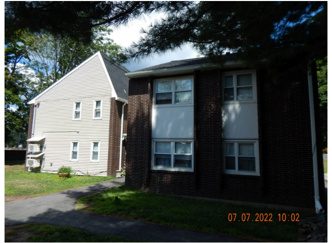
90. Sidewall System: Building 2 east facade.
