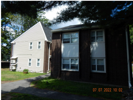
Sidewall System: Building 2 east facade.
