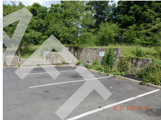
Stormwater Drainage: Typical retaining wall found throughout the site.
