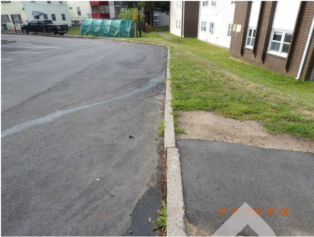
13. Paving, Curbing, & Parking: Typical concrete curving found throughout the site.
