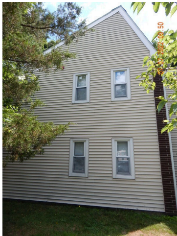
103. Windows: Typical single-hung style double-pane vinyl windows found throughout the site.
