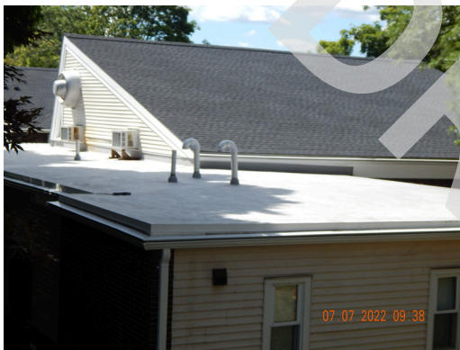
Roof Frame & Sheathing: Typical low-slope roofs found throughout the property.
