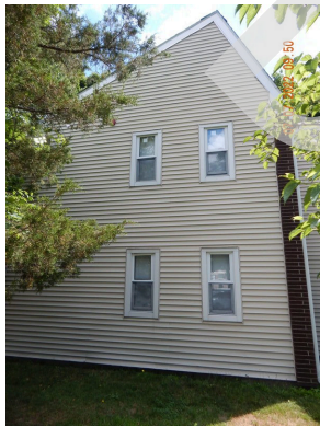
Sidewall System: Building 3 west facade.
