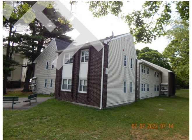
8. Stormwater Drainage: Typical downspout found throughout site.
