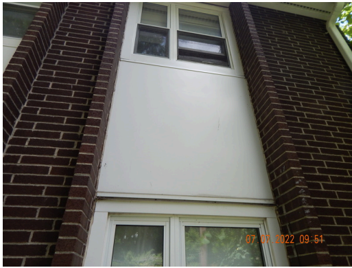
Sidewall System: Typical sidewall vinyl siding and unpainted brick found throughout the site.
