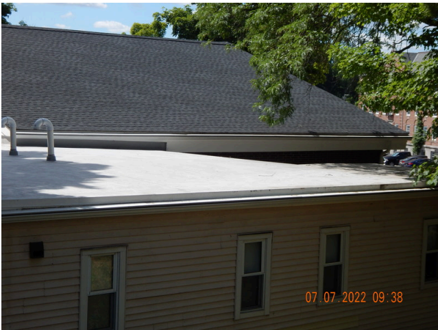
111. Roofing Finish: Typical TPO roofing found throughout the site.
