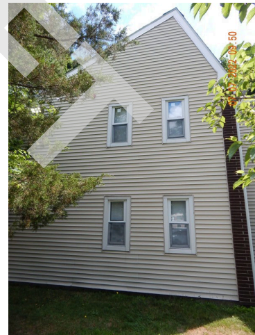
64. Sidewall System: Typical sidewall vinyl siding found throughout the site.
