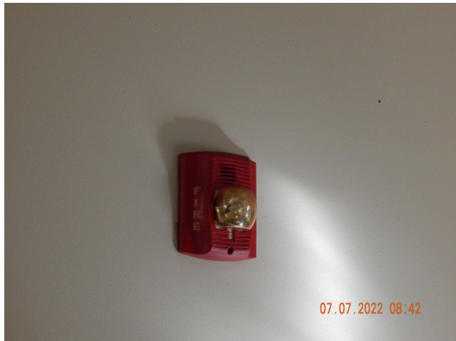
131. Life & Fire Safety: Typical strobe light found in individual units throughout the site.
