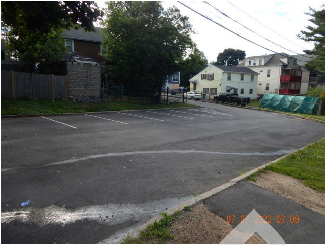
9. Access & Egress: North access drive to the property.
