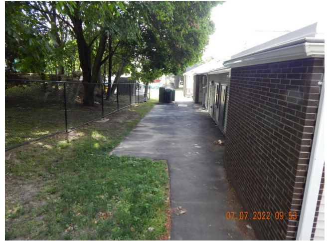
18. Flatwork (Walks, Plazas, Terraces, Patios): Typical asphalt sidewalk found around the property.
