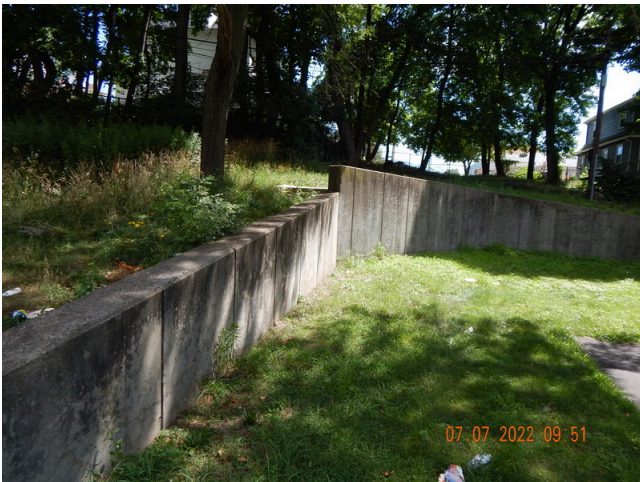
3. Stormwater Drainage: Typical retaining wall found throughout the site.
