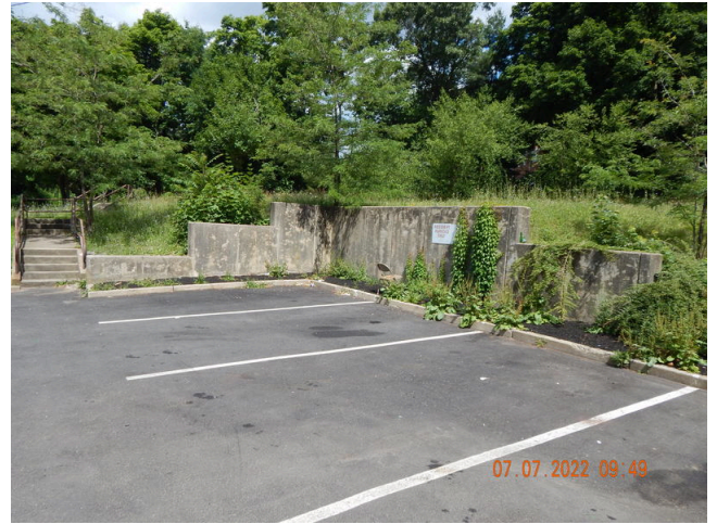
14. Paving, Curbing, & Parking: Typical striping found throughout the property.
