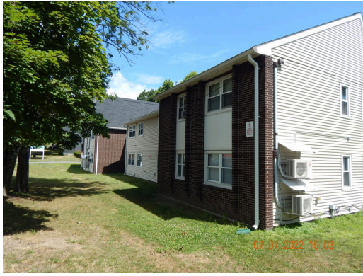
Sidewall System: Building 2 southeast facade.
