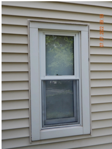
75. Sidewall System: Typical vinyl trim found throughout the site.
