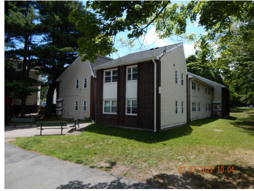
Sidewall System: Building 3 southeast facade.
