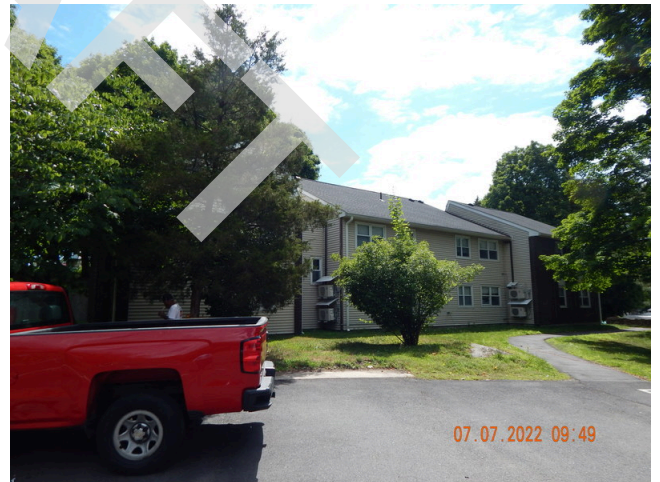
80. Sidewall System: Building 3 south facade.
