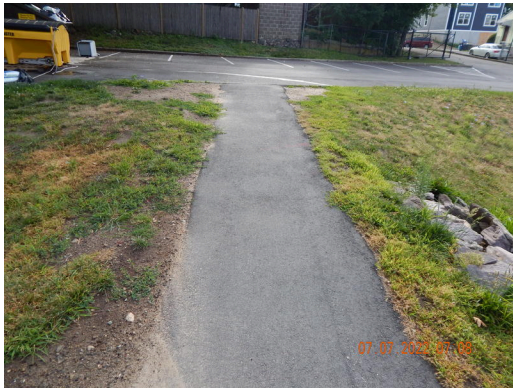
Flatwork (Walks, Plazas, Terraces, Patios): Typical asphalt sidewalk found around the property.
