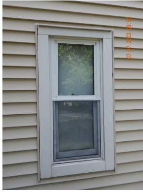
Sidewall System: Typical vinyl trim found throughout the site.
