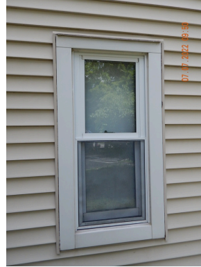
Windows: Typical single-hung style double-pane vinyl windows found throughout the site.
