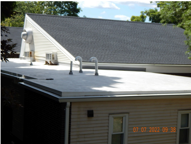
43. Roof Frame & Sheathing: Typical low-slope roofs found throughout the property.
