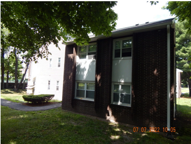
95. Sidewall System: Building 3 west facade.
