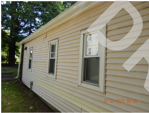
Sidewall System: Community Building west facade.
