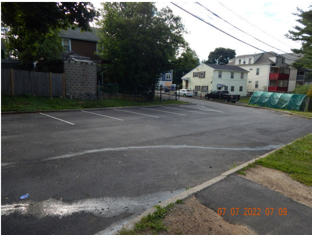
11. Paving, Curbing, & Parking: Typical asphalt pavement found throughout the site.
