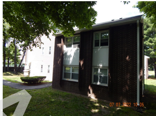
Sidewall System: Building 3 west facade.
