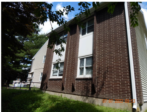
Sidewall System: Building 3 east facade.
