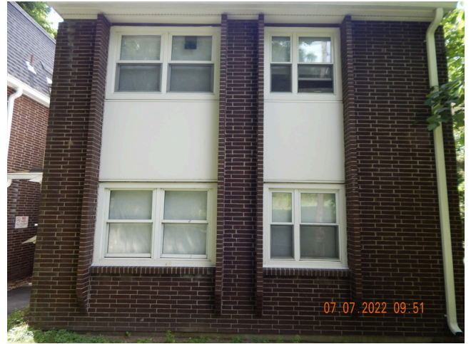
74. Sidewall System: Typical sidewall unpainted brick found throughout the site.
