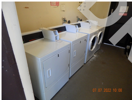
Common Area Interior Elements: Common laundry room.
