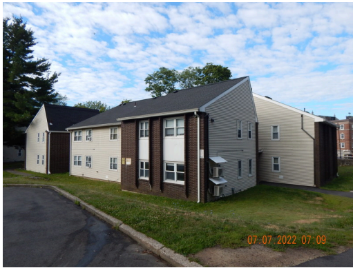
Roof Frame & Sheathing: Typical sloped roofs found throughout the property.
