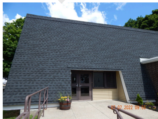
Roofing Finish: Typical asphalt shingle roofing found throughout the site.
