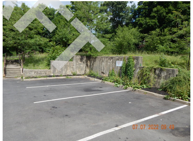
4. Stormwater Drainage: Typical retaining wall found throughout the site.
