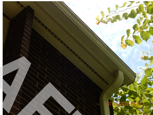
Attics & Eaves: Typical perforated eaves vents found throughout the site.
