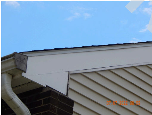
Flashing & Moisture Protection: Typical flashing found throughout the site.
