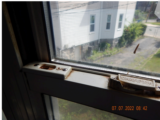
Windows: Typical single-hung style double-pane vinyl windows found throughout the site.
