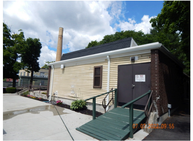
102. Sidewall System: Community Building east facade.
