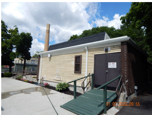
Sidewall System: Community Building east facade.
