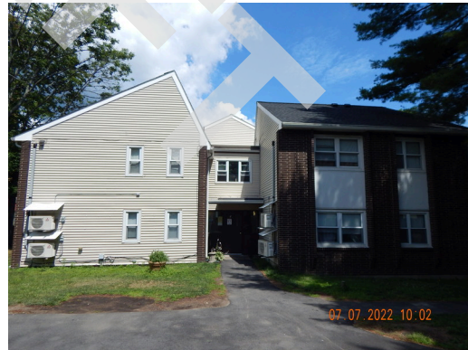
Sidewall System: Building 2 east facade.
