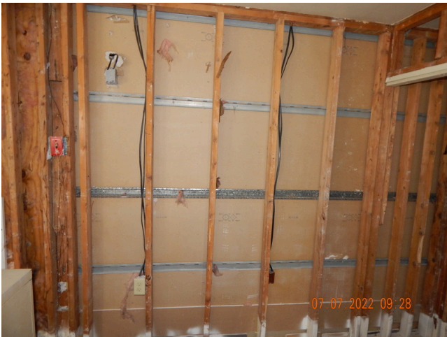
39. Framing System, Floors & Walls: Typical wood framing found throughout the site.
