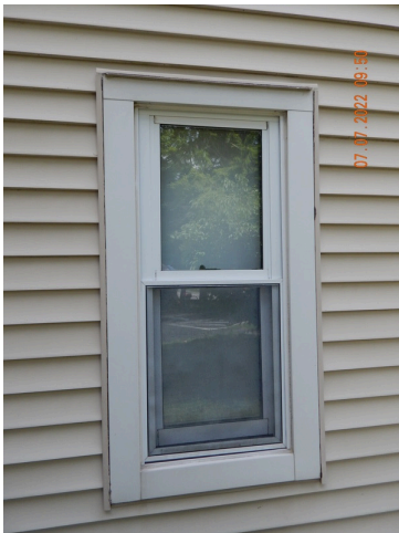
47. Flashing & Moisture Protection: Typical flashing found throughout the site.
