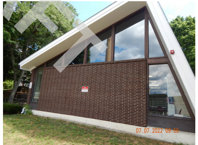
72. Sidewall System: Typical sidewall unpainted brick found throughout the site.
