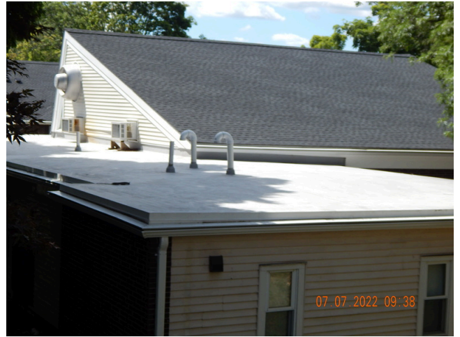
110. Roofing Finish: Typical TPO roofing found throughout the site.
