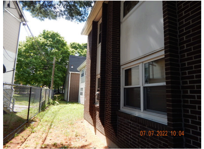
94. Sidewall System: Building 3 north facade.
