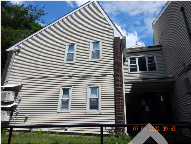
85. Sidewall System: Building 3 east facade.
