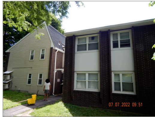
Sidewall System: Building 3 west facade.
