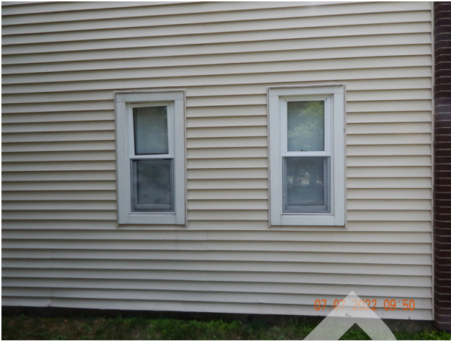
65. Sidewall System: Typical sidewall vinyl siding found throughout the site.
