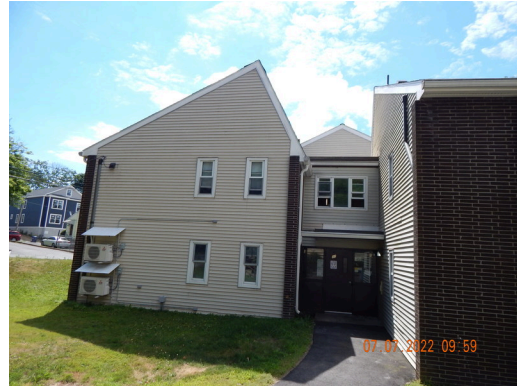
Sidewall System: Building 2 east facade.
