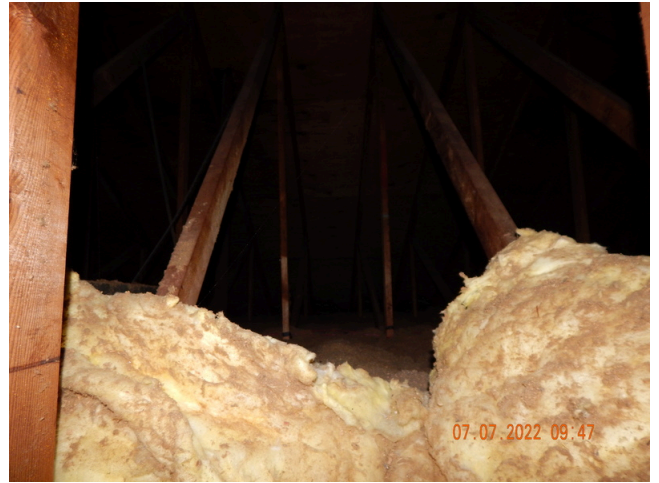
54. Insulation: Typical blown-in cellulose and fiber glass batt insulation found throughout the site.
