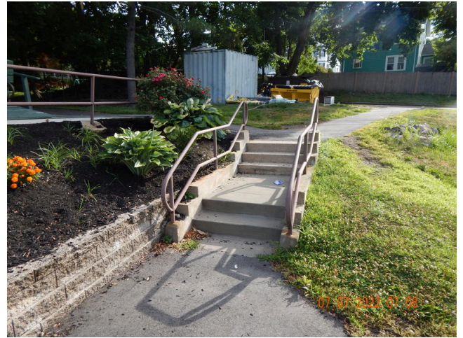
22. Flatwork (Walks, Plazas, Terraces, Patios): Concrete steps with steel handrails found at the property.
