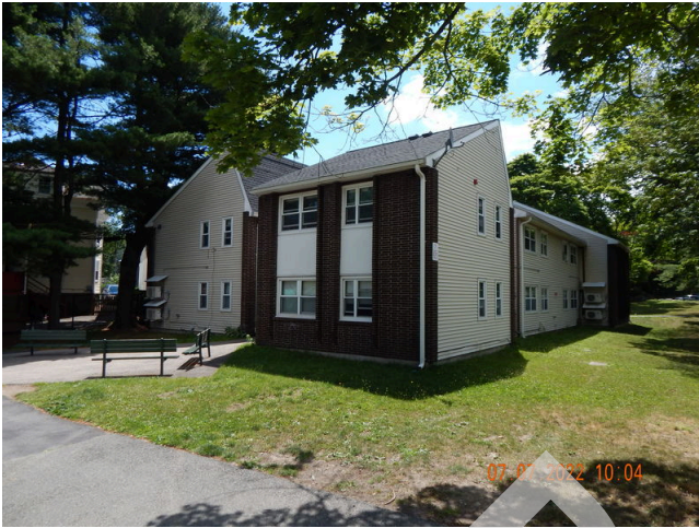
93. Sidewall System: Building 3 southeast facade.
