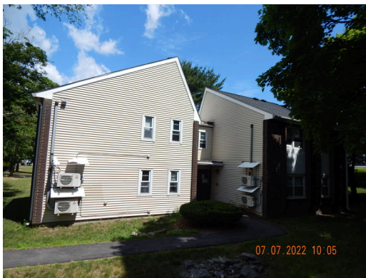
Sidewall System: Building 3 north facade.
