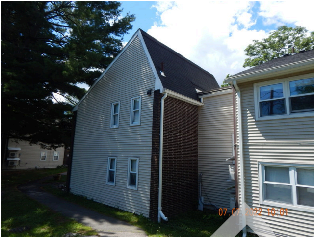
89. Sidewall System: Building 2 north facade.
