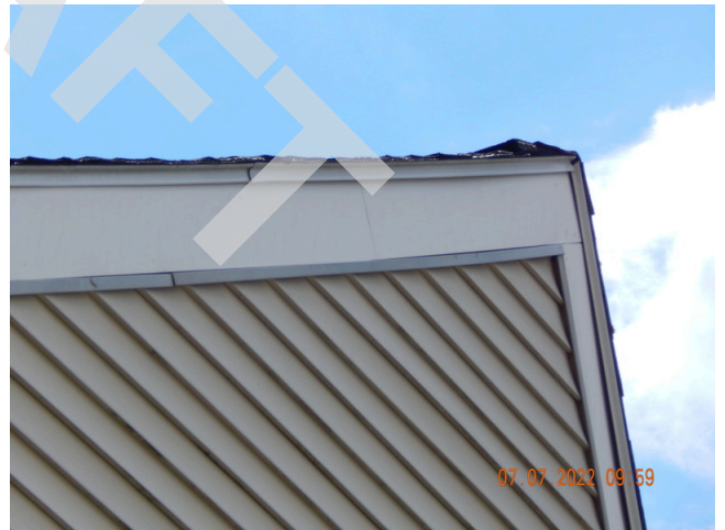
48. Flashing & Moisture Protection: Typical flashing found throughout the site.
