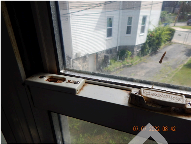
105. Windows: Typical single-hung style double-pane vinyl windows found throughout the site.
