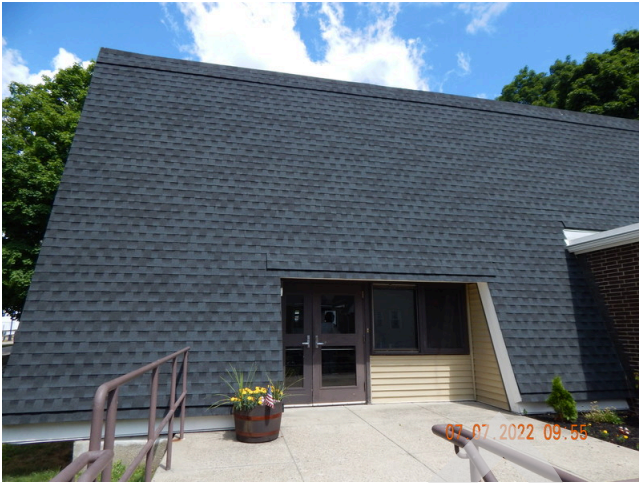
109. Roofing Finish: Typical asphalt shingle roofing found throughout the site.
