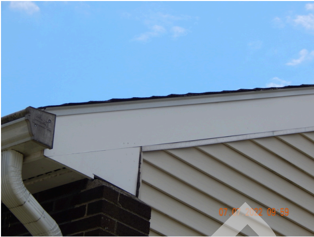
49. Flashing & Moisture Protection: Typical flashing found throughout the site.
