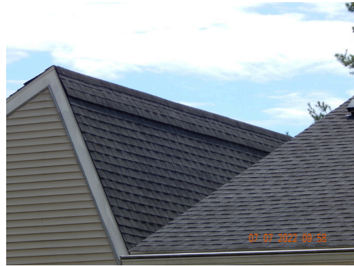
Attics & Eaves: Typical ridge vents found throughout the site.
