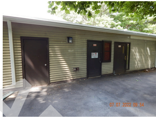
Sidewall System: Community Building north facade.
