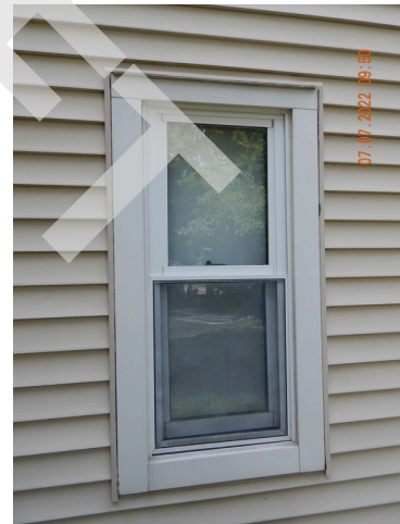
104. Windows: Typical single-hung style double-pane vinyl windows found throughout the site.
