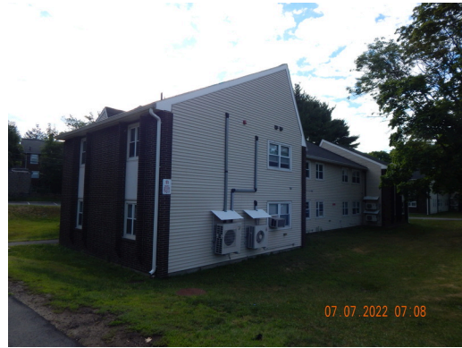
Roof Frame & Sheathing: Typical sloped roofs found throughout the property.
