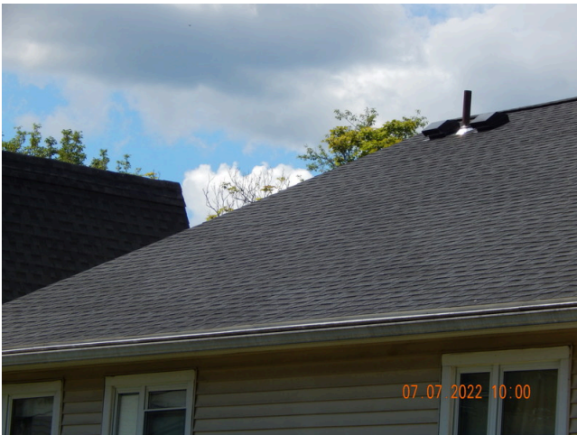
107. Roofing Finish: Typical asphalt shingle roofing found throughout the site.
