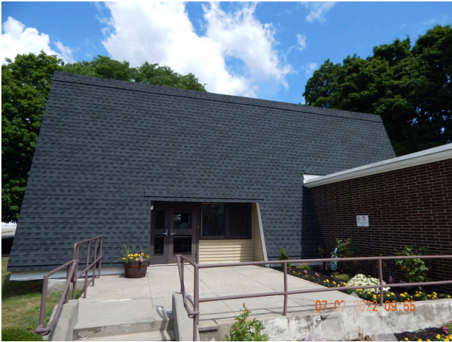
97. Sidewall System: Community Building east facade.
