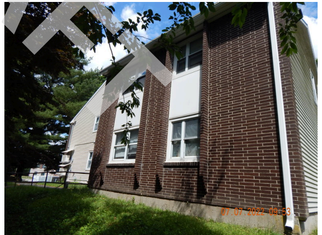
84. Sidewall System: Building 3 east facade.
