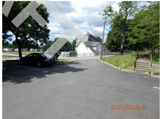
12. Paving, Curbing, & Parking: Typical asphalt pavement found throughout the site.
