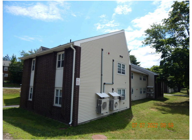
86. Sidewall System: Building 2 southeast facade.
