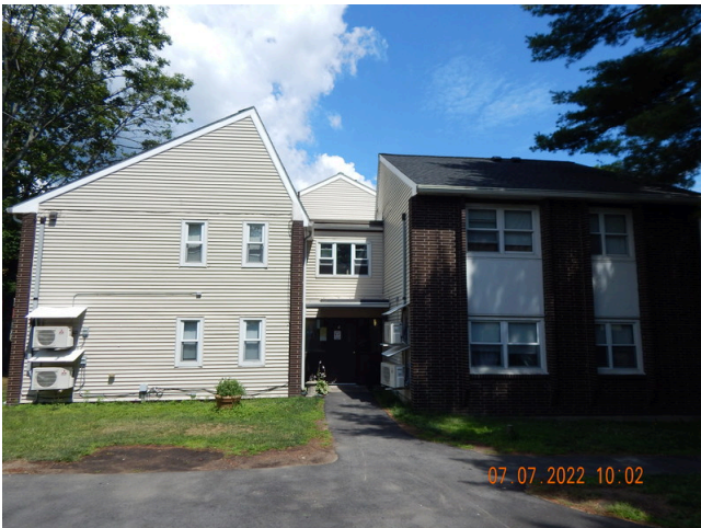
91. Sidewall System: Building 2 east facade.
