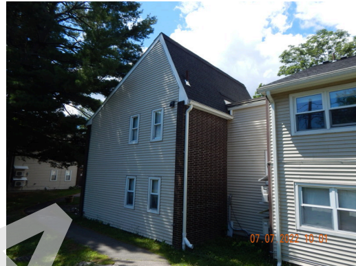
Sidewall System: Building 2 north facade.
