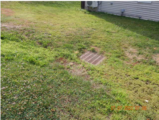
7. Stormwater Drainage: Typical landscaping drainage found throughout site.
