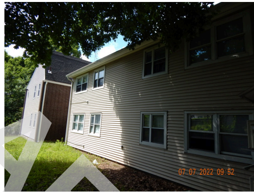
Sidewall System: Building 3 north facade.
