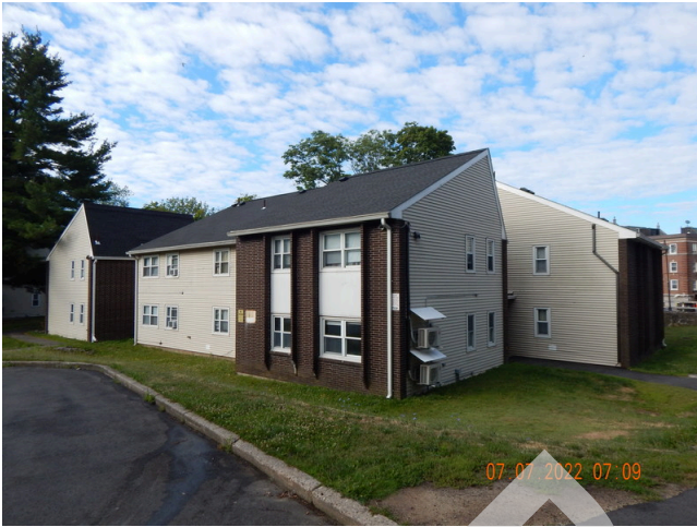
61. Sidewall System: Typical sidewall vinyl siding and unpainted brick found throughout the site.
