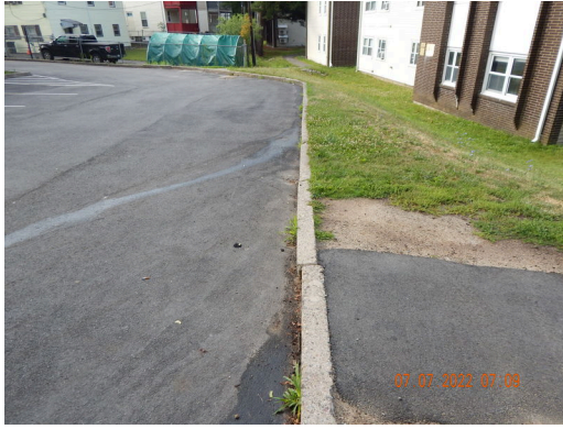
Paving, Curbing, & Parking: Typical concrete curving found throughout the site.
