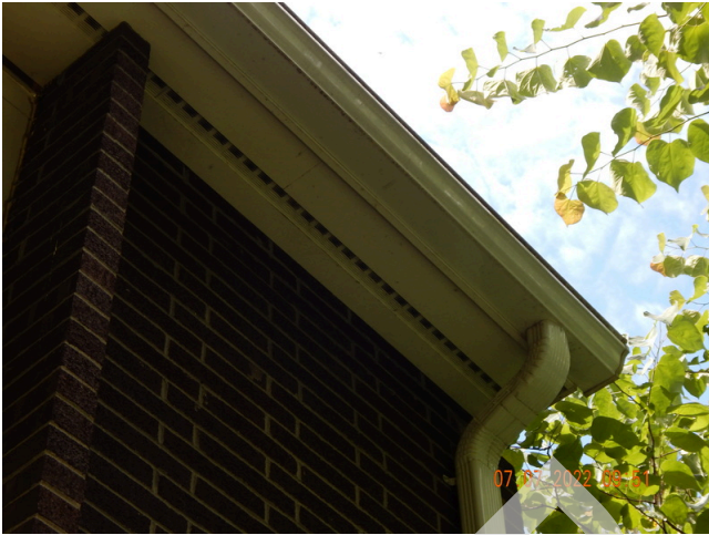
53. Attics & Eaves: Typical perforated eaves vents found throughout the site.
