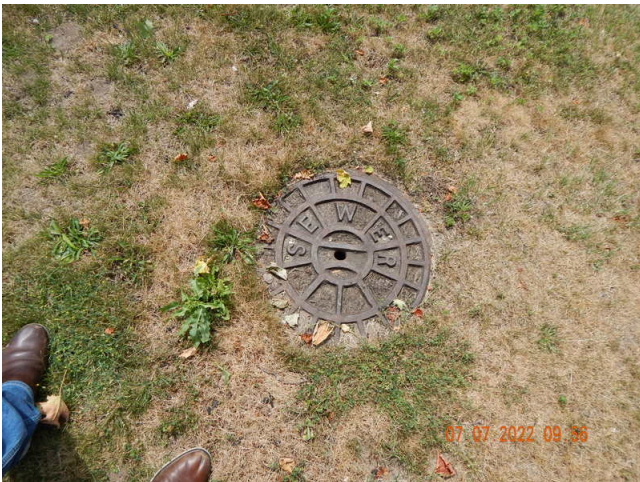
35. Site Utilities: Sewer system found at the site.
