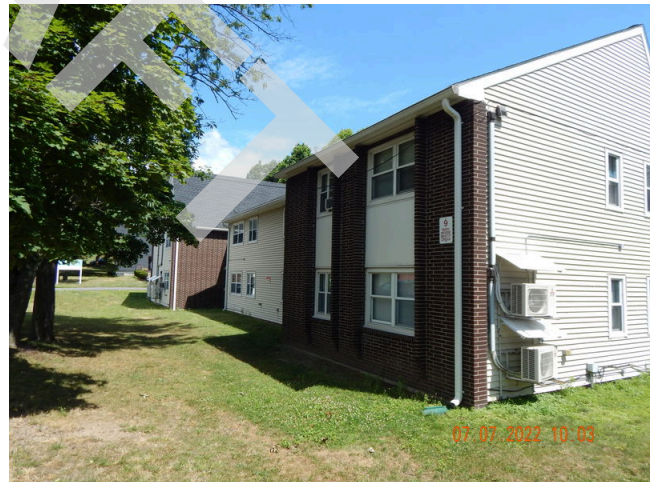
92. Sidewall System: Building 2 southeast facade.
