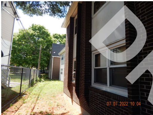
Sidewall System: Building 3 north facade.
