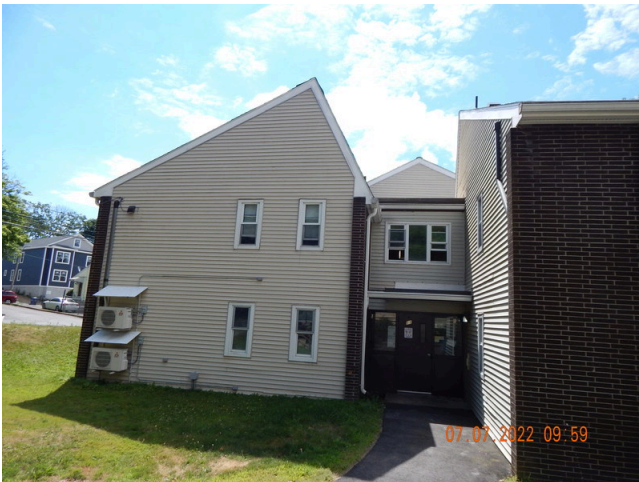
87. Sidewall System: Building 2 east facade.
