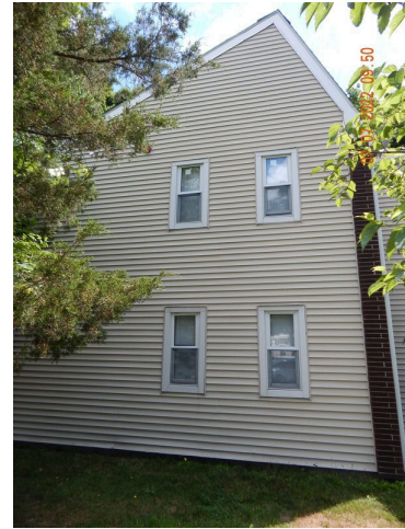
82. Sidewall System: Building 3 west facade.
