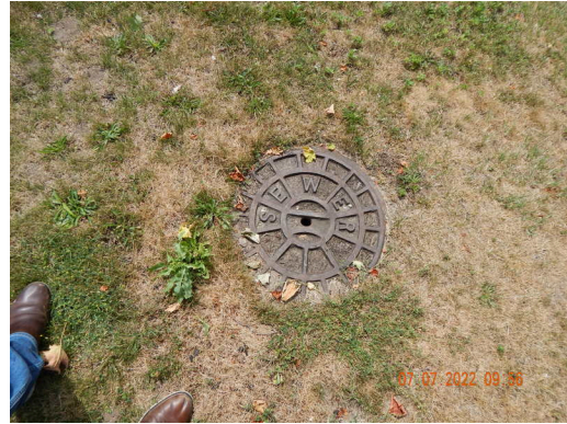
Site Utilities: Sewer system found at the site.
