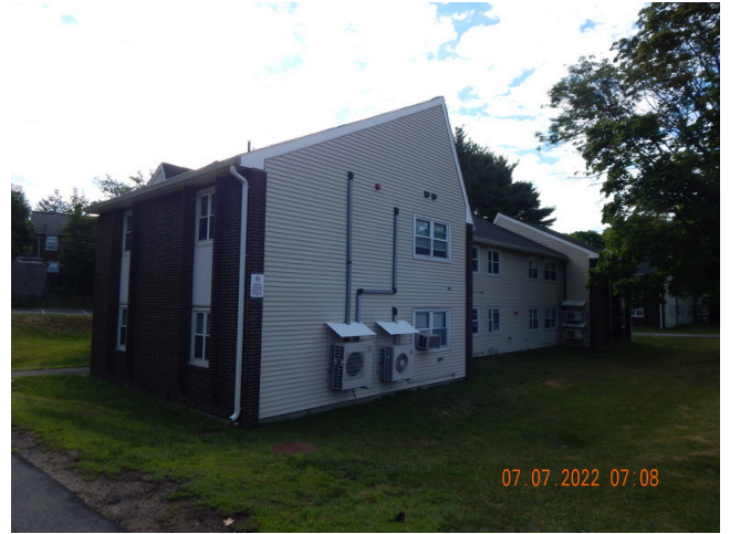
42. Roof Frame & Sheathing: Typical sloped roofs found throughout the property.
