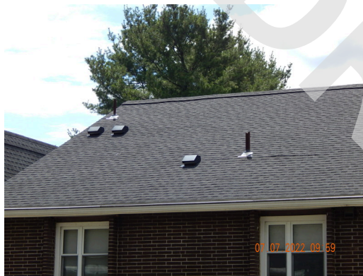
Roofing Finish: Typical asphalt shingle roofing found throughout the site.
