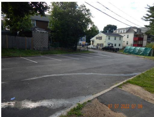
Paving, Curbing, & Parking: Typical asphalt pavement found throughout the site.
