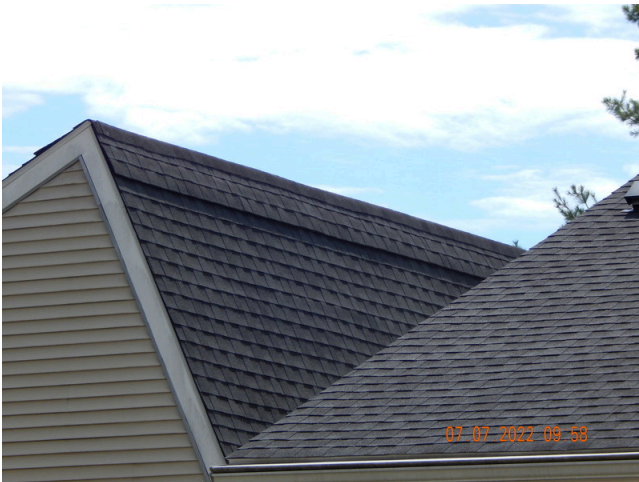
51. Attics & Eaves: Typical ridge vents found throughout the site.
