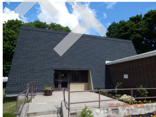
Sidewall System: Community Building east facade.
