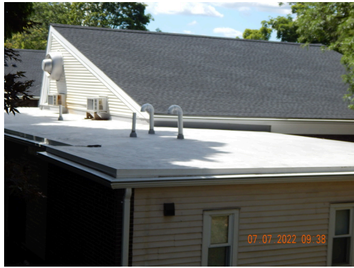
Roofing Finish: Typical TPO roofing found throughout the site.
