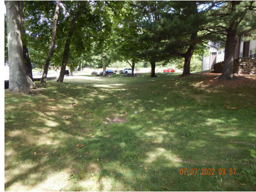
Stormwater Drainage: Typical topography found throughout the site.
