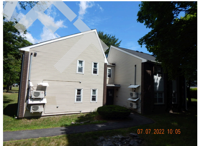
96. Sidewall System: Building 3 north facade.
