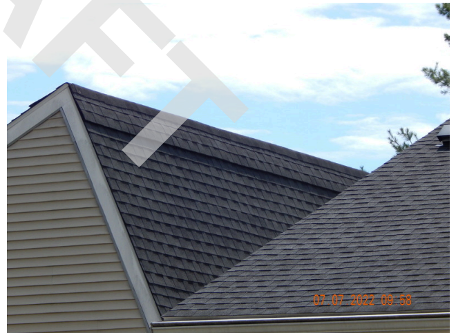
108. Roofing Finish: Typical asphalt shingle roofing found throughout the site.
