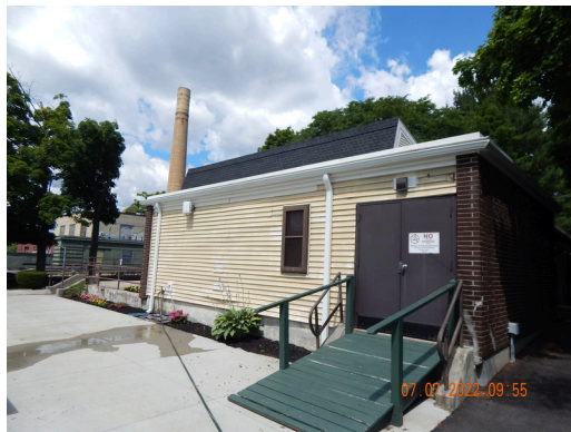
Exterior Doors & Entry Systems: Typical service door found throughout the site.
