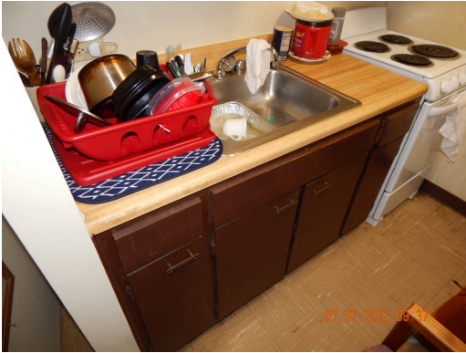
Cabinets & Fixtures: Typical dwelling unit kitchen sink, countertop, and wood cabinets found throughout the site.
