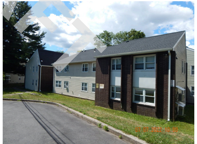
88. Sidewall System: Building 2 north facade.
