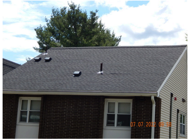
50. Attics & Eaves: Typical ridge vents found throughout the site.
