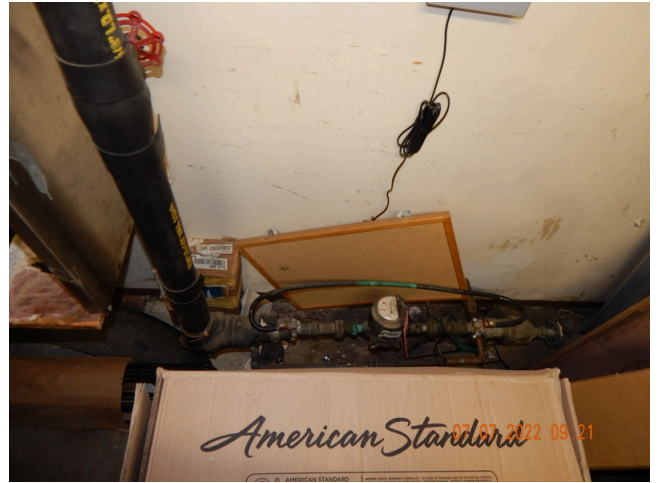
34. Site Utilities: Central water meter found at the site.
