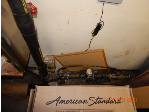
Site Utilities: Central water meter found at the site.
