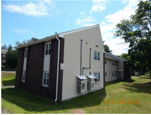
Sidewall System: Building 2 southeast facade.
