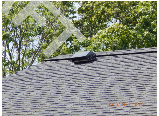
52. Attics & Eaves: Typical roof vents found throughout the site.
