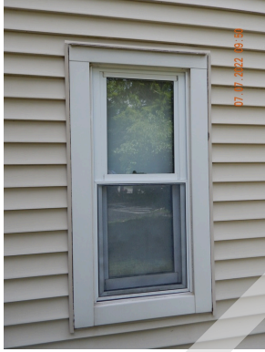
Flashing & Moisture Protection: Typical flashing found throughout the site.
