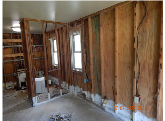
146. Dwelling Unit Interior Elements: Unit 26 gutted and unfinished. (Critical Repair)
