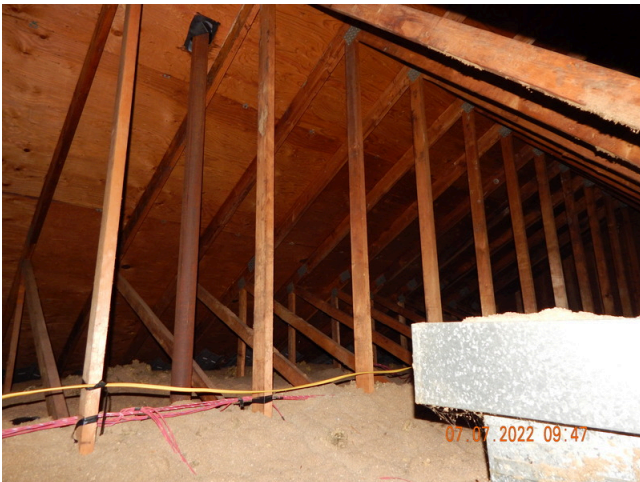
55. Insulation: Typical blown-in cellulose insulation found throughout the site.
