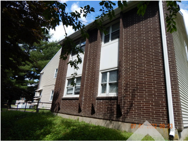
73. Sidewall System: Typical sidewall unpainted brick found throughout the site.
