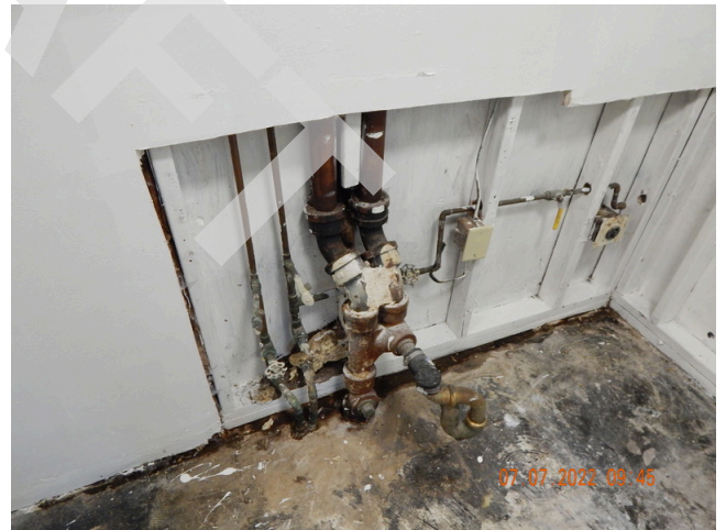
116. Plumbing: Typical cast iron waste pipes found throughout the exterior of the property.
