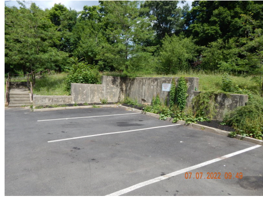
Paving, Curbing, & Parking: Typical striping found throughout the property.
