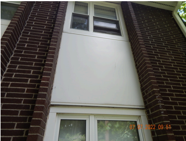
63. Sidewall System: Typical sidewall vinyl siding and unpainted brick found throughout the site.
