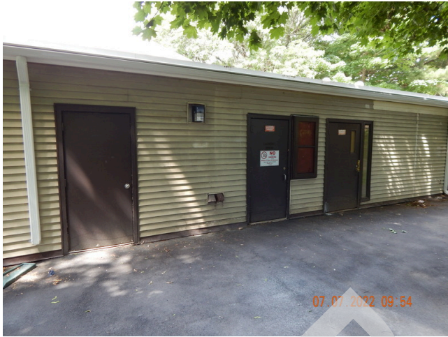
101. Sidewall System: Community Building north facade.
