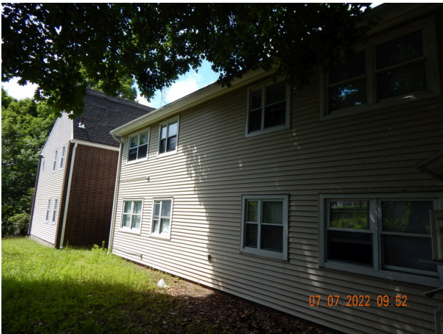
83. Sidewall System: Building 3 north facade.
