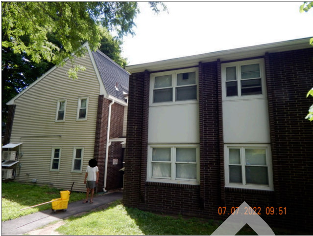
81. Sidewall System: Building 3 west facade.
