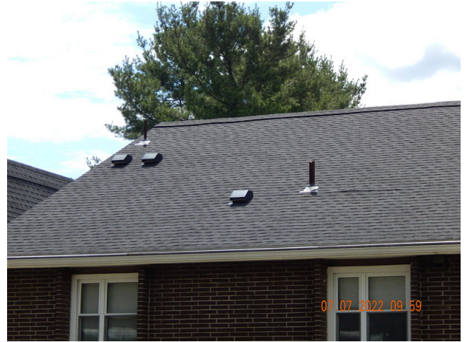
106. Roofing Finish: Typical asphalt shingle roofing found throughout the site.
