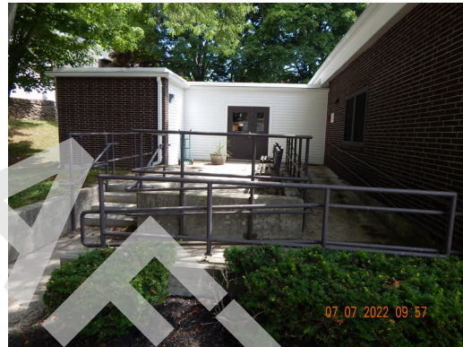
Flatwork (Walks, Plazas, Terraces, Patios): Poured in place concrete ramp and sidewalks found at the property.
