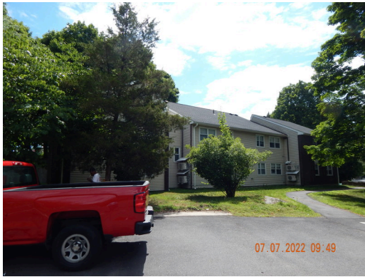
Sidewall System: Building 3 south facade.
