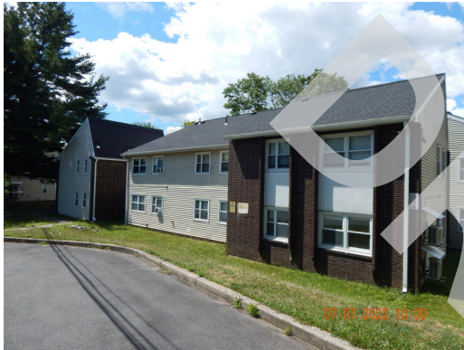
Sidewall System: Building 2 north facade.
