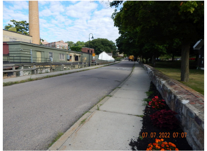
6. Stormwater Drainage: Typical adjoining property found around the site.
