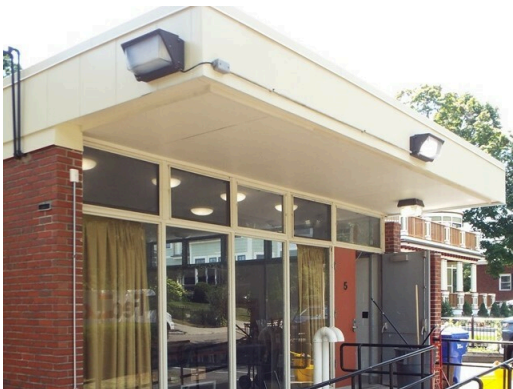
Building mounted lighting
