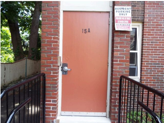
43. Typical exterior building entry door
