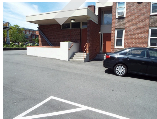
Pavement and striping condition
