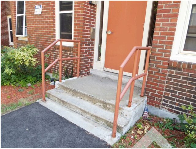
17. Typical entry steps
