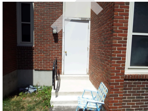
Typical building exit door
