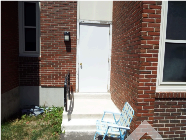
41. Typical building exit door
