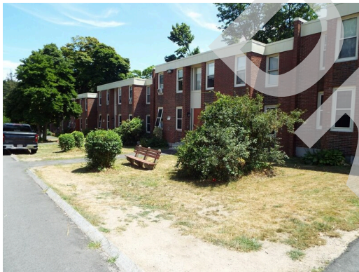
Landscaping - bare earth (Non-Critical Repair)
