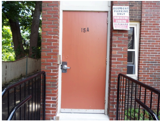
Typical exterior building entry door
