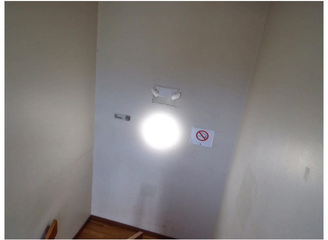
66. Interior stair - building 15
