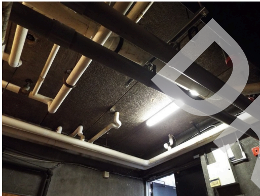
Framing - boiler room
