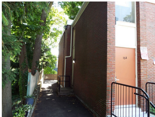
Gutter and downspout
