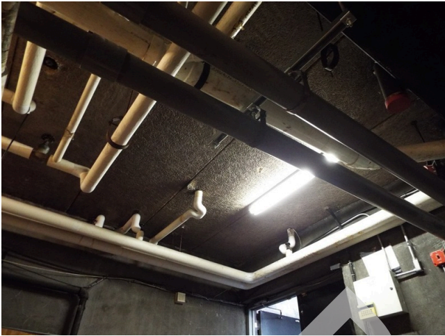
33. Framing - boiler room
