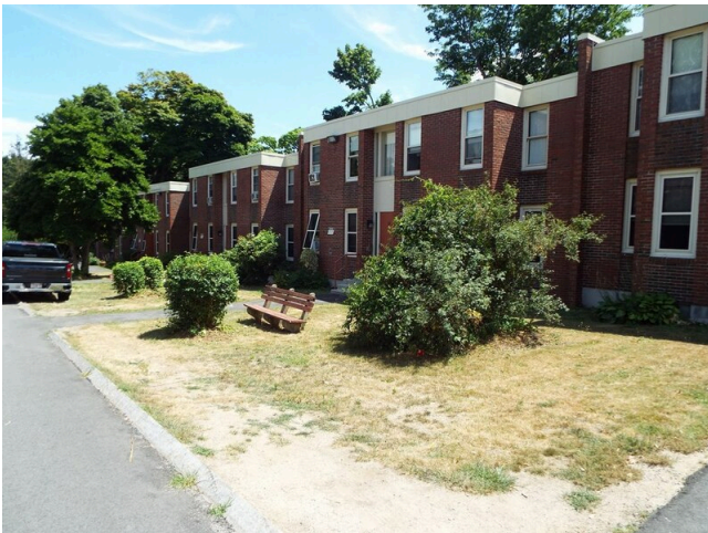
23. Landscaping - bare earth (Non-Critical Repair)
