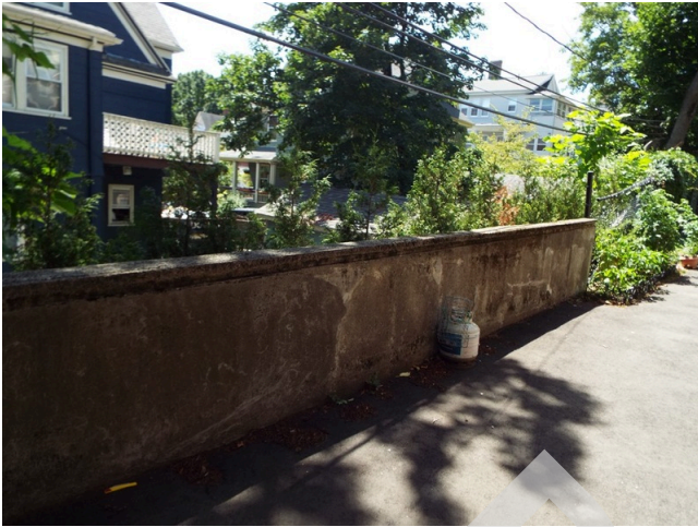
5. Retaining wall - south
