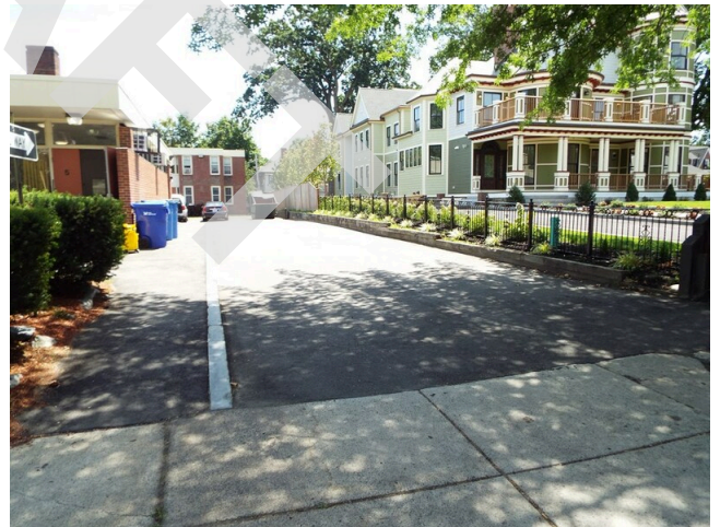
8. Access drive - west
