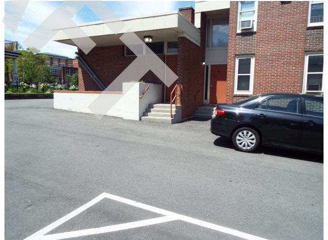
12. Pavement and striping condition
