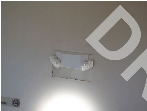
Interior stair - building 15
