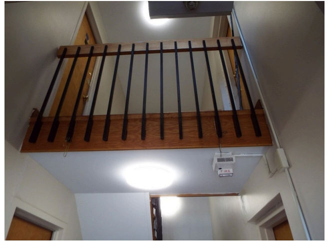
126. Typical apartment upper landing
