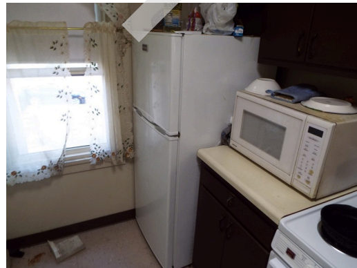
1-bed-1-bath - unit 6 - typical refrigerator
