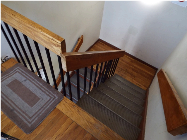
71. Interior stair - building 15
