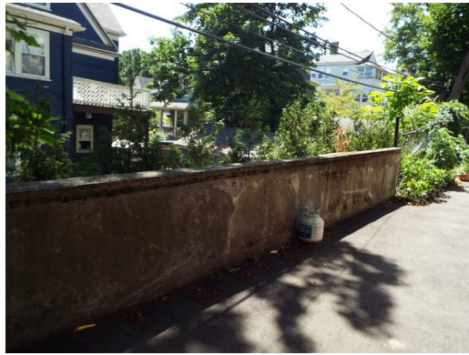
Retaining wall - south
