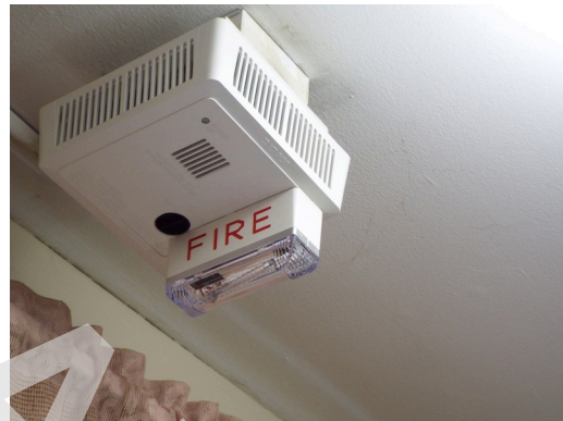
Interior stair - building 15
