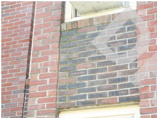
Brick masonry condition
