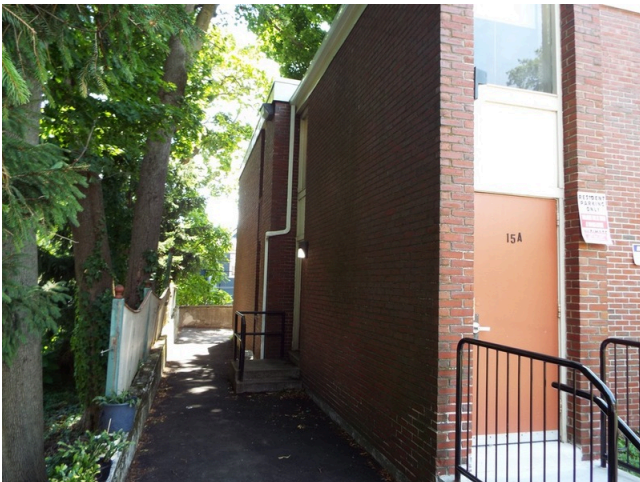
3. Gutter and downspout
