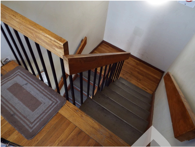
85. Typical common stairwell
