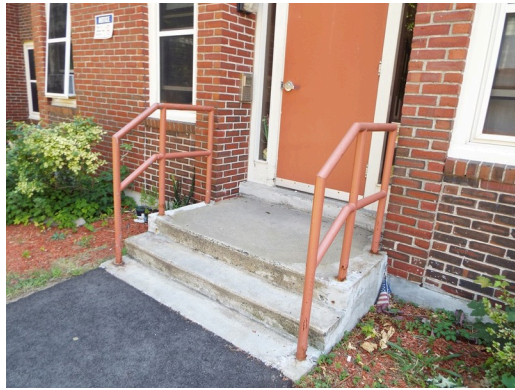
Typical entry steps
