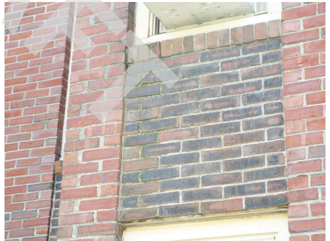
48. Brick masonry condition
