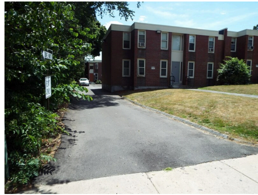
Exit drive - east
