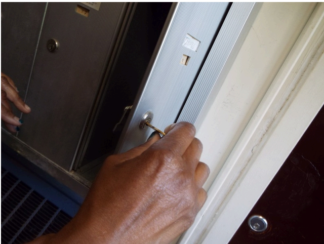
23. Mailbox key operation - building 15
