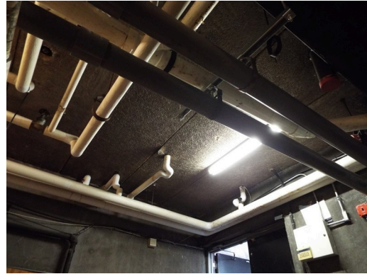
Framing - boiler room
