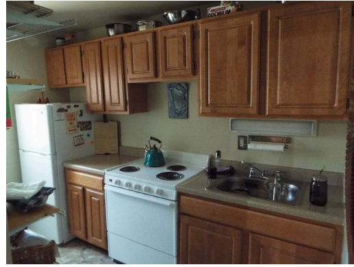
1-bed-1-bath - unit 2 - range malfunction (Critical Repair)
