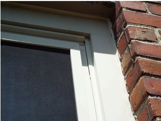
51. Typical window frame
