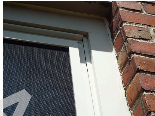
Typical window frame
