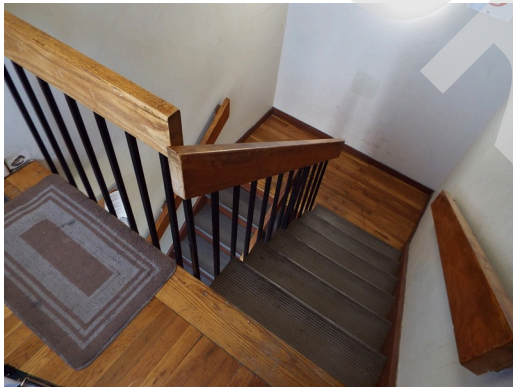
Interior stair - building 15
