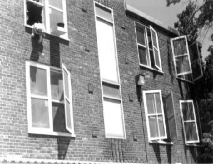
Mission Main Housing Development, 1999
