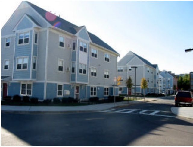
Part of the new Mission Main Development, 2002
