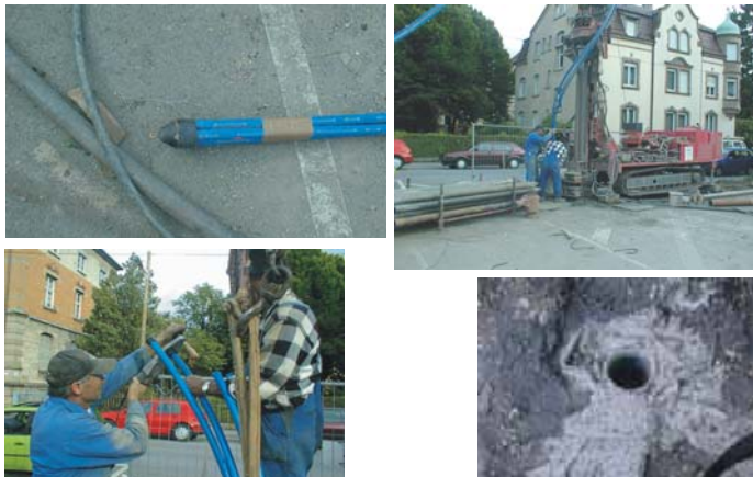
Geothermal borehole installation
