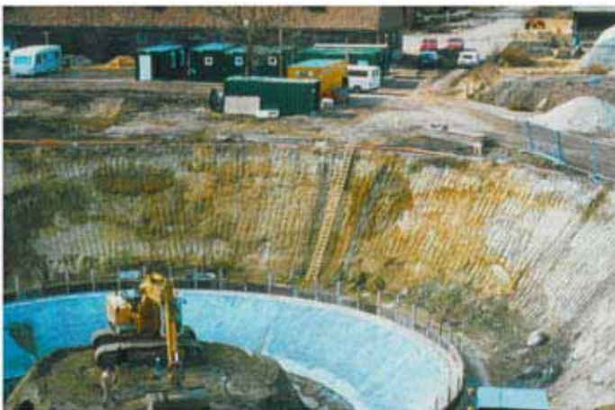
Thermal storage tank under construction, Hamburg
