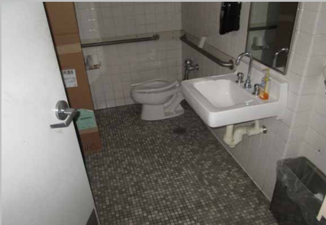
View of common restroom
