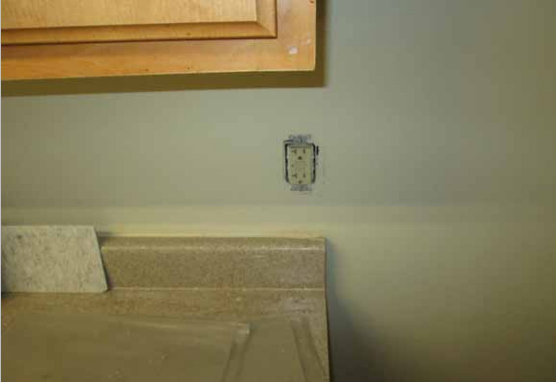
View of GFCI electrical outlet – dwelling unit
