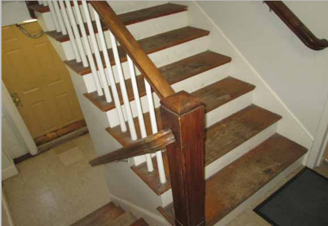
View of common interior stairwell
