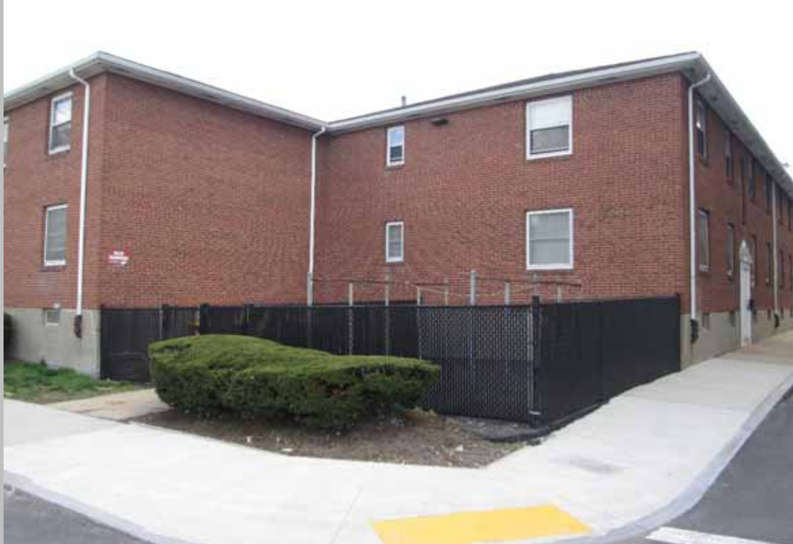
View of building exterior and curb access
