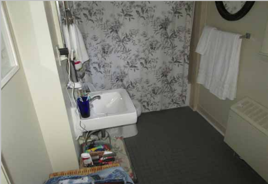
View of bathroom at Unit 3
