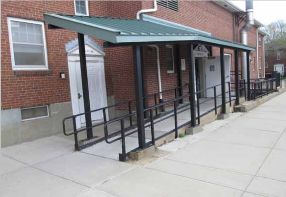
View of a property entry ramp with a metal roofing covered walkway
