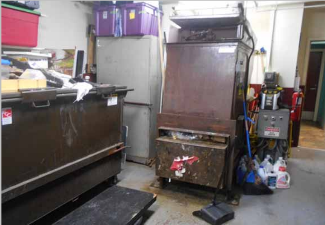
View of the trash compactor
