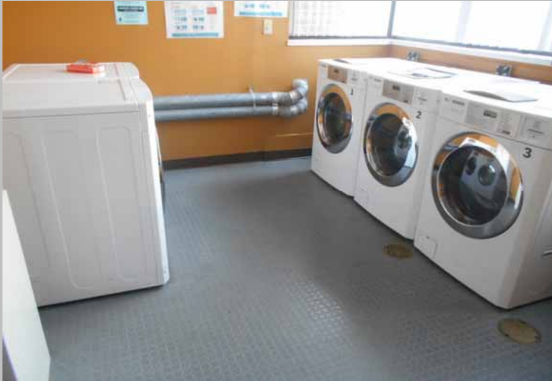
View of the common area laundry room
