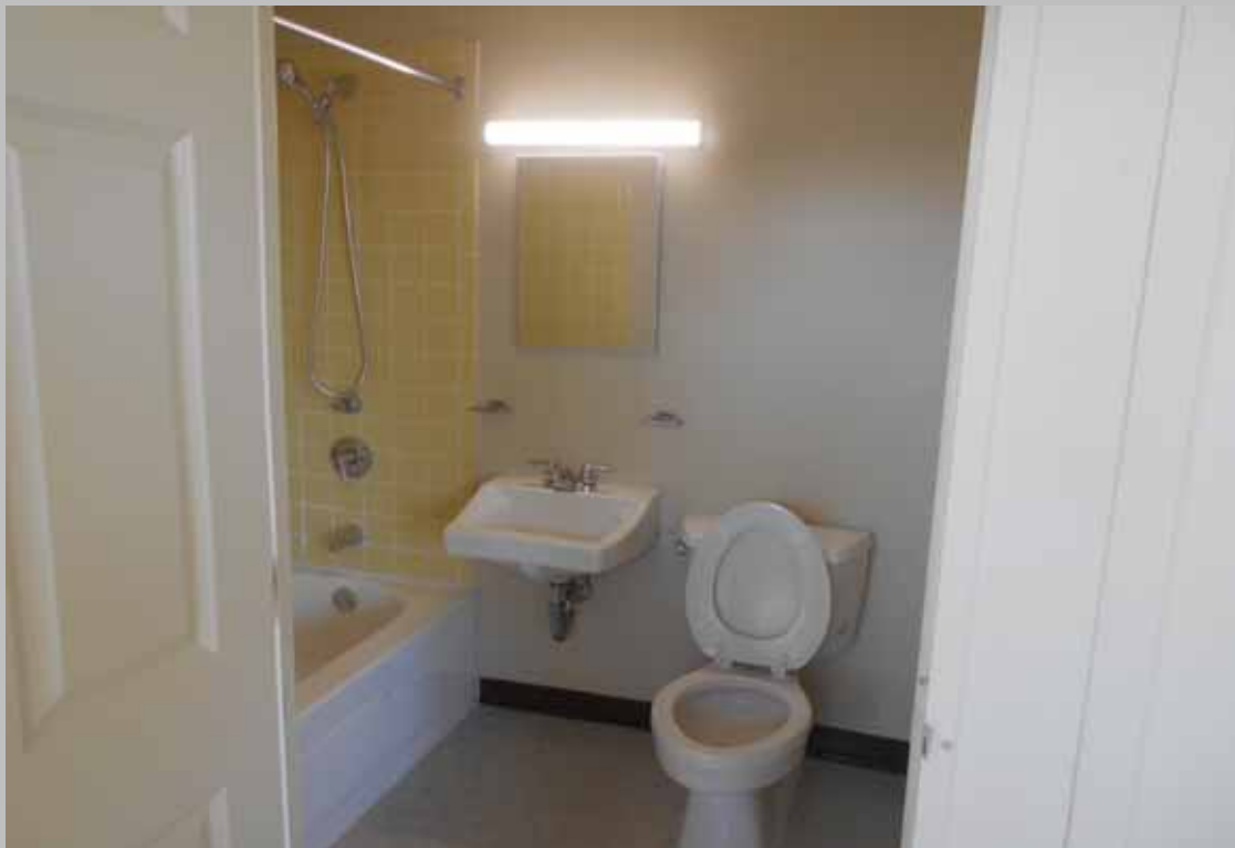
View of bathroom at Unit 710
