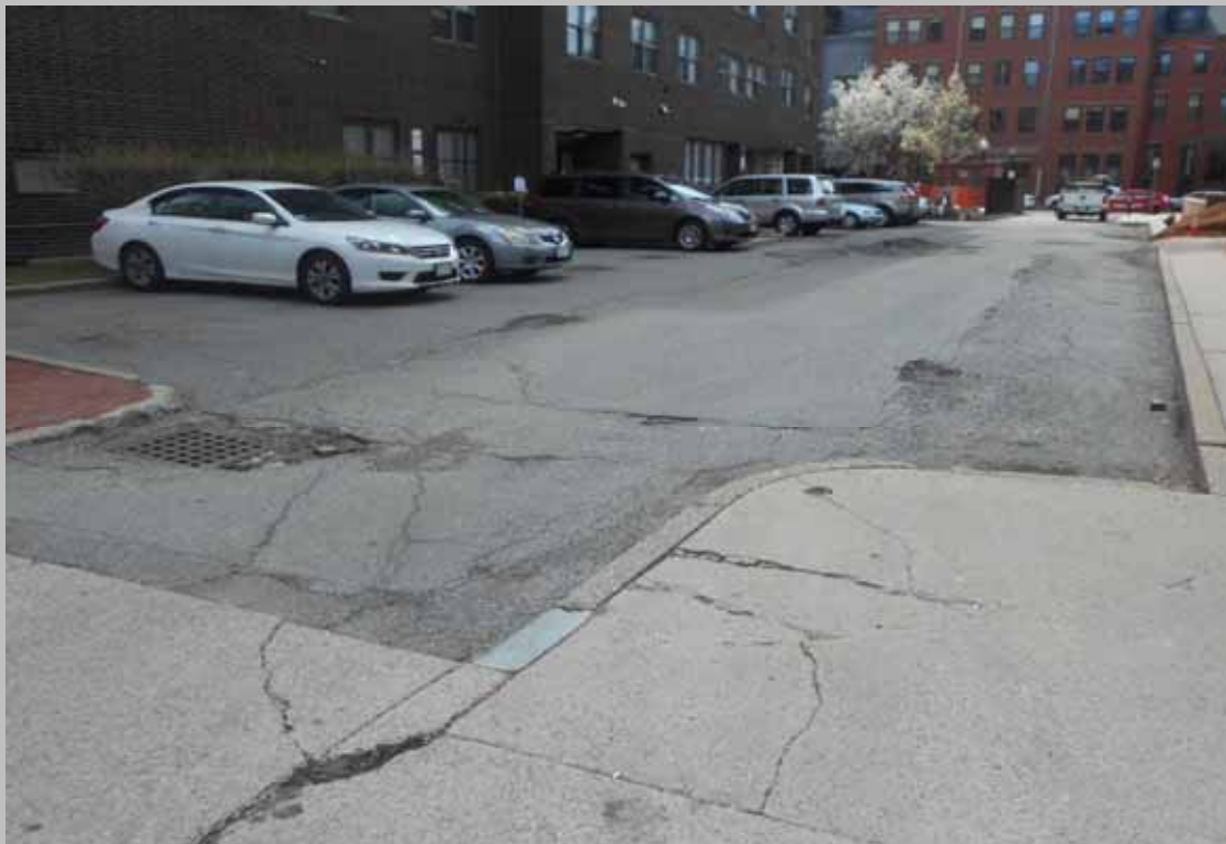
View of asphalt parking surface
