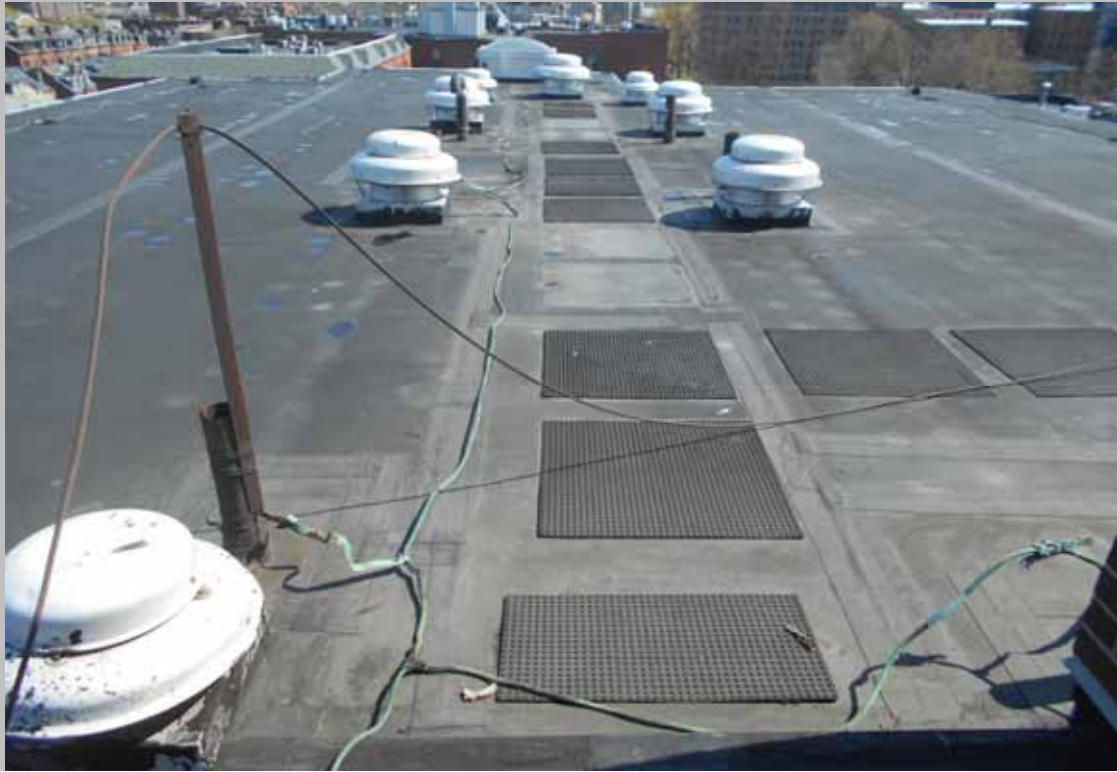
View of building roof
