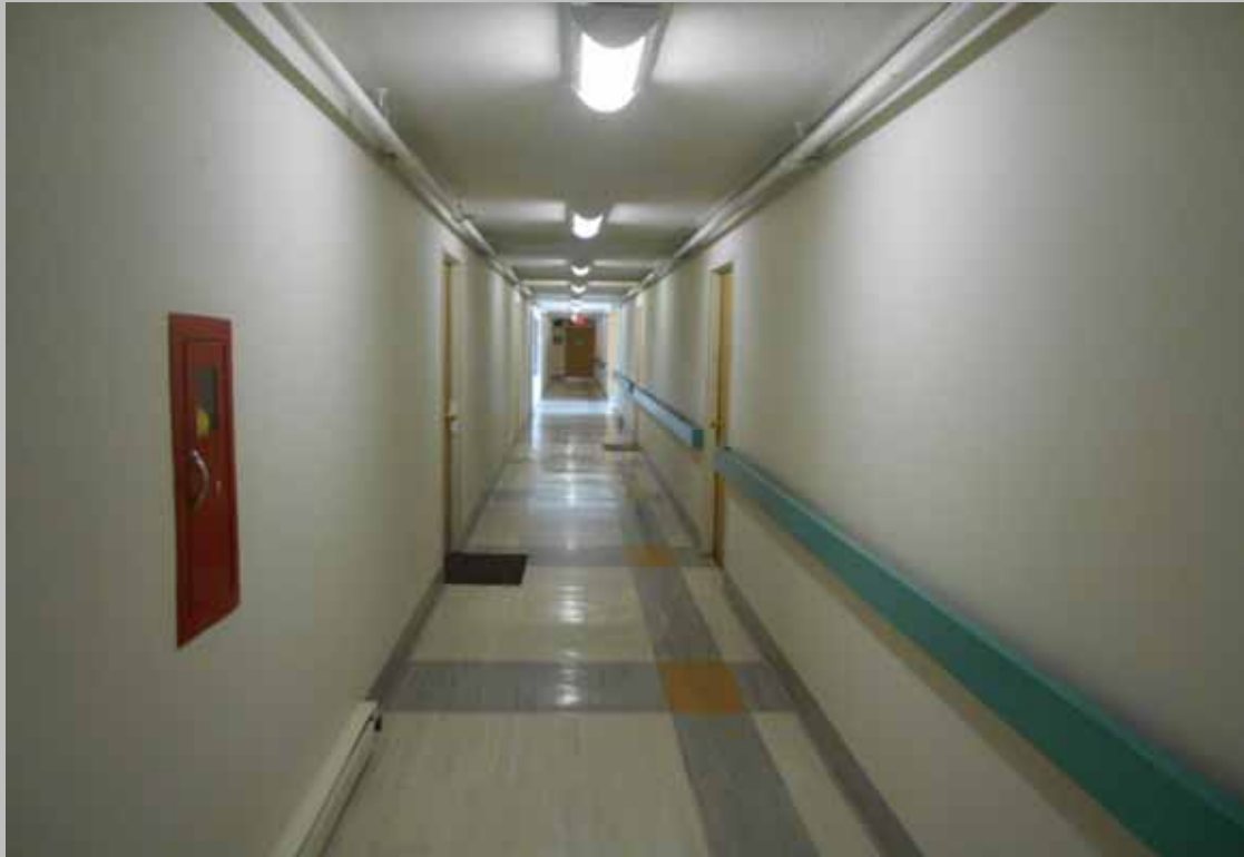
View of a common interior hallway
