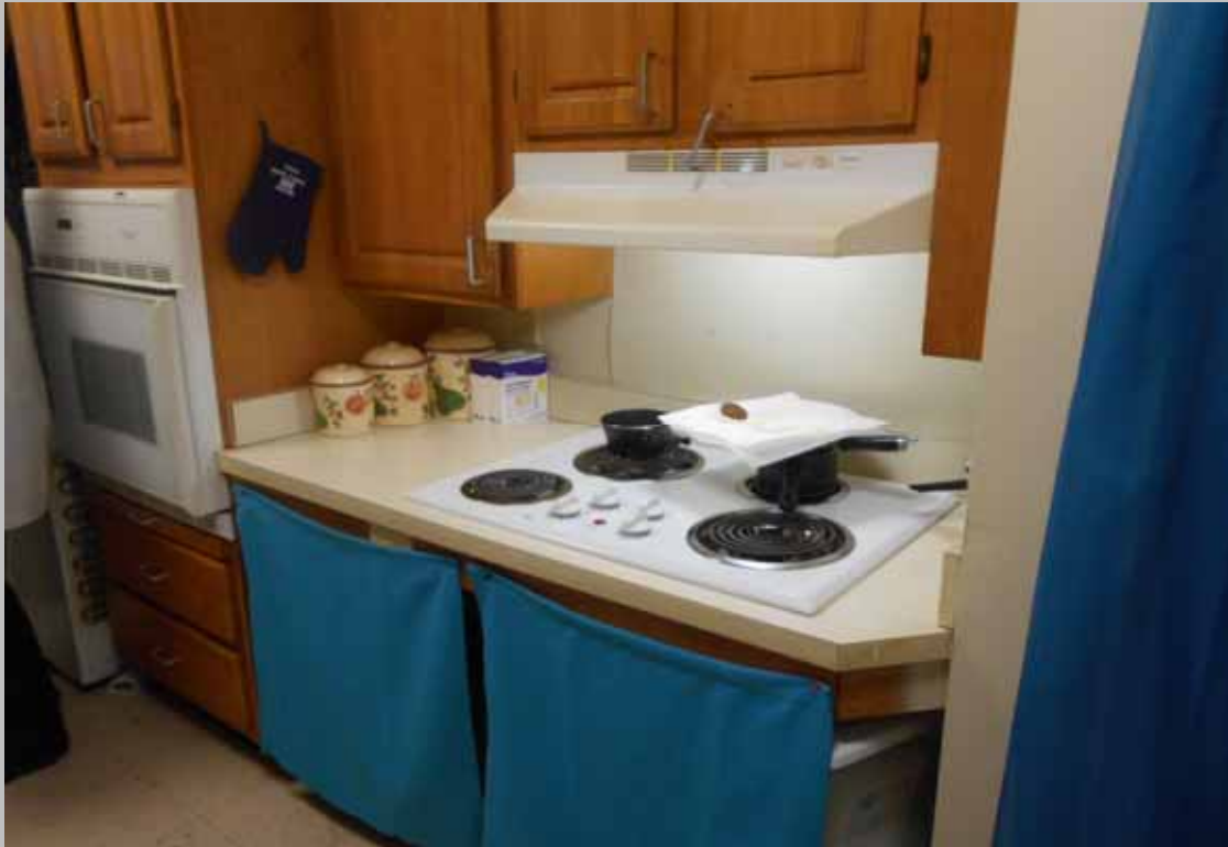
View of the roll-under stove-top and cabinet mounted oven within designated handicapped Unit 507
