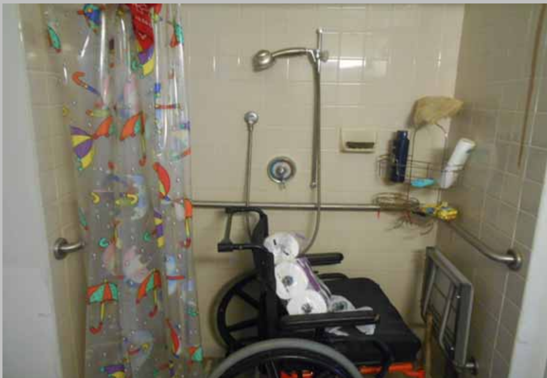
View of the roll-in shower within designated handicapped Unit 407 featuring compliant grab bars, levered hardware, and a 60-inch shower hose
