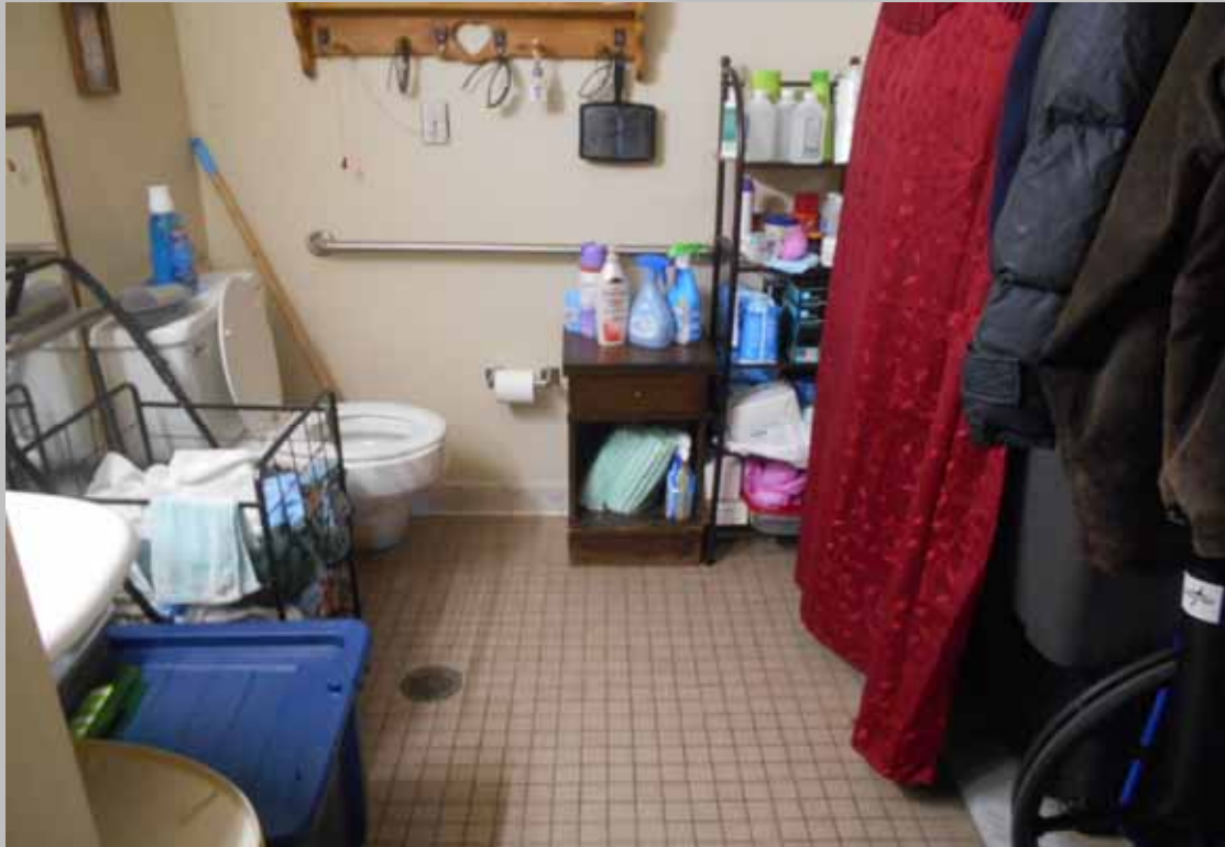
View of the bathroom within designated handicapped Unit 507 featuring compliant clear floor space, roll-under access to the sink, and side and rear grab bars at the toilet
