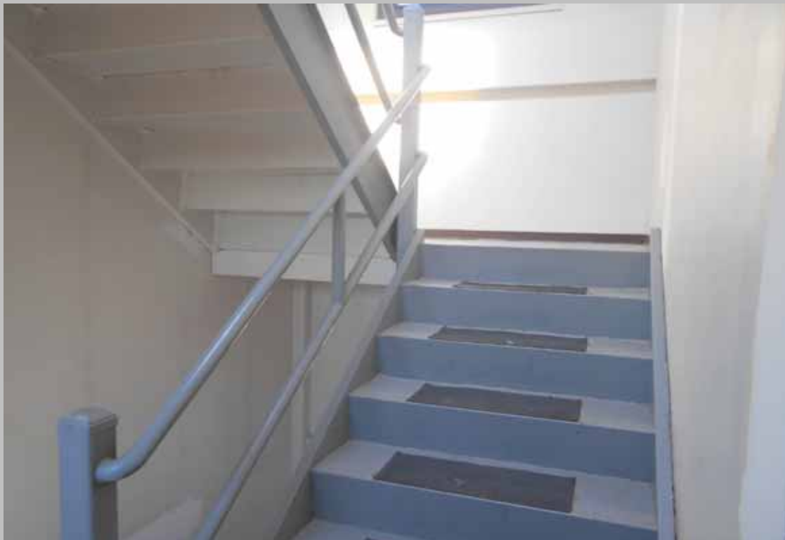
View of the interior stairwell leading to the roof access
