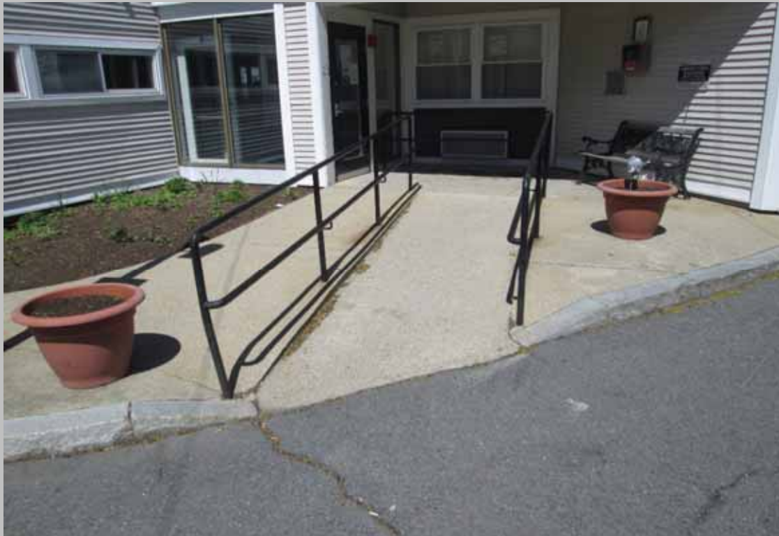
Community building entrance
