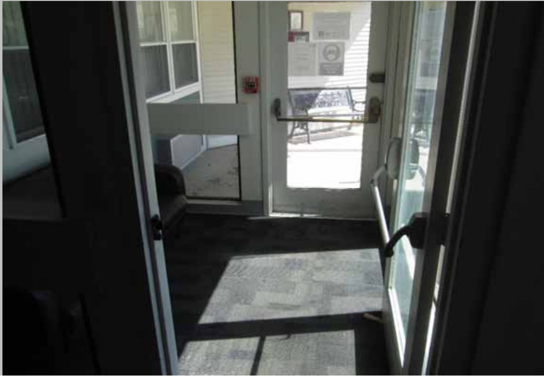
Compliant community building entrance - interior
