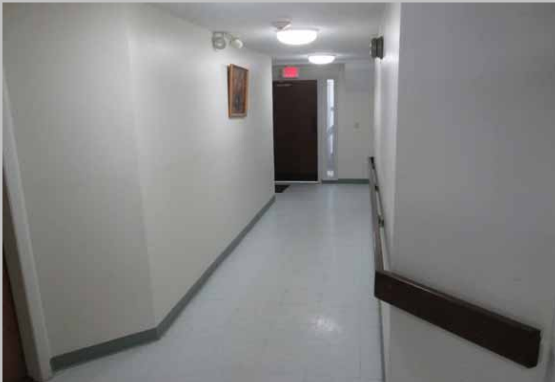
Building hallway view
