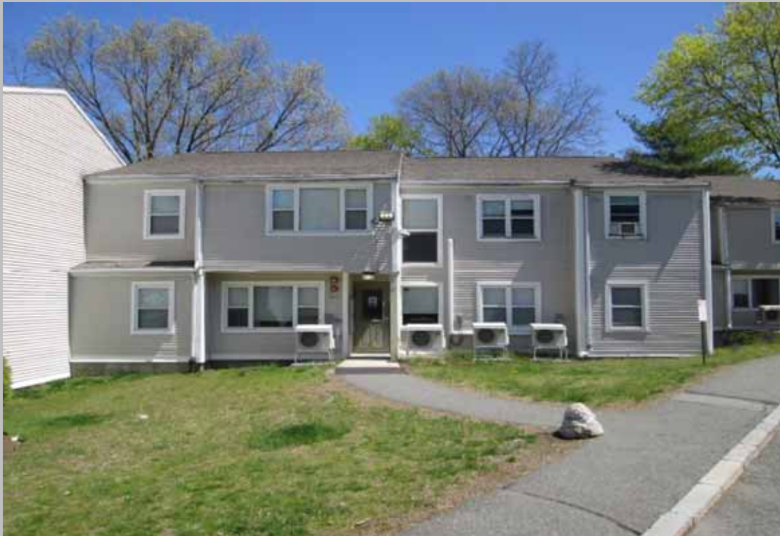
Additional front elevation view
