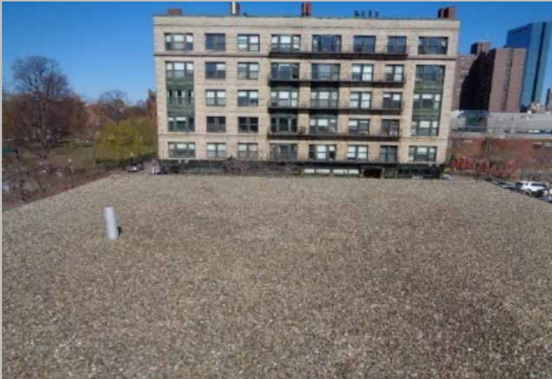
Apartment flat roof view
