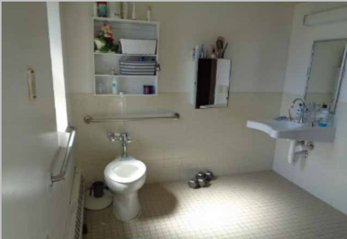
Accessible unit bathroom
