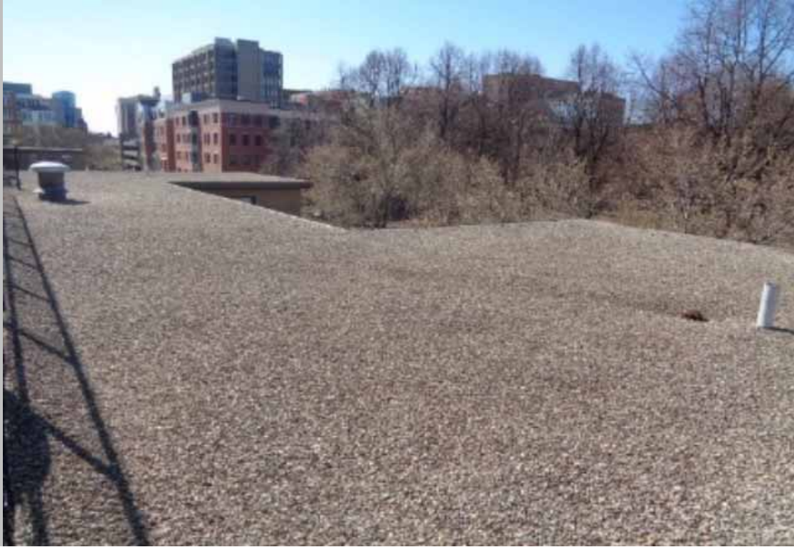
Flat roof view
