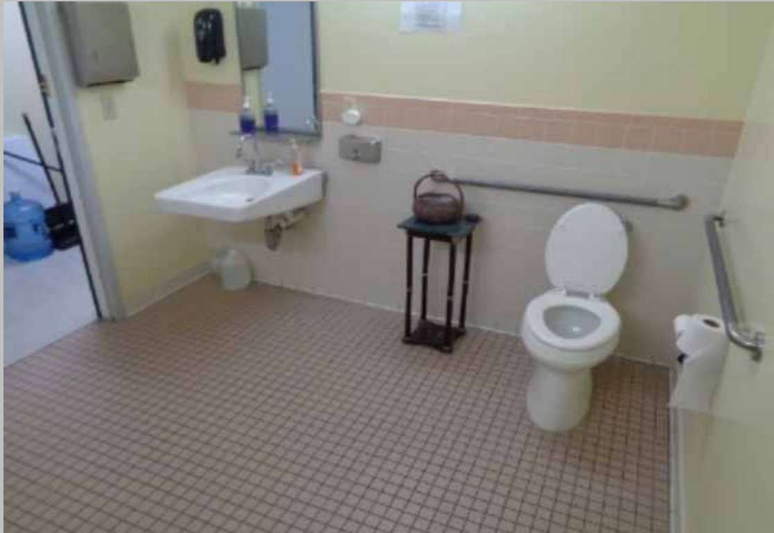
Typical common accessible restroom
