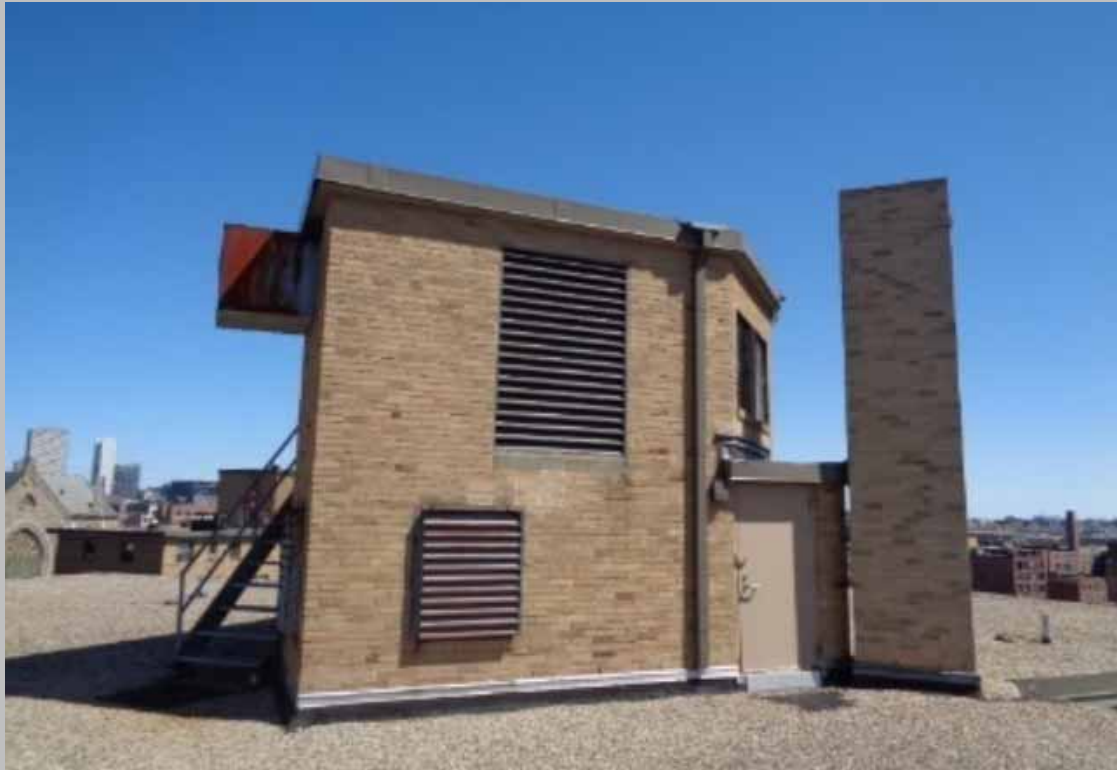
Hoist elevator rooftop mechanical room
