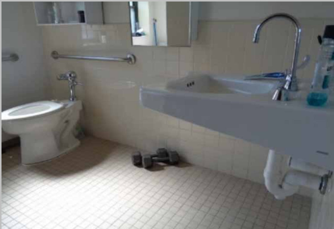
Accessible unit bathroom
