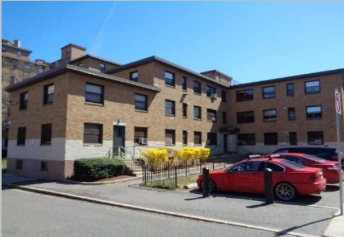
3-Story Walk-up and Townhome front view
