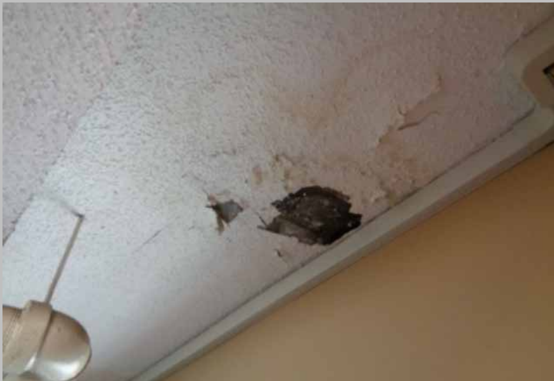
14 E Brookline hallway repair (Non-Critical Repair)
