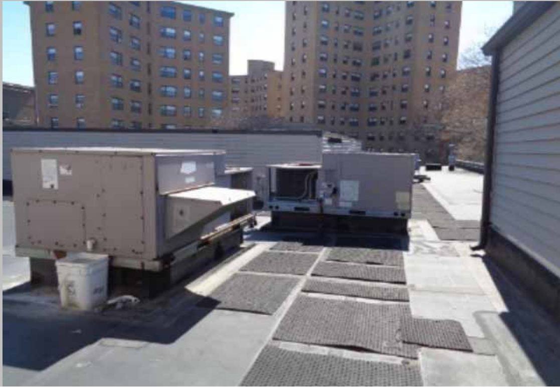
Community/leasing/maintenance building roof
