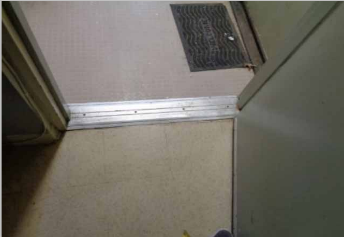
Accessible compliant threshold
