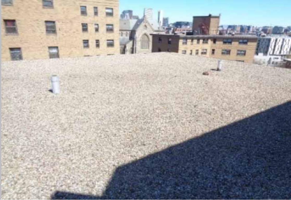
Additional flat roof view
