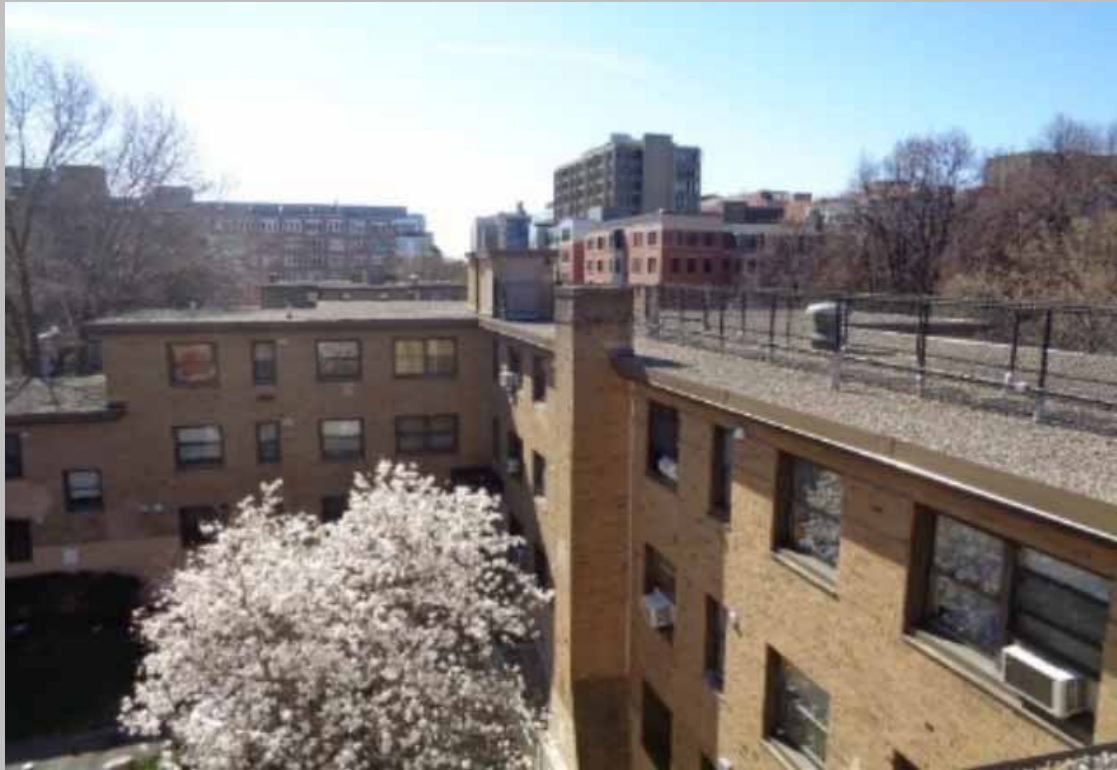
Building side elevation and flat roof view
