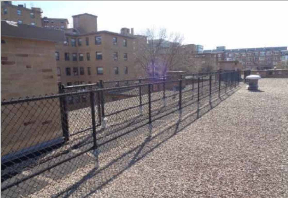
Chain-link security rooftop fencing
