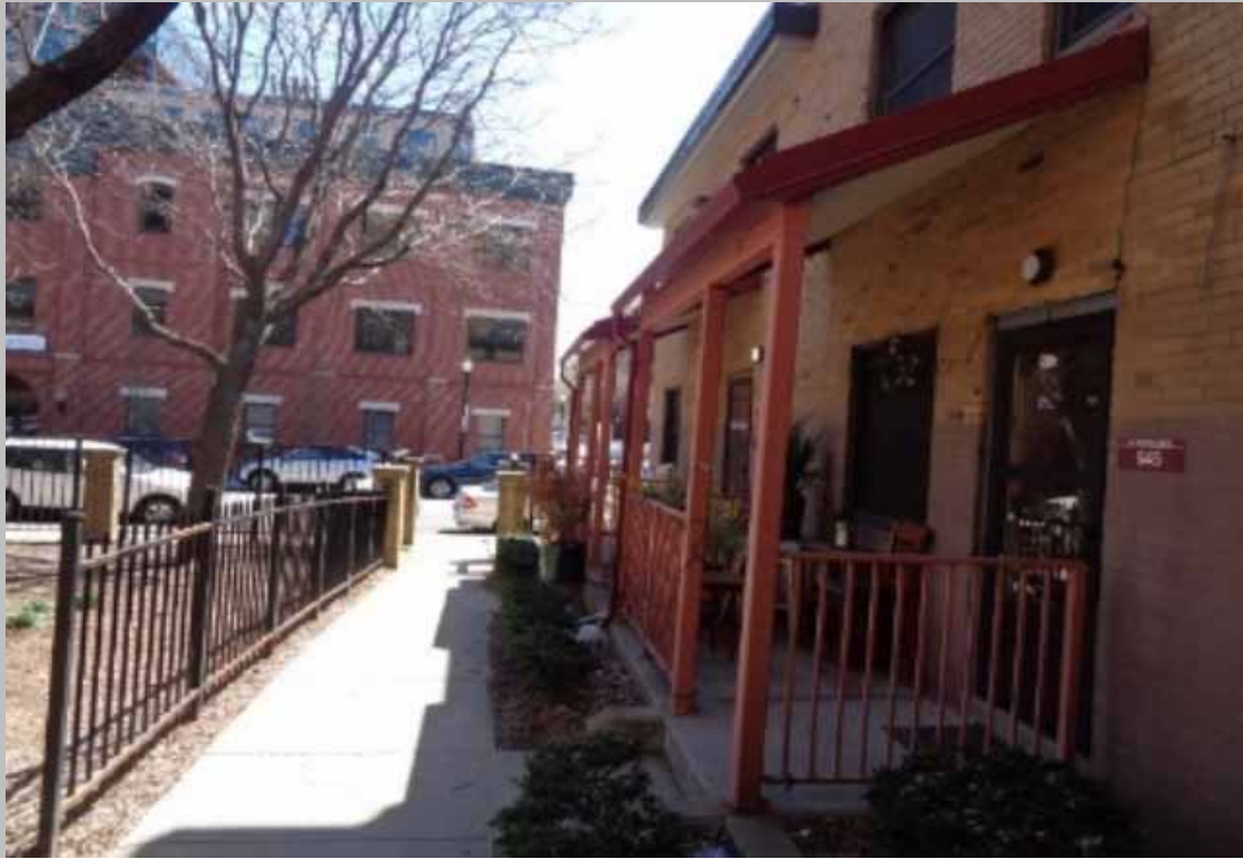
Townhome entry view
