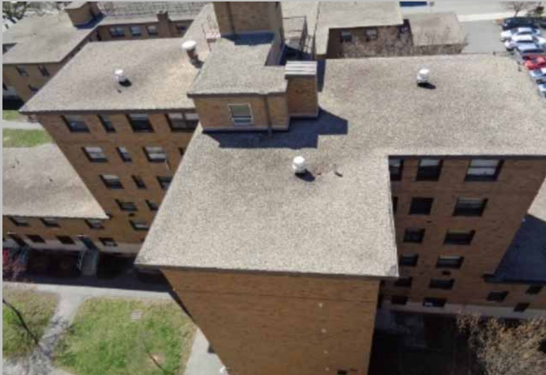
6-Story Building Rooftop view
