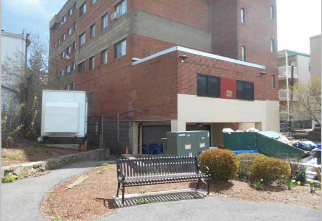
View of building exterior
