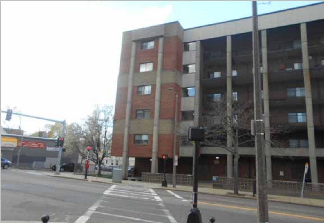
View of building exterior
