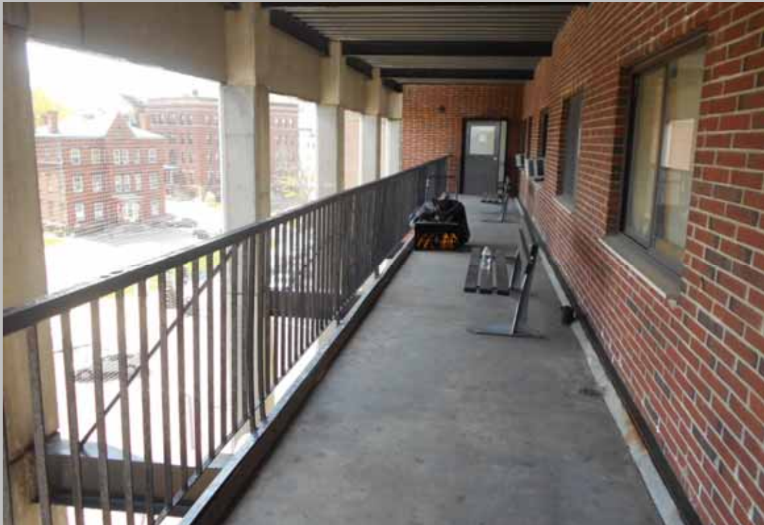
View of common exterior balcony
