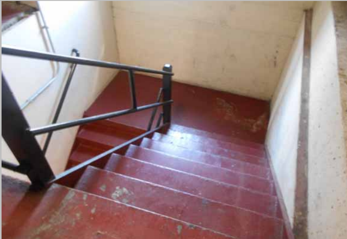
View of the maintenance stairwell leading to the roof-top
