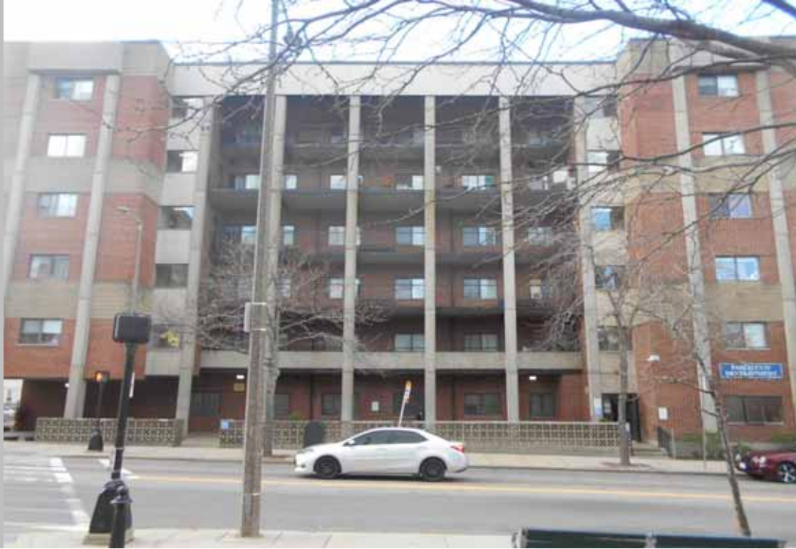
View of building exterior and balcony areas
