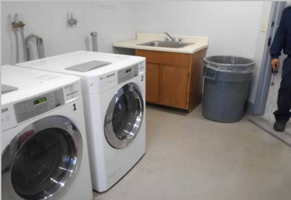
View of the non-compliant common area laundry room sink lacking roll-under access and levered handle hardware
