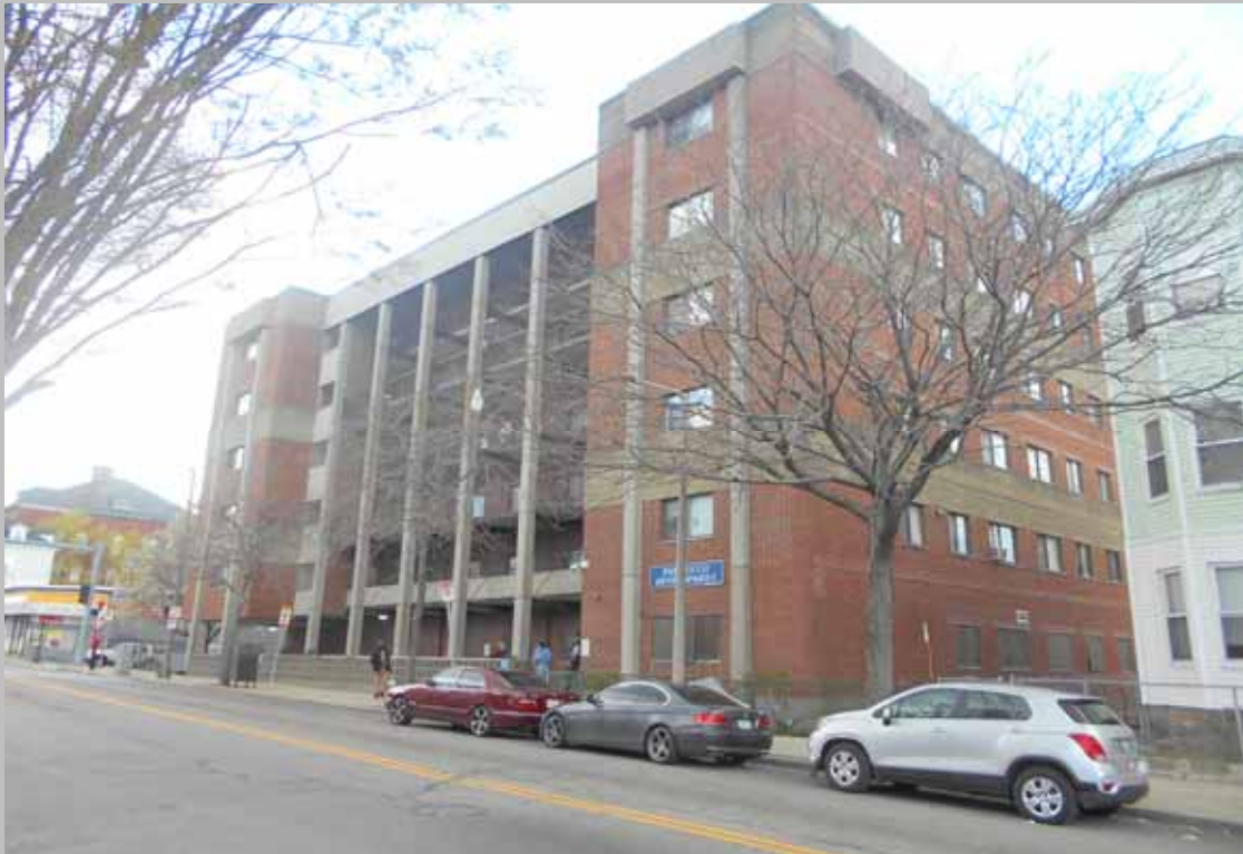
View of building exterior
