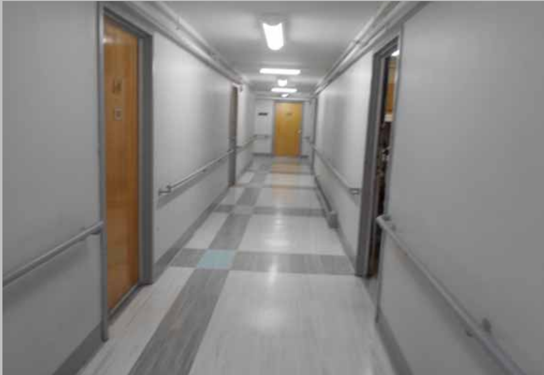
View of common interior hallway
