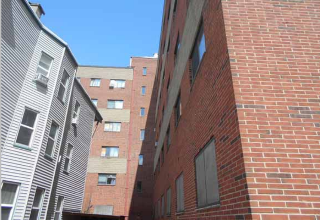
View of building exterior
