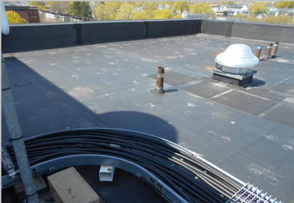
View of building roofing
