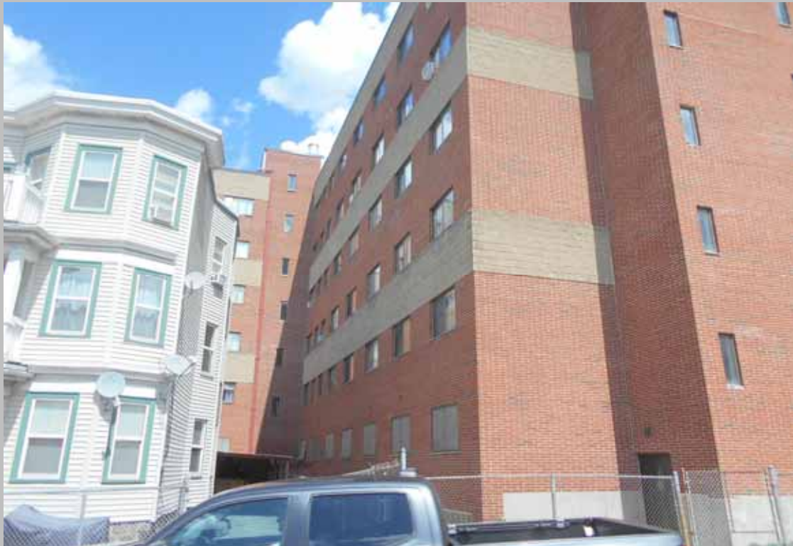
View of building exterior
