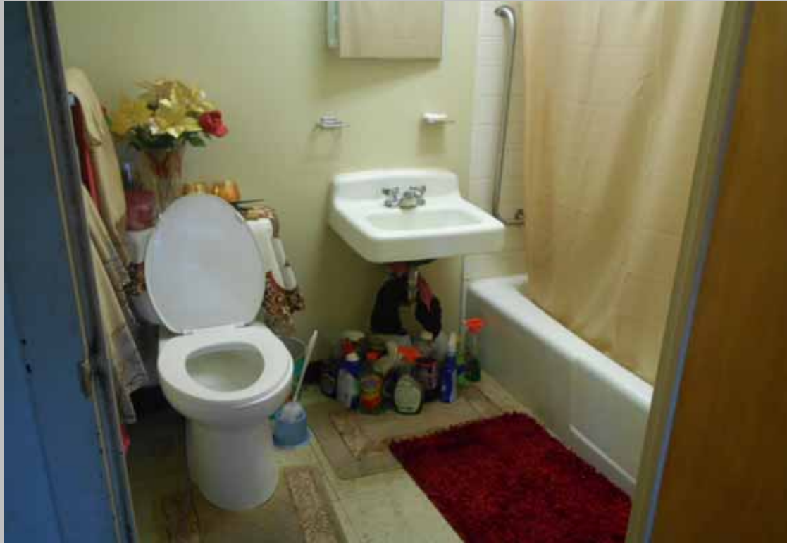
View of bathroom at Unit 502
