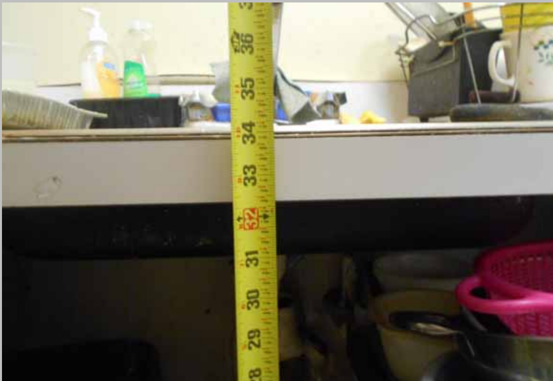
View of a compliant height kitchen counter-top within a designated handicapped dwelling unit
