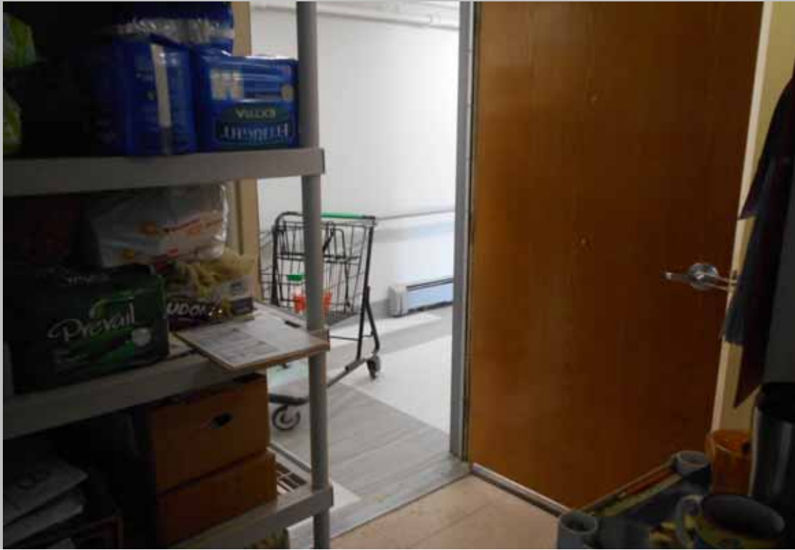
View of a typical entry area within a designated handicapped dwelling unit – featuring 18-inches at the pull-side and levered handle entry door hardware
