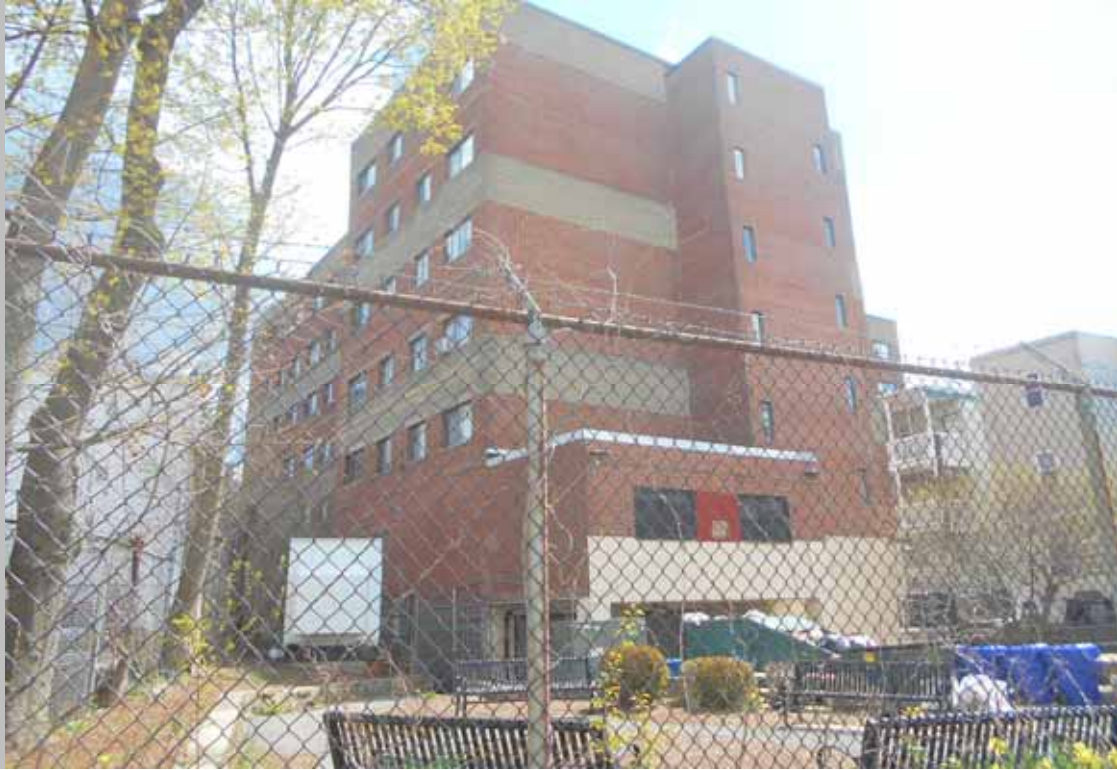
View of building exterior
