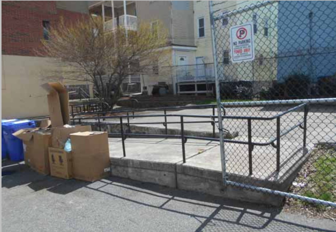
View of concrete ramp leading to the dumpsters (connected to the accessible route)
