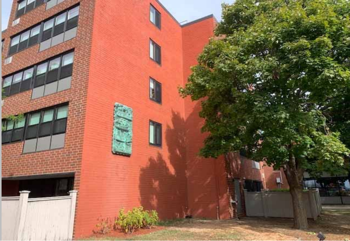
Typical building exterior
