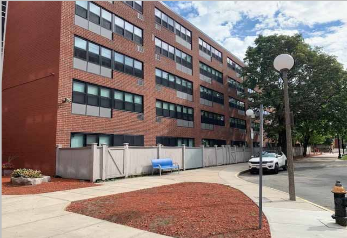
Typical building exterior
