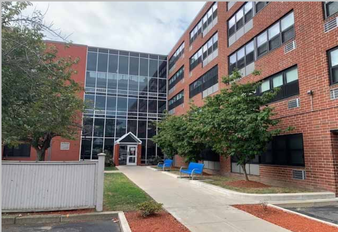
Typical building exterior
