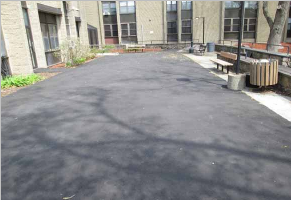
Rear common area asphalt patio
