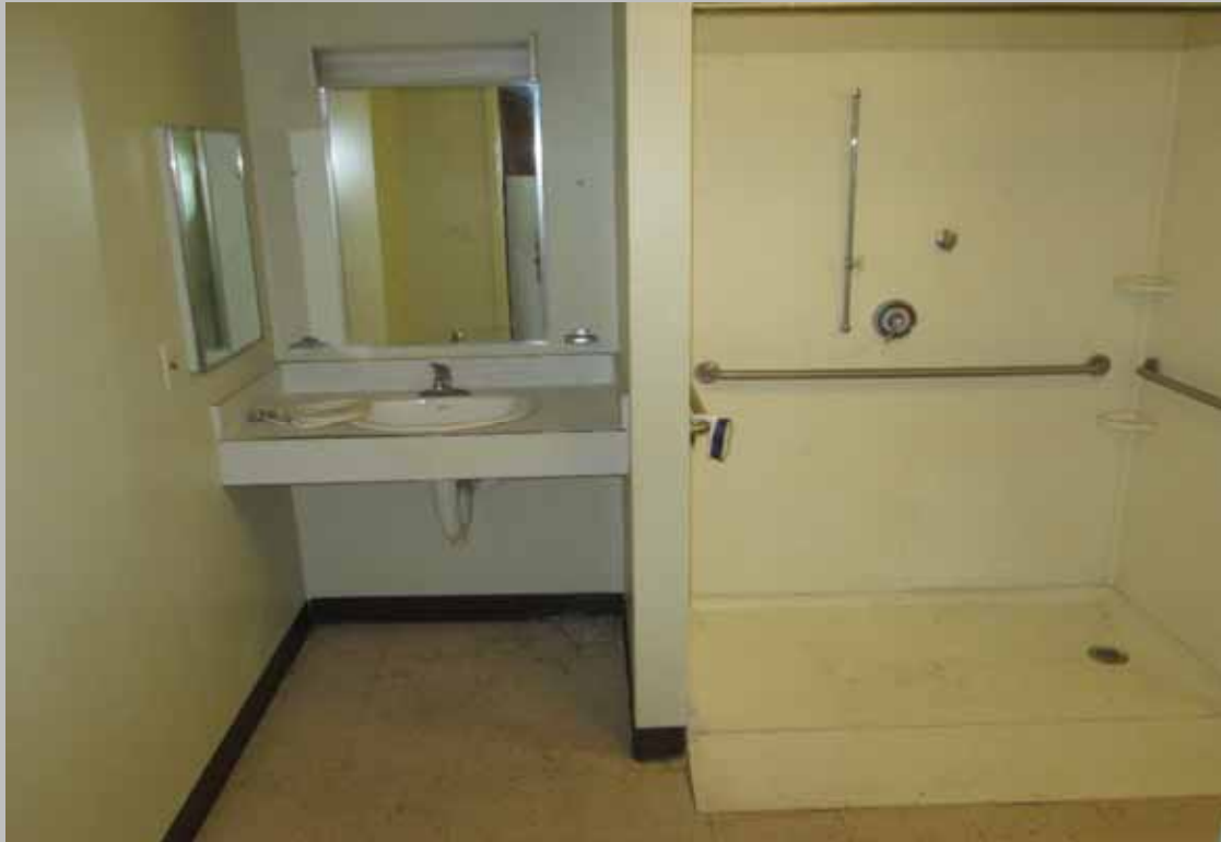
Designated handicapped unit bathroom
