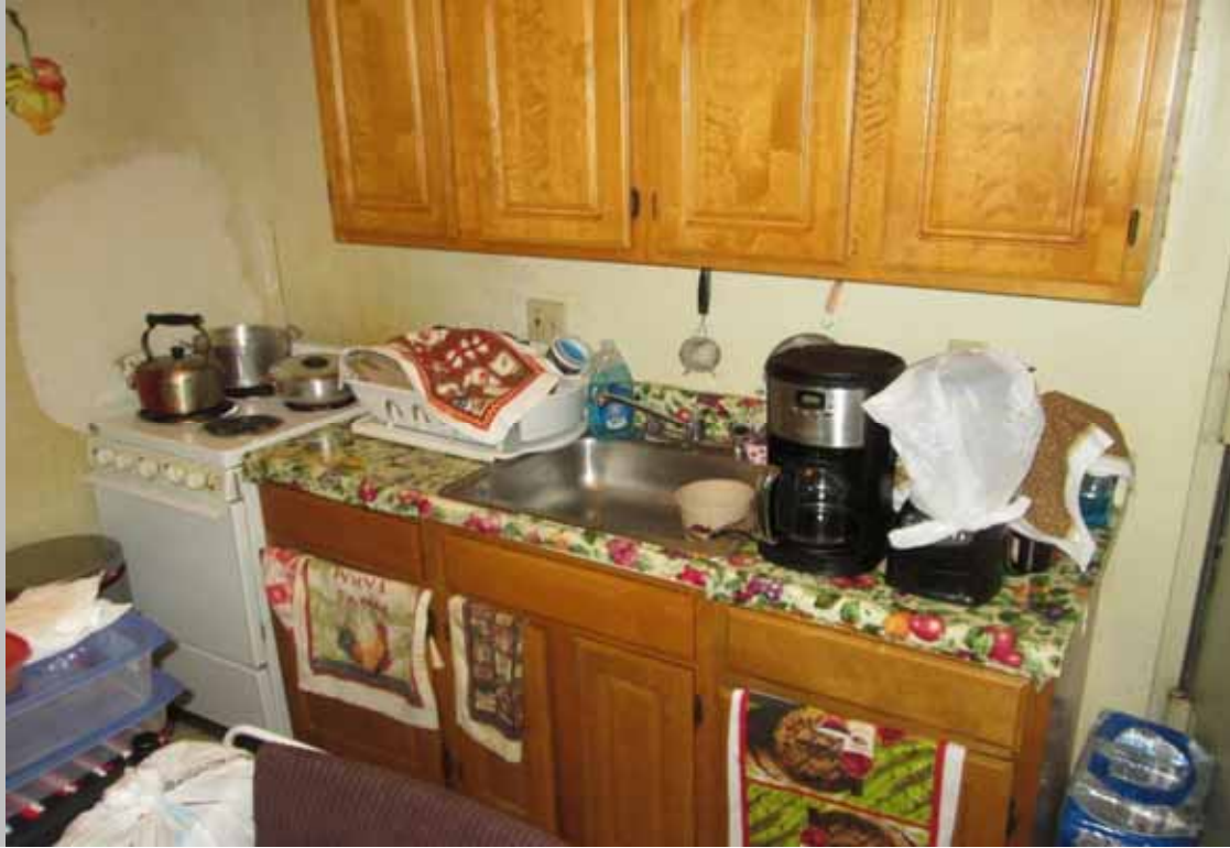
Dwelling unit cabinetry
