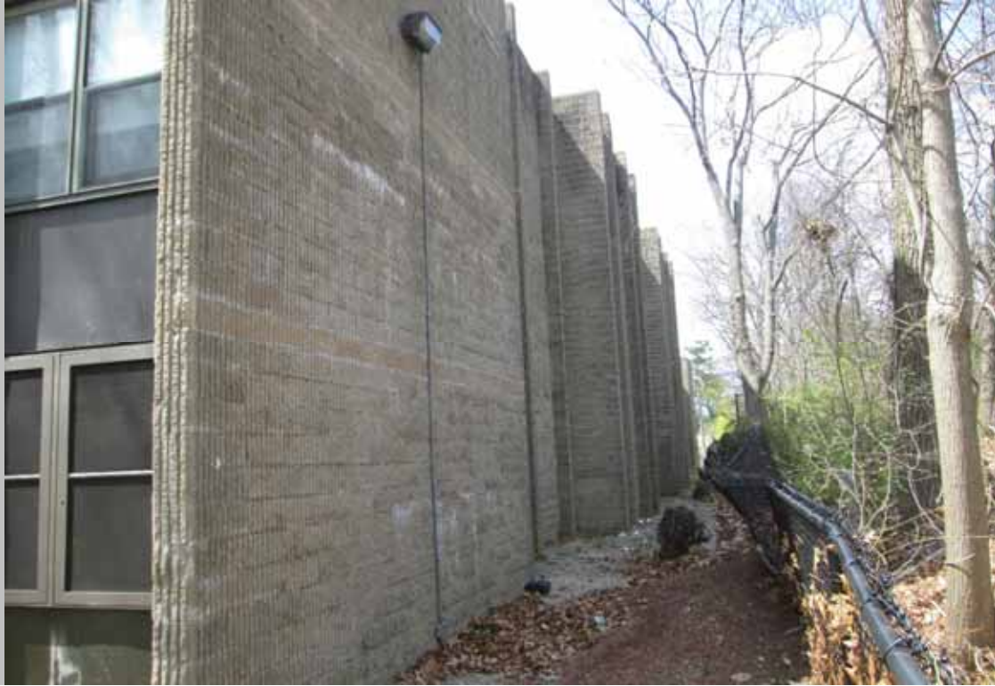
Damaged perimeter chain-link fencing (Non-Critical Repair)
