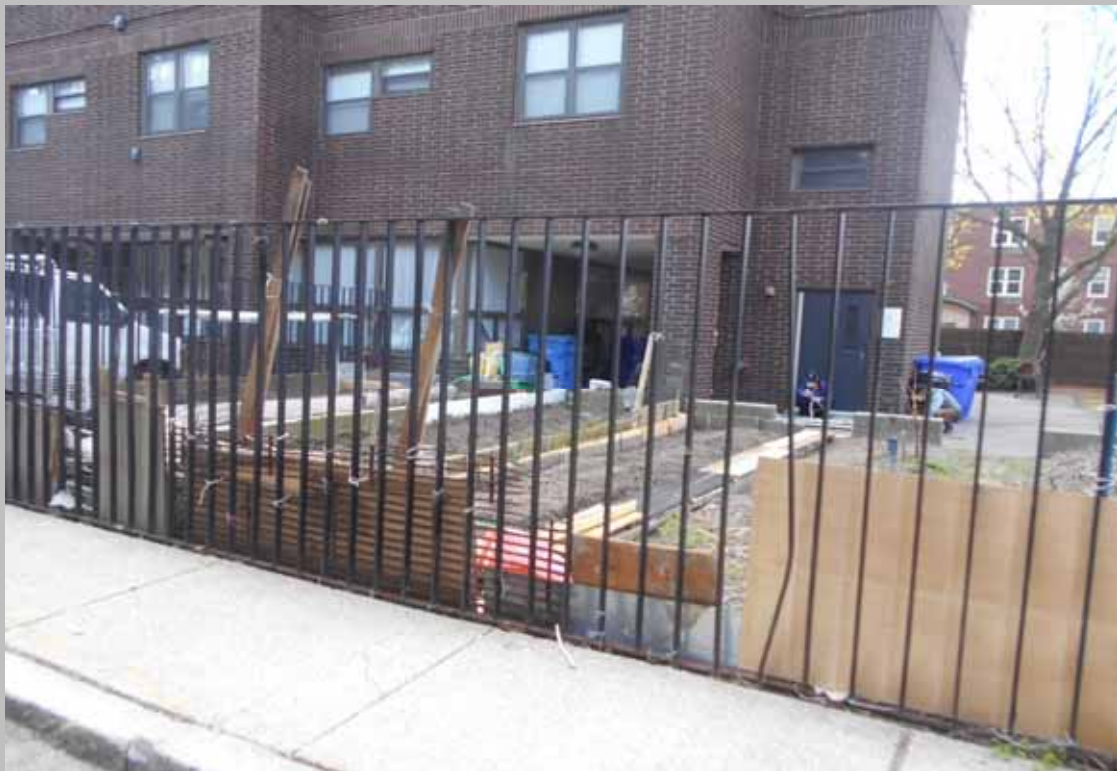
View of the damaged section of fencing outside of the community garden (Non-Critical Repair)
