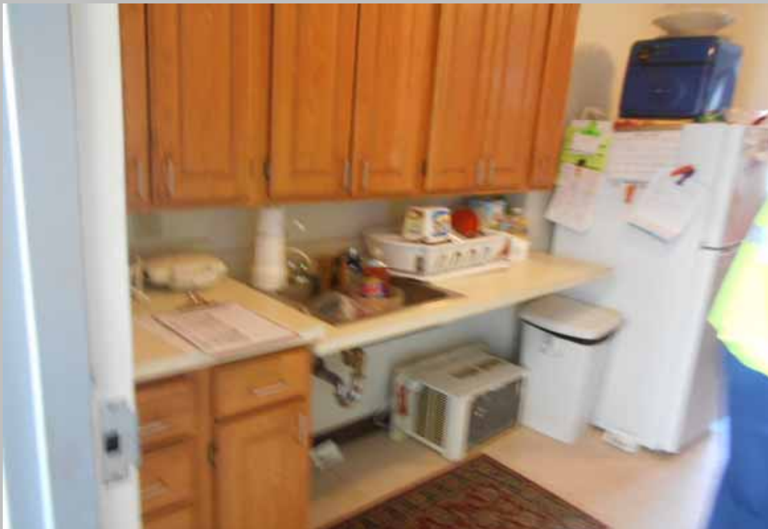
View of the kitchen within designated handicapped dwelling unit 607 – featuring a compliant roll-under sink and lowered cabinetry
