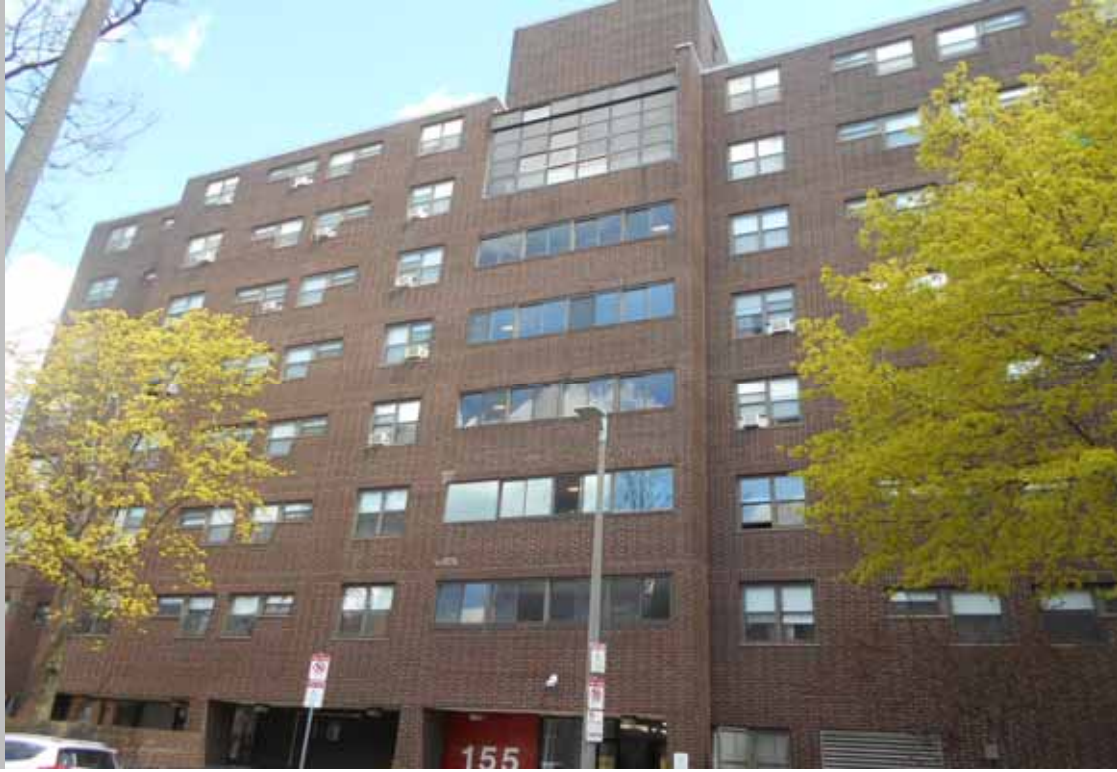
View of building exterior
