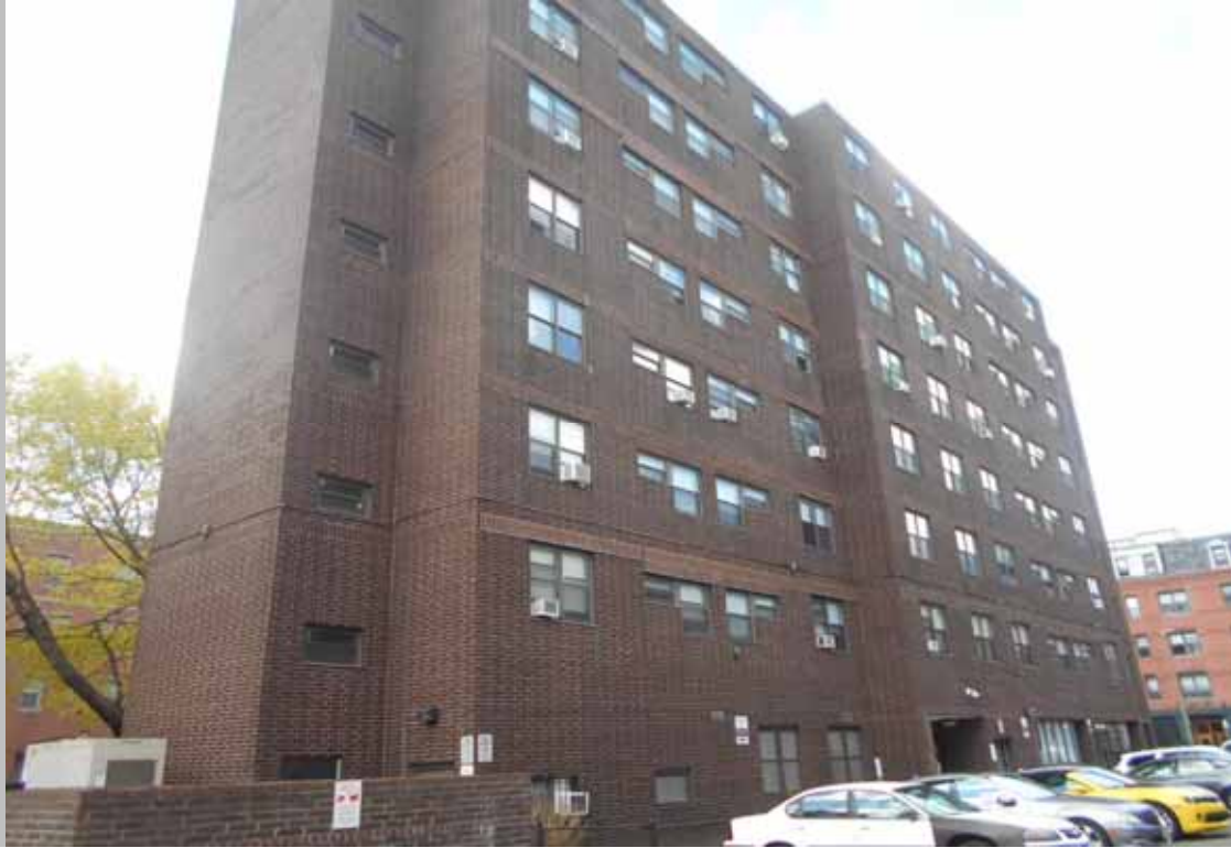
View of building exterior
