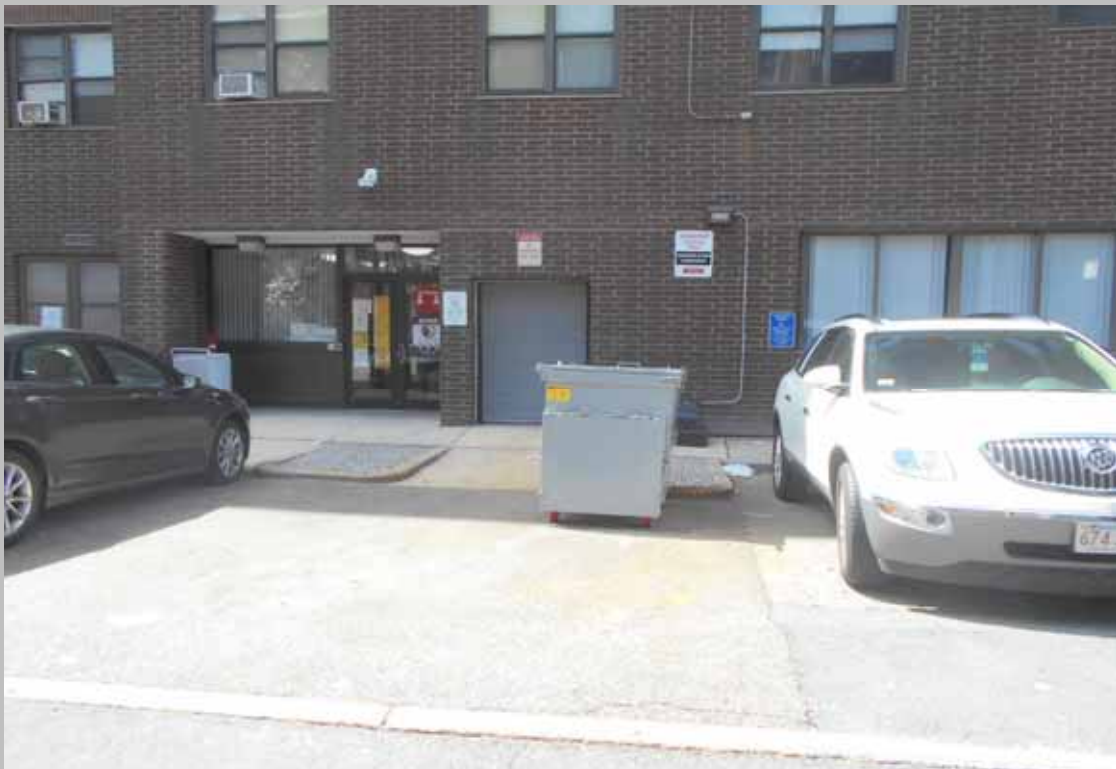
View of the designated handicapped parking space at the property (Critical Repair)
