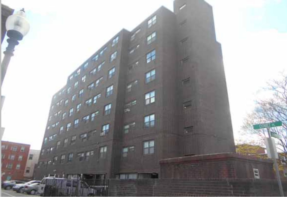
View of building exterior
