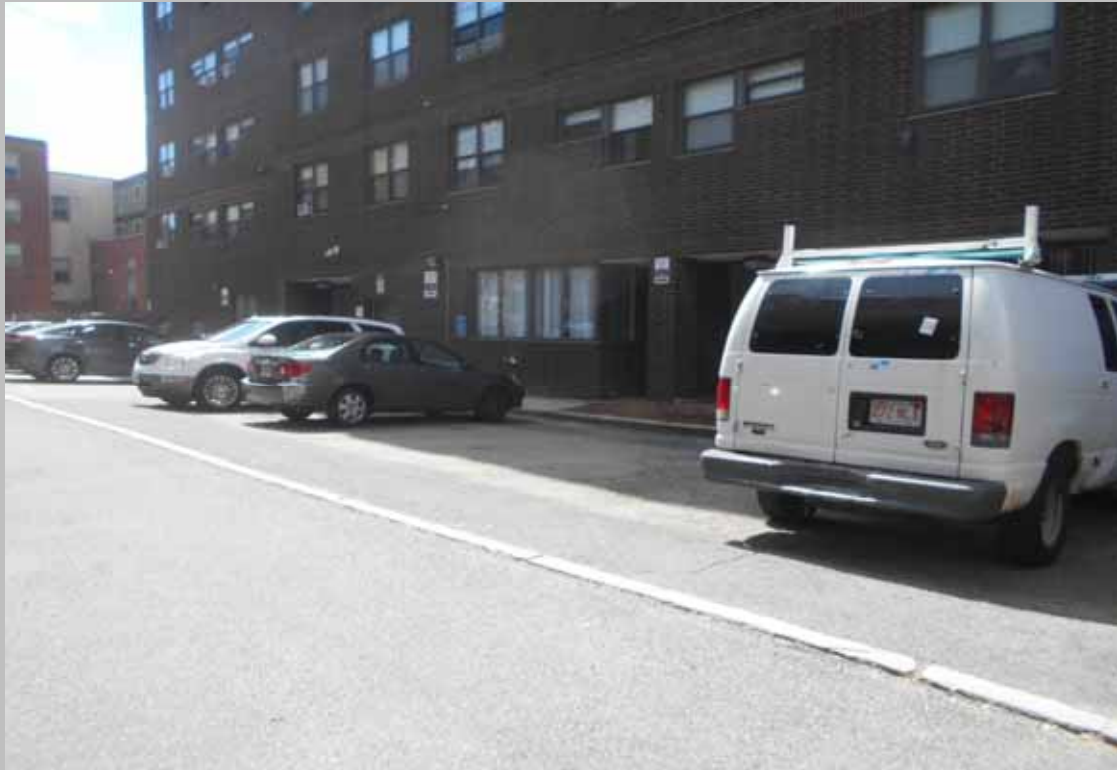
View of asphalt parking surface
