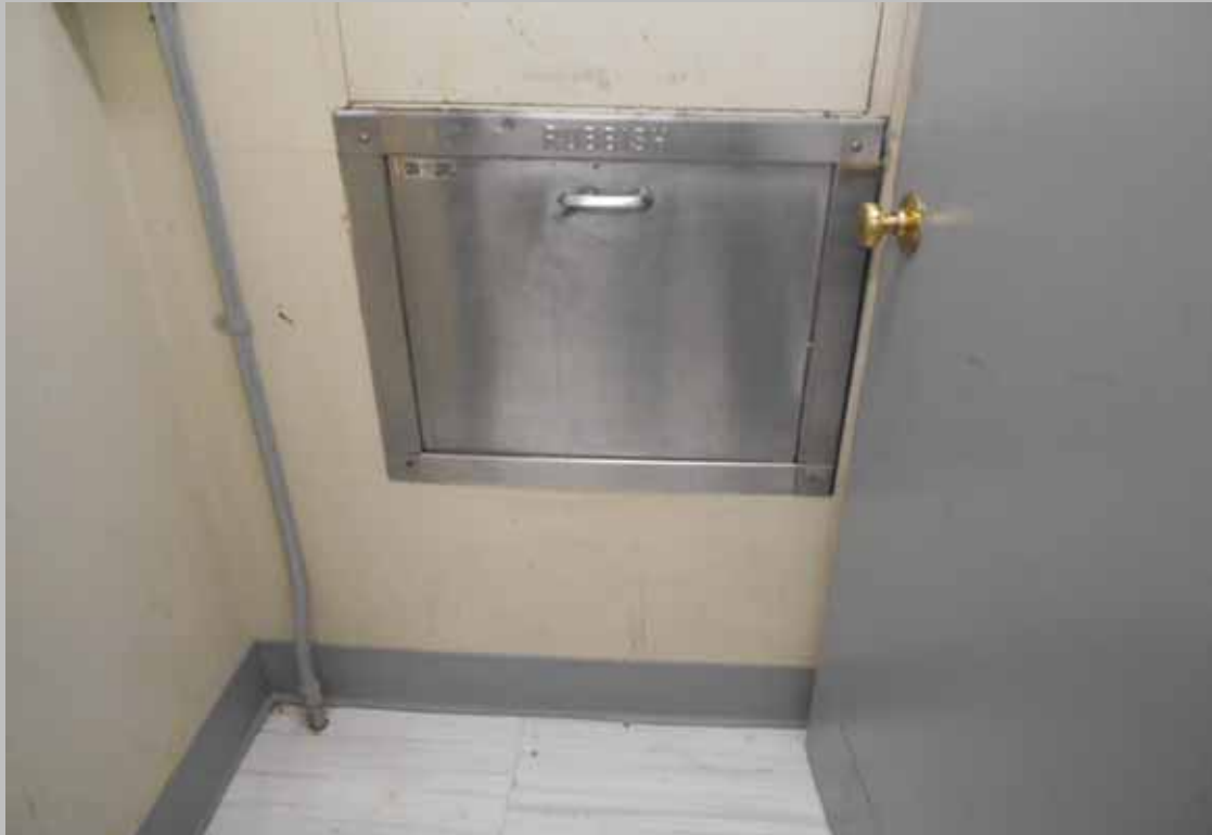
View of a trash chute room
