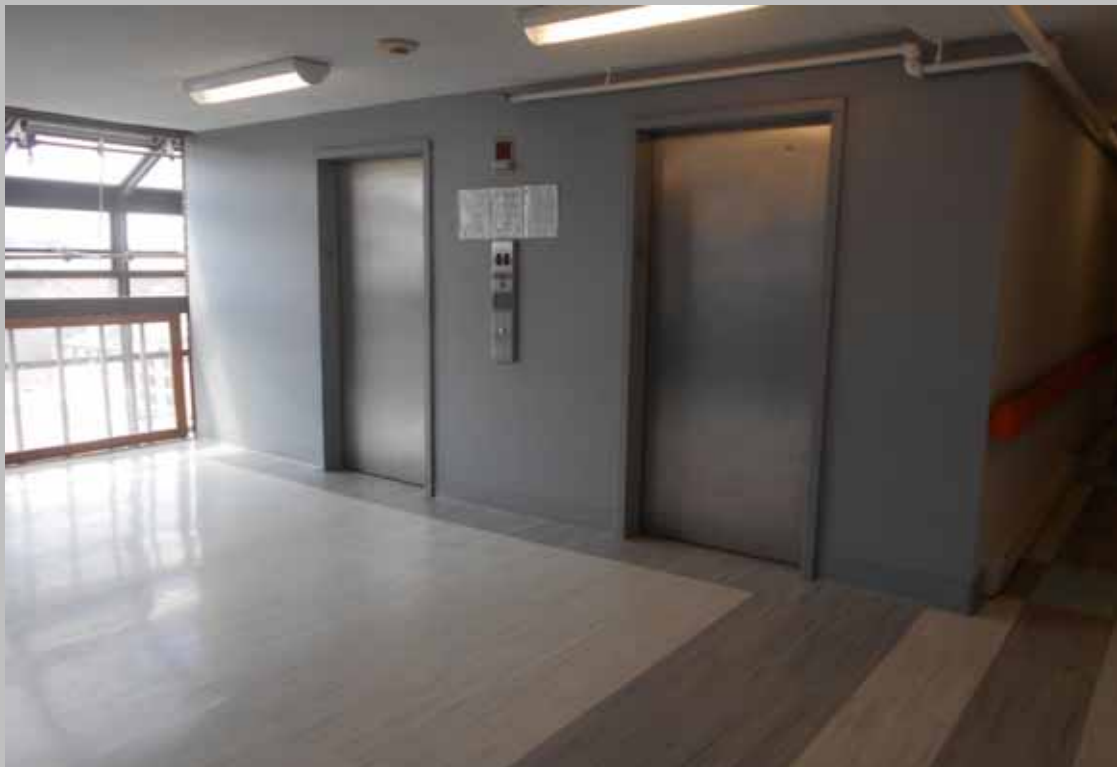
View of elevator lobby
