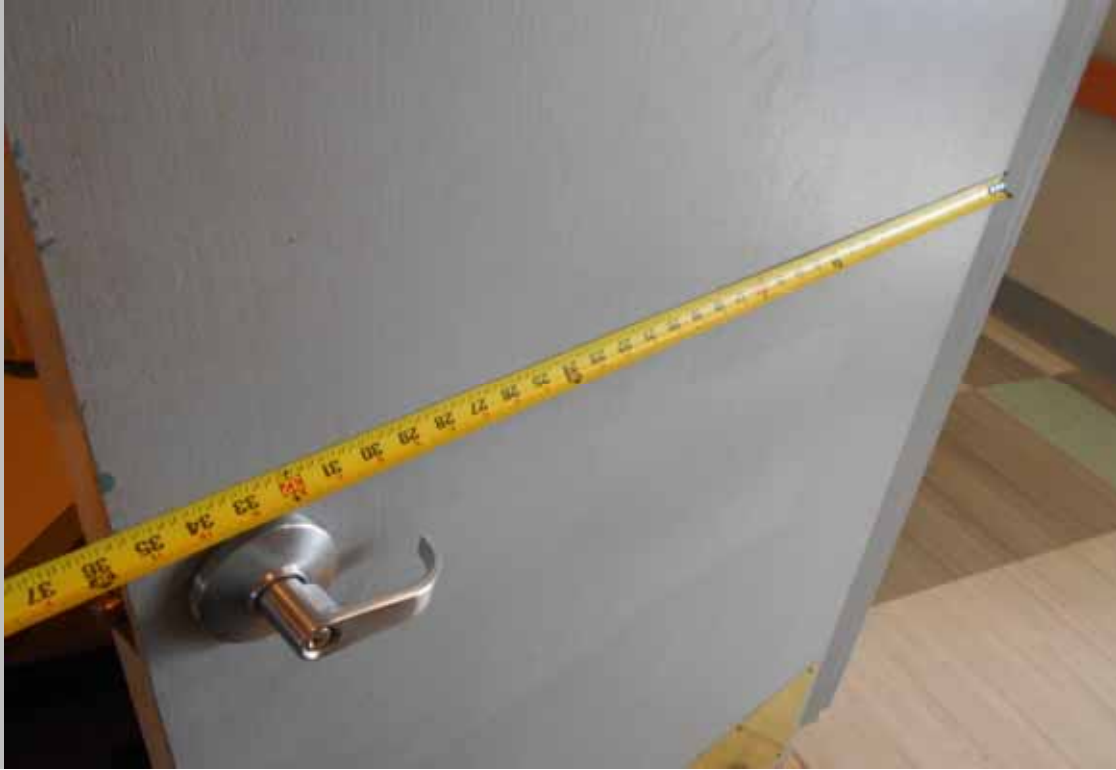
View of the compliant entry door at designated handicapped dwelling unit 607
