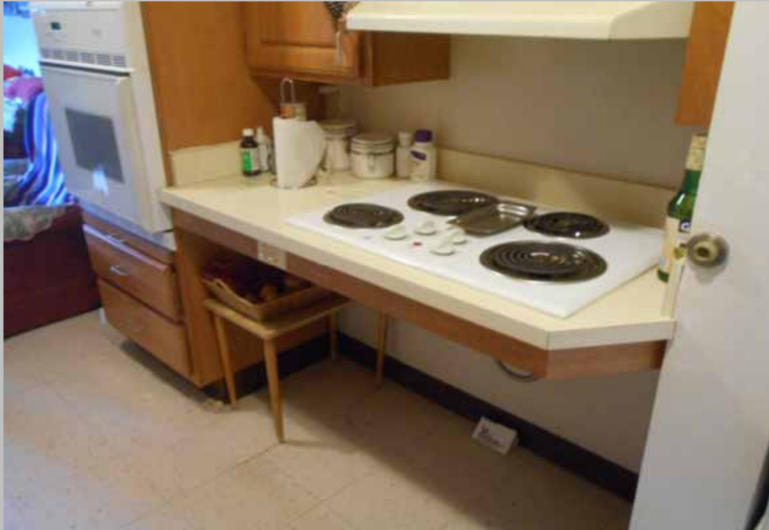
View of the kitchen within designated handicapped dwelling unit 607 - featuring a roll-under electric range
