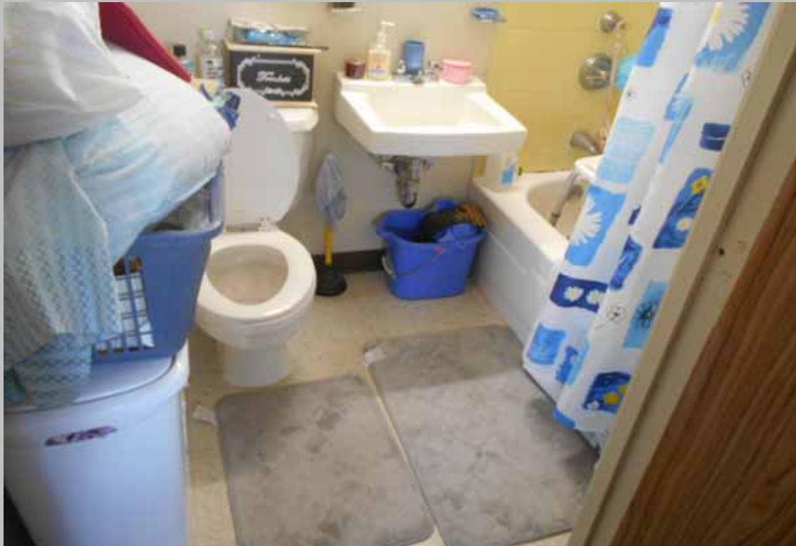
View of bathroom at Unit 803
