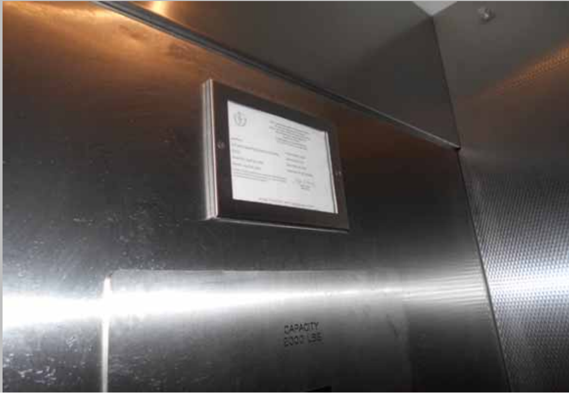
View of an elevator cab
