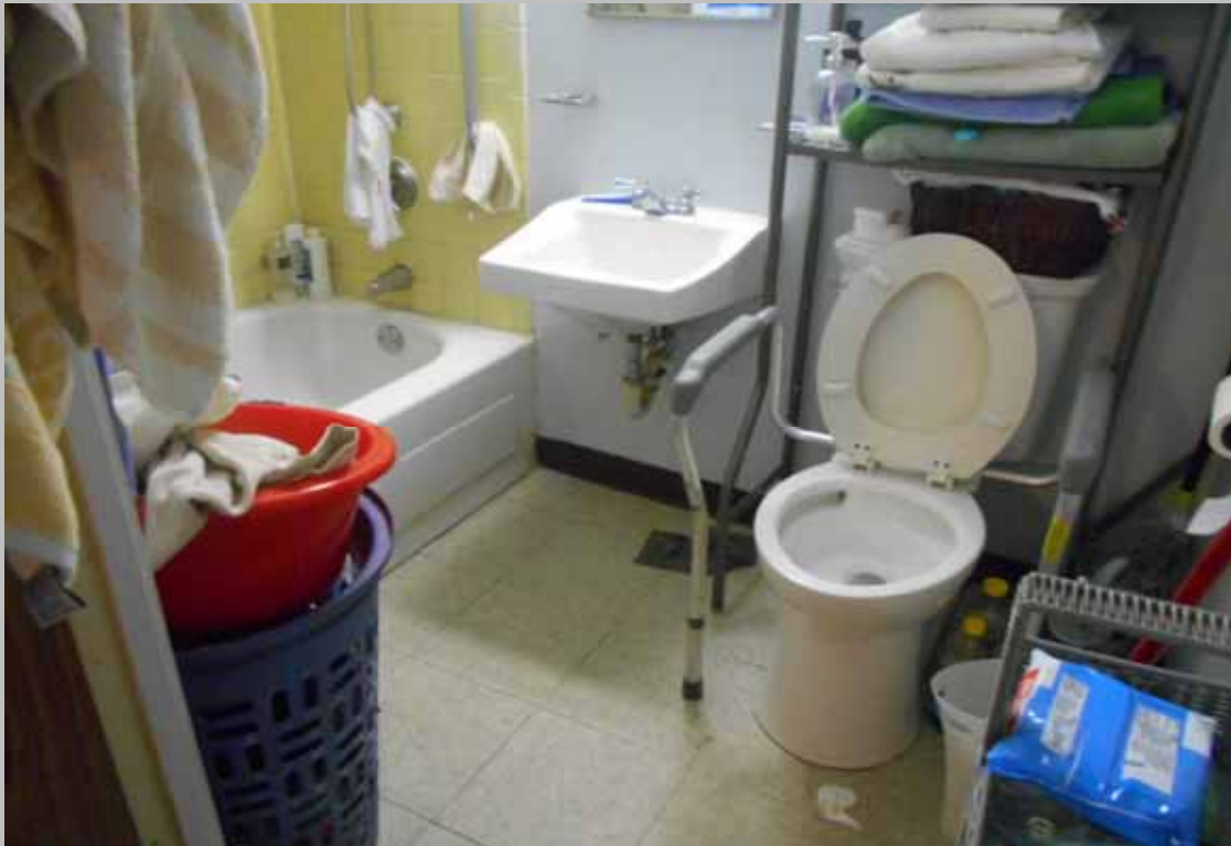
View of bathroom at Unit 702
