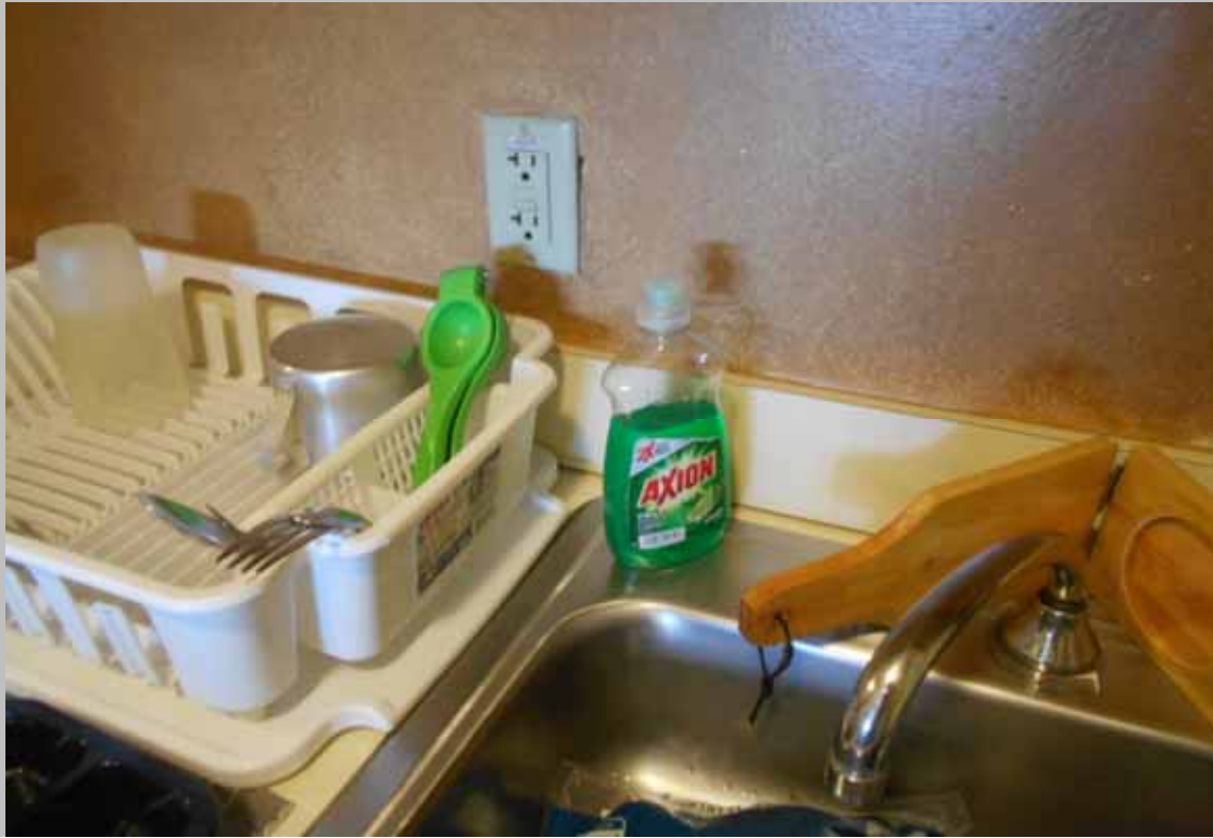
View of GFCI electrical outlet – dwelling unit
