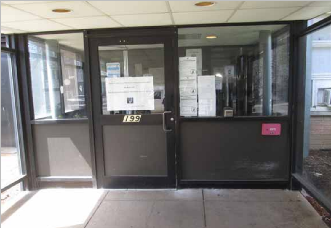
Main building entry doors/vestibule area
