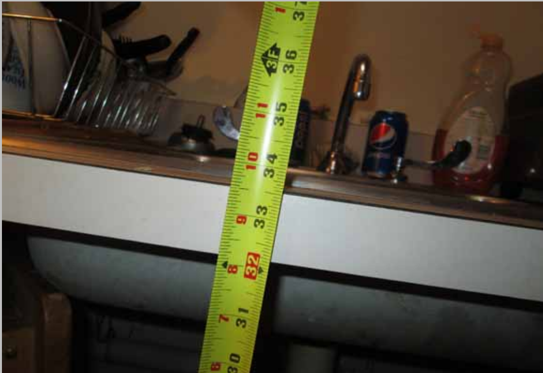
HC unit with compliant kitchen countertop/sink height
