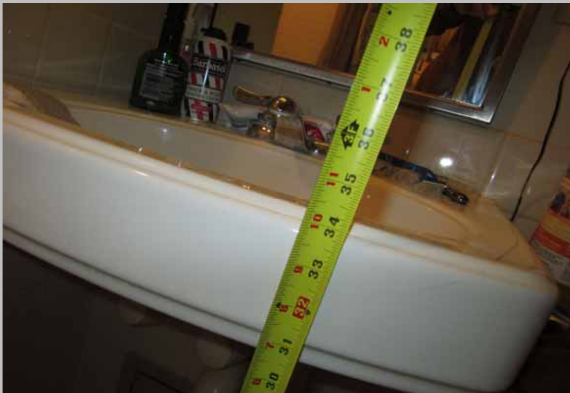
HC unit with compliant bathroom sink height
