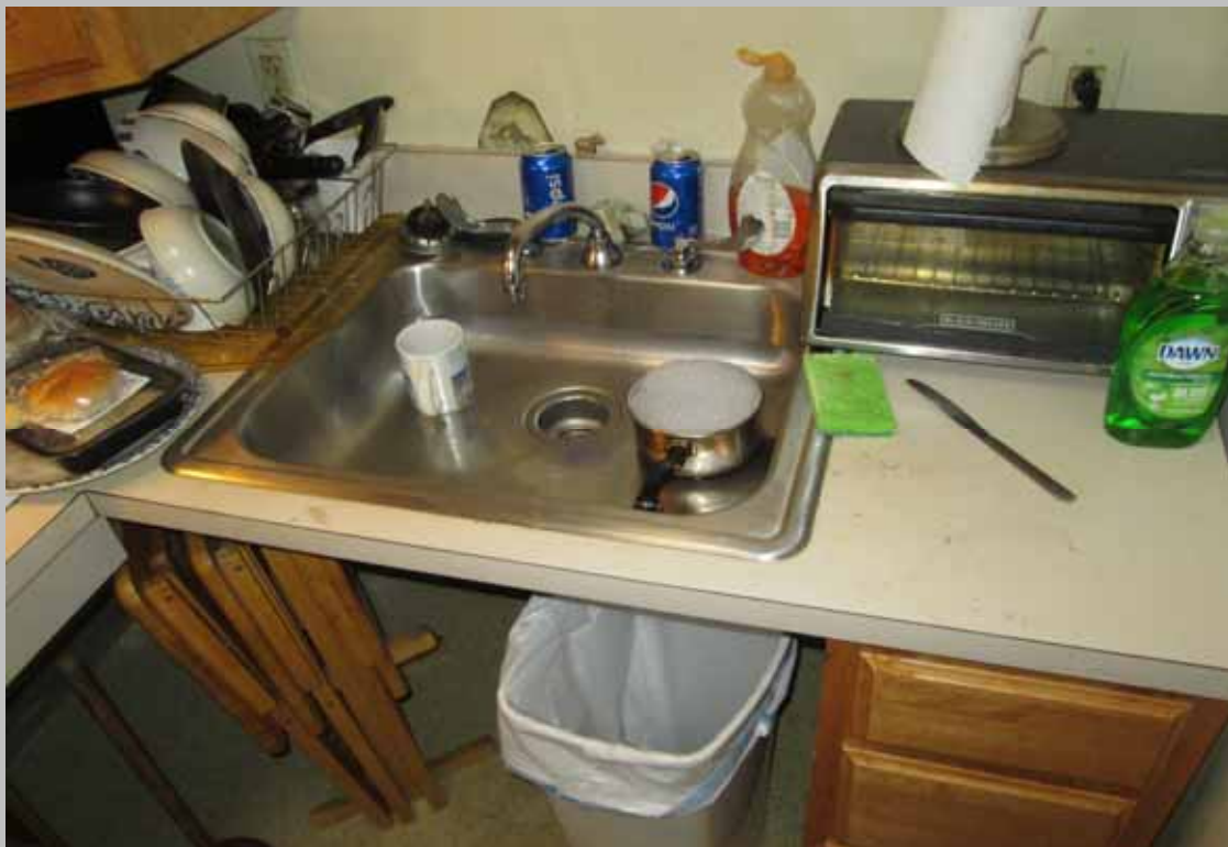
HC unit with compliant kitchen sink roll-under access and levered faucet hardware
