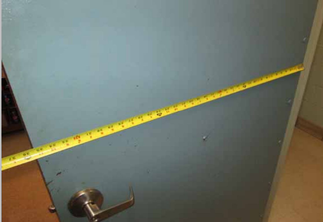
Handicapped (HC) dwelling unit with compliant entry door
