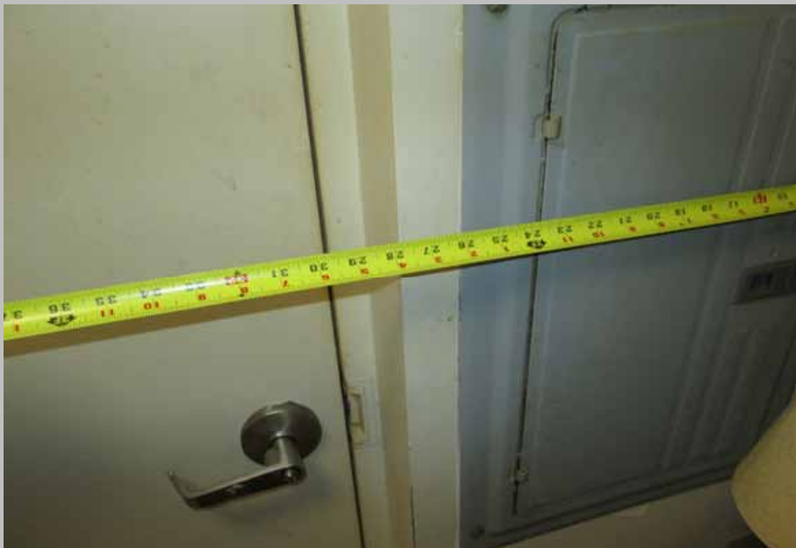
HC unit with compliant clear maneuvering space at entry door
