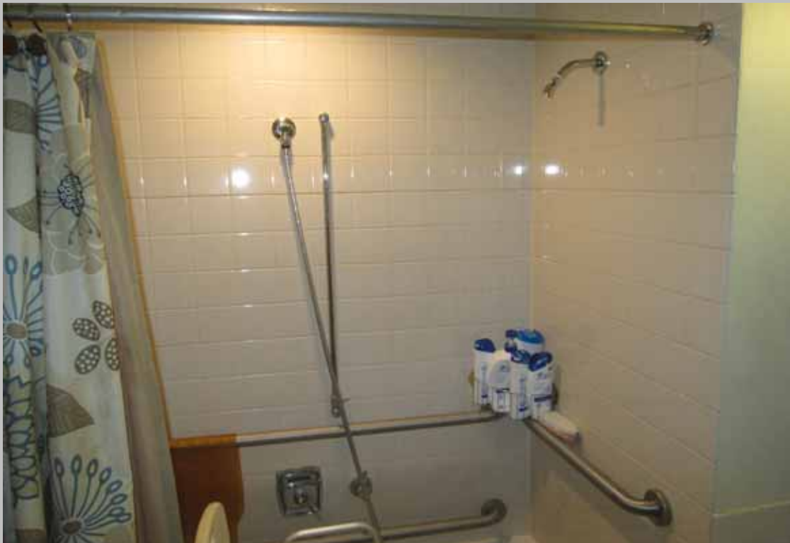
HC unit tub with compliant 60-inch shower spray unit
