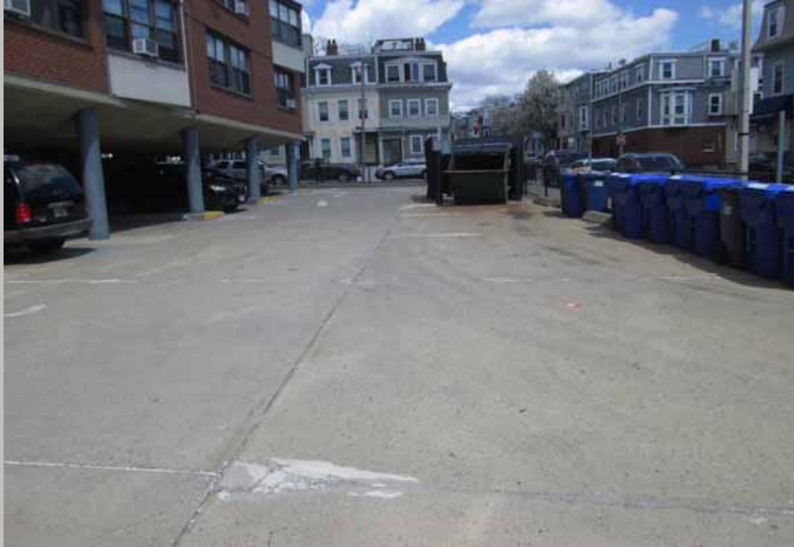
Concrete drive aisle
