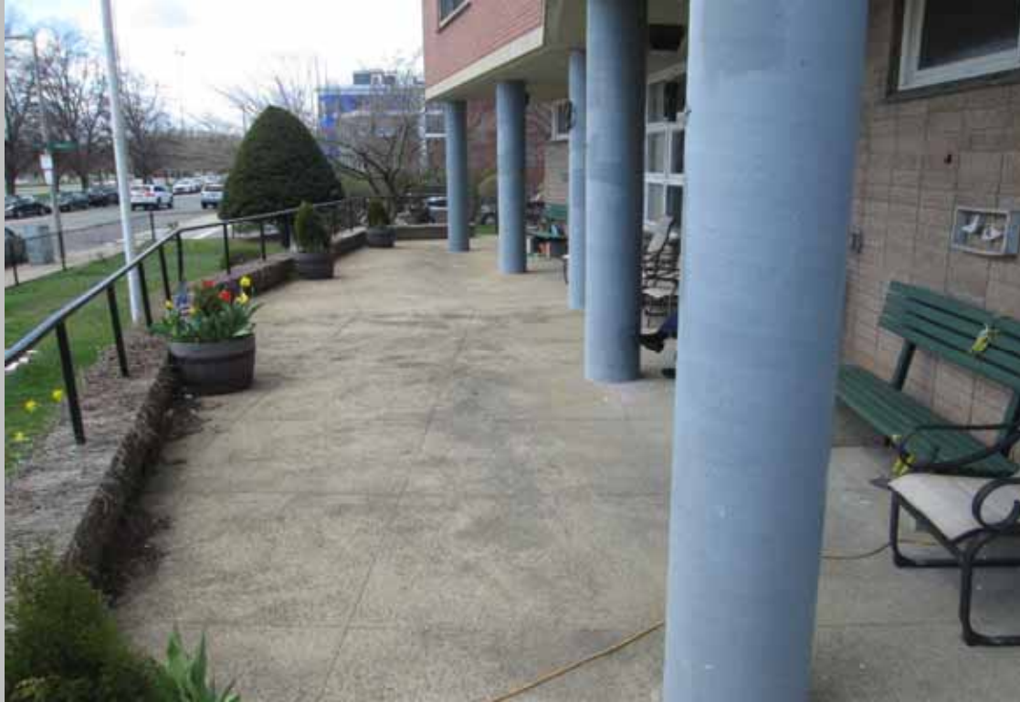
Patio/sitting area on south side of building
