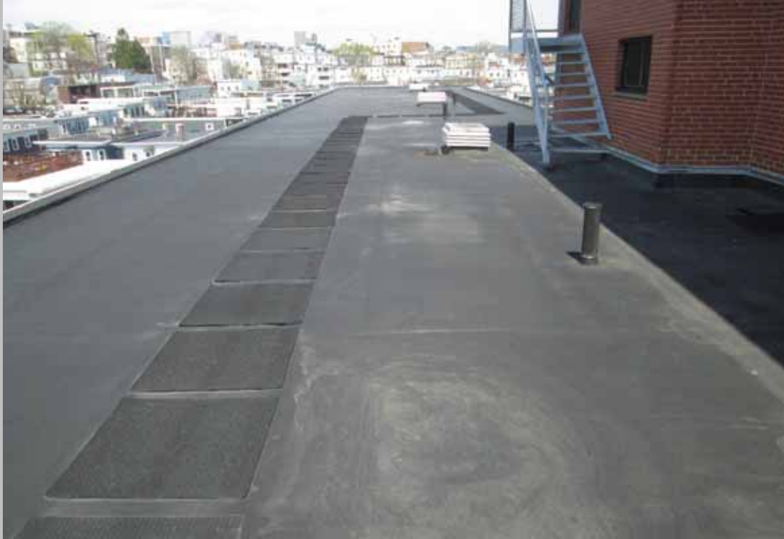
Roof surface – west side
