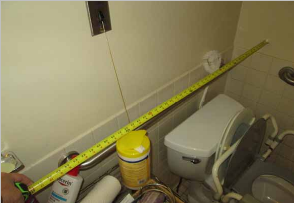
HC unit with compliant toilet rear grab bar
