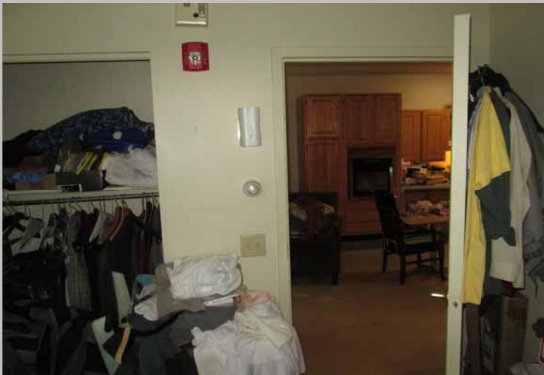
HC unit with compliant maneuvering space at interior door
