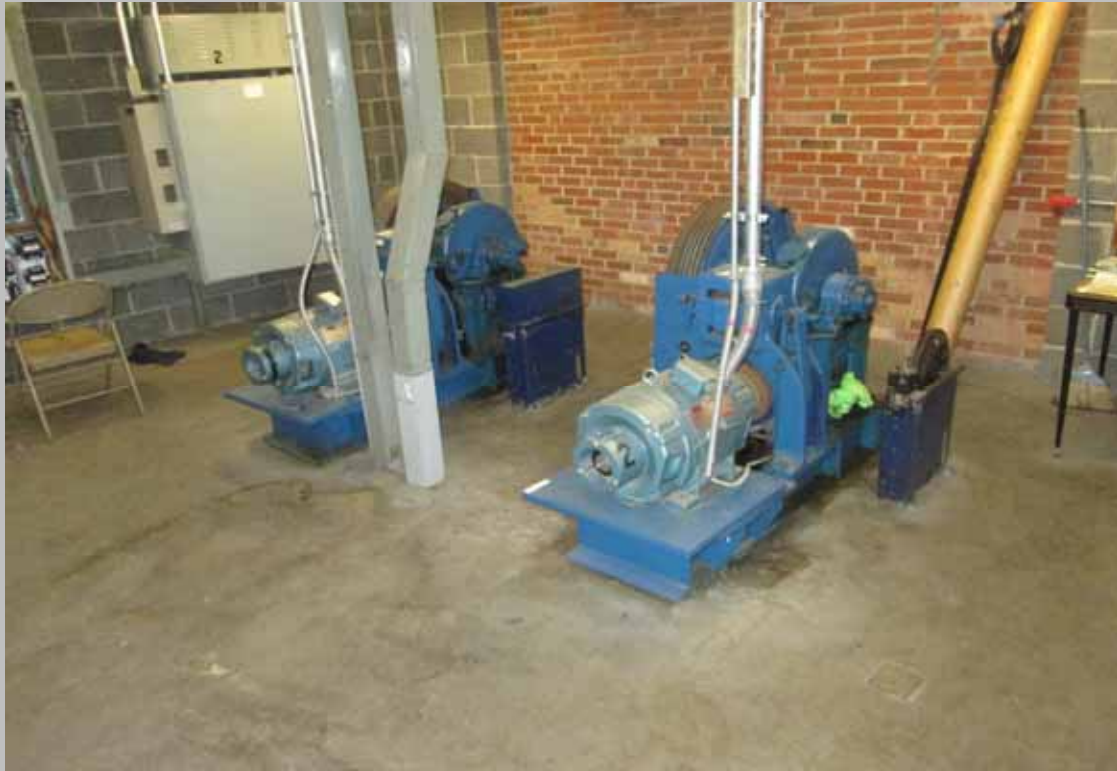
Elevator machinery
