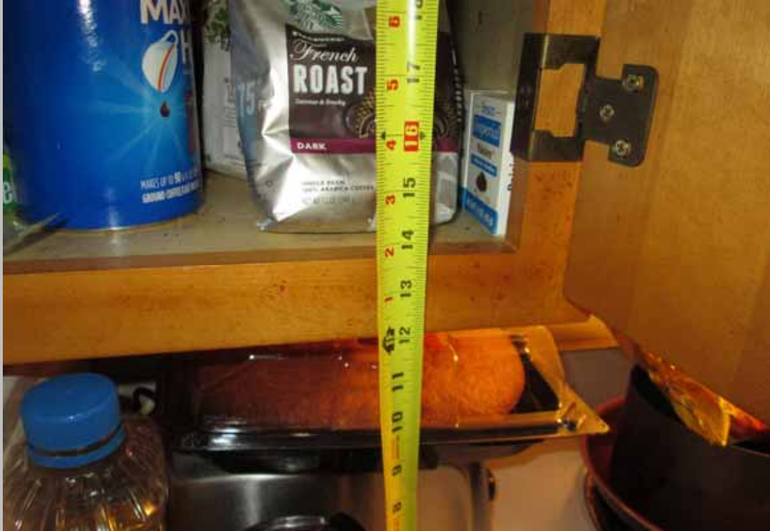
HC unit with compliant kitchen upper cabinetry at 48-inches above the finished flooring (AFF) [countertop height is 34-inches (AFF)]
