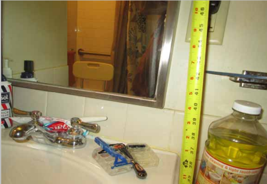
HC unit with compliant mirror height
