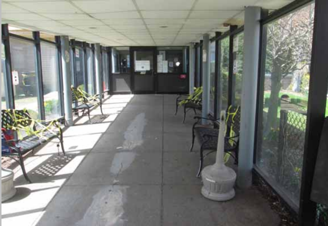
Walkway awning at main building entrance
