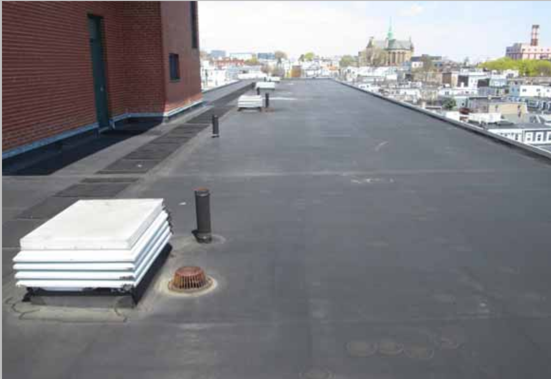
Roof surface – east side
