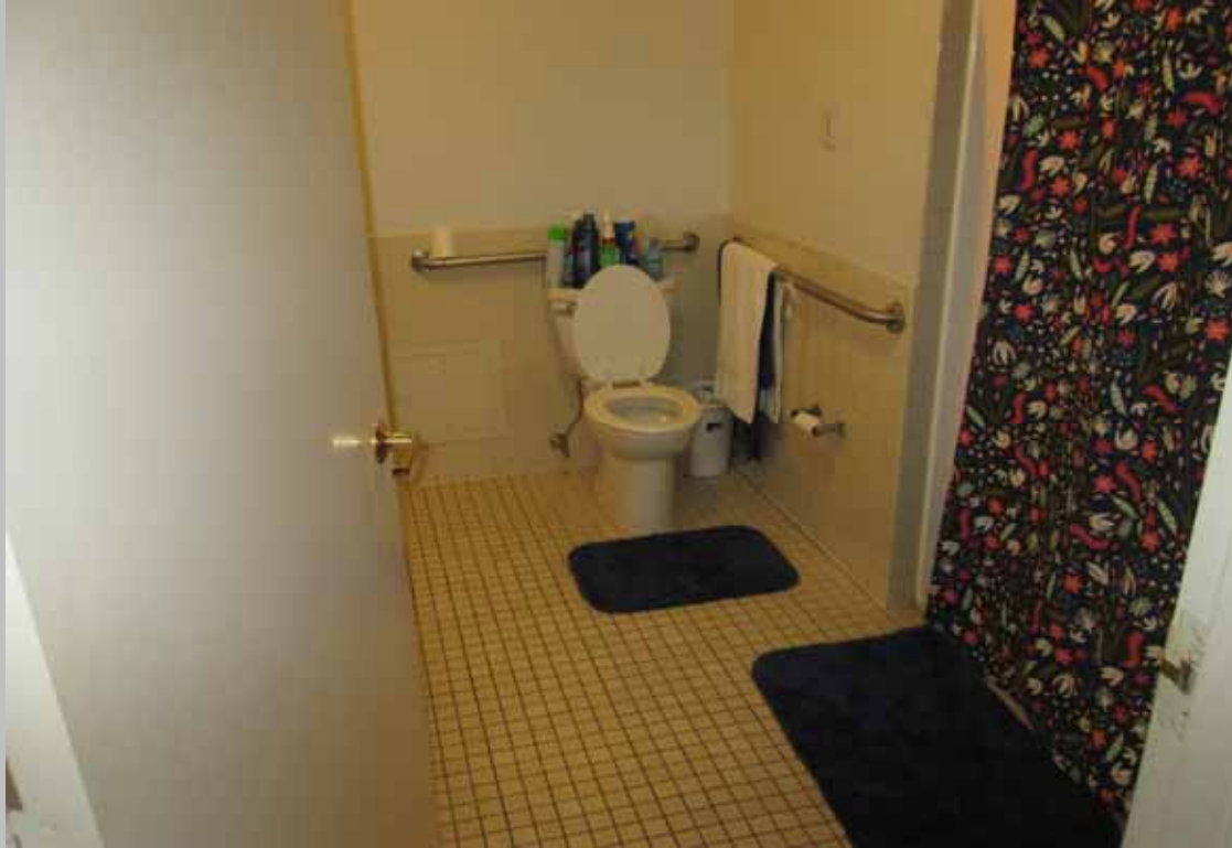
View of the bathroom within designated handicapped dwelling unit 404 featuring levered entry door hardware and compliant side and rear grab bars at the toilet
