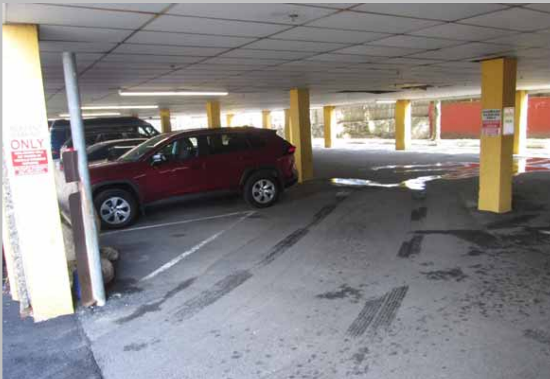
View of water damage to ceiling at covered parking area (Non-Critical Repair)
