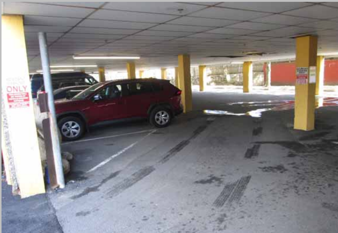
View of covered parking garage
