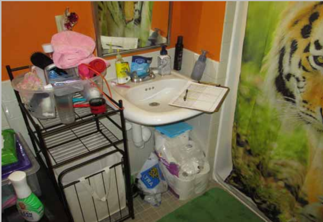
View of the bathroom sink within designated handicapped dwelling unit 514 featuring levered handle hardware and scald and abrasion protection
