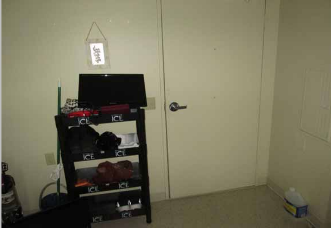
View of the entry area within designated handicapped unit 514 featuring levered handle hardware
