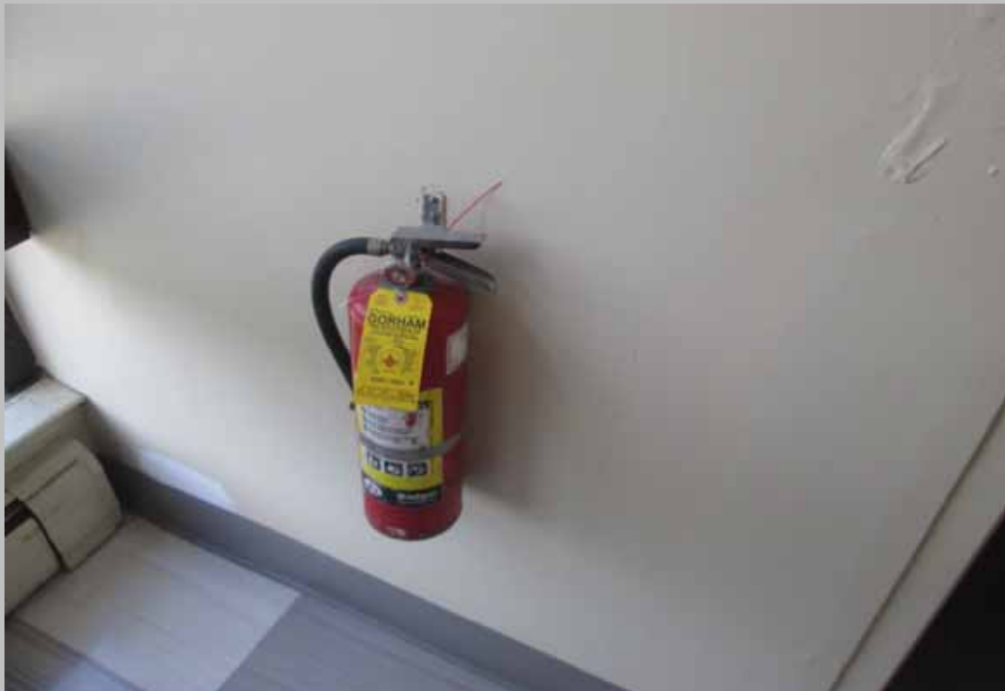
View of fire extinguisher
