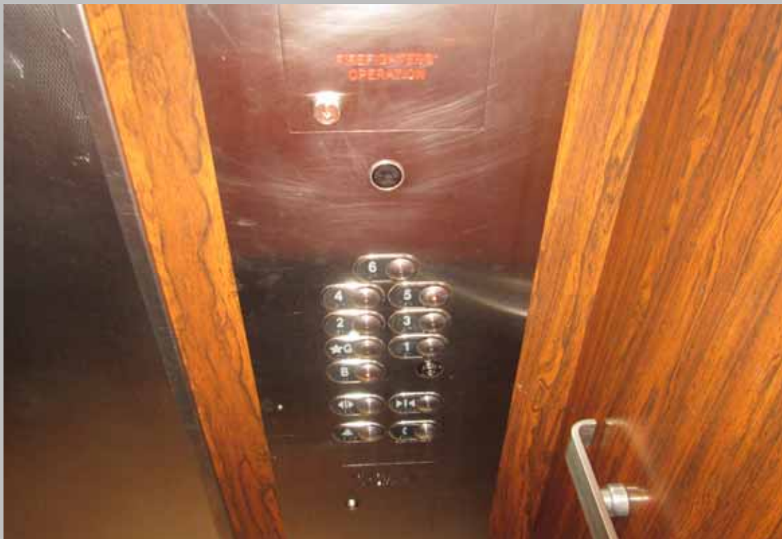
View of elevator cab
