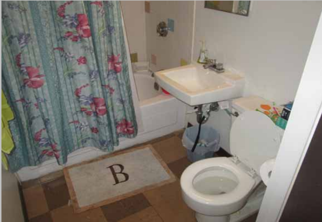
View of bathroom at Unit 510
