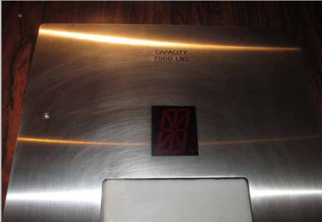
View of elevator cab
