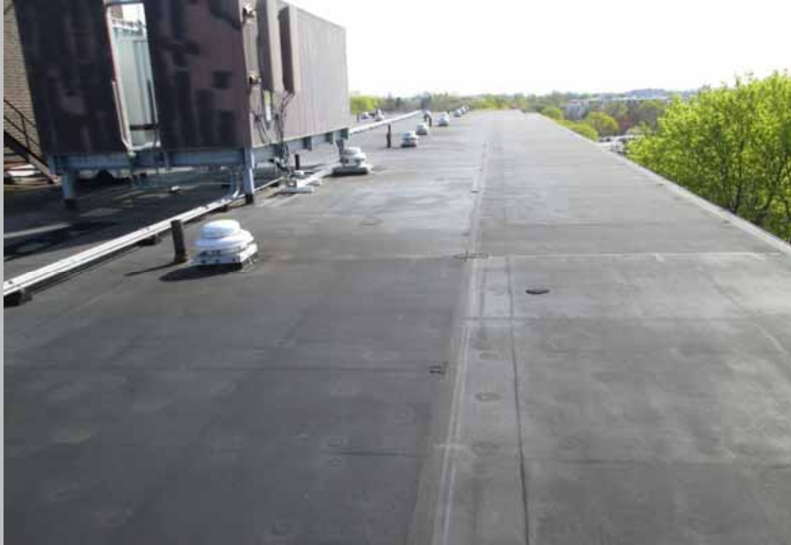
View of building roofing
