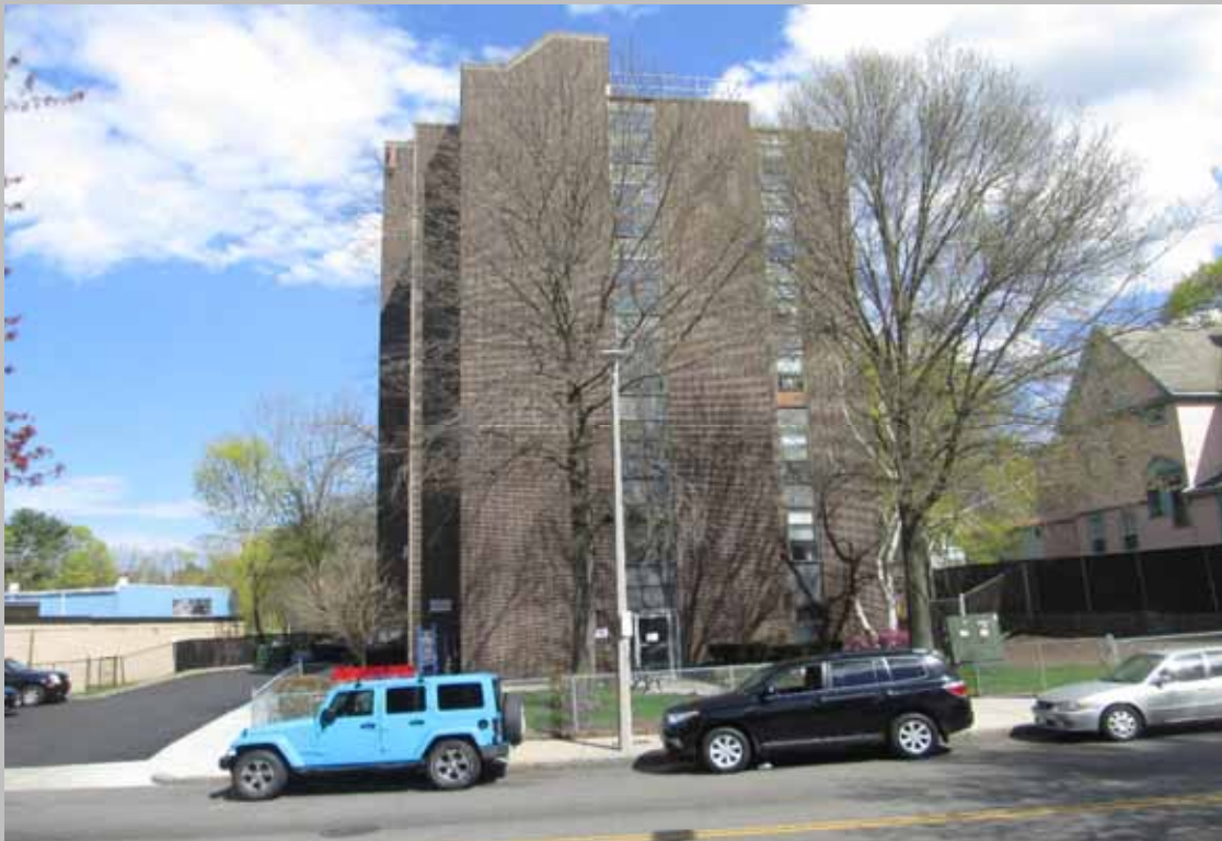
View of building exterior
