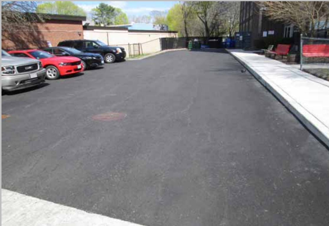
View of asphalt parking surface
