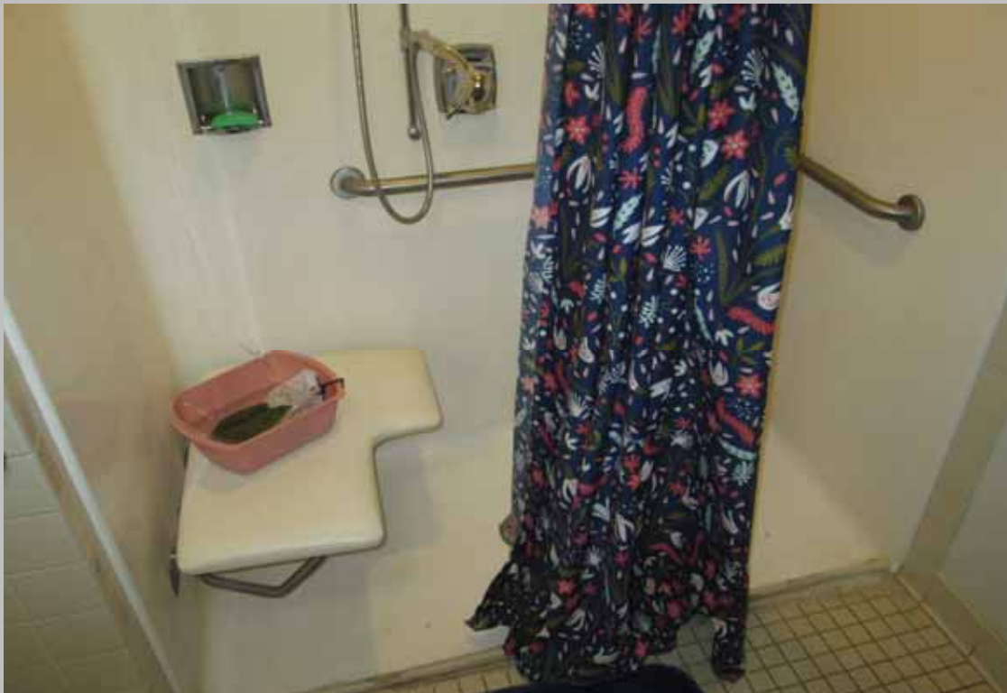
View of the shower within designated handicapped dwelling unit 404 featuring compliant grab bars and a 60-inch shower hose
