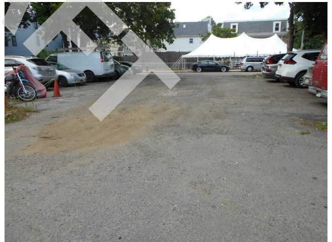
200. Asphalt parking lot by building 30
