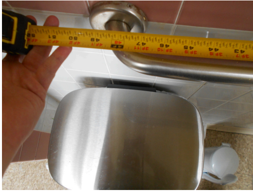
Community building, task force headquarters, restroom, rear grab bar 48"
