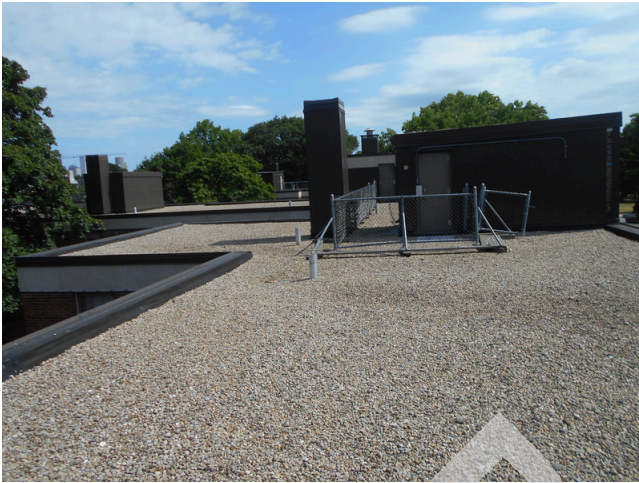
153. Building 32 EPDM Roof with gravel
