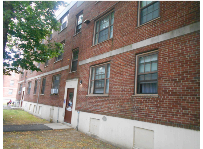
218. Building 32, front façade
