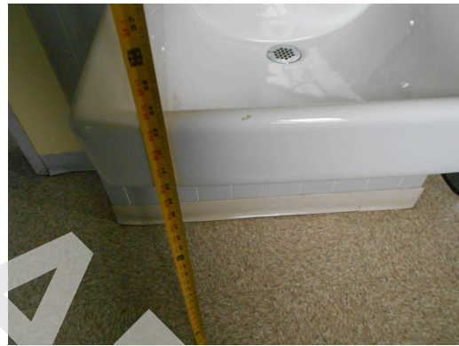
Community building, task force headquarters, restroom, sink height, 33"
