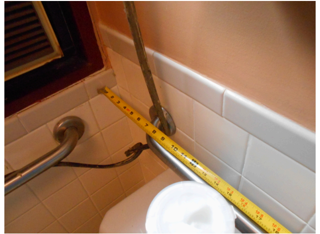
26. Leasing office public restroom rear grab bar
