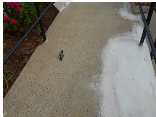
Leasing office handicap ramp slope 2, compliant
