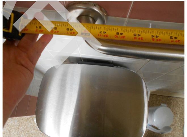
268. Community building, task force headquarters, restroom, rear grab bar 48"
