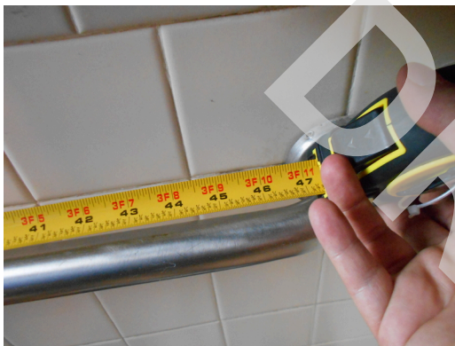
Leasing office public restroom rear grab bar, 47"
