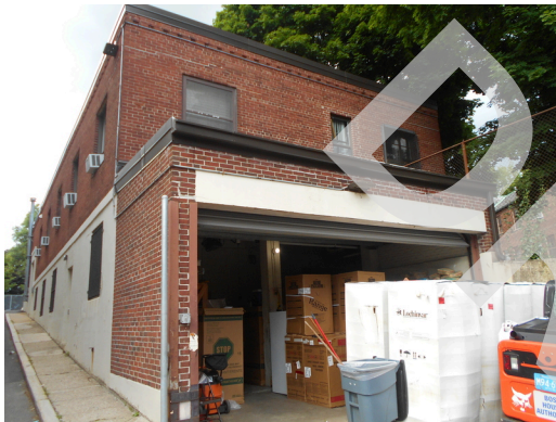
Leasing office rear façade and maintenance garage storage
