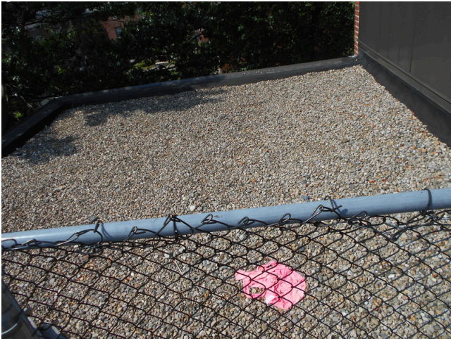
151. Building 32 EPDM Roof with gravel
