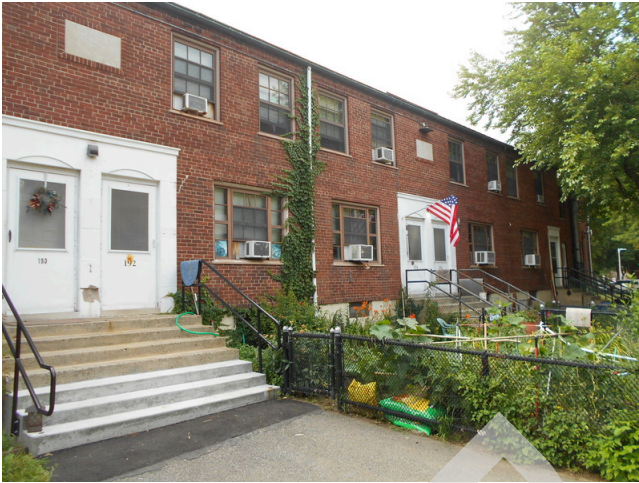
89. Building 11 front façade
