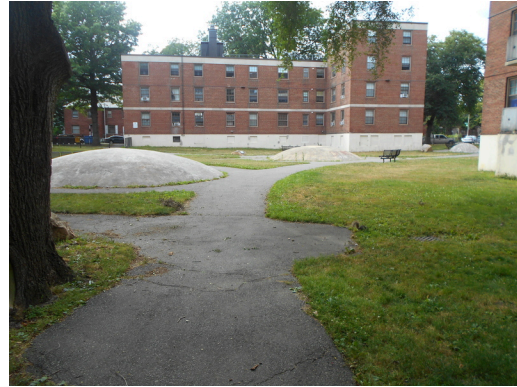
Rock park by building 23
