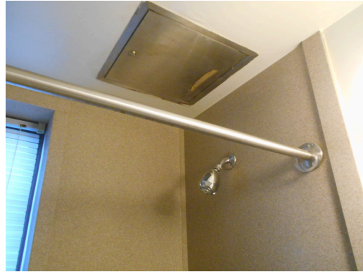
Building 1 unit 238, 1br/1ba - Bathroom shower, pipe access
