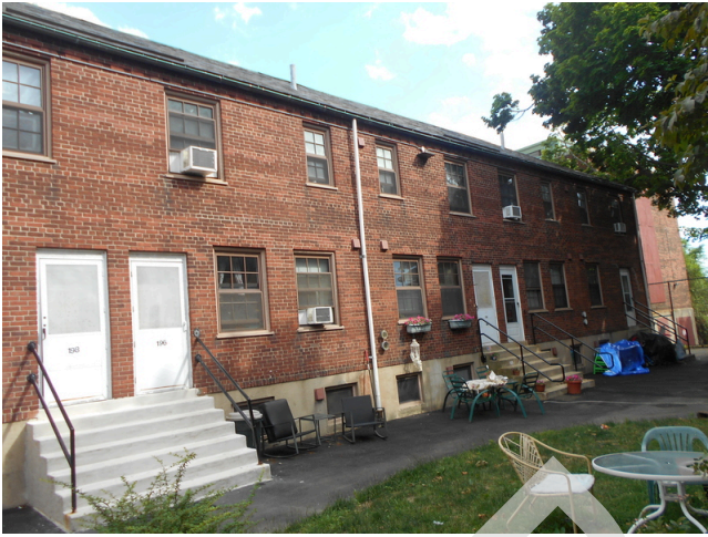
85. Building 11 rear façade
