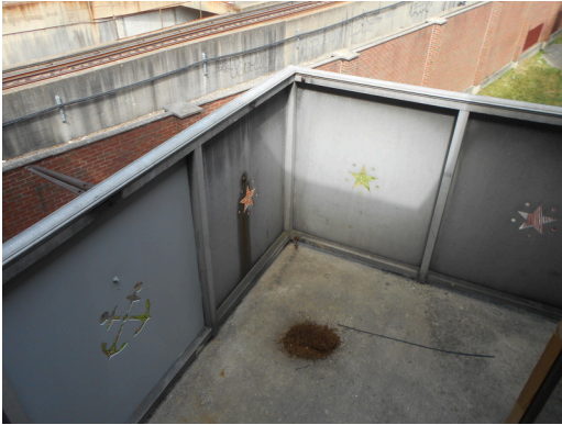
Building 1 unit 266, 2br/1ba, vacant - Concrete balcony
