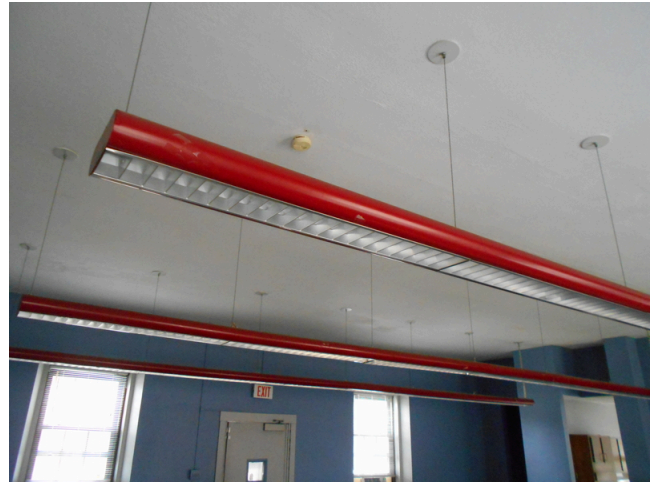
258. Community building, task force headquarters, ceiling
