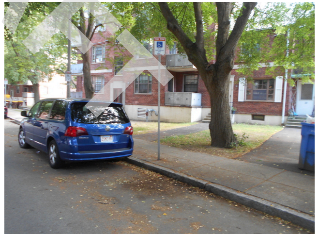
44. Building 3 handicap street parking, no curb cut or access aisle (Critical Repair)
