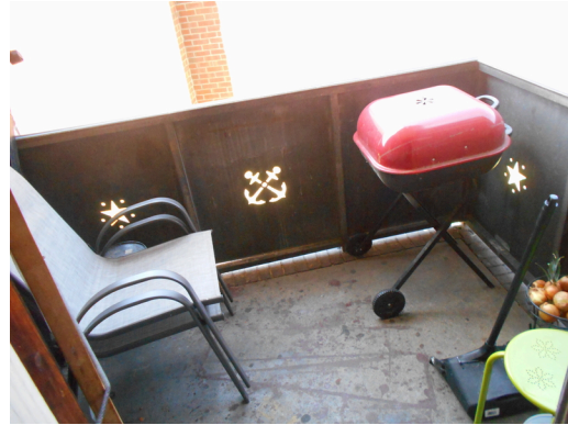
Building 2 unit 222, 2br/1ba - Balcony
