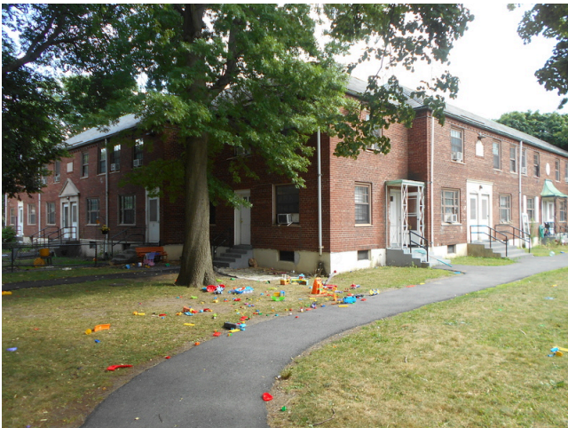
119. Building 3 front façade
