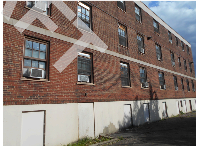
136. Building 2 front façade
