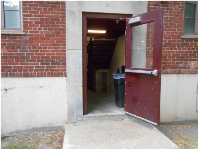
49. Building 3 stairwell entrance
