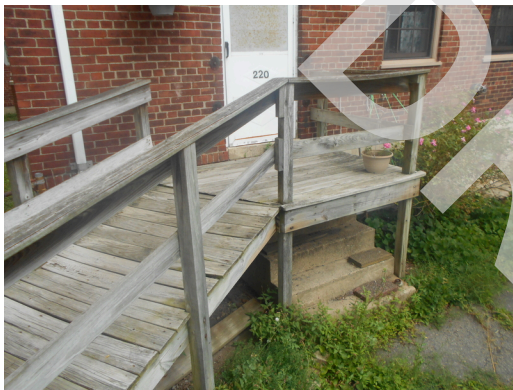
Wood ramp leading to 220 O'Callaghan Way, not a designated handicap unit
