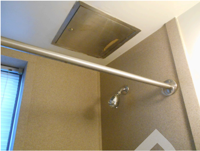
9. Building 1 unit 238, 1br/1ba - Bathroom shower, pipe access
