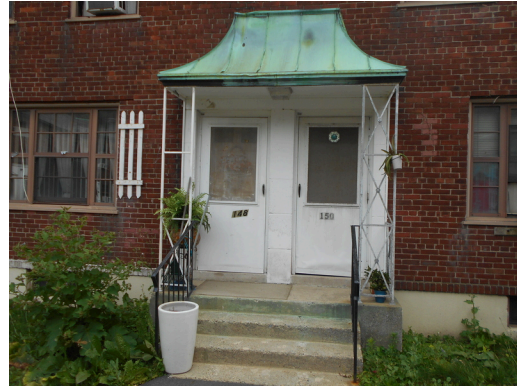
Building 5 front façade
