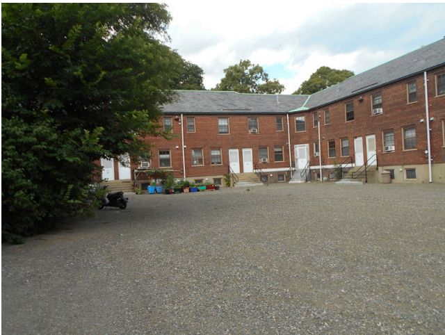
111. Building 4 rear façade
