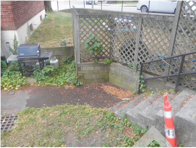
241. Wood retaining wall by buildings
