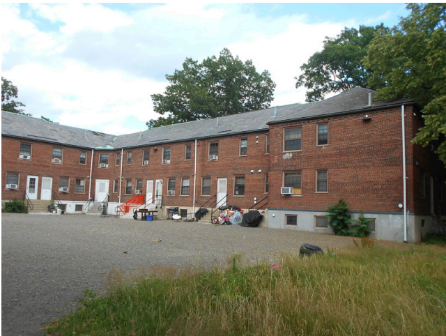
123. Building 3 rear façade
