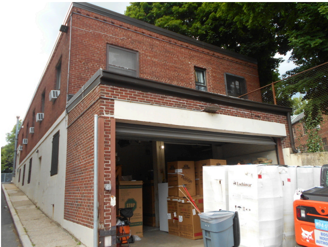
79. Leasing office rear façade and maintenance garage storage
