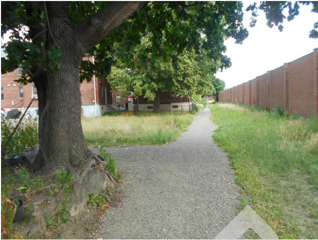
121. Gravel path to the rear of building 3
