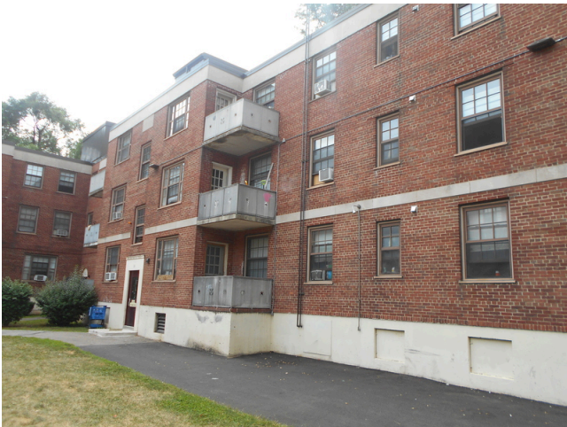
219. Building 32, front façade
