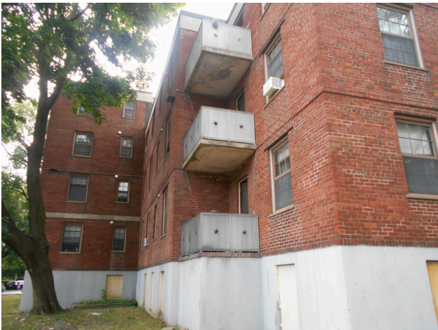
211. Building 32 rear façade
