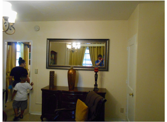
102. Building 5 unit 186, 64 O'Callaghan Way, 3br/ 1ba Townhouse - Rear door, damaged (Non-Critical Repair)
