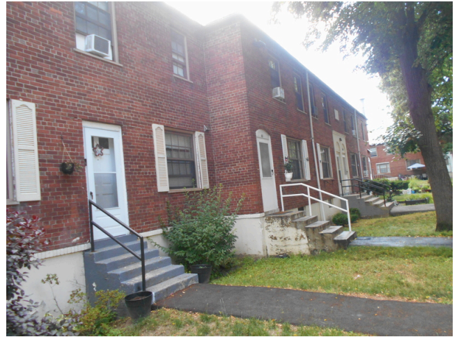
130. Building 4 front façade
