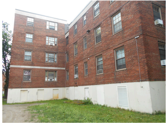
210. Building 32 rear façade
