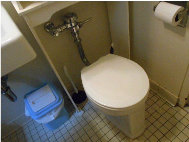
7. Building 1 unit 238, 1br/1ba - Bathroom toilet
