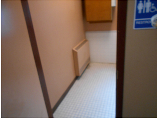
Leasing office public restroom entrance
