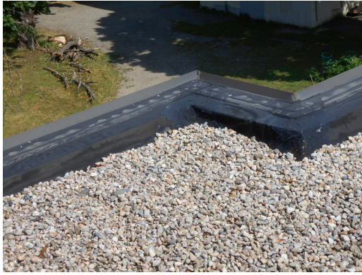
Building 32 EPDM Roof with gravel
