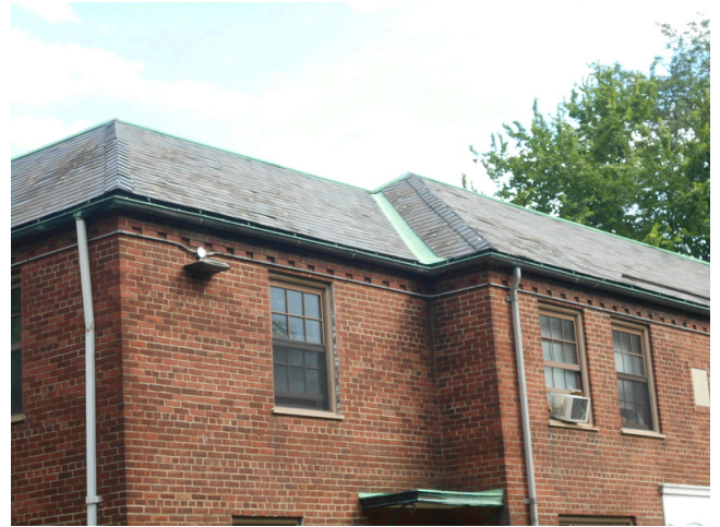
94. Building 6 front façade, slate tile roof (Non-Critical Repair)
