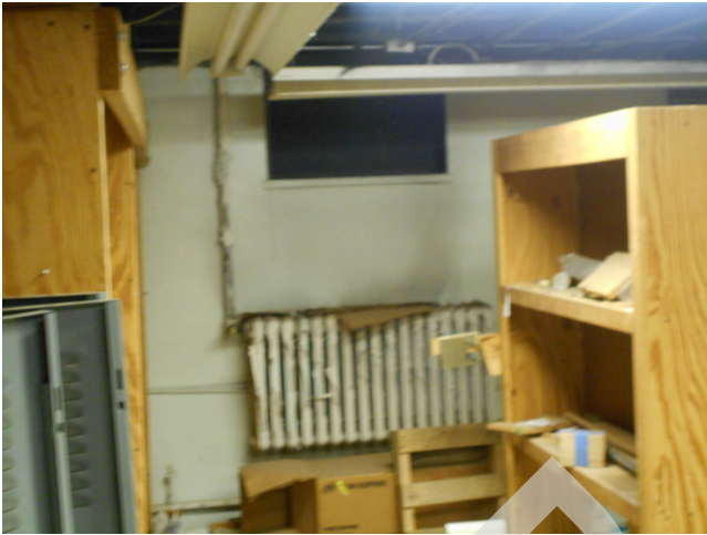
185. Building 19, 2 Sterling square basement, maintenance woodshop
