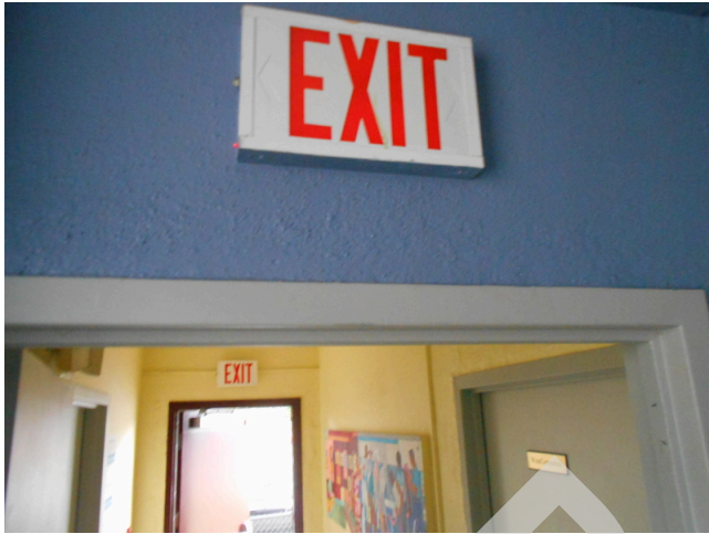
273. Community building, task force headquarters, exit sign
