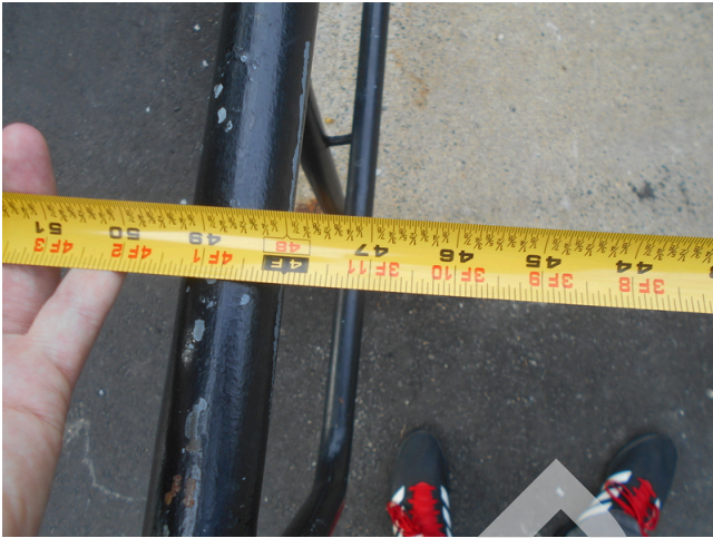
5. Leasing office handicap ramp rail width, 48"
