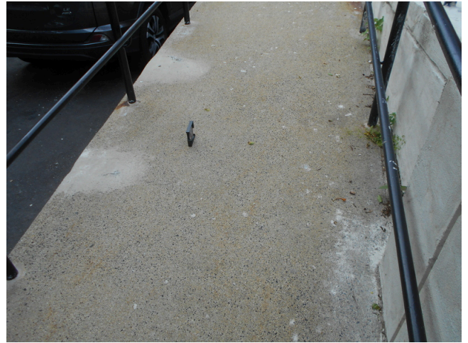
6. Leasing office handicap ramp slope
