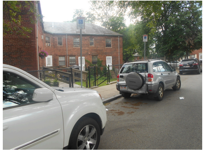
250. Handicap designated street parking by building 11, 16 Kemp Street, unit 116, no access aisle or curb cut (Critical Repair)
