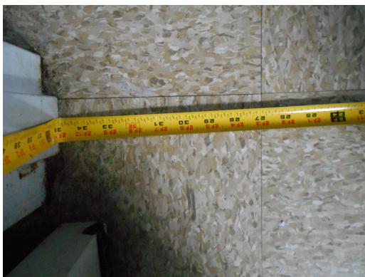
Community building, task force headquarters, restroom, entrance door width, 35"
