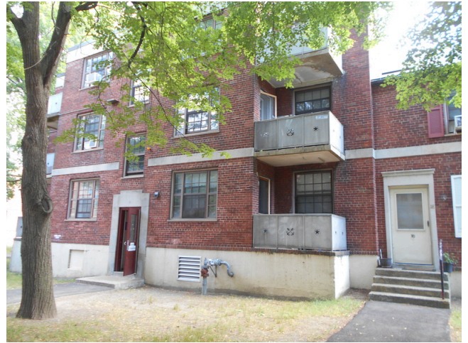
46. Building 3 front façade
