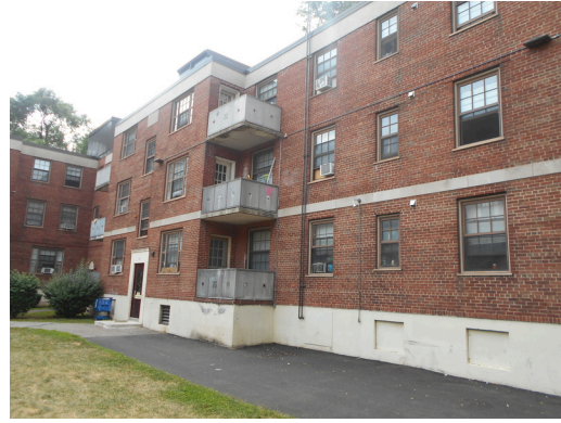
Building 32, front façade
