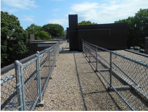
Building 32 EPDM Roof with gravel
