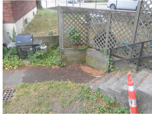
Wood retaining wall by buildings
