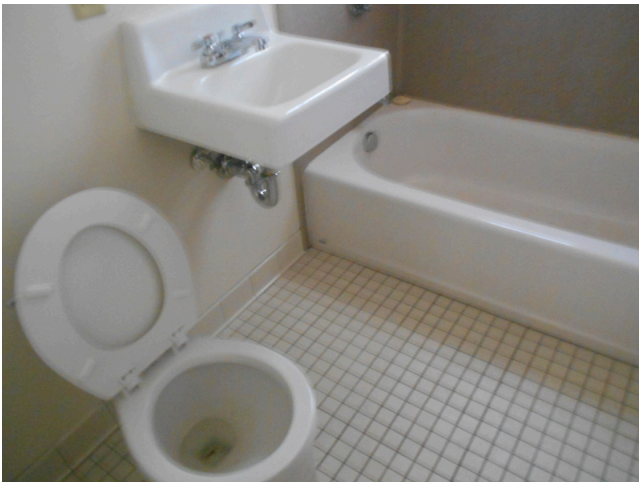
39. Building 1 unit 266, 2br/1ba, vacant - Bathroom
