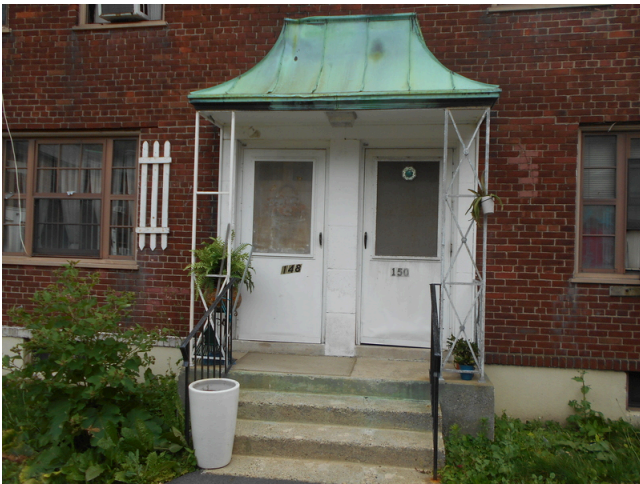
103. Building 5 front façade
