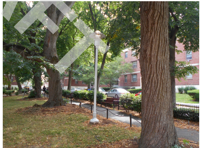
244. Exterior pole mounted lighting
