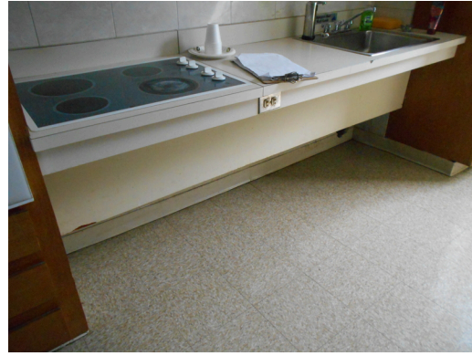
Community building, task force headquarters, kitchen roll-under sink
