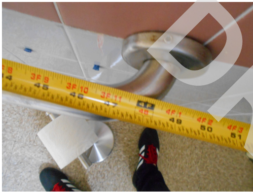
Community building, task force headquarters, restroom, side grab bar, 48"
