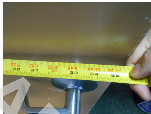
Leasing office, typical door width, 35"
