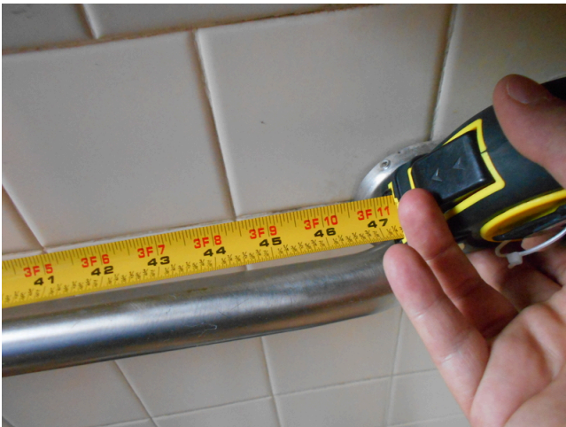
27. Leasing office public restroom rear grab bar, 47"
