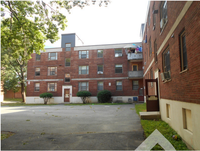
137. Building 2 front façade
