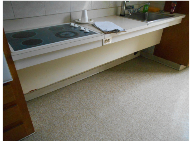
262. Community building, task force headquarters, kitchen roll-under sink
