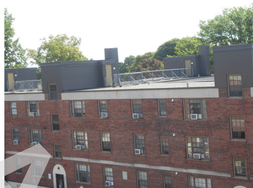
Building 31 EPDM Roof with gravel
