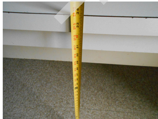
Community building, task force headquarters, kitchen countertop height, 34"
