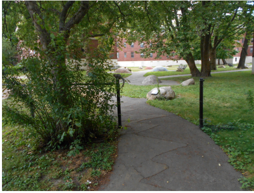
Asphalt paved rock park path
