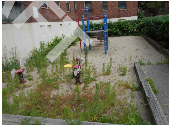
228. Playground by building 22, overgrown (Non-Critical Repair)
