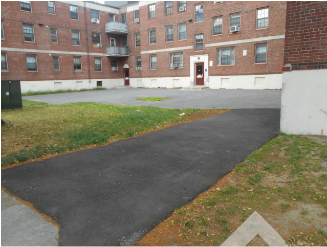
213. Building 32, asphalt paved courtyard
