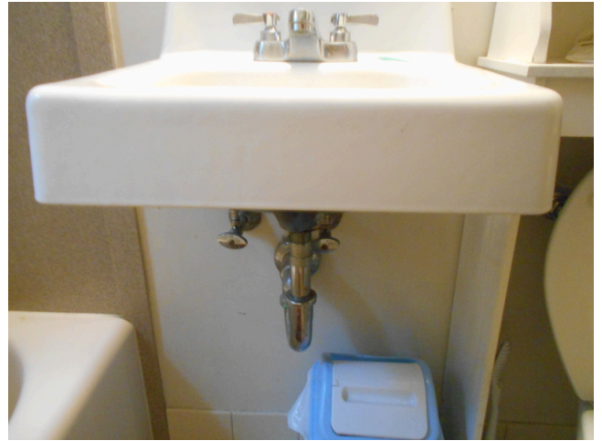
6. Building 1 unit 238, 1br/1ba - Bathroom sink
