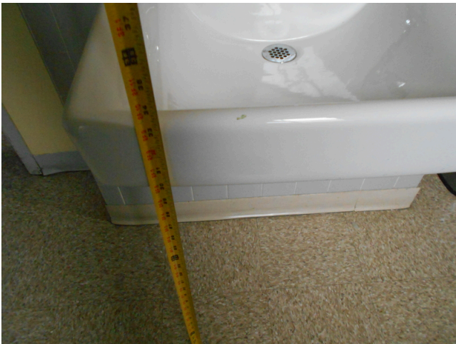
271. Community building, task force headquarters, restroom, sink height, 33"
