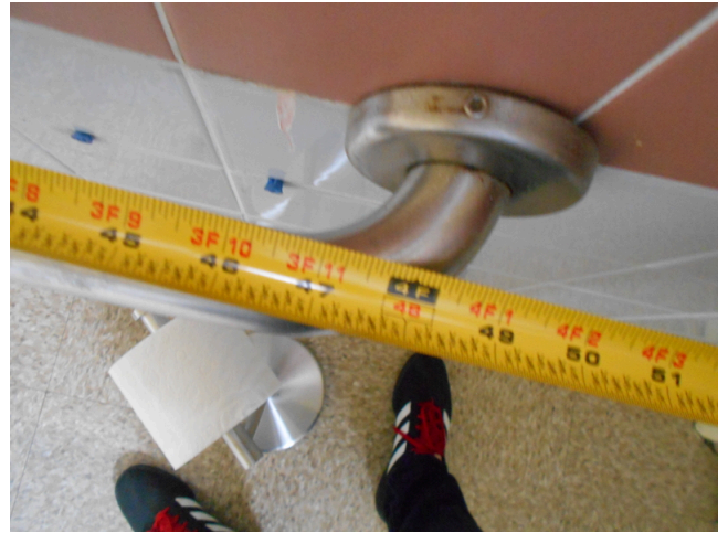
270. Community building, task force headquarters, restroom, side grab bar, 48"
