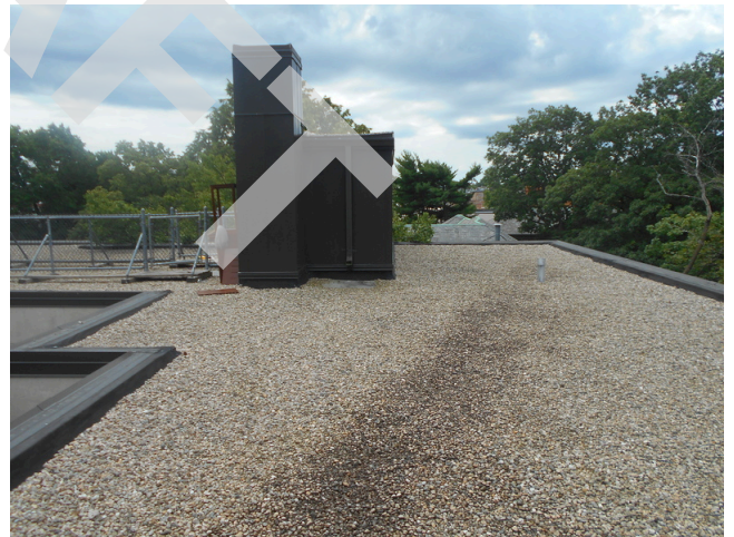
180. Building 17 EPDM roof with gravel roof
