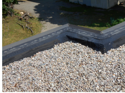
Building 32 EPDM Roof with gravel
