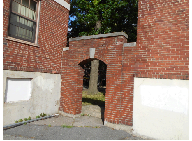
134. Building 2 side façade archway
