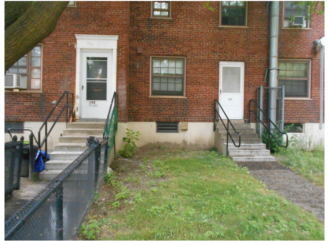
90. Building 11 front façade
