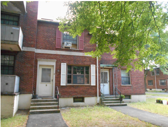
47. Building 3 front façade
