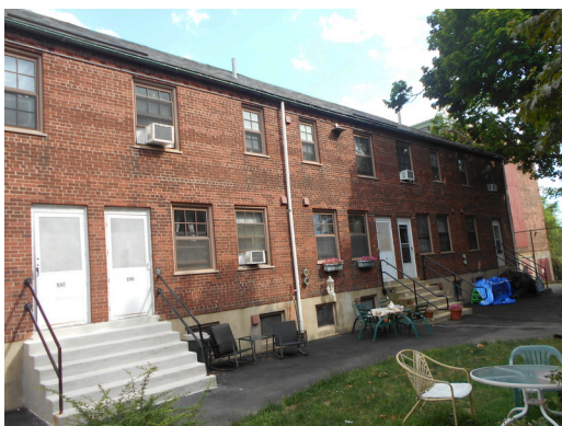
Building 11 rear façade
