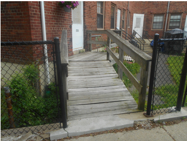
239. Wood ramp leading to 220 O'Callaghan Way, not a designated handicap unit
