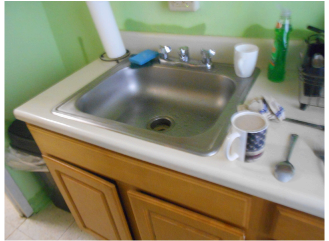
14. Building 1 unit 238, 1br/1ba - Kitchen sink
