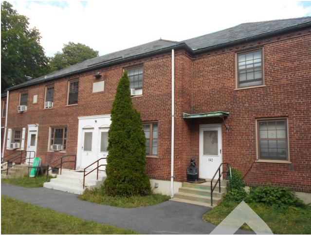
113. Building 4 rear façade
