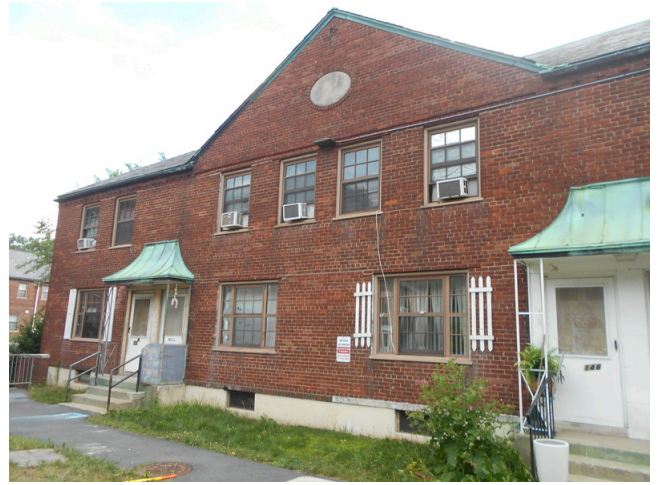
102. Building 5 front façade
