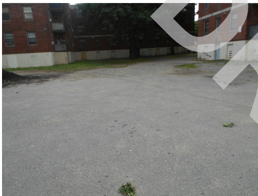
Asphalt parking lot by building 30
