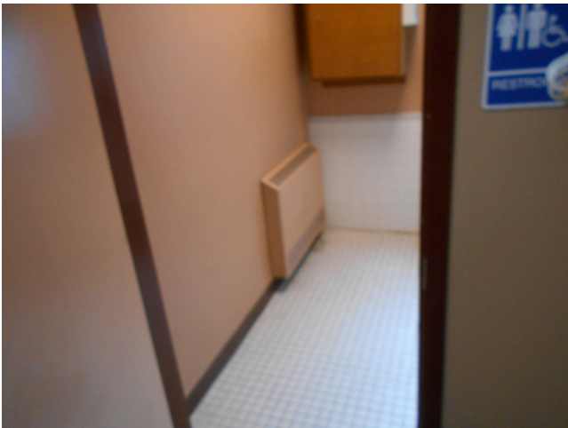
19. Leasing office public restroom entrance
