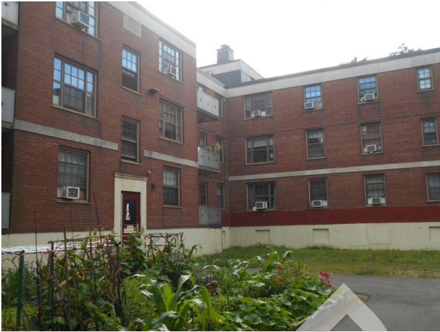
145. Building 12 front façade
