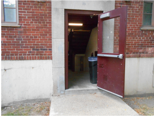
Building 3 stairwell entrance
