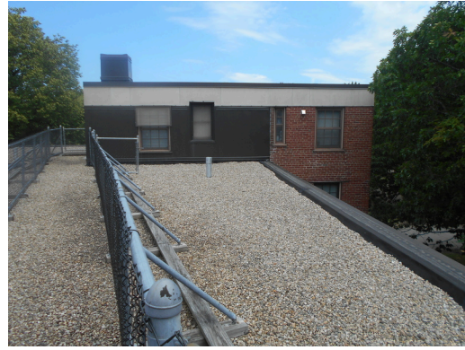
Building 17 EPDM roof with gravel roof
