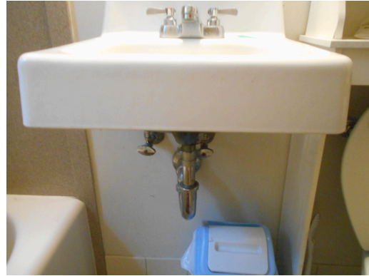
Building 1 unit 238, 1br/1ba - Bathroom sink
