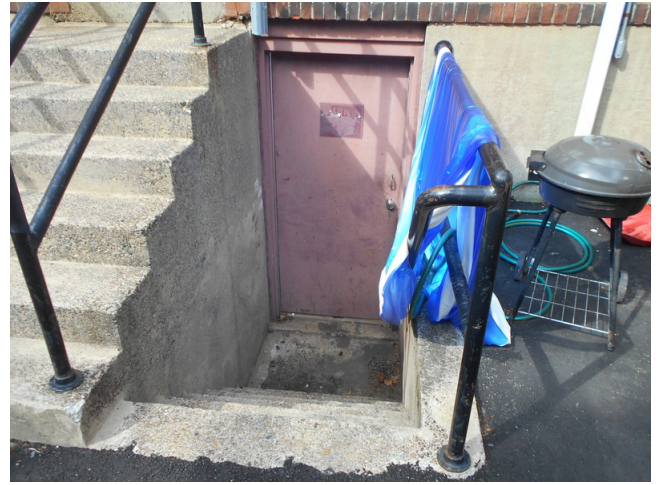
86. Building 11 rear façade, entrance to basement
