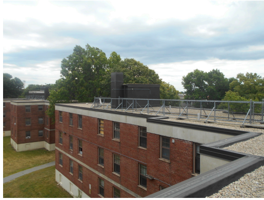
Building 17 EPDM roof with gravel roof
