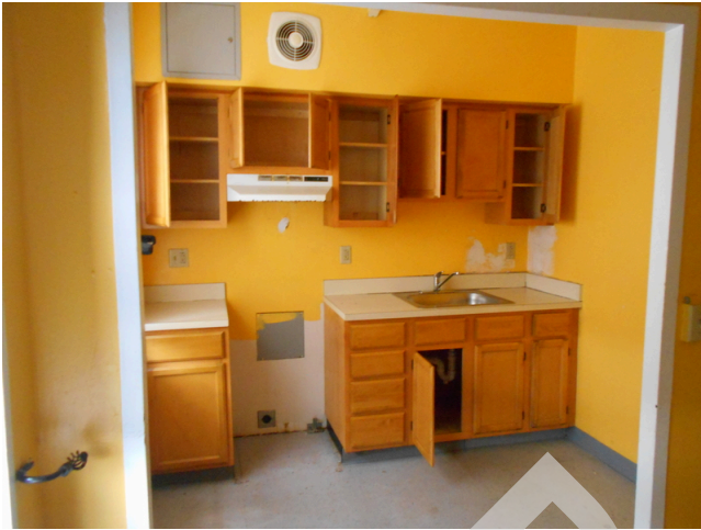
97. Building 4 unit 200, 36 O'Callaghan Way, 3br/ 1ba Townhouse - Kitchen
