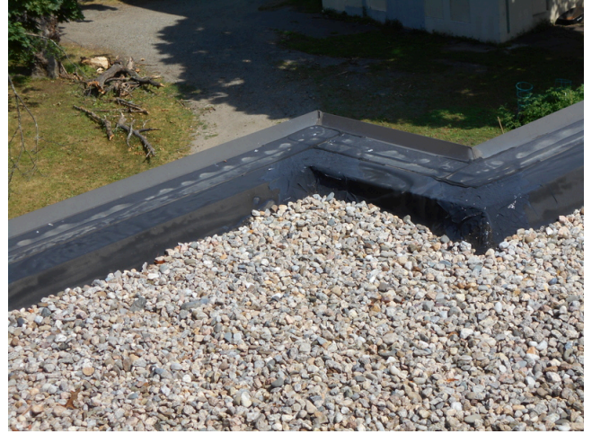
150. Building 32 EPDM Roof with gravel
