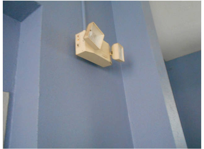
274. Community building, task force headquarters, emergency light
