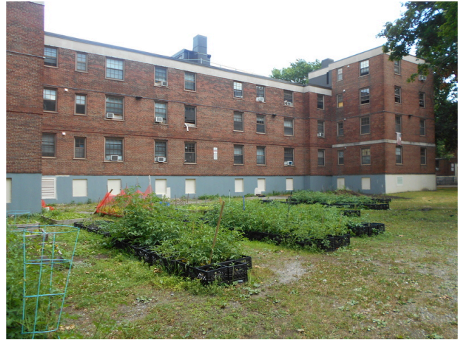
190. Building 31 rear façade
