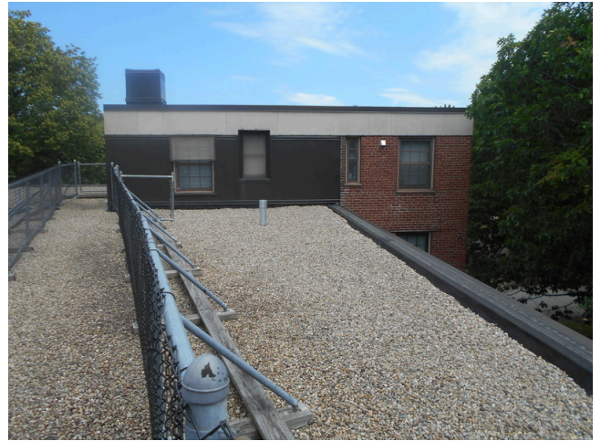
182. Building 17 EPDM roof with gravel roof
