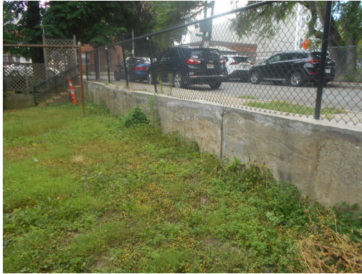
Concrete retaining wall by building 27
