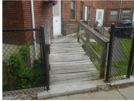
Wood ramp leading to 220 O'Callaghan Way, not a designated handicap unit
