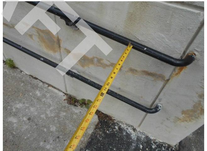
4. Leasing office handicap ramp rail width
