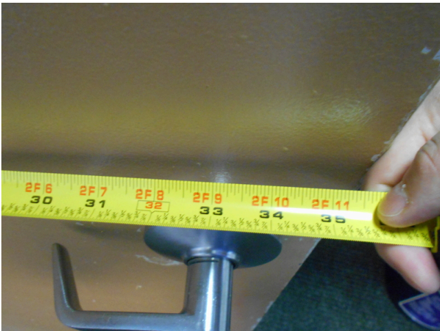
15. Leasing office, typical door width, 35"
