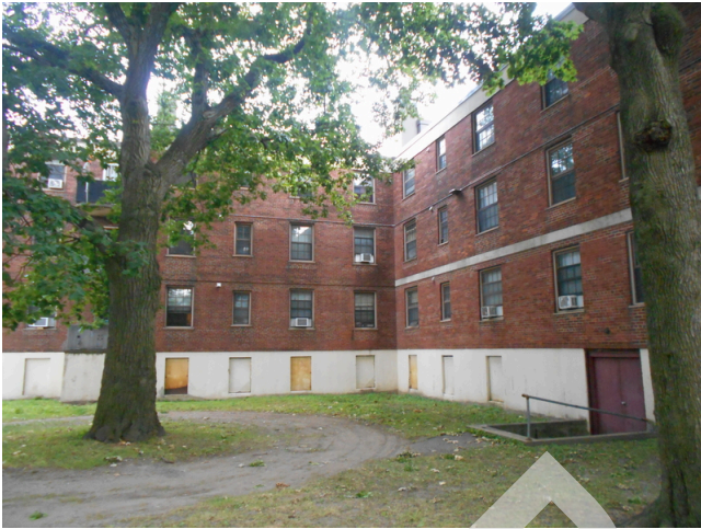
209. Building 32 rear façade
