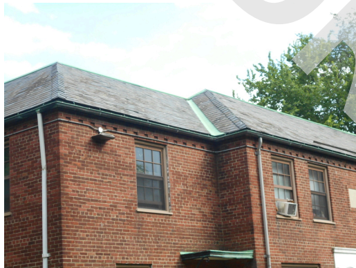
Building 6 front façade, slate tile roof (Non-Critical Repair)
