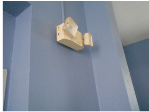
Community building, task force headquarters, emergency light
