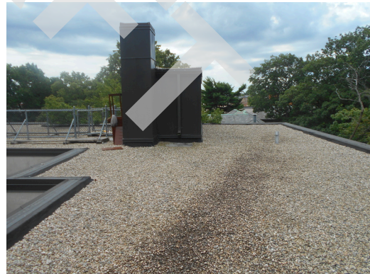
Building 17 EPDM roof with gravel roof
