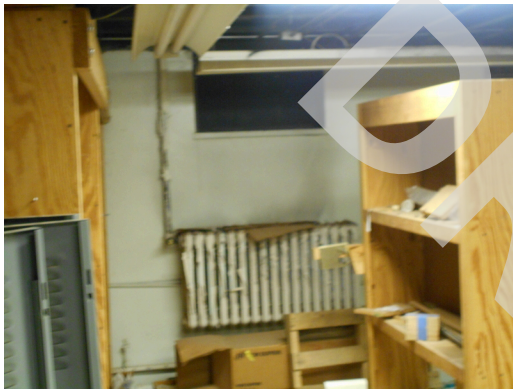
Building 19, 2 Sterling square basement, maintenance woodshop
