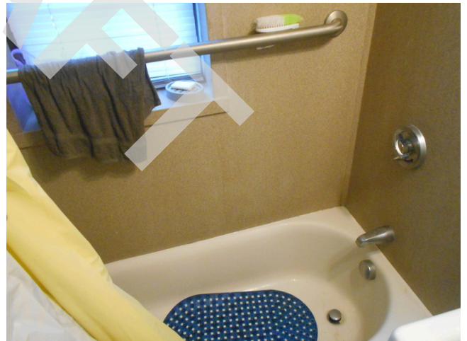
8. Building 1 unit 238, 1br/1ba - Bathroom shower
