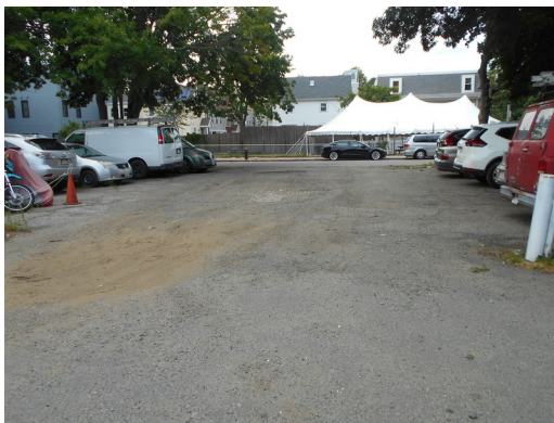
Asphalt parking lot by building 30
