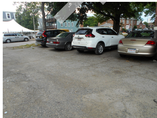
Asphalt parking lot by building 30
