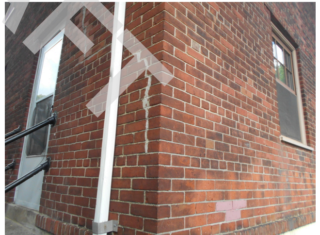
88. Building 11 side façade, repaired facade
