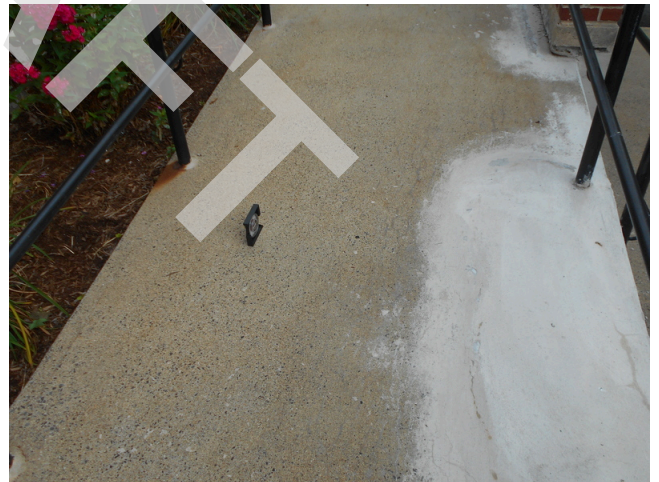
8. Leasing office handicap ramp slope 2, compliant
