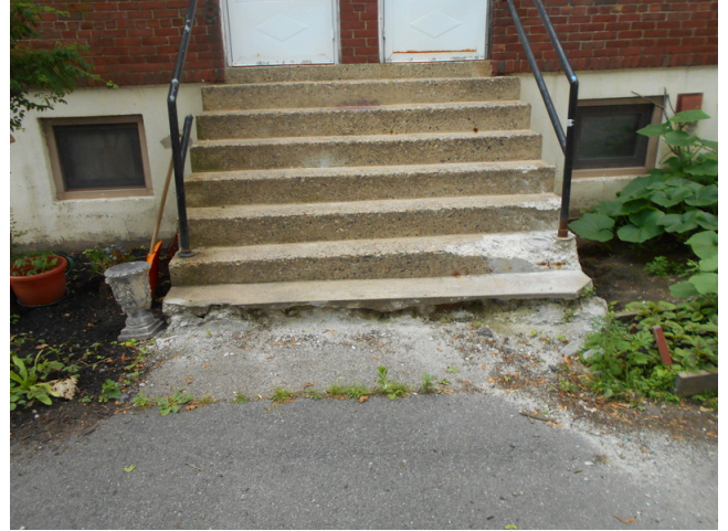
206. Concrete steps for the rear of building 34, 49 Logan Way
