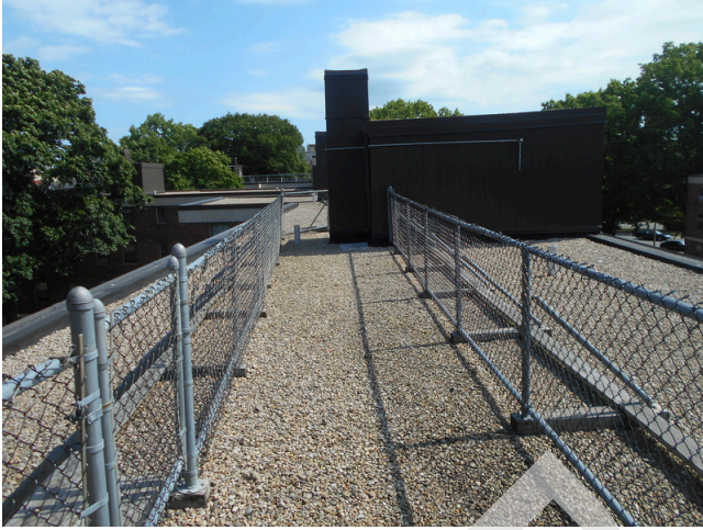
149. Building 32 EPDM Roof with gravel
