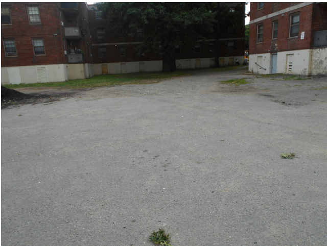
199. Asphalt parking lot by building 30
