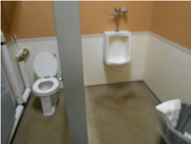
31. Leasing office basement staff restrooms
