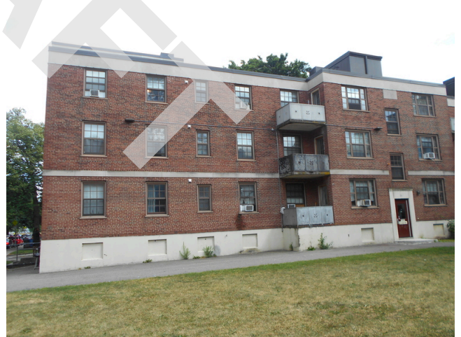
220. Building 32, front façade
