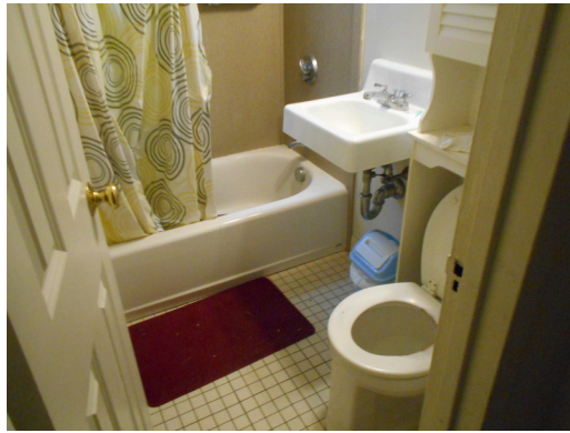
Building 1 unit 238, 1br/1ba - Bathroom
