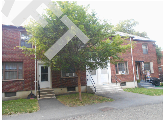
124. Building 3 front façade
