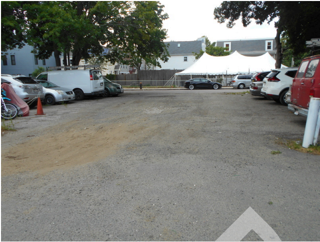
201. Asphalt parking lot by building 30
