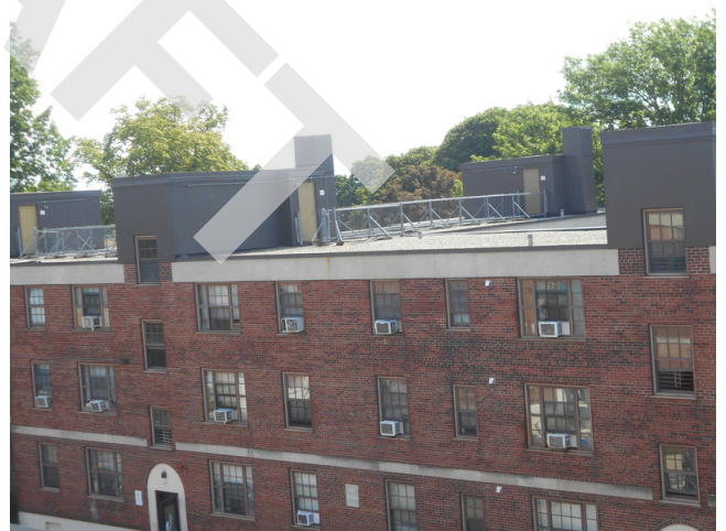
152. Building 31 EPDM Roof with gravel
