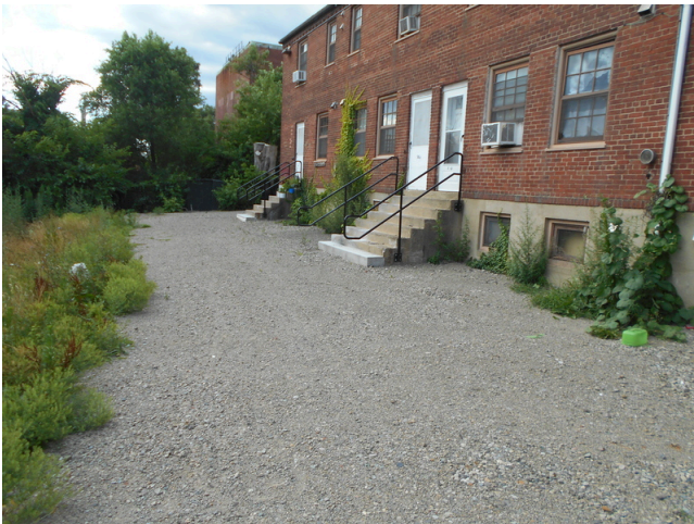
107. Building 5 rear façade
