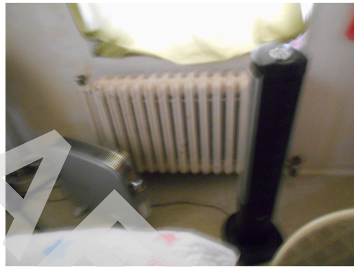
Building 1 unit 238, 1br/1ba - Bedroom radiator
