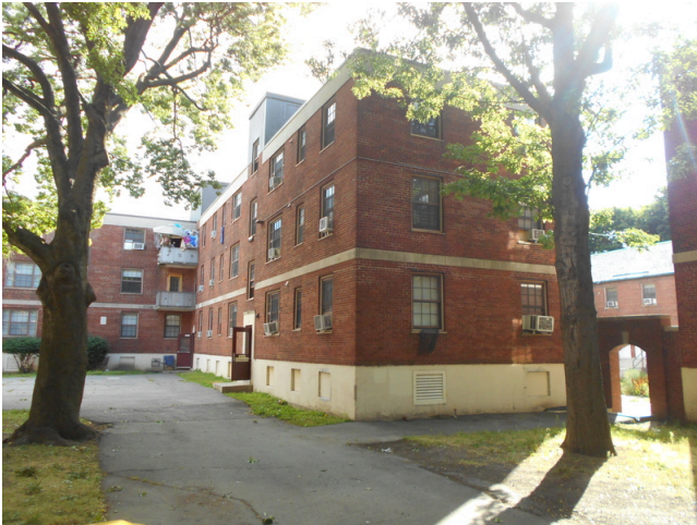
135. Building 2 front façade
