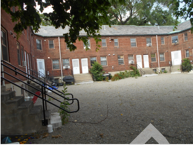
97. Building 6 rear façade
