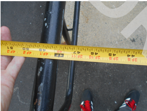
Leasing office handicap ramp rail width, 48"
