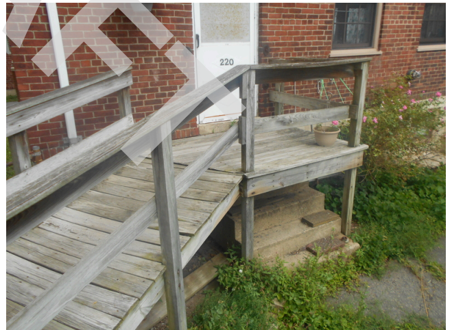
240. Wood ramp leading to 220 O'Callaghan Way, not a designated handicap unit
