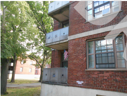
Building 3 concrete balconies
