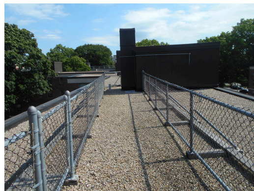
Building 32 EPDM Roof with gravel
