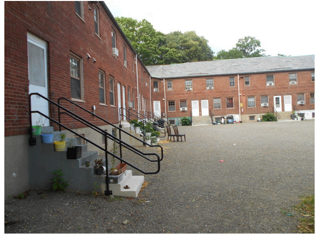
122. Building 3 rear façade
