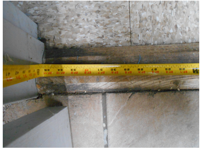
278. Community building, task force headquarters, restroom 2 entrance door width, 36"
