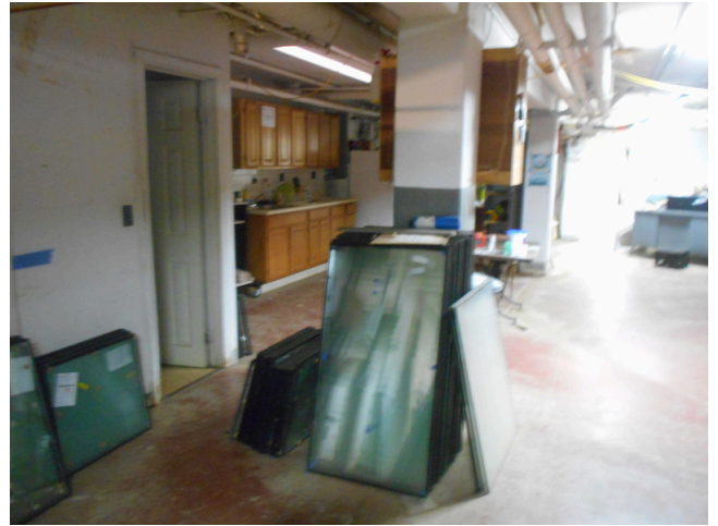
166. Building 30 basement, maintenance storage
