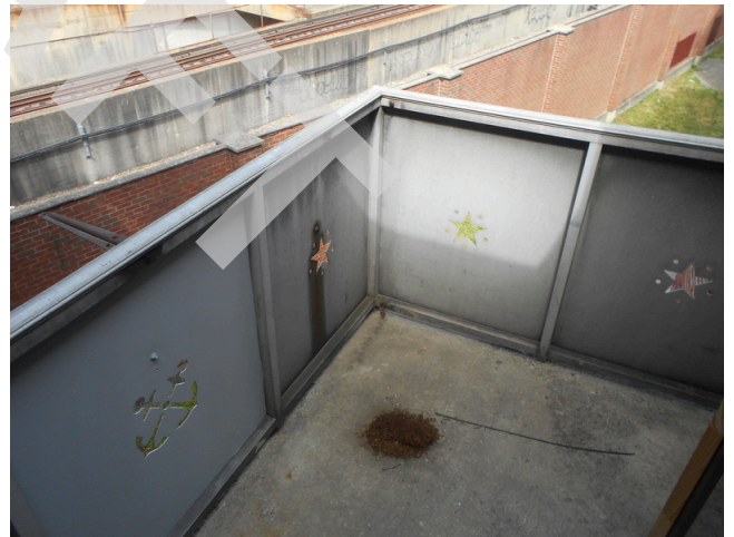
36. Building 1 unit 266, 2br/1ba, vacant - Concrete balcony
