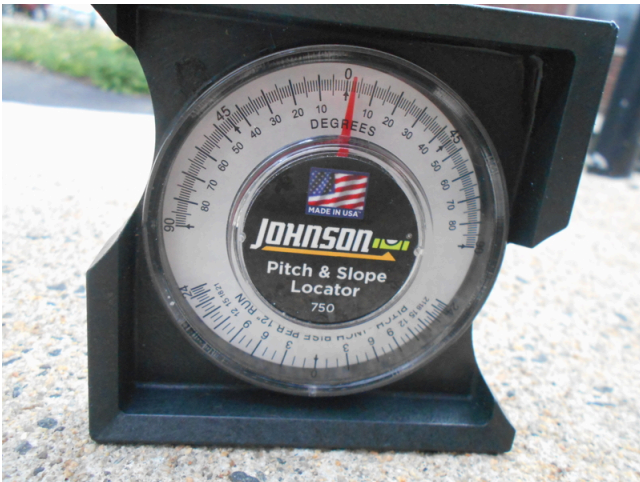
7. Leasing office handicap ramp slope, compliant
