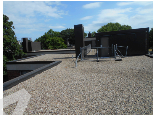
Building 32 EPDM Roof with gravel
