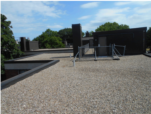
Building 32 EPDM Roof with gravel
