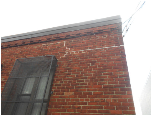
Leasing office front façade, repaired cracking
