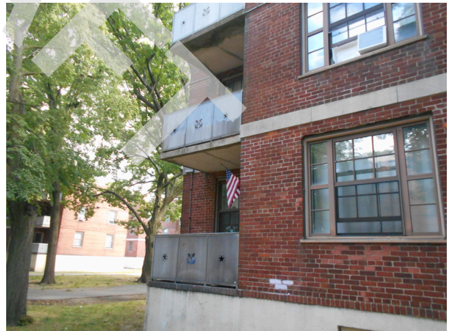
48. Building 3 concrete balconies
