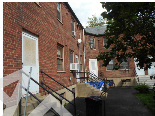
Building 11 rear façade
