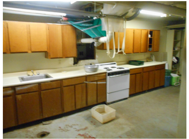
162. Building 30 staff kitchen in basement, not in use
