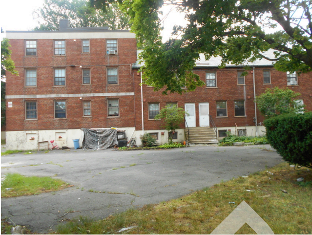
205. Building 34 rear façade
