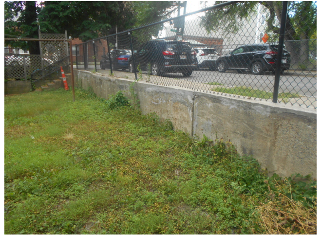
238. Concrete retaining wall by building 27
