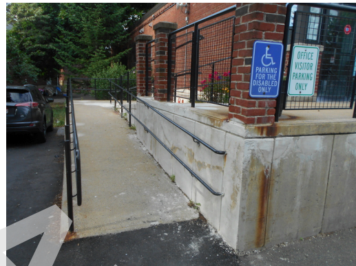
Leasing office handicap ramp
