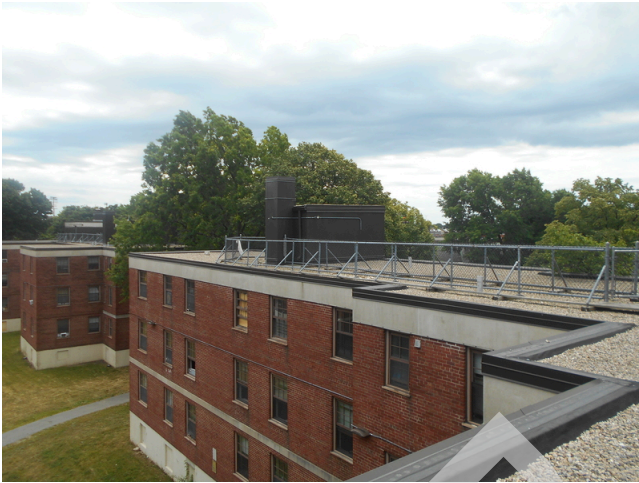
181. Building 17 EPDM roof with gravel roof
