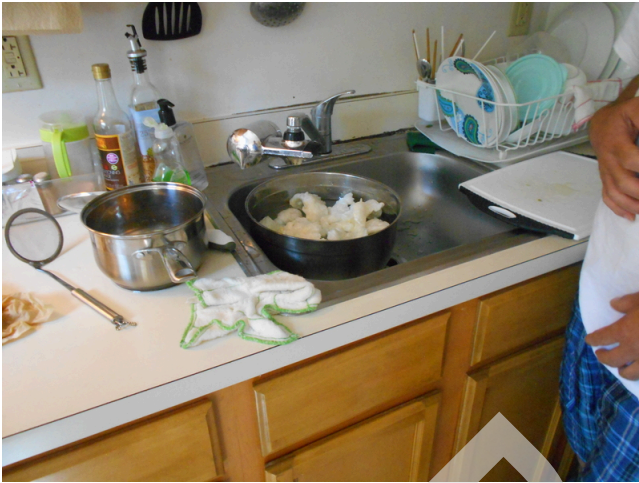
61. Building 3 unit 204, 28 O'Callaghan Way, 3br/ 1ba Townhouse - Kitchen sink
