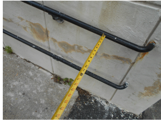
Leasing office handicap ramp rail width
