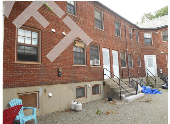
96. Building 6 rear façade
