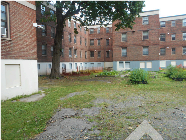
189. Building 31 rear façade
