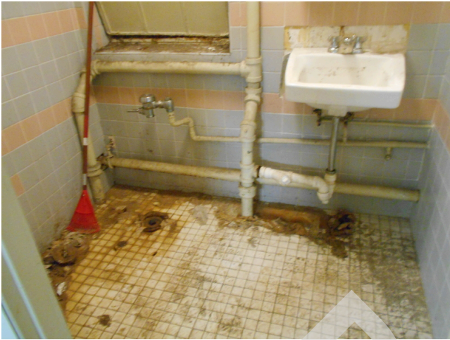
165. Building 30 basement sink
