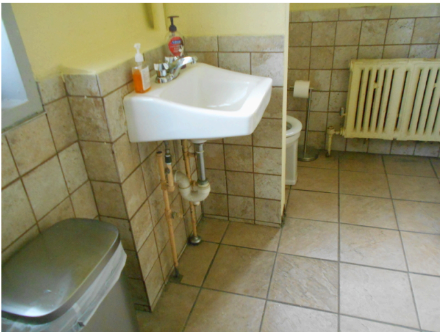
279. Community building, task force headquarters, restroom 2 sink, no scald abrasion protection (Critical Repair)
