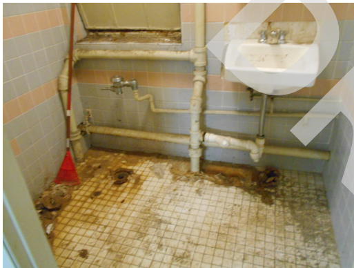
Building 30 basement sink
