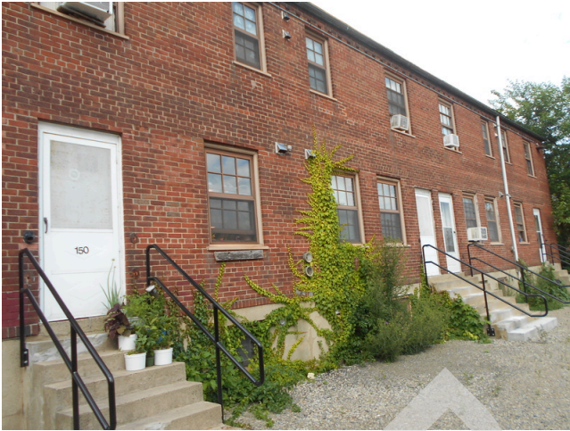
105. Building 5 rear façade
