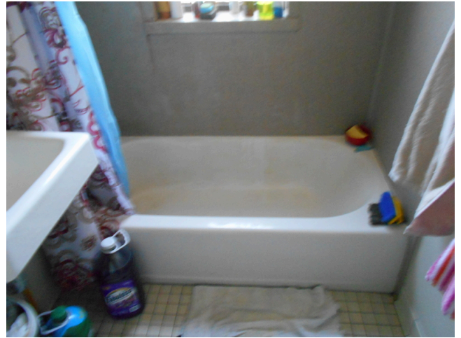
54. Building 2 unit 222, 2br/1ba - Bathroom
