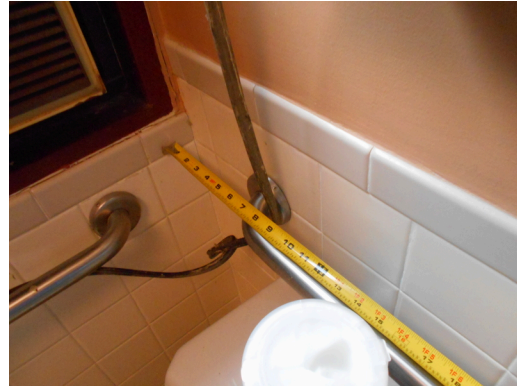
Leasing office public restroom rear grab bar
