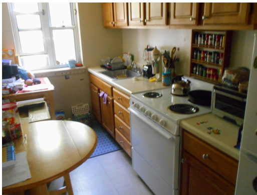
Building A, Unit 7, 1br/1ba - Kitchen
