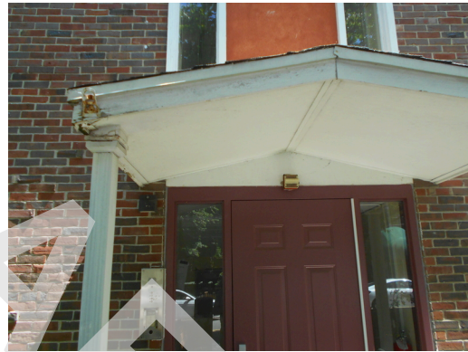
Building D common stairwell entrance
