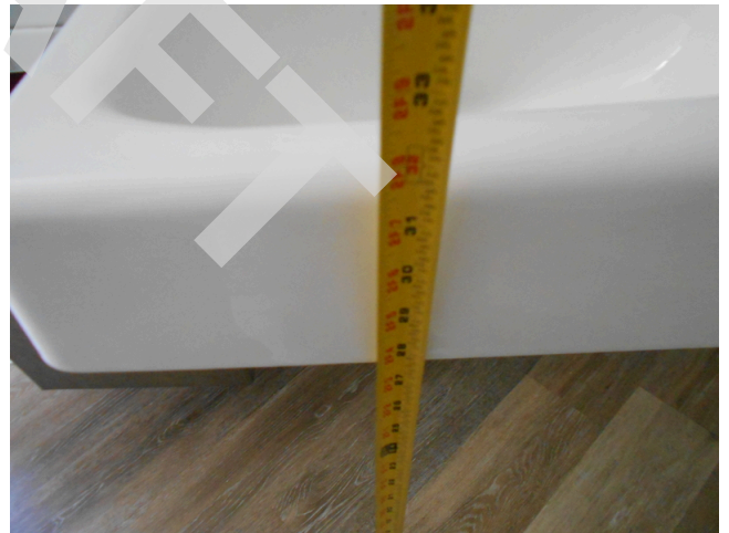
32. Men's public restroom sink height, 32"
