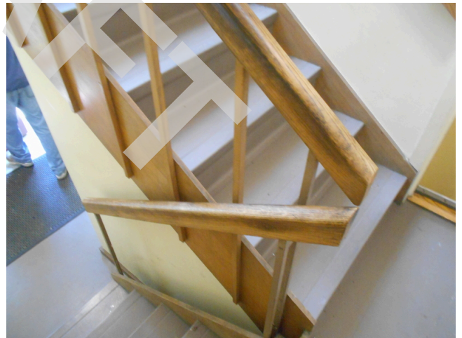
116. Typical rear stairwell
