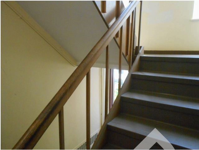
113. Typical rear stairwell
