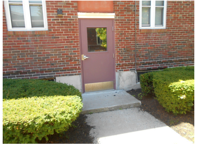
110. Typical rear stairwell
