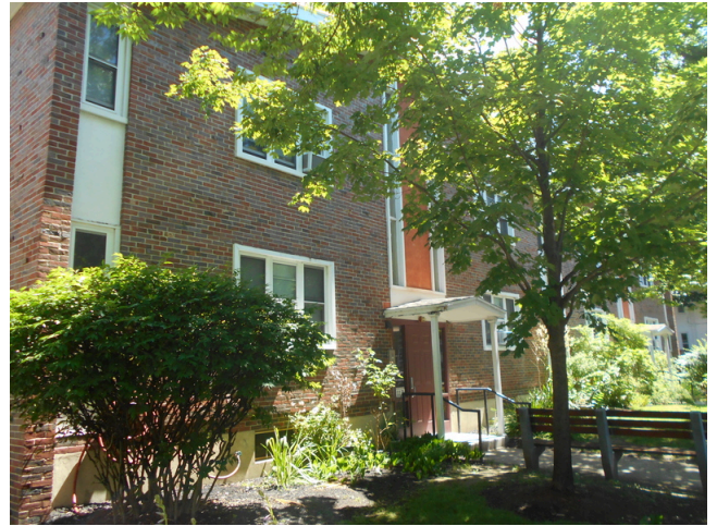
74. Building D front façade
