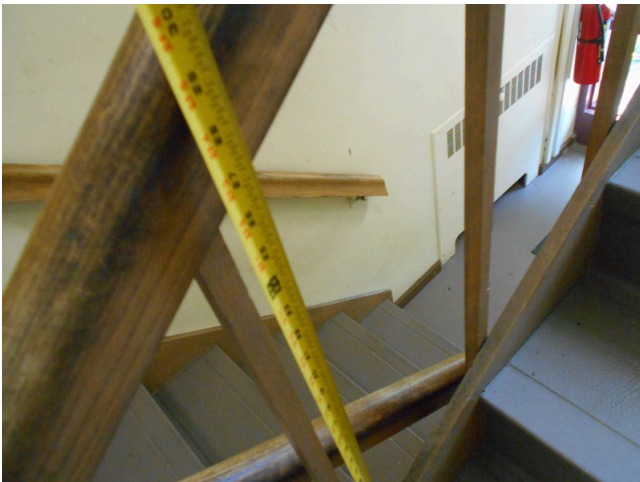
115. Typical rear stairwell
