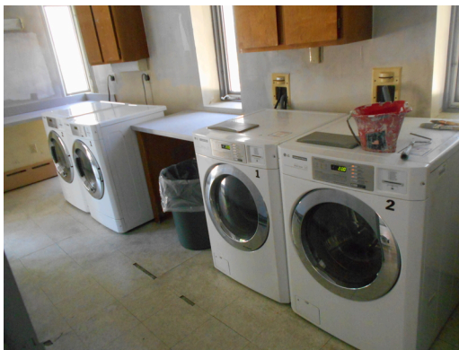
Community building laundry room
