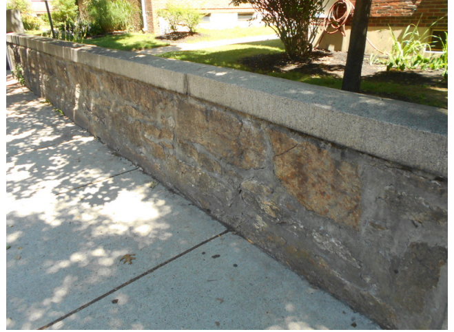
82. Stone fence wall along pond street
