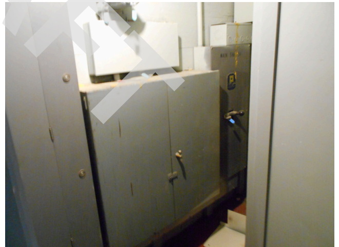
52. Basement electrical room
