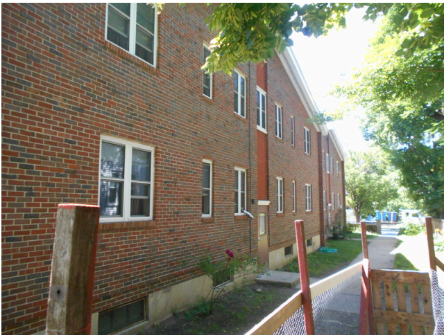
91. Building B rear façade
