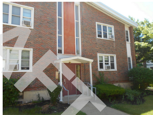
Building B front façade
