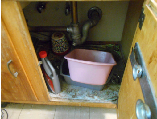
Building B, Unit 27, 2br/1ba - Kitchen sink piping and cabinetry
