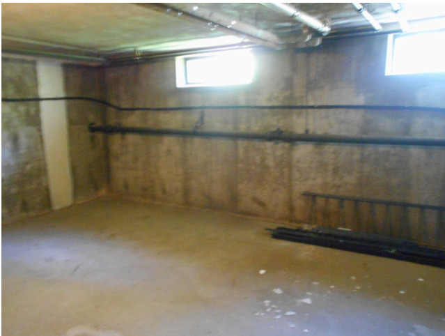
67. Building B basement
