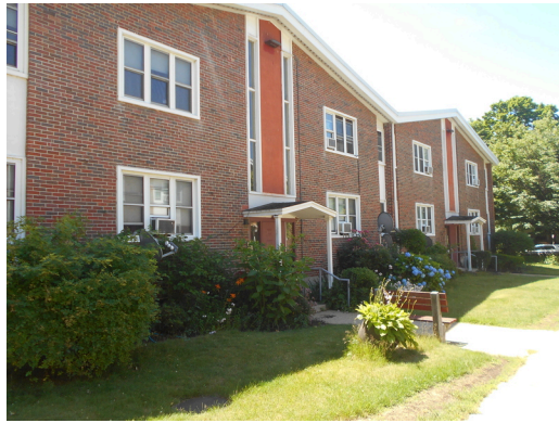
Building C front façade
