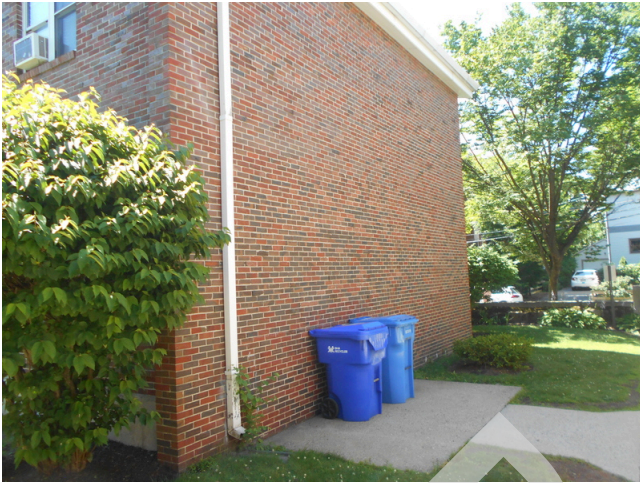
77. Building D side façade
