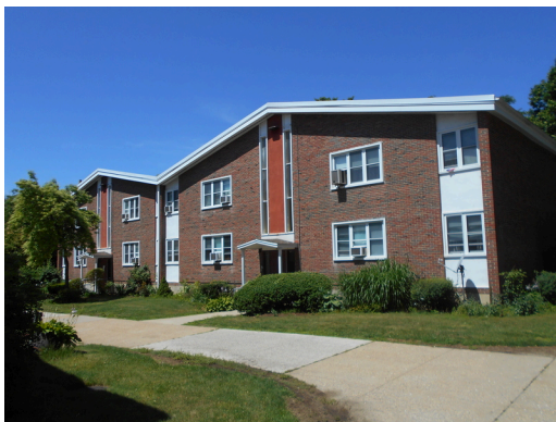
Building B front façade
