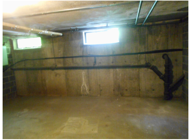
66. Building B basement
