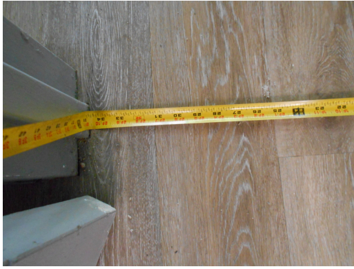
Community building entrance to men's restroom
