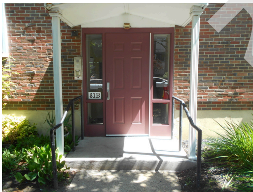
Building D common stairwell entrance
