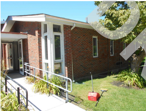
Community building side façade
