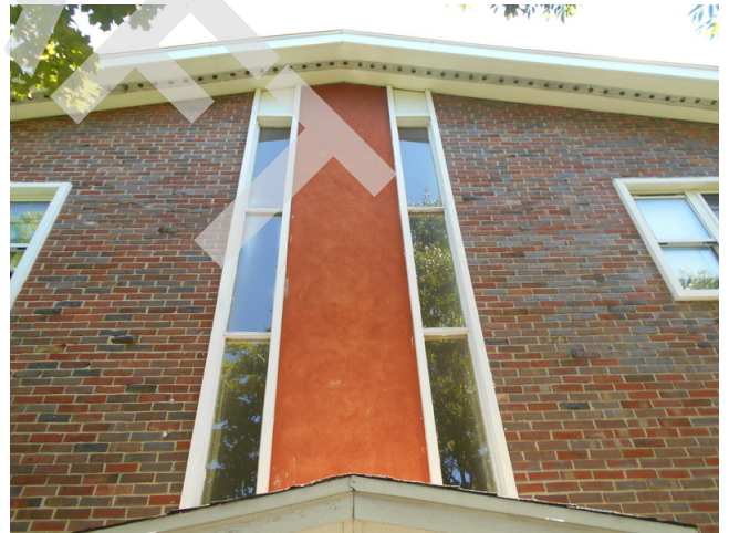
80. Building D common stairwell entrance
