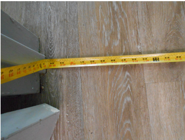
27. Community building entrance to men's restroom
