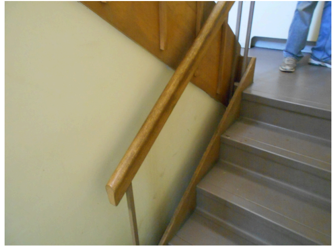
114. Typical rear stairwell
