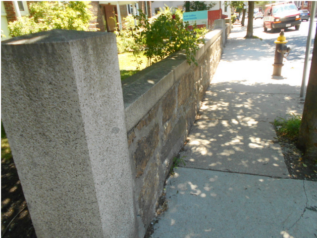
83. Stone fence wall along pond street
