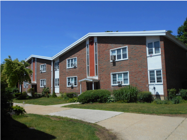
87. Building B front façade
