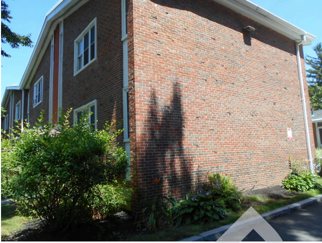
81. Building D side façade
