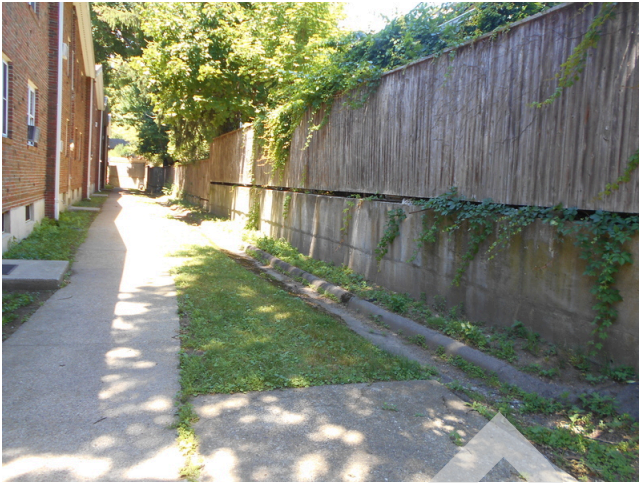
97. Building wood fencing and concrete retaining wall
