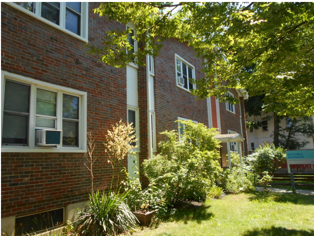
75. Building D front façade
