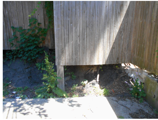
Building wood fencing and concrete retaining wall
