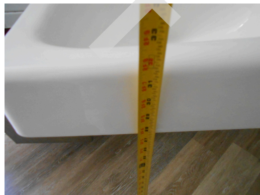
Men's public restroom sink height, 32"
