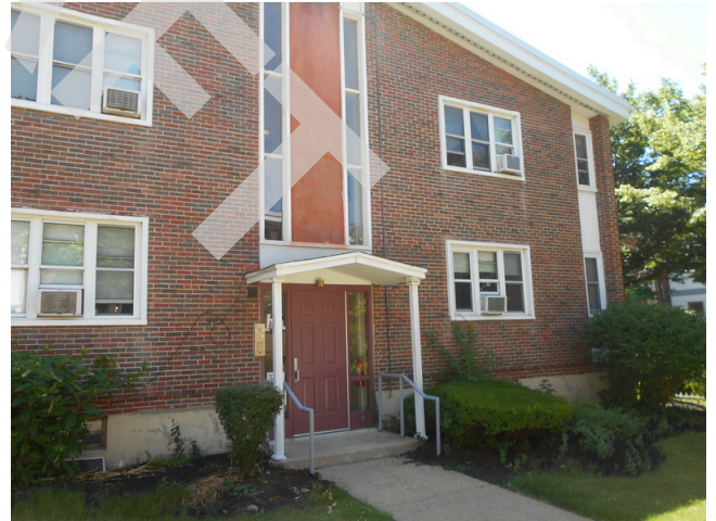
88. Building B front façade
