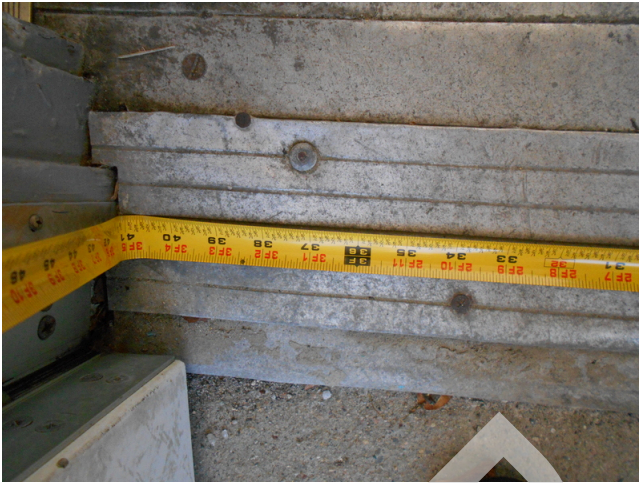
25. Community building entrance, 41"
