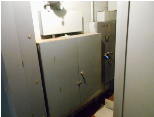
Basement electrical room
