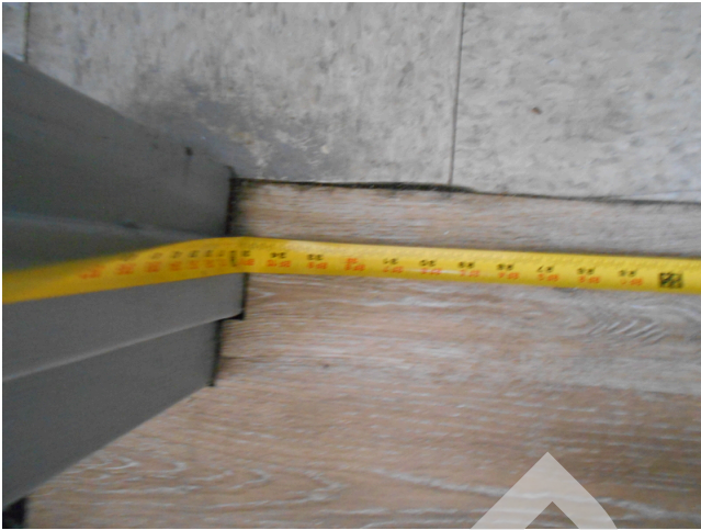
41. Community building laundry room entrance, 34"
