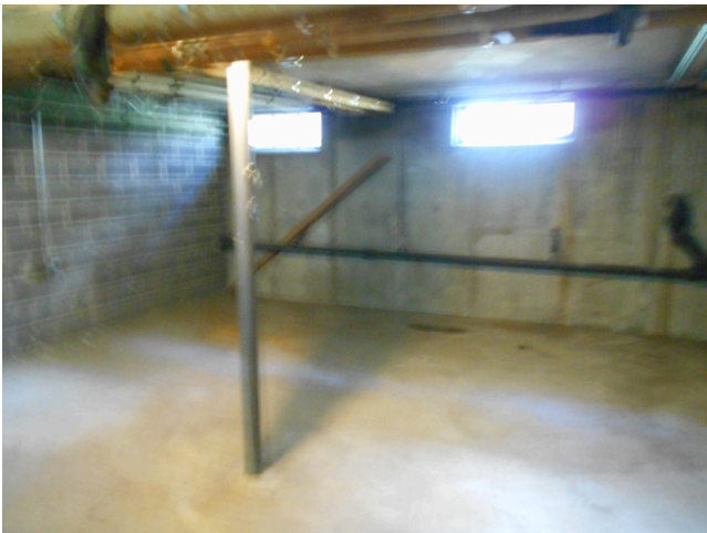
71. Building D basement
