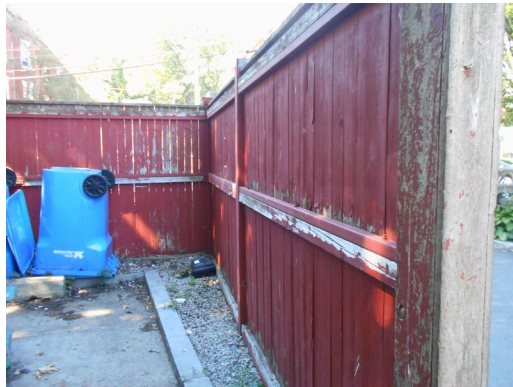
Refuse area wood fencing
