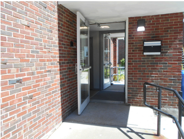
23. Community building entrance
