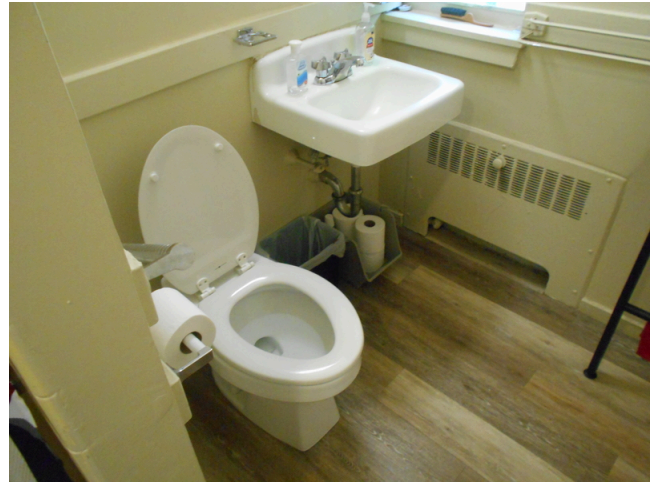
10. Building A, Unit 9, 1br/1ba - Bathroom
