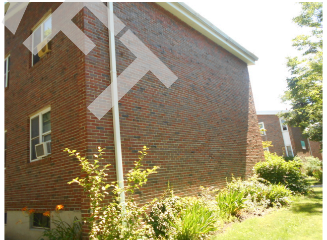
92. Building B Side façade
