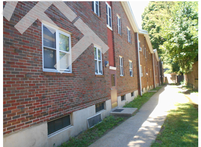
96. Building A rear façade
