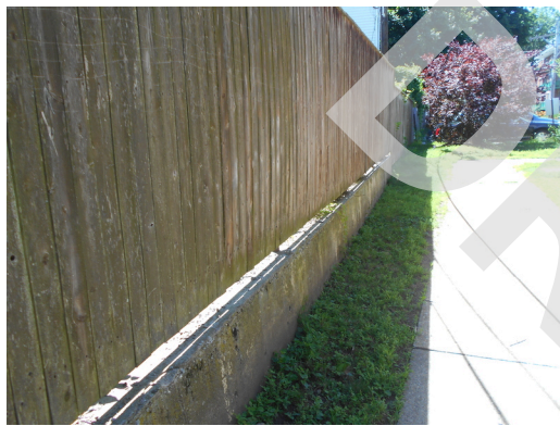
Building wood fencing and concrete retaining wall
