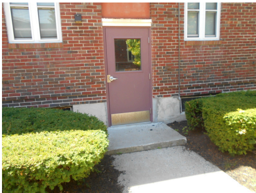
Typical rear stairwell
