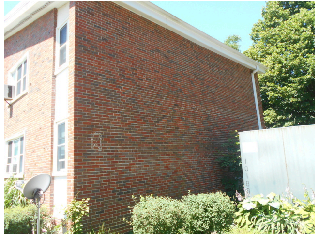
90. Building B side façade
