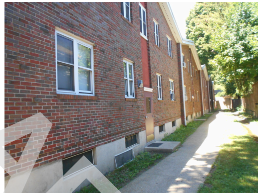
Building A rear façade
