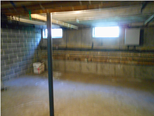
63. Building A basement
