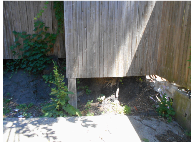
98. Building wood fencing and concrete retaining wall
