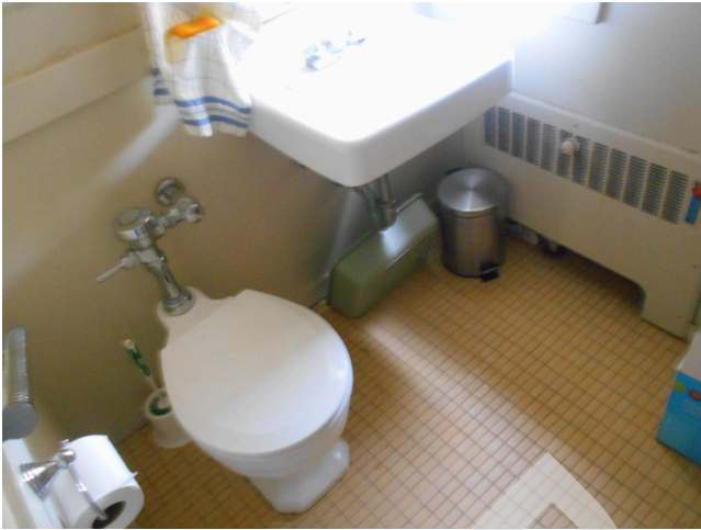
17. Building A, Unit 7, 1br/1ba - Bathroom
