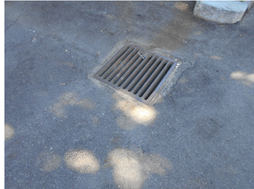
Parking lot drainage
