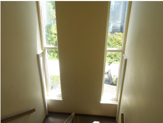
111. Typical rear stairwell
