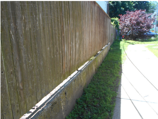
99. Building wood fencing and concrete retaining wall
