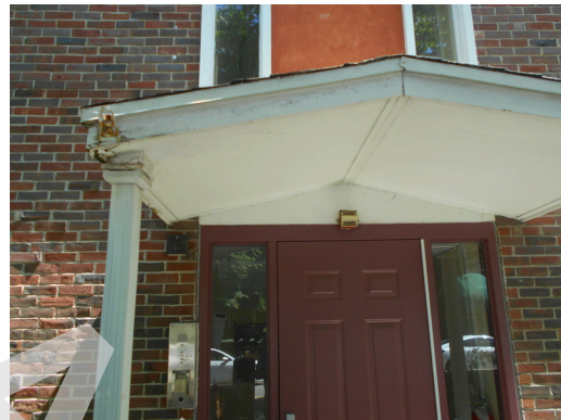
Building D common stairwell entrance
