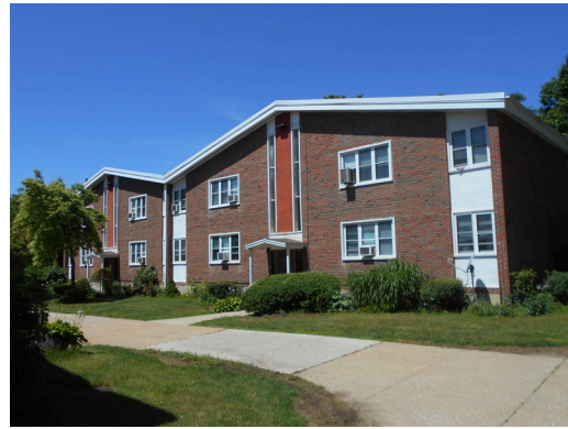
Building B front façade
