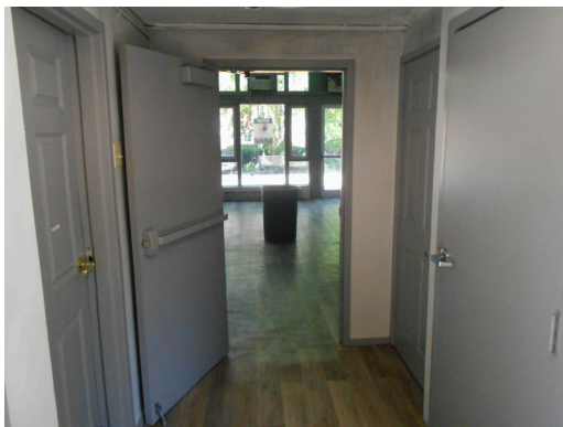
Community building, entrance to main room and restrooms
