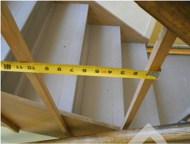
117. Typical rear stairwell, 10" between bars
