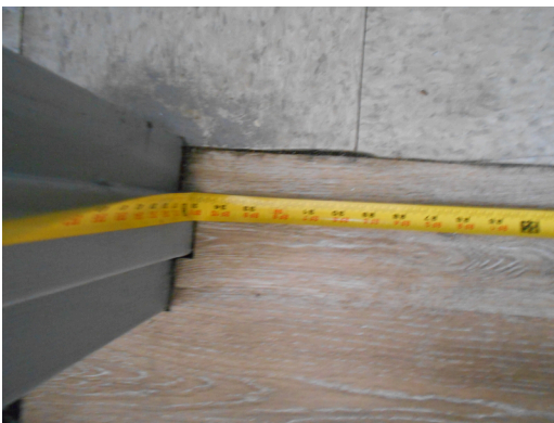
Community building laundry room entrance, 34"
