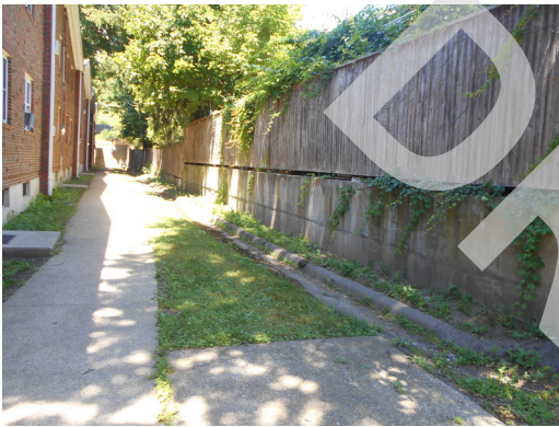
Building wood fencing and concrete retaining wall
