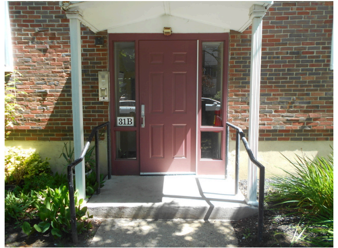
78. Building D common stairwell entrance
