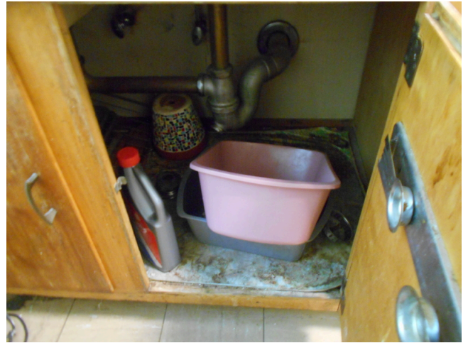
22. Building B, Unit 27, 2br/1ba - Kitchen sink piping and cabinetry
