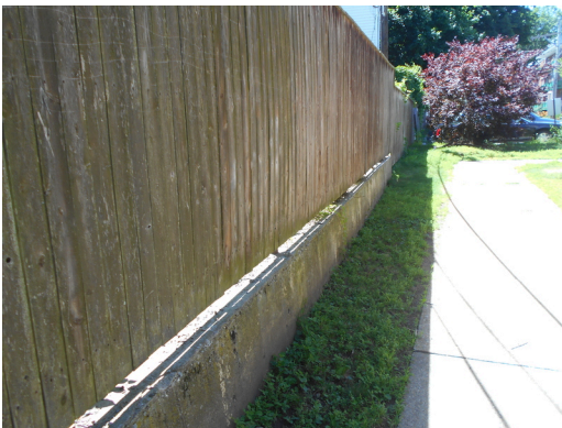
Building wood fencing and concrete retaining wall
