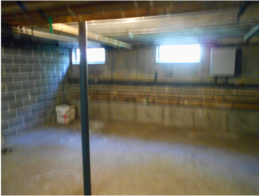
Building A basement
