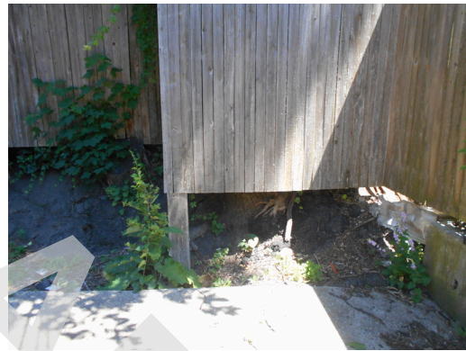
Building wood fencing and concrete retaining wall
