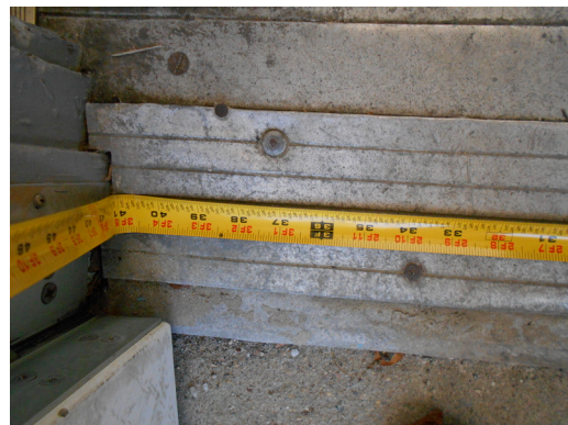
Community building entrance, 41"
