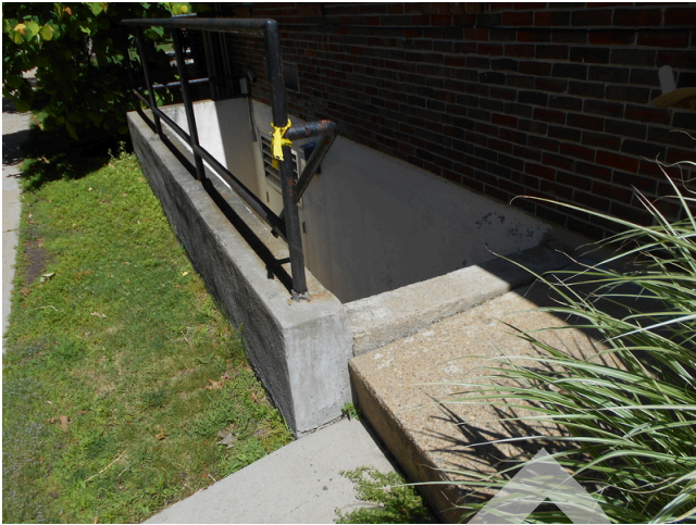
21. Community building, stairwell to basement
