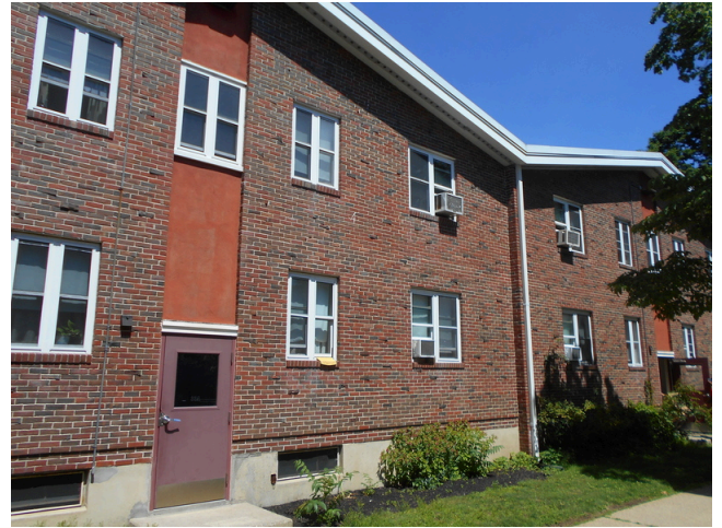
86. Building C rear façade
