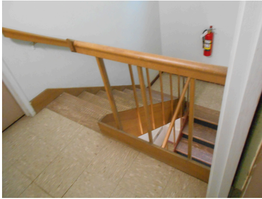
Typical rear stairwell
