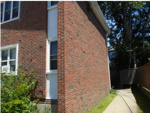
95. Building A side façade
