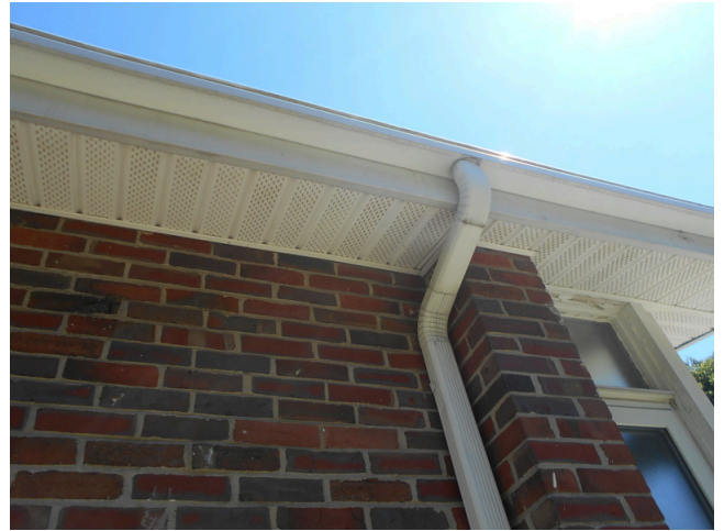
22. Community building typical soffit
