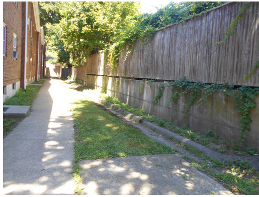
Building wood fencing and concrete retaining wall
