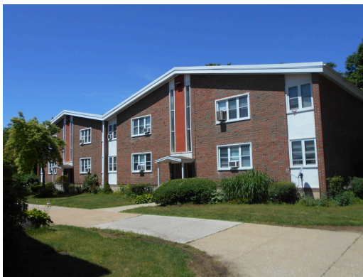
Building B front façade
