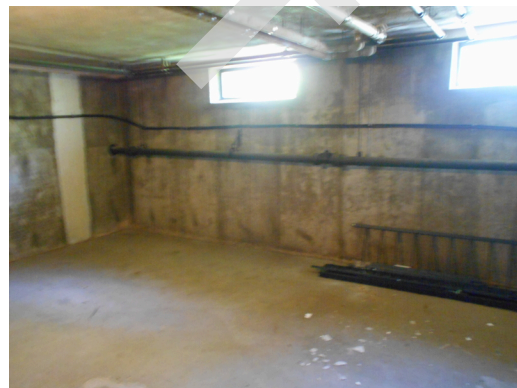
Building B basement
