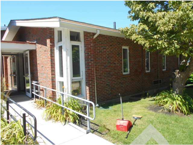
17. Community building side façade
