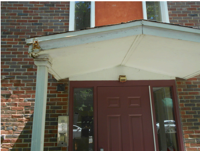
79. Building D common stairwell entrance
