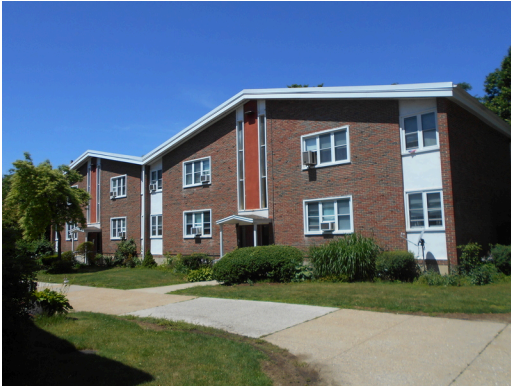
Building B front façade
