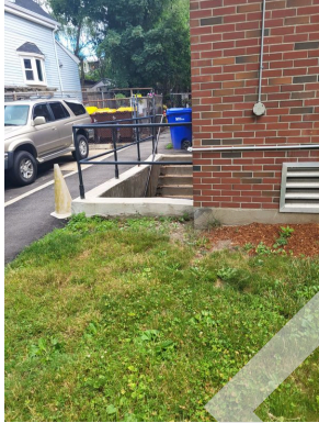
Basement ingress/egress stairs
