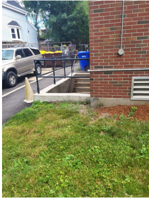
Basement ingress/egress stairs
