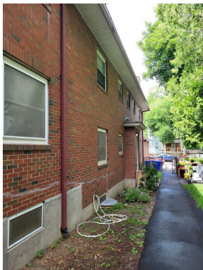
Apartment building fascia
