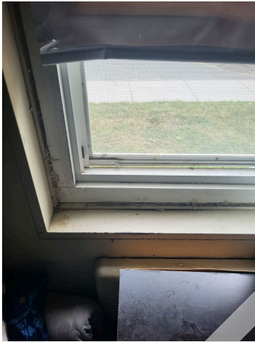
85. Apartment 364-36 bedroom window and frame
