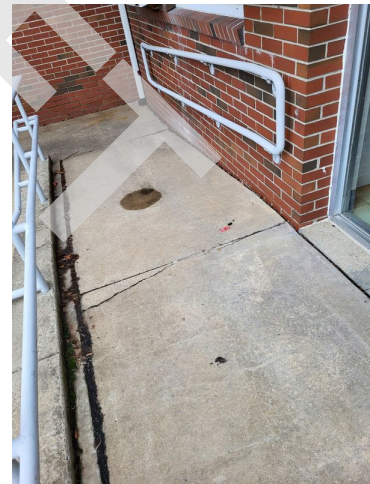
40. Building ingress/egress handicap ramp
