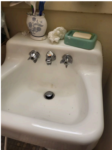
123. Apartment 342-1 bathroom sink and faucet
