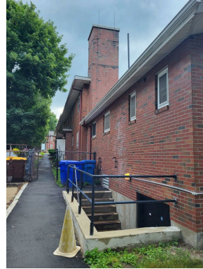
Basement ingress/egress stairs
