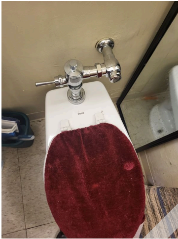
89. Apartment 364-36 bathroom toilet
