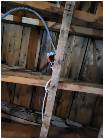
51. Common area restroom roofing
