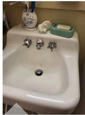
Apartment 342-1 bathroom sink and faucet
