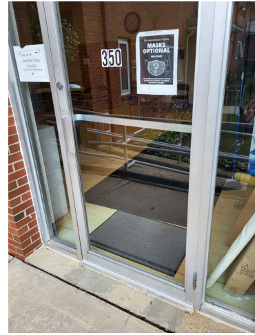
38. Building ingress/egress door
