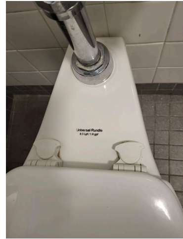
58. Common area restroom toilet gallons per flush
