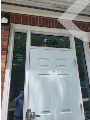
Apartment building 342-356 ingress/egress door
