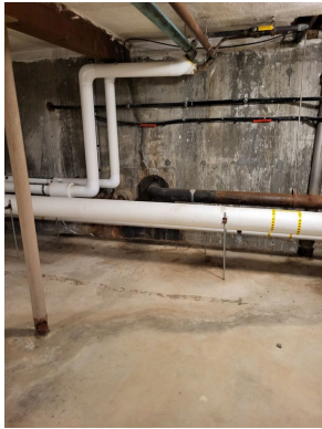
Basement PVC pipe
