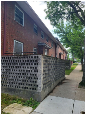
Exterior concrete block wall
