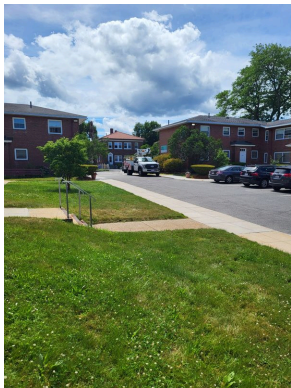
Property parking lot (Non-Critical Repair)
