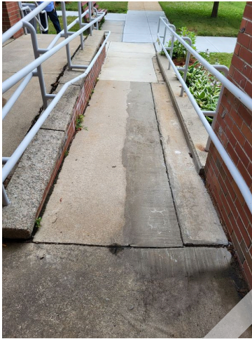
41. Building ingress/egress handicap ramp
