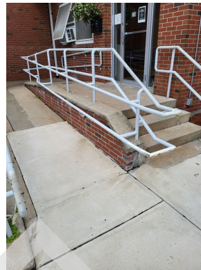
Building ingress/egress stairs and handicap ramp railings
