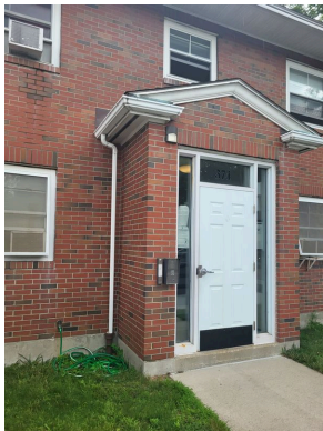
Apartment building 358-374 building ingress/egress door
