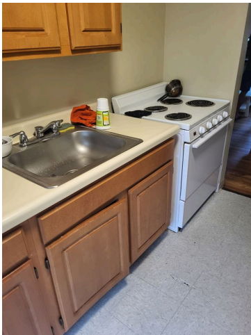
79. Apartment 364-36 kitchen cabinets, sink, faucet, countertop and range/stove
