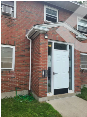
Apartment building 358-374 building ingress/egress door
