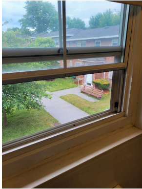
Apartment 346-10 bedroom window and frame
