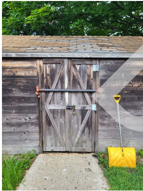
Property storage shed
