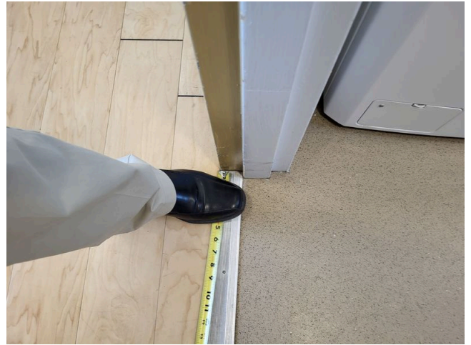
6. Common area laundry room doorway floorspace
