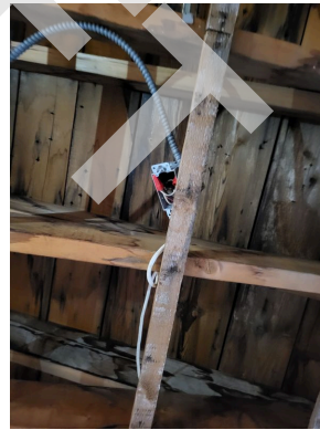
Common area restroom roofing
