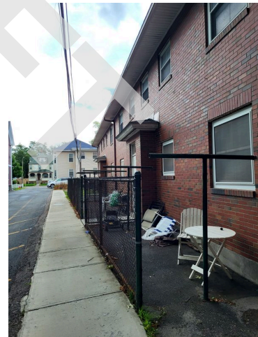
132. Apartment building chain link fence
