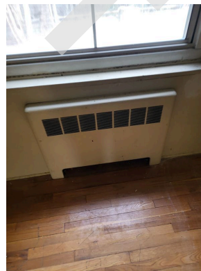
Apartment 356-25 bedroom window, frame and radiator
