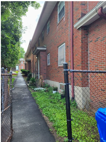
131. Apartment building chain link fence and gutter/ down spout
