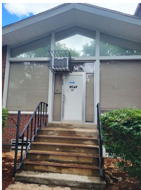
Common area ingress/egress stairs and railings
