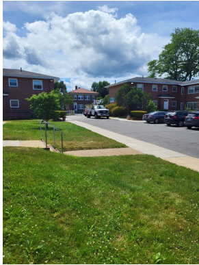
Property parking lot (Non-Critical Repair)
