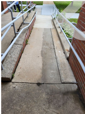
Building ingress/egress handicap ramp
