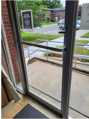
Building ingress/egress door
