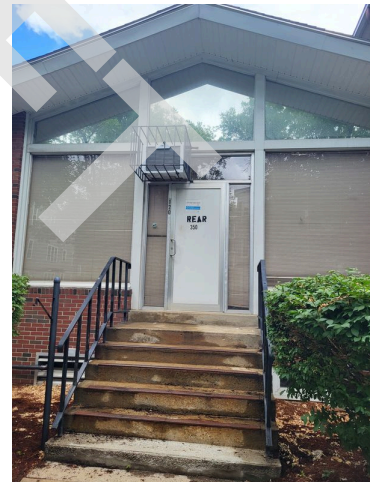
68. Common area ingress/egress stairs and railings
