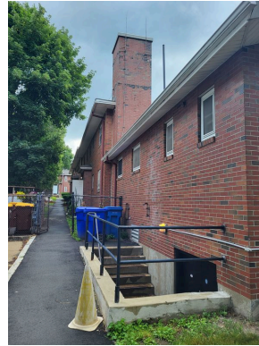
Basement ingress/egress stairs
