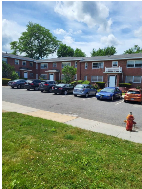
Property parking lot (Non-Critical Repair)
