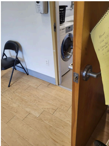
3. Common area laundry room door hardware
