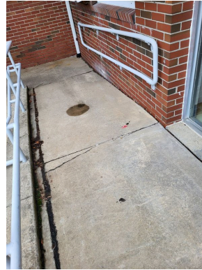
Building ingress/egress handicap ramp
