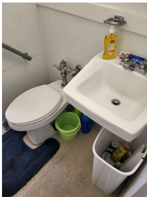
Apartment 352-19 bathroom toilet, sink a faucet
