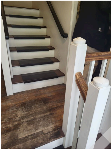
89. Apartment building 358-374 ingress/egress interior stairs
