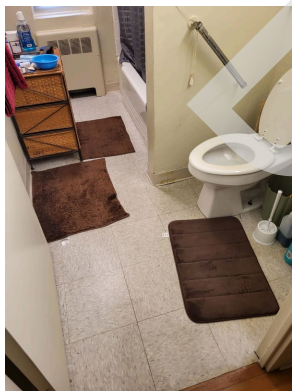
Apartment 354-21 bathroom floor
