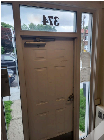
101. Apartment building 358-374 common door ingress/egress
