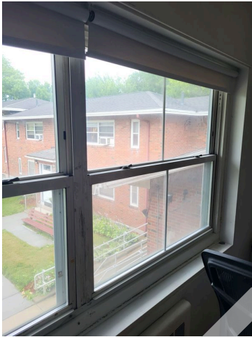
25. Apartment 352-19 living room area windows and frame
