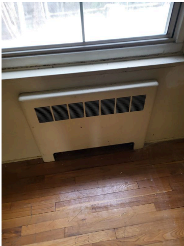
59. Apartment 356-25 bedroom window, frame and radiator
