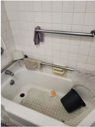
109. Apartment 374-54 bathroom bathtub hardware
