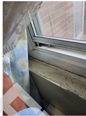
Apartment 342-1 kitchen window and frame
