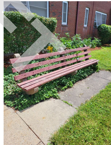
80. Exterior common area bench (Non-Critical Repair)
