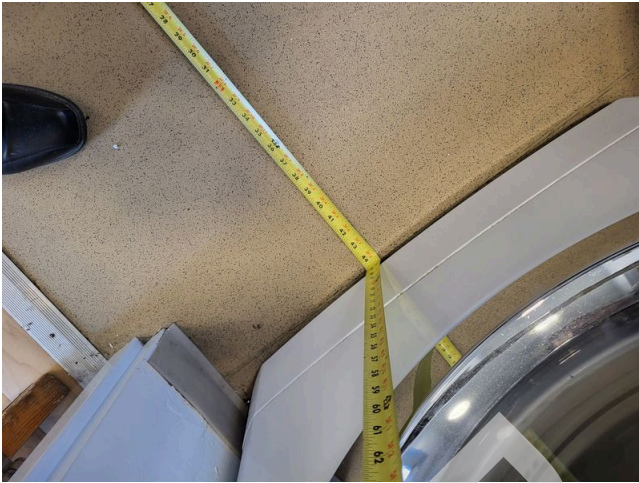
9. Common area laundry room floorspace
