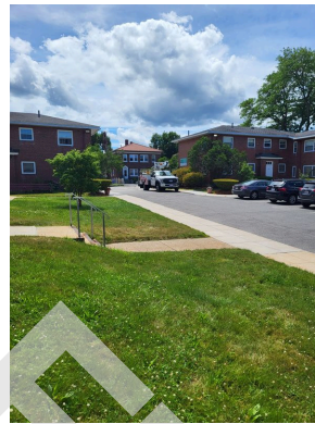
Property parking lot (Non-Critical Repair)
