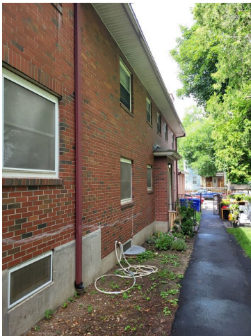
135. Apartment building fascia
