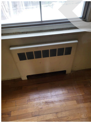
Apartment 356-25 bedroom window, frame and radiator
