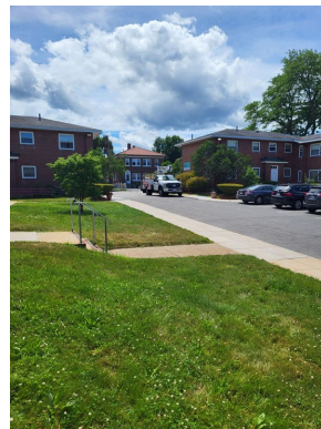
Property parking lot (Non-Critical Repair)
