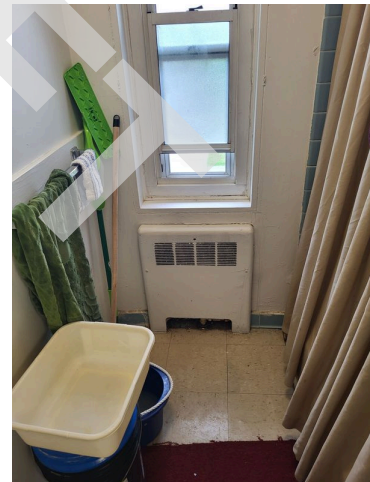
36. Apartment 352-19 bathroom radiator and window
