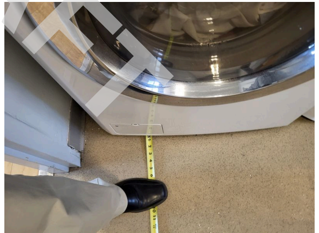
8. Common area laundry room floorspace
