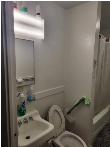
107. Apartment 374-54 bathroom toilet, grab bar, sink, faucet and medicine cabinet
