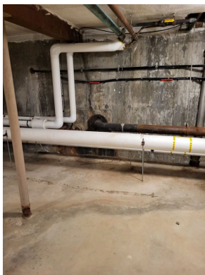
Basement PVC pipe
