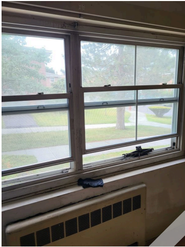
53. Apartment 356-25 living room area windows and frame
