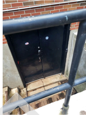
Basement ingress/egress doors
