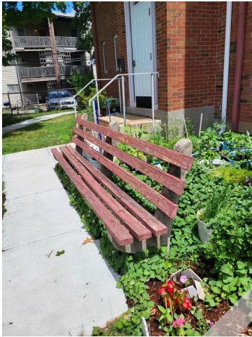
81. Exterior common area bench (Non-Critical Repair)
