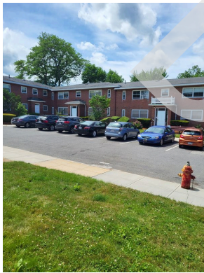
Property parking lot (Non-Critical Repair)
