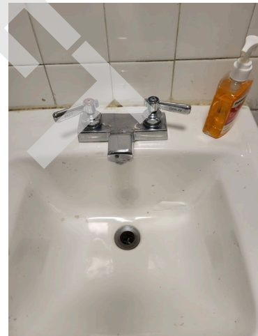
56. Common area restroom sink and faucet
