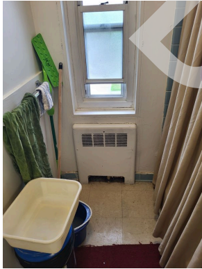
Apartment 352-19 bathroom radiator and window
