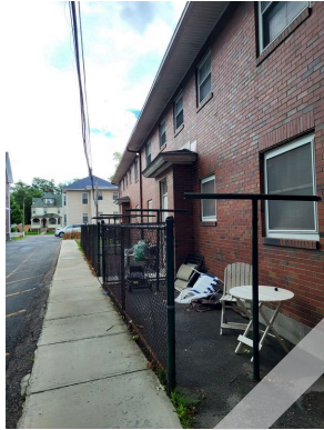
Apartment building chain link fence
