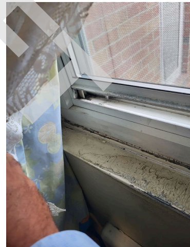
116. Apartment 342-1 kitchen window and frame
