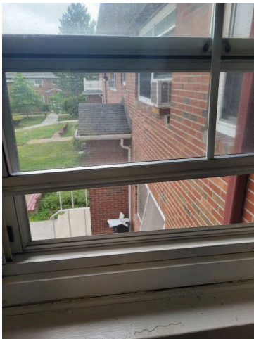
99. Apartment 374-54 living room area window and frame
