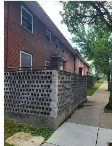
74. Exterior concrete block wall
