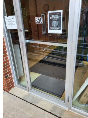
Building ingress/egress door
