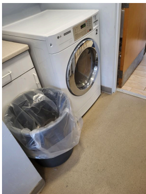
Common area laundry room front load dryer
