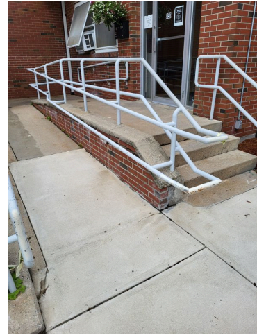
42. Building ingress/egress stairs and handicap ramp railings
