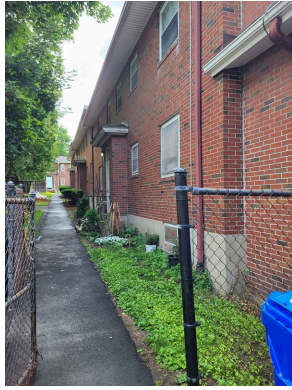
Apartment building chain link fence and gutter/down spout
