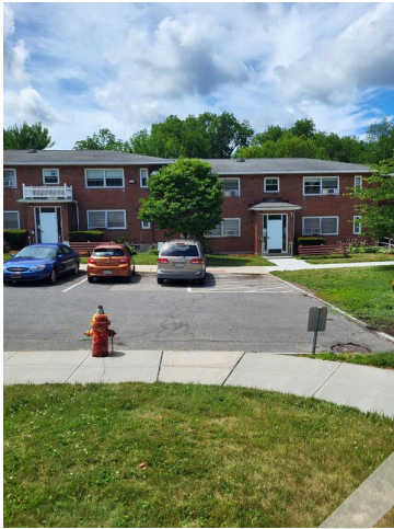
85. Property parking lot install handicap accessible parking (Critical Repair)
