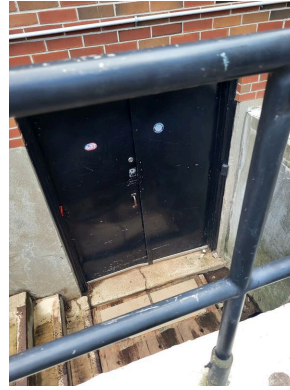
Basement ingress/egress doors
