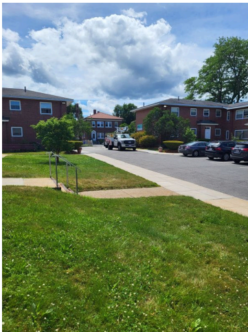
83. Property parking lot (Non-Critical Repair)
