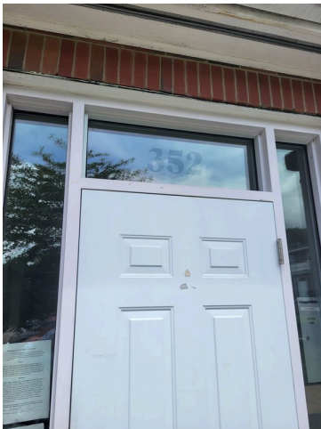
159. Apartment building 342-356 ingress/egress door
