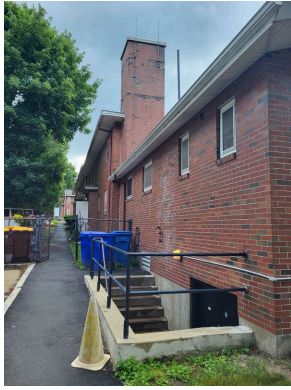
Basement ingress/egress stairs
