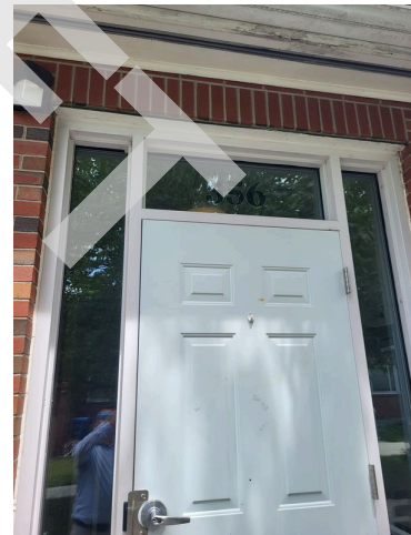
60. Apartment building 342-356 ingress/egress door
