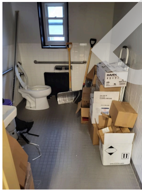
Common area restroom
