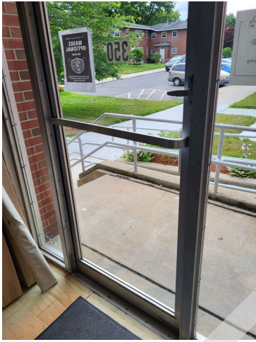
37. Building ingress/egress door
