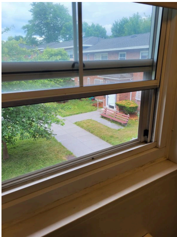
23. Apartment 346-10 bedroom window and frame
