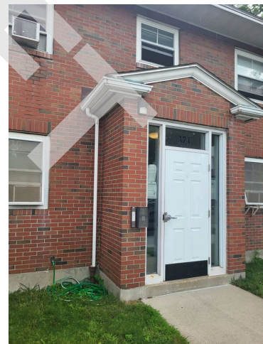
100. Apartment building 358-374 building ingress/egress door
