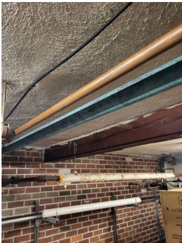
111. Basement support beam
