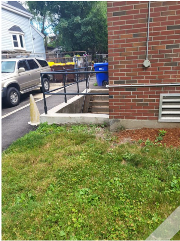
69. Basement ingress/egress stairs
