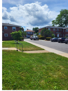
Property parking lot (Non-Critical Repair)
