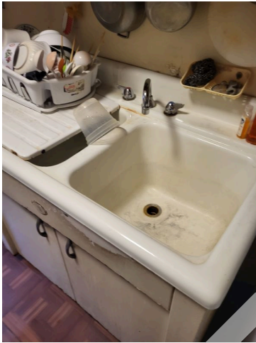
9. Apartment 346-10 kitchen sink
