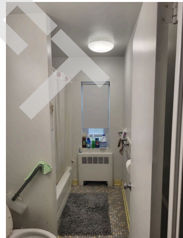
108. Apartment 374-54 bathroom light fixture, window, radiator and floor
