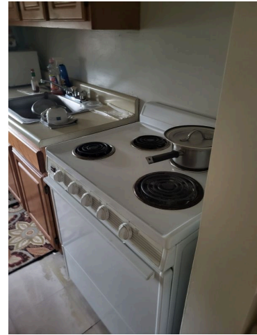
106. Apartment 374-54 kitchen range/stove
