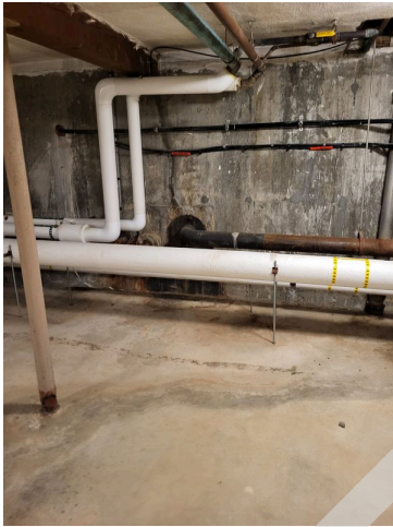
117. Basement PVC pipe
