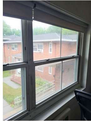
Apartment 352-19 living room area windows and frame
