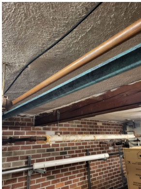
Basement support beam
