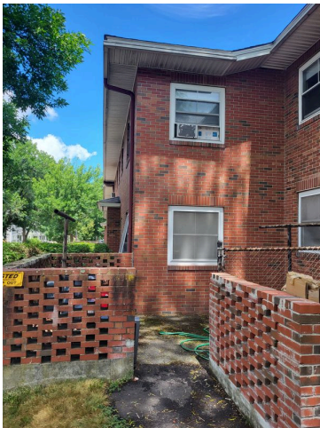
75. Exterior soffit and fascia
