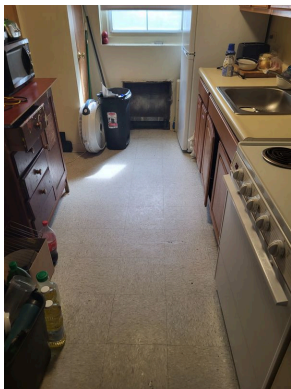
Apartment 364-36 kitchen floor (Non-Critical Repair)
