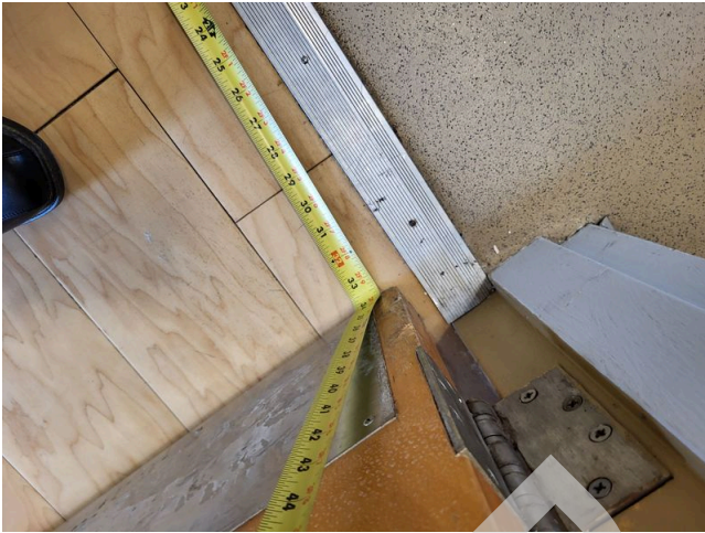
5. Common area laundry room doorway floorspace
