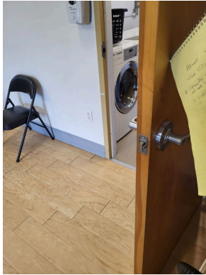
Common area laundry room door hardware
