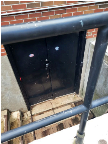
71. Basement ingress/egress doors
