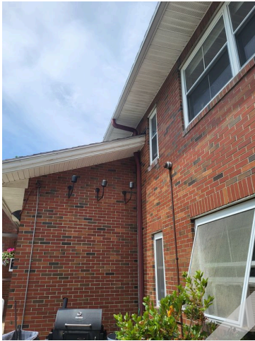
161. Apartment building 342-356 exterior façade, fascia and windows
