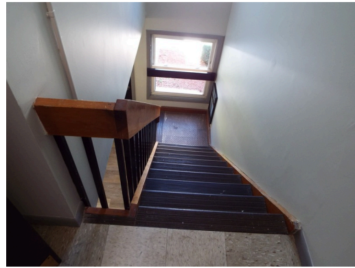
Typical stair - building 110-112
