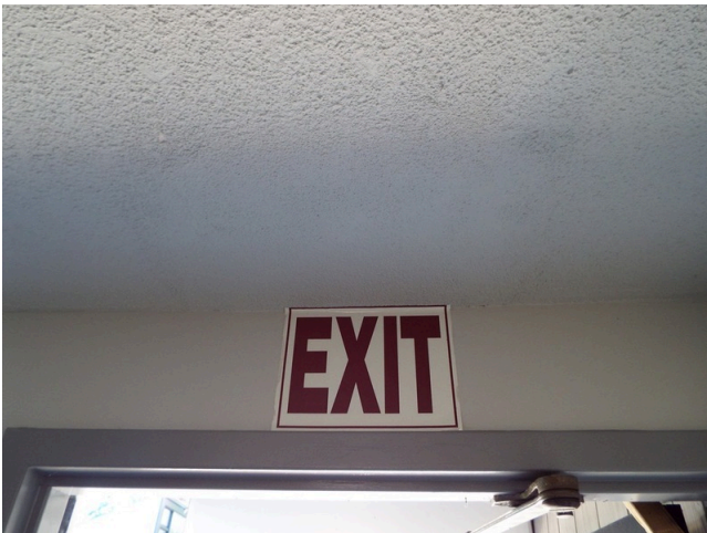
43. Building hallway exit sign
