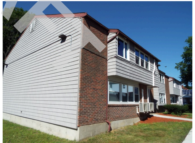
32. Typical brick veneer and vinyl siding
