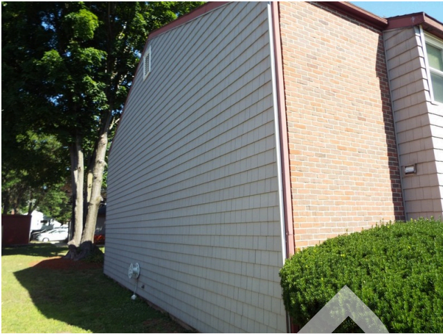
33. Typical vinyl siding
