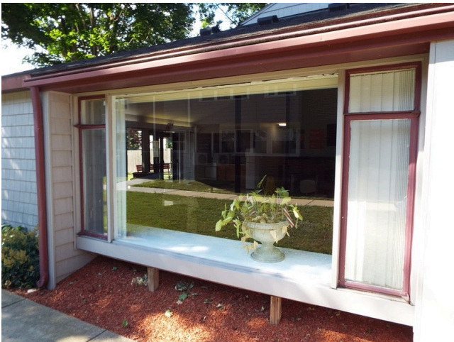
35. Community building - fixed and casement windows
