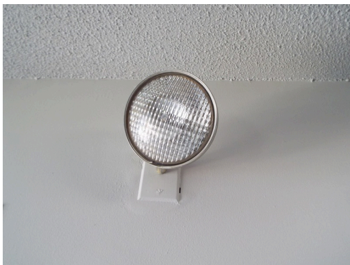
Building hallway emergency light
