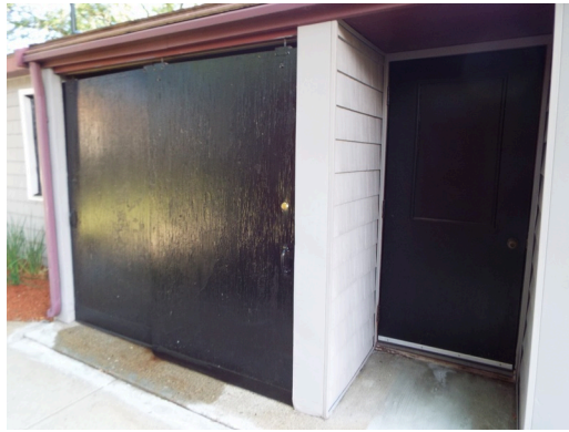
Community building - service doors
