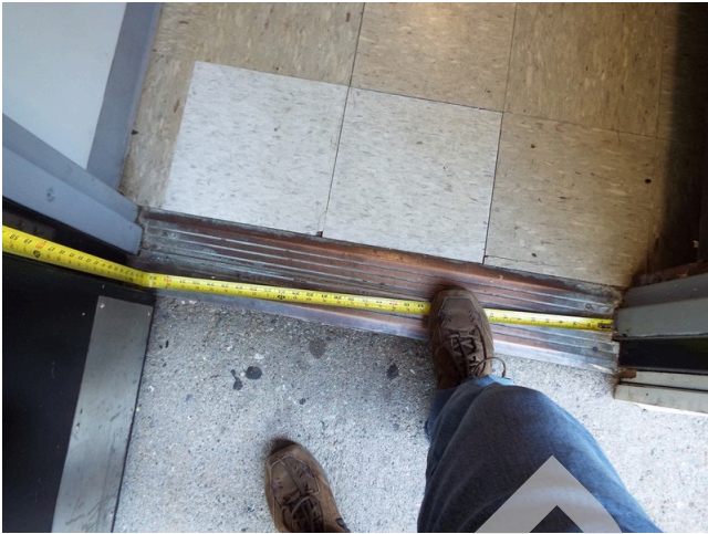
69. Building entry - building 105-109
