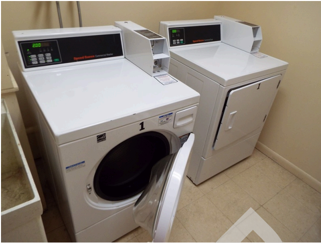
57. Community building - washer lacks front controls (Critical Repair)
