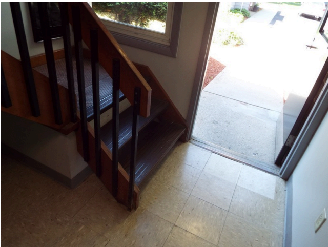
75. Building entry - building 105-109
