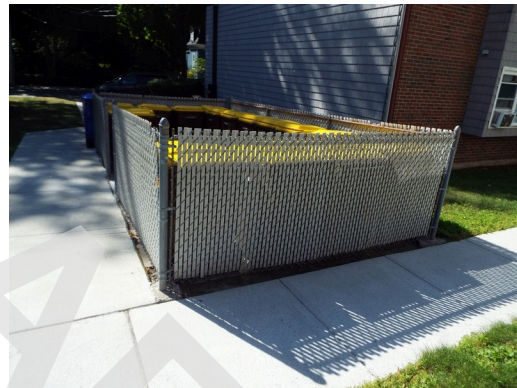
Trash bin enclosure chain link fencing
