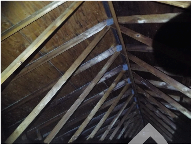
89. Roof framing - building 110-112
