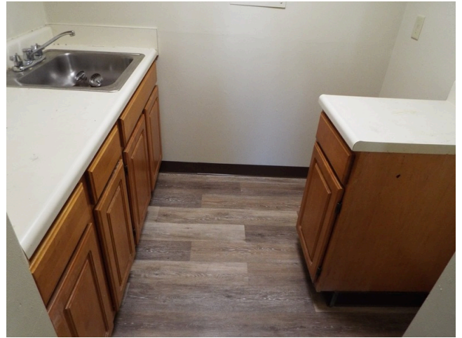
150. 0-bed-1-bath - unit 41 - building 110-112 - kitchen cabinets
