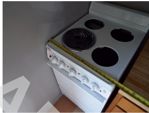
Community building - range lacks 30 inch front approach (Critical Repair)
