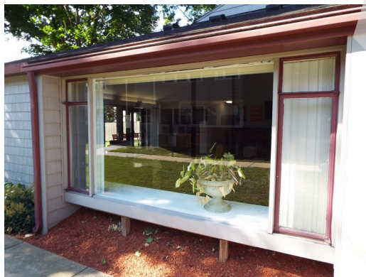
Community building - fixed and casement windows
