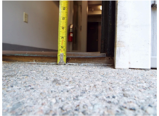
70. Building entry - building 105-109
