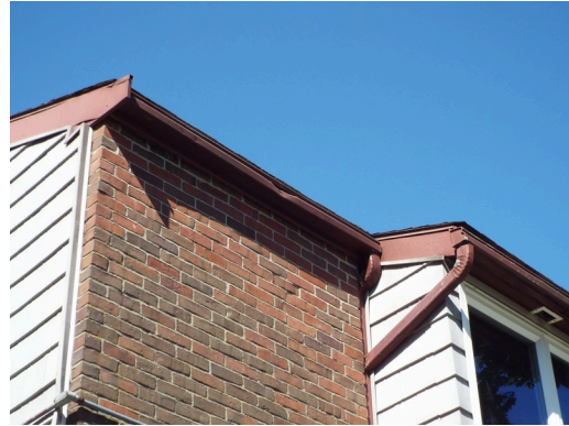
Gutter and downspout
