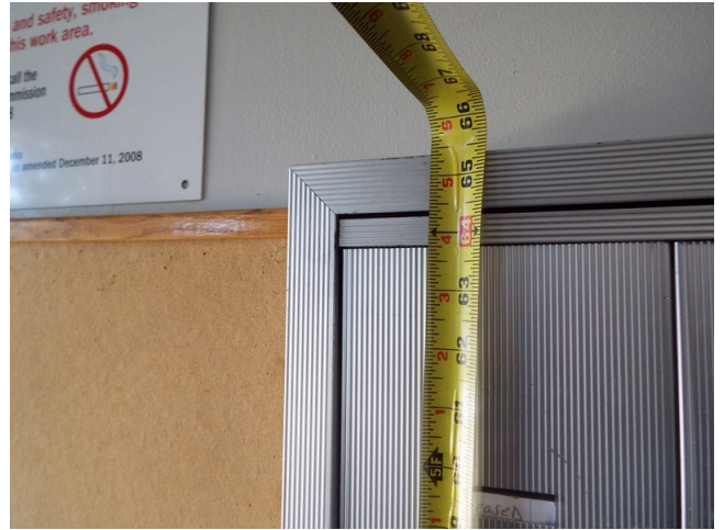
74. Building entry - building 105-109
