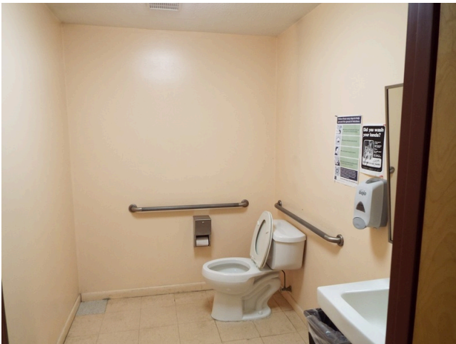
51. Community building - womens restroom
