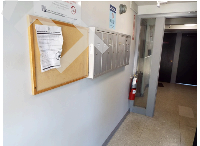
72. Building entry - building 105-109
