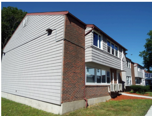
Typical brick veneer and vinyl siding
