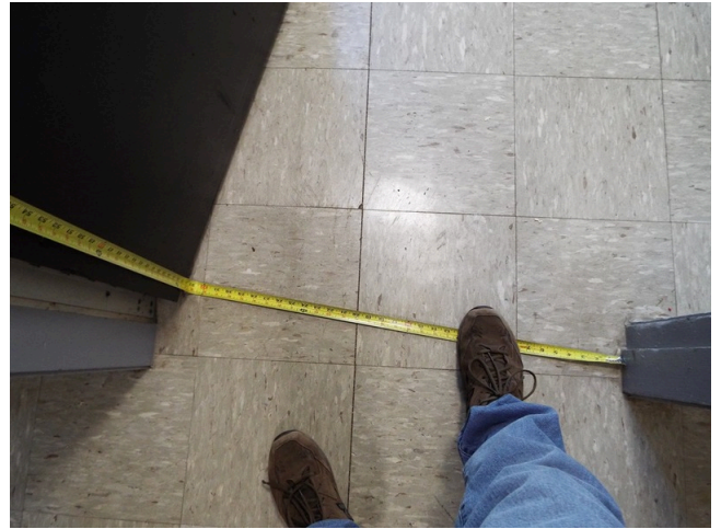
78. Building entry - building 105-109
