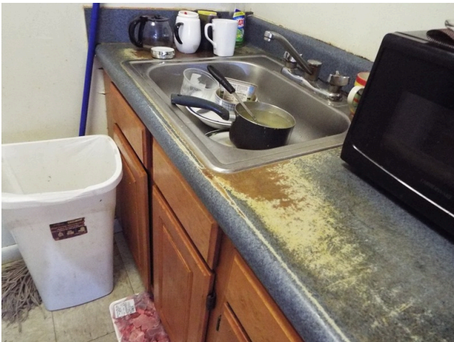
11. 0-bed-1-bath - unit 13 - building 93-95 - countertop condition (Non-Critical Repair)
