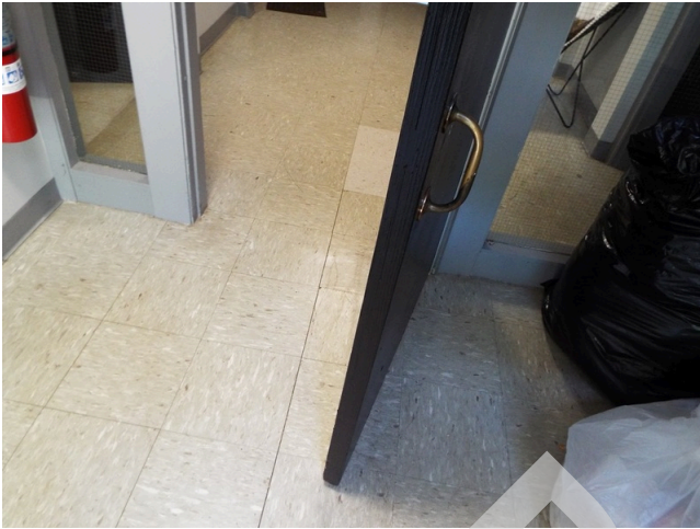
77. Building entry - building 105-109
