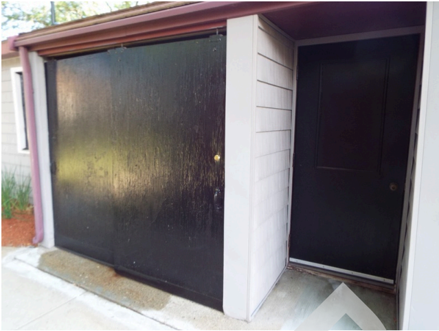
25. Community building - service doors
