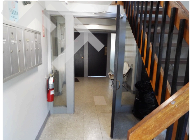
76. Building entry - building 105-109
