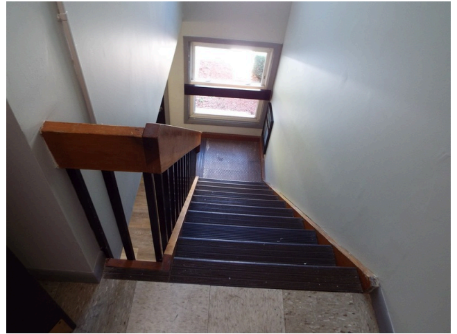
54. Typical stair - building 110-112
