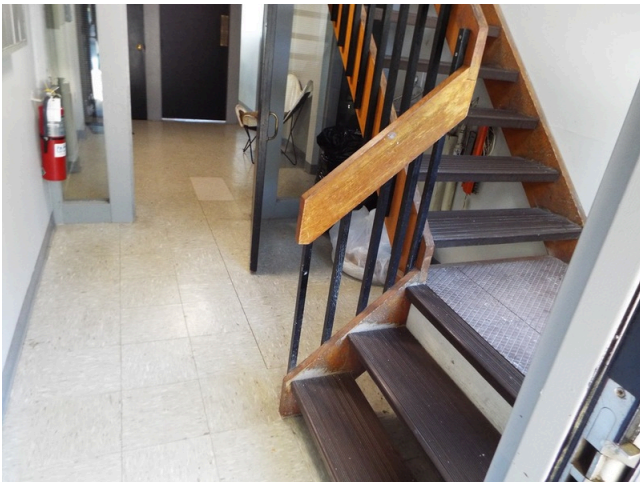
71. Building entry - building 105-109
