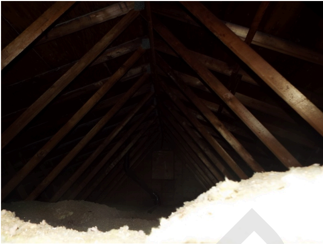
21. Attic insulation - building 110-112
