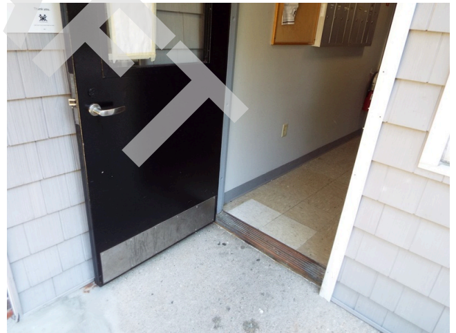
68. Building entry - building 105-109
