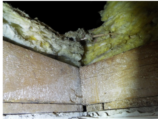
Attic insulation - building 110-112
