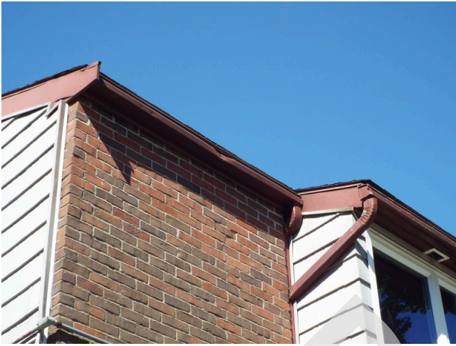
37. Gutter and downspout
