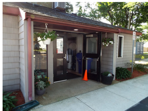
Community building - aluminum storefront entry
