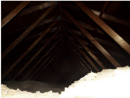
Attic insulation - building 110-112
