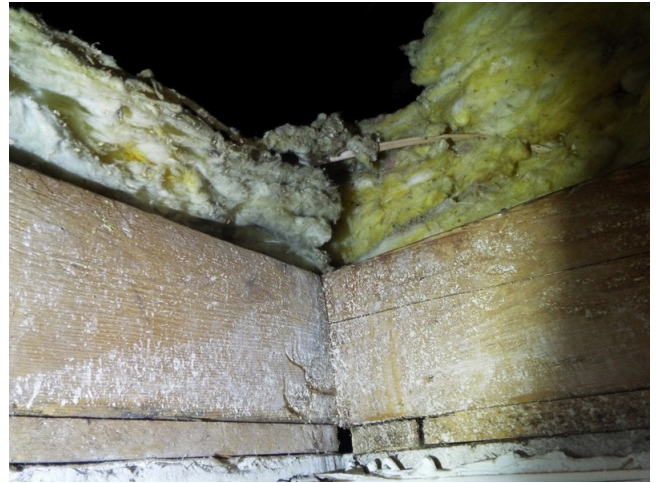
22. Attic insulation - building 110-112
