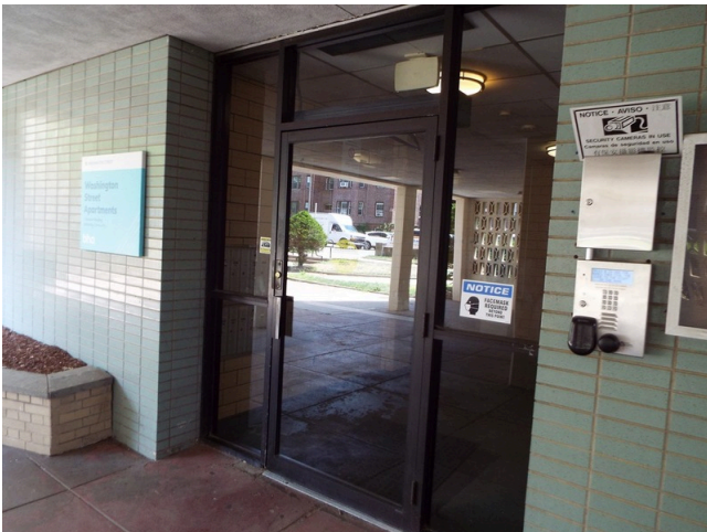
43. Main entry door
