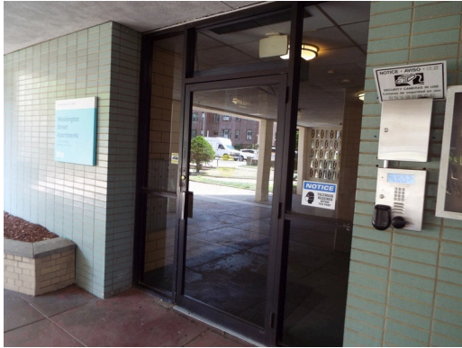
Main entry door
