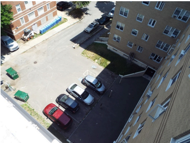
7. Rear parking overview
