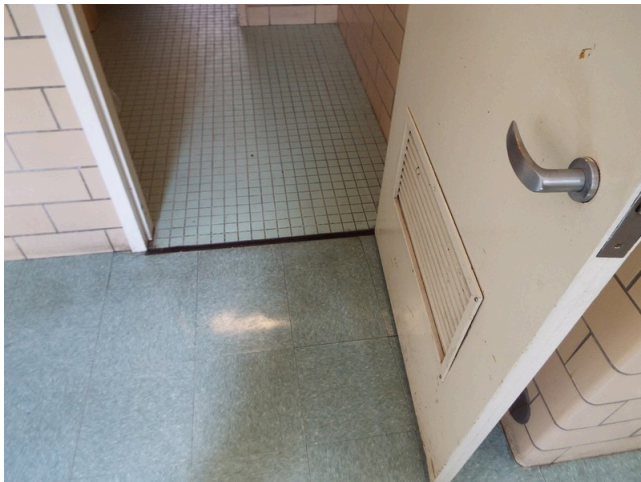
139. Common area - restroom
