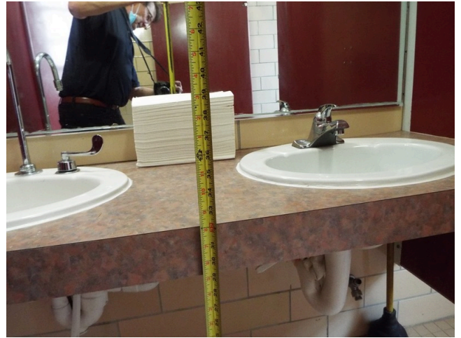
158. Common area - restroom
