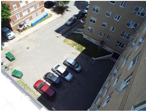
Rear parking overview
