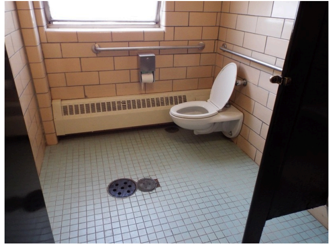
150. Common area - restroom
