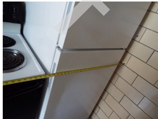
Common area - refrigerator lacks 48 inch side access
