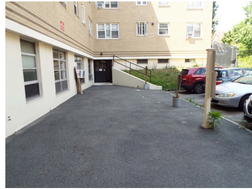
Rear entry asphalt pavement
