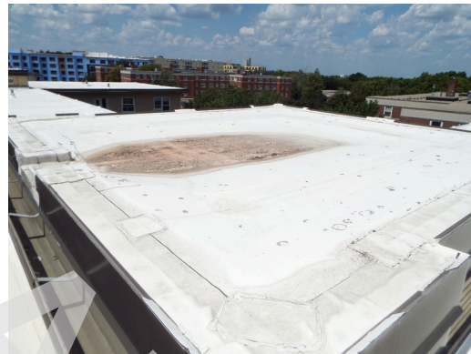
Roof ponding
