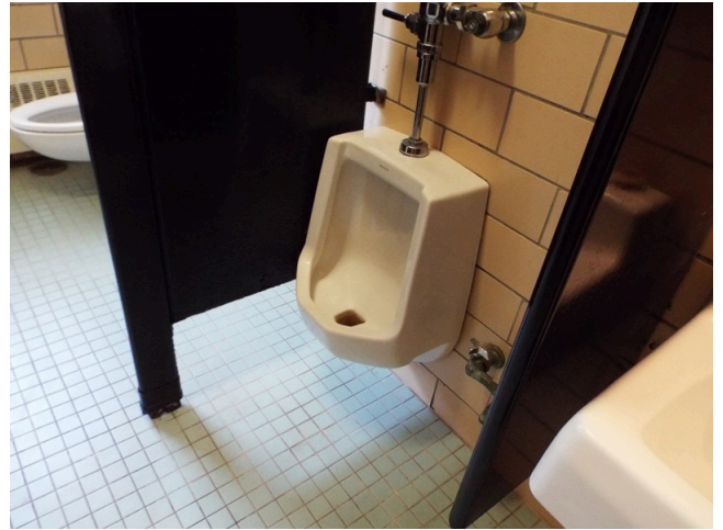
146. Common area - restroom
