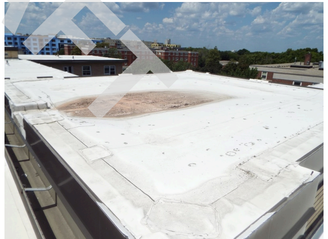
60. Roof ponding
