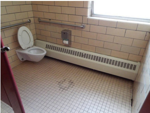
159. Common area - restroom
