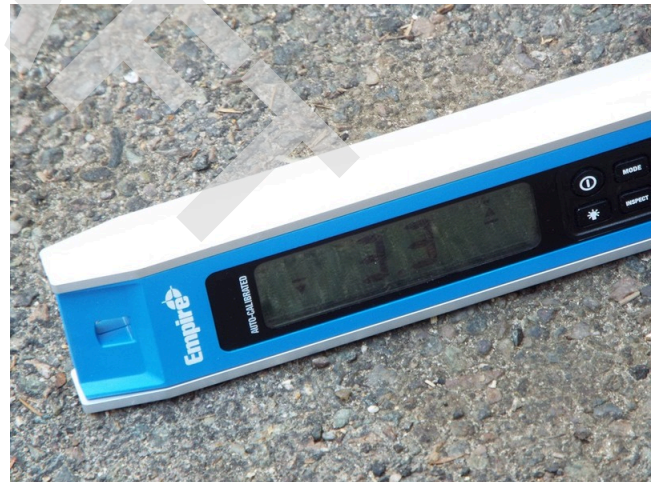
88. Accessible parking - running slope exceeds allowable (Critical Repair)
