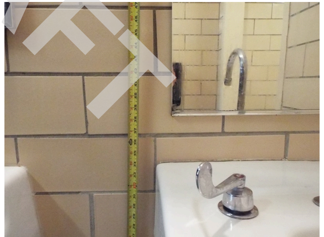
144. Common area - restroom
