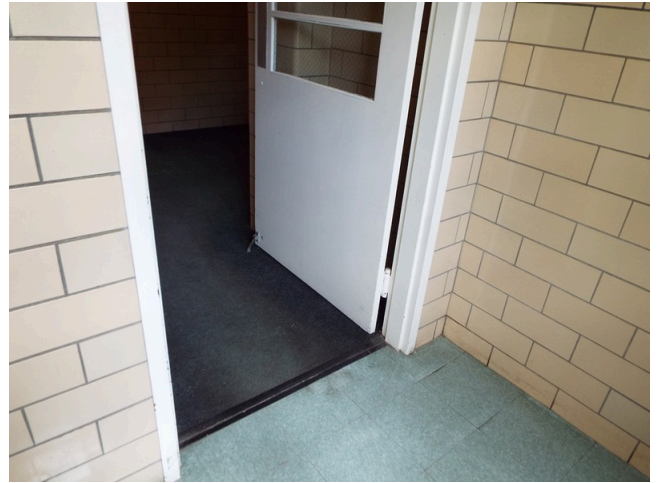
126. Common area - community room
