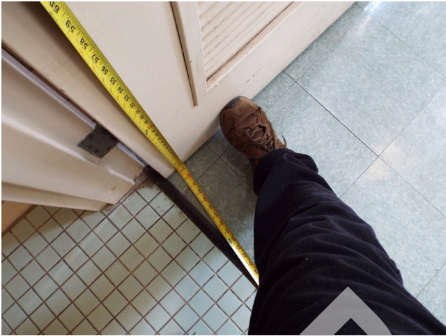
141. Common area - restroom
