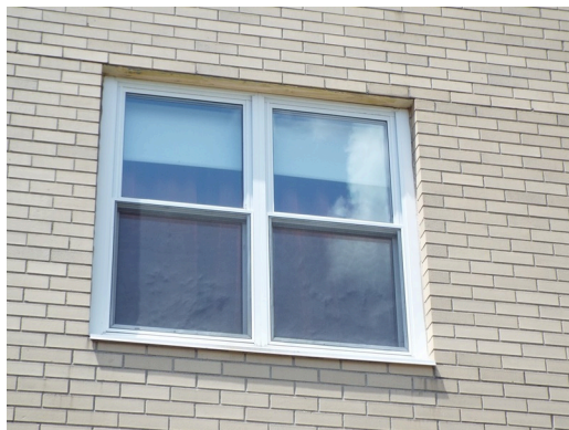
Typical windows - dwelling units
