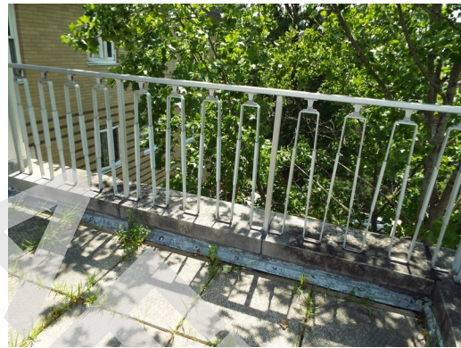
Rooftop terrace railing
