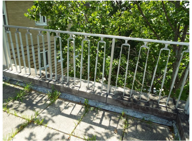
42. Rooftop terrace railing
