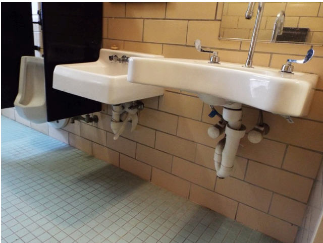
143. Common area - restroom
