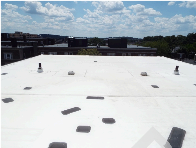
57. Roof overview (Non-Critical Repair)
