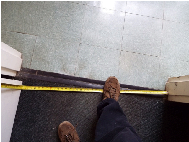
127. Common area - community room
