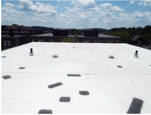
Roof overview (Non-Critical Repair)
