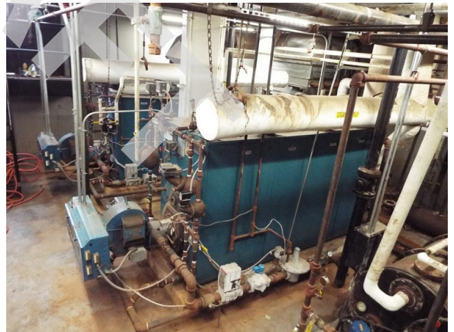
64. Heating boilers
