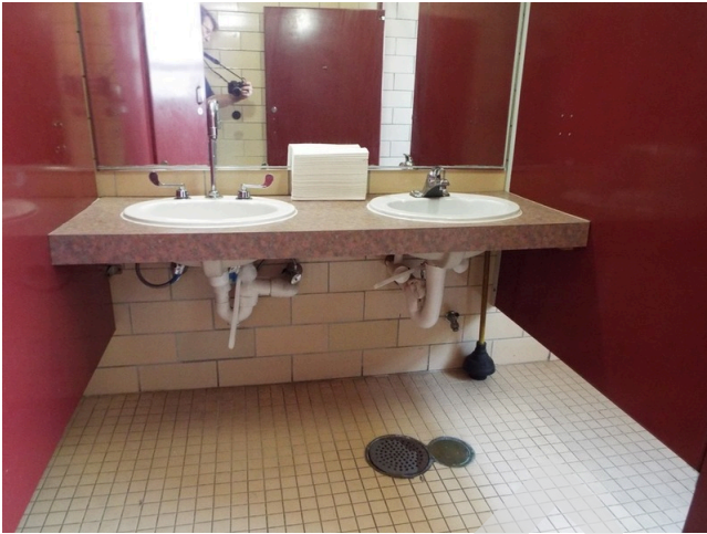
157. Common area - restroom
