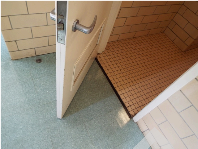
153. Common area - restroom
