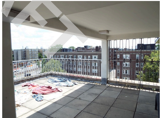
40. Rooftop terrace - 91 wing
