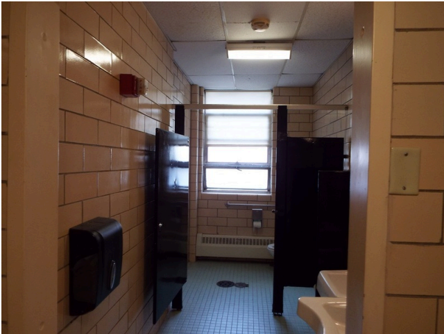
151. Common area - restroom
