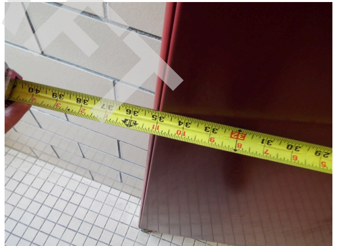
160. Common area - restroom
