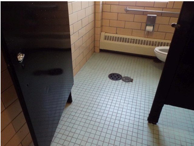
147. Common area - restroom
