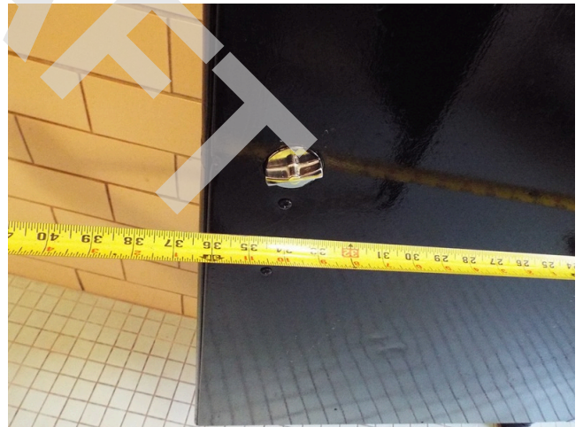
148. Common area - restroom
