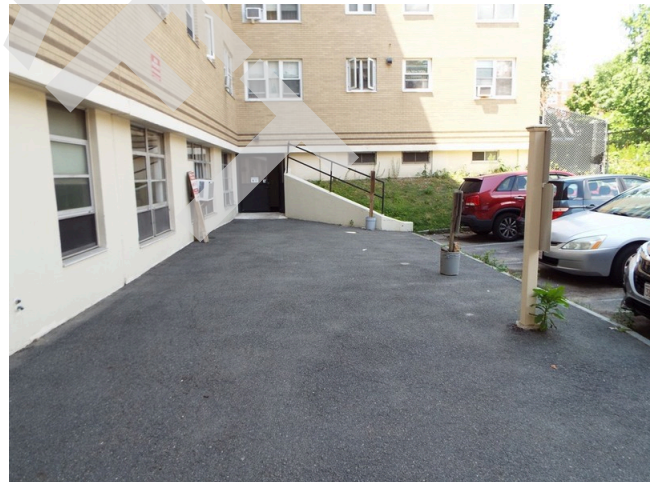
16. Rear entry asphalt pavement
