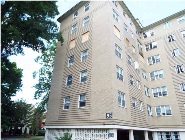
195. Exterior front, down unit windows seen covered by plywood
