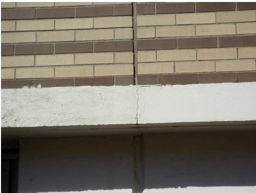
Sealant condition (Non-Critical Repair)
