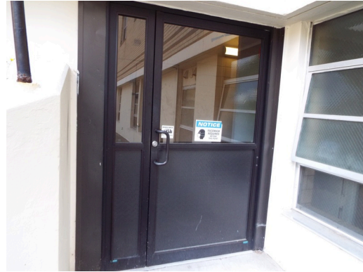
Rear entry door
