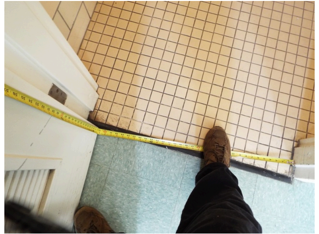
154. Common area - restroom
