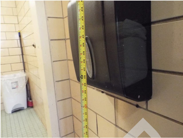
145. Common area - restroom
