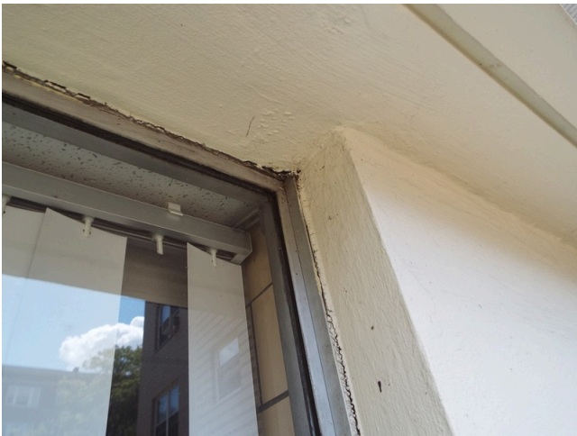
323. Typical windows - ground level
