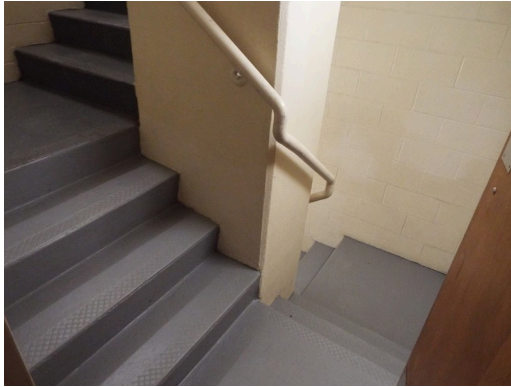
Interior exit stair
