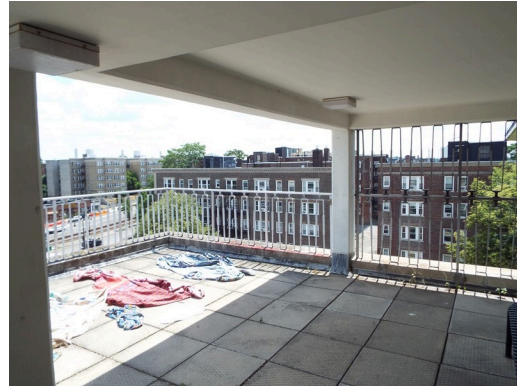
Rooftop terrace - 91 wing
