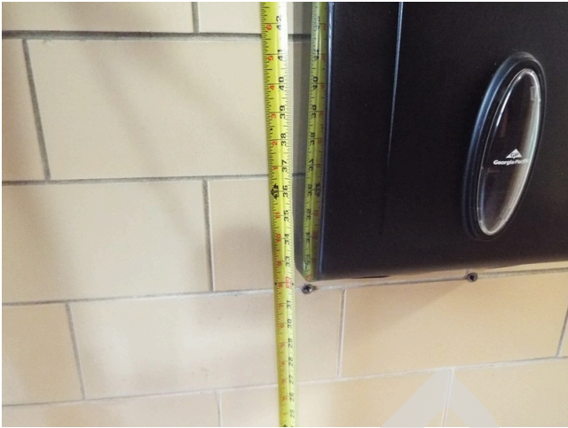
161. Common area - restroom
