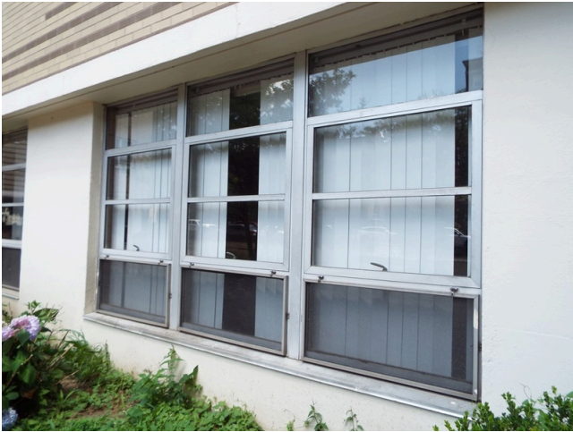
54. Typical windows - ground level
