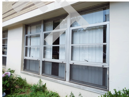
Typical windows - ground level
