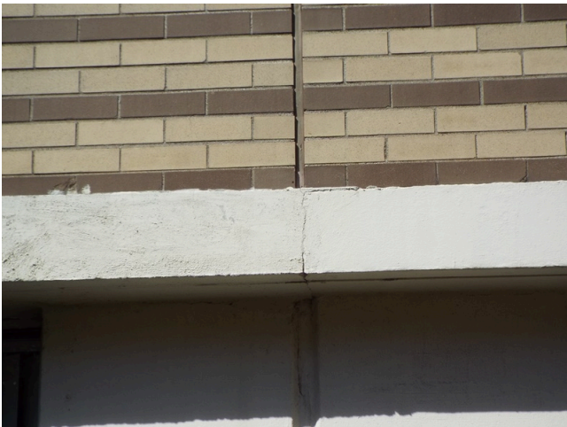
51. Sealant condition (Non-Critical Repair)
