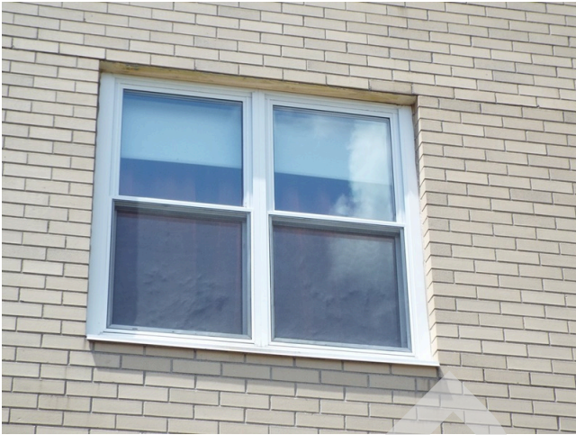
53. Typical windows - dwelling units
