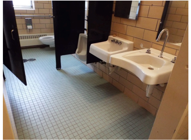
82. Common area - restroom
