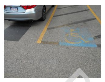
141. Handicap parking space marking in access aisle by removed handicap parking space (Critical Repair)
