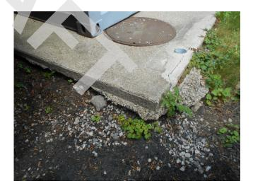
144. Concrete sidewalk along western side of building, erosion under sidewalk (Non-Critical Repair)
