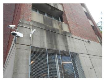
130. Rear façade, dirt buildup (Non-Critical Repair)
