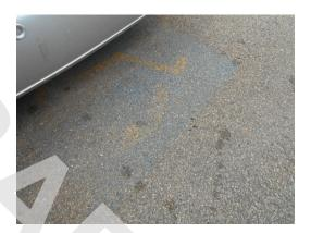
Handicap parking space, faded lines (Non-Critical Repair)
