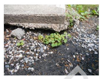
145. Concrete sidewalk along western side of building, erosion under sidewalk (Non-Critical Repair)
