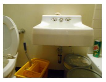
6. 0br/1ba, Unit 7 - Bathroom sink, no scald abrasion protection
