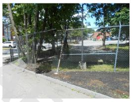
Chain link fencing, damaged (Non-Critical Repair)
