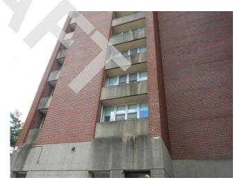
132. Rear façade, dirt buildup (Non-Critical Repair)
