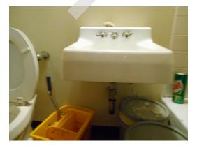
0br/1ba, Unit 7 - Bathroom sink, no scald abrasion protection
