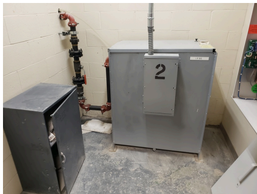
Elevator Machine Room
