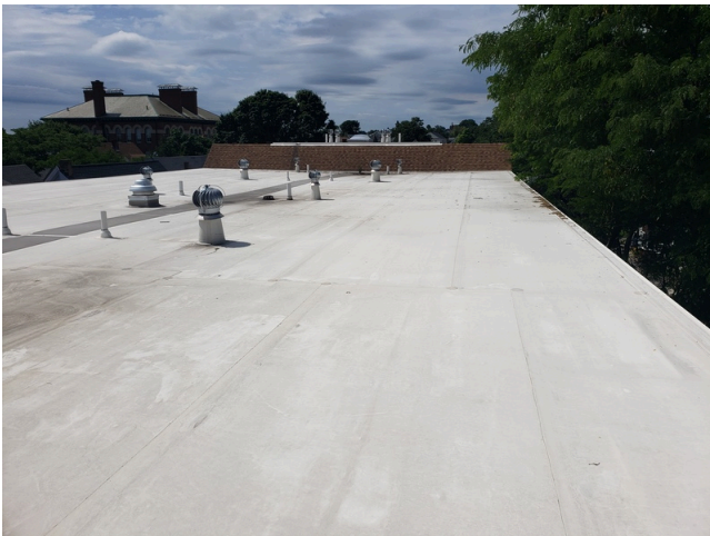
87. TPO Roofing (Low-Rise)
