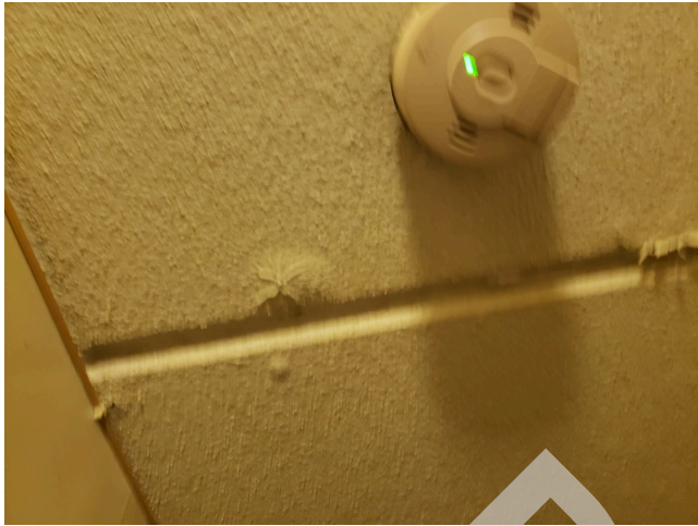
73. Hardwire Smoke Detector
