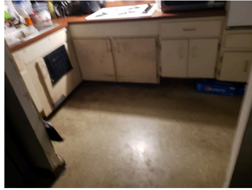
Unit 216- UFAS- 1bed/1bath- Kitchen- Replace Cabinets/Tops (Dwelling Units) (Older)(Non-Critical Repair)
