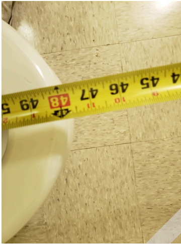
29. Unit 315- UFAS- 1bed/1bath- Bathroom- Clear Floor Space at WC
