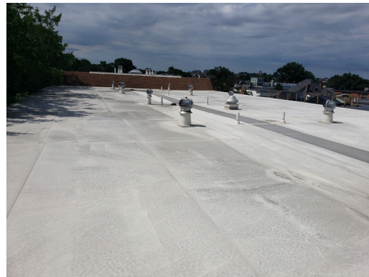
TPO Roofing (Low-Rise) and Asphalt Shingle Roofing
