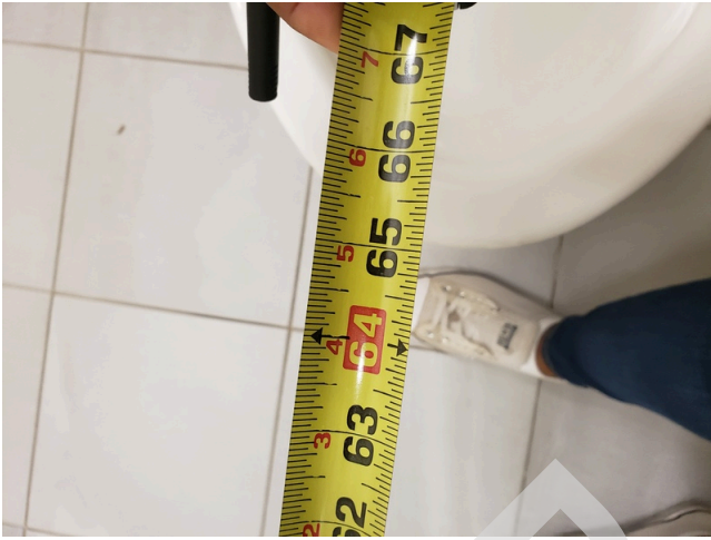
37. Common Area- Public Men's Restroom- Clear Floor Space at WC
