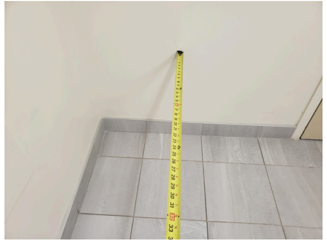
38. Common Area- Public Men's Restroom- Clear Floor Space at WC
