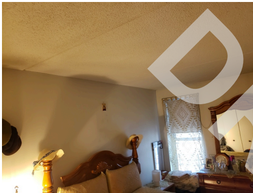
Unit 409- 1bed/1bath- Bedroom- Install Bedroom Smoke Detectors Per HUD (Critical Repair)
