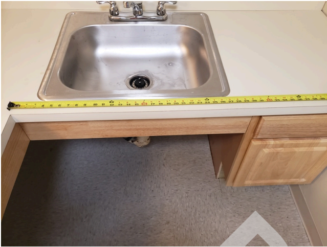
21. Unit 315- UFAS- 1bed/1bath- Kitchen- Clear Floor Space at Sink
