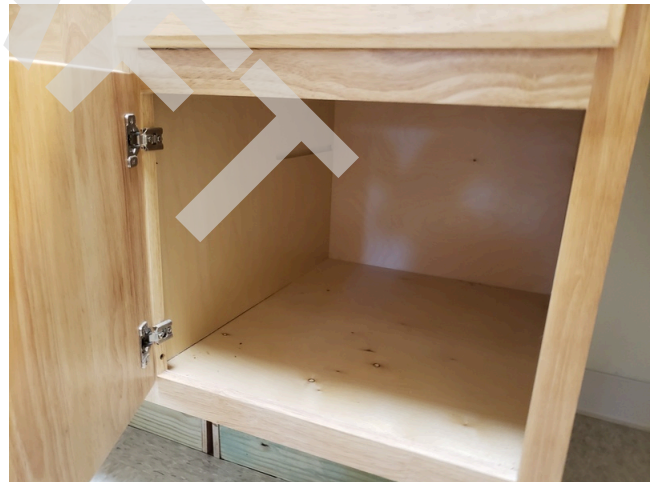
24. Unit 315- UFAS- 1bed/1bath- Kitchen- UFAS Unit Kitchen Cabinet Modifications (Critical Repair)
