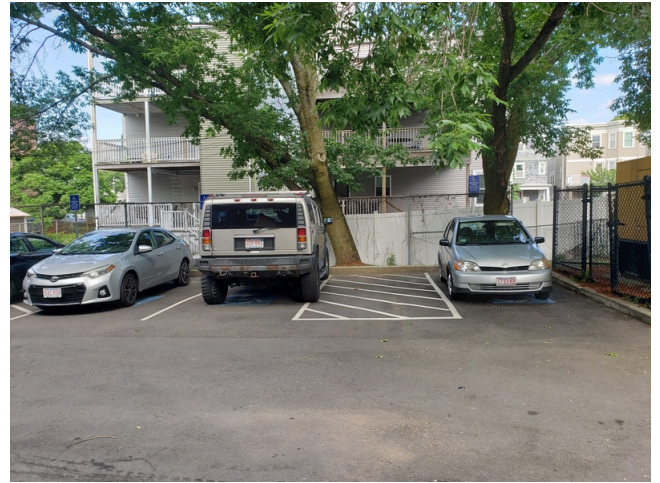
6. ADA Parking Lot- Install Van Accessible Parking Signage (Critical Repair)
