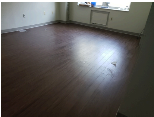
Unit 101-ANSI- 2bed/1bath- Bedroom- Install Audio / Visual Smoke Detectors (Critical Repair)
