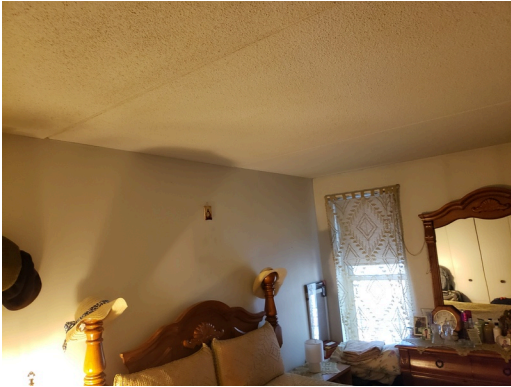
Unit 409- 1bed/1bath- Bedroom- Install Bedroom Smoke Detectors Per HUD (Critical Repair)
