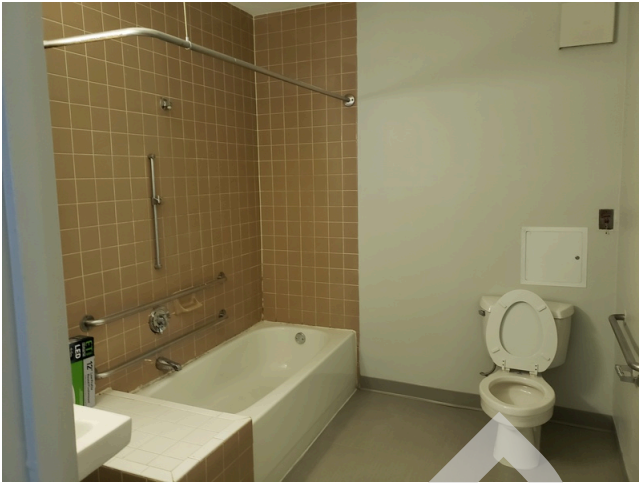
49. Unit 101-UFAS HDCP- 2bed/1bath- Bathroom
