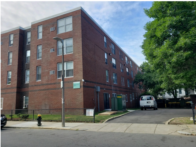
15. Northwestern Building Exterior
