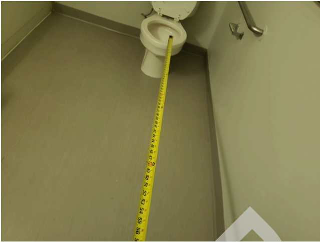
53. Unit 101-UFAS HDCP- 2bed/1bath- Bathroom- Clear Floor Space at WC
