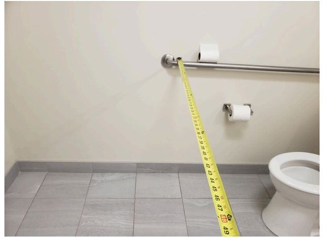
42. Common Area- Public Women's Restroom- Clear Floor Space
