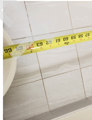
44. Common Area- Public Women's Restroom- Clear Floor Space at WC
