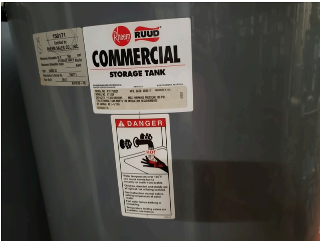
79. Water Storage Tank 115-Gallon
