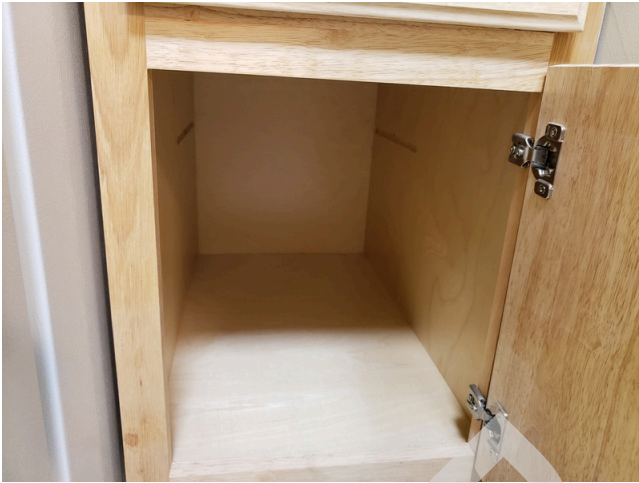
25. Unit 315- UFAS- 1bed/1bath- Kitchen- UFAS Unit Kitchen Cabinet Modifications (Critical Repair)
