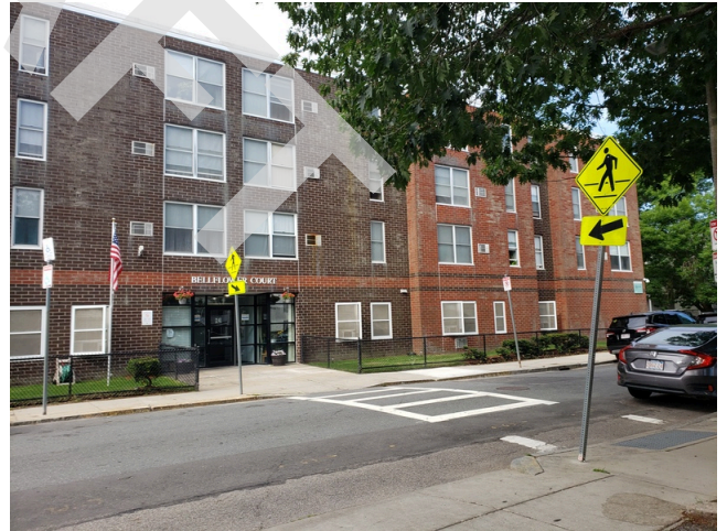
12. Crosswalk at Entry
