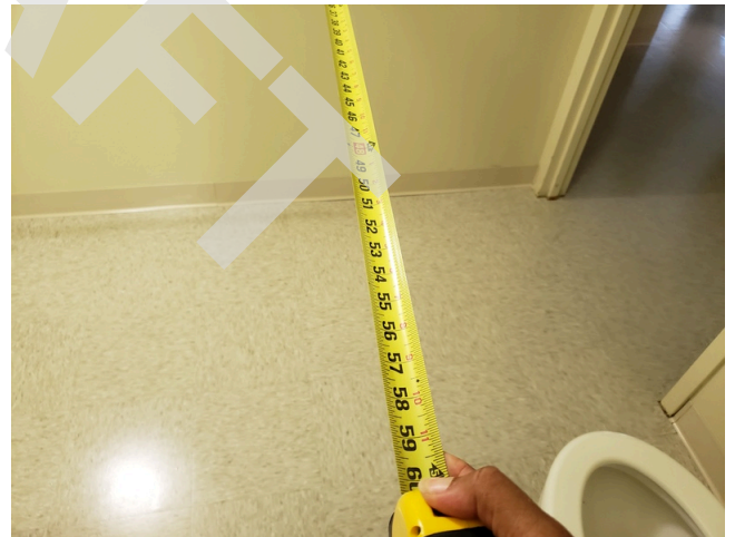
32. Unit 315- UFAS- 1bed/1bath- Bathroom- Clear Floor Space
