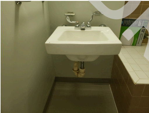
Unit 101-UFAS HDCP- 2bed/1bath- Bathroom- Install Scald and Abrasion Sink Wrap (Critical Repair)
