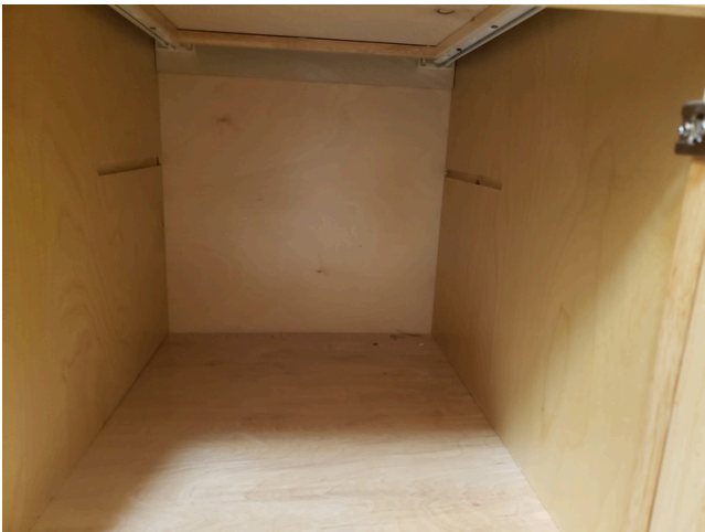
23. Unit 315- UFAS- 1bed/1bath- Kitchen- UFAS Unit Kitchen Cabinet Modifications (Critical Repair)
