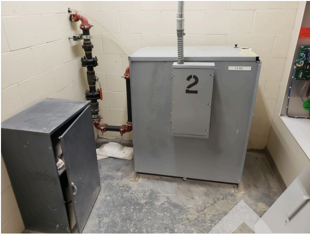
69. Elevator Machine Room
