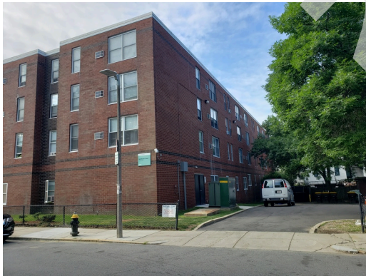
Northwestern Building Exterior
