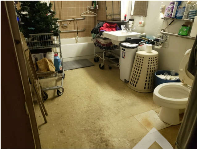
37. Unit 216- UFAS- 1bed/1bath- Replace Vinyl Flooring -1-Bed-Living Room, Kitchens and Baths (Dwelling Units) (Older) (Non-Critical Repair)
