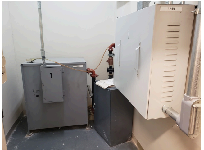
66. Elevator Machine Room 1
