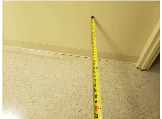
30. Unit 315- UFAS- 1bed/1bath- Bathroom- Clear Floor Space at WC
