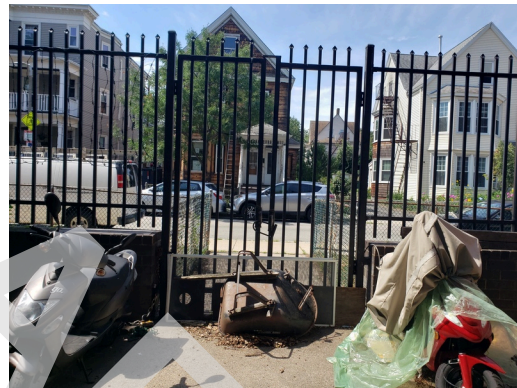
Courtyard Fencing- Gate Not Currently in Use
