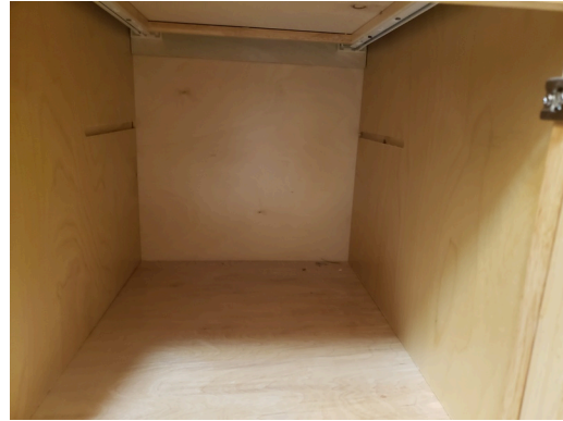
Unit 315- UFAS- 1bed/1bath- Kitchen- UFAS Unit Kitchen Cabinet Modifications (Critical Repair)
