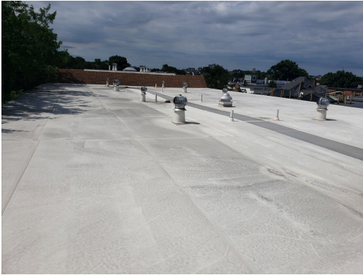
TPO Roofing (Low-Rise) and Asphalt Shingle Roofing
