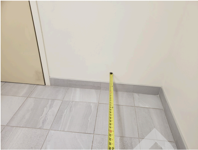
45. Common Area- Public Women's Restroom- Clear Floor Space at WC
