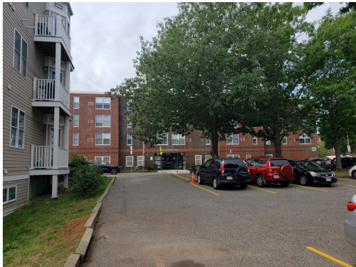
Parking Lot Entry
