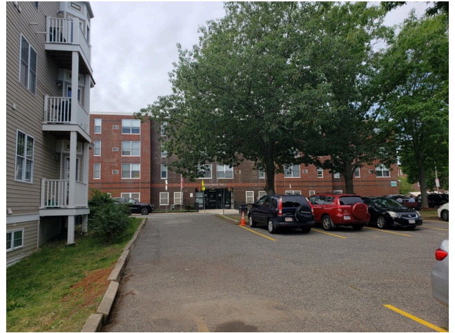
2. Parking Lot Entry
