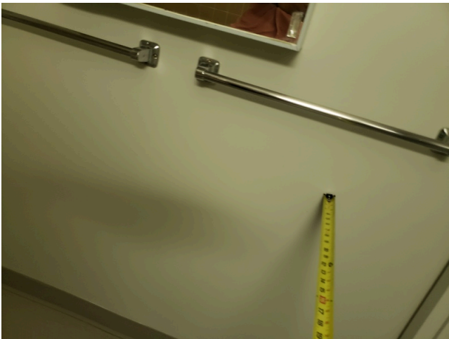
55. Unit 101-UFAS HDCP- 2bed/1bath- Bathroom- Clear Floor Space at WC
