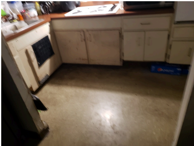
35. Unit 216- UFAS- 1bed/1bath- Kitchen- Replace Cabinets/Tops (Dwelling Units) (Older)(Non-Critical Repair)
