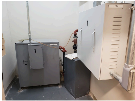
Elevator Machine Room 1
