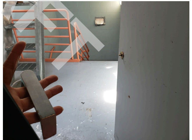
56. Repair Emergency Exit Door Hardware (Critical Repair)
