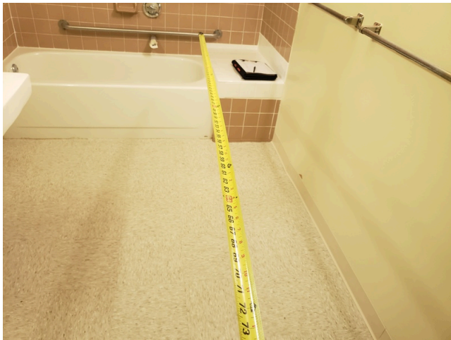
31. Unit 315- UFAS- 1bed/1bath- Bathroom- Clear Floor Space at Door
