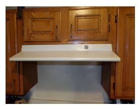
Building 4 - unit 422 - 3-bed/1.5-bath - UFAS - kitchen range hood missing front end controls (Critical Repair)
