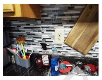
277. Building 12 - unit 1224 - 5-bed/2bath - TH - kitchen missing GFCI (Critical Repair)
