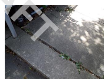
496. Building 13 - plaza area concrete stairs trip hazard (Critical Repair)
