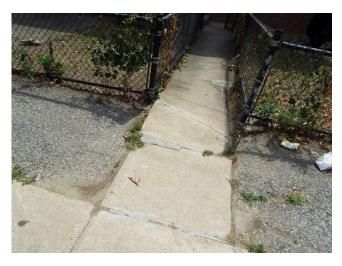
422. Building 10 - sidewalk trip hazard (Critical Repair)
