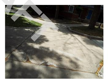
400. Building 8 - sidewalk trip hazard (Critical Repair)
