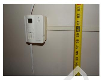
117. Building 4 - unit 415 - 3-bed/2-bath - TH - UFAS - thermostat to high (Critical Repair)
