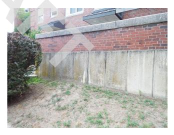
392. Building 8 - power wash foundation (Non-Critical Repair)
