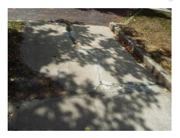
399. Building 8 - sidewalk trip hazard (Critical Repair)
