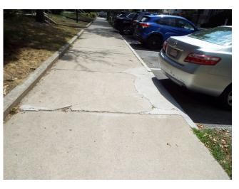
410. Building 9 - sidewalk trip hazard (Critical Repair)
