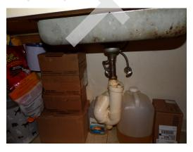
Building 4 - unit 432 - 4-bed/1.5-bath - UFAS - kitchen sink missing partial scald and abrasion protection (Critical Repair)
