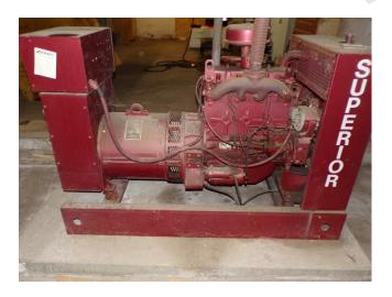
143. Building 4 - fire pump emergency generator not operational (Critical Repair)
