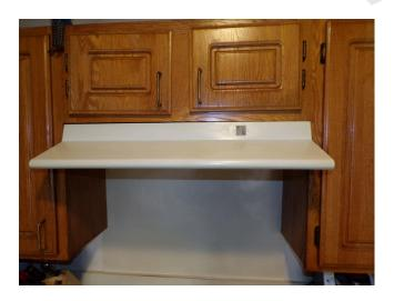
67. Building 4 - unit 422 - 3-bed/1.5-bath - UFAS - kitchen range hood missing front end controls (Critical Repair)
