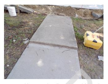
257. Building 5 - sidewalk trip hazard (Critical Repair)
