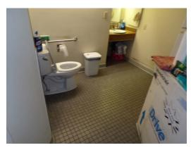
Building 4 - unit 414 - 3-bed/2-bath - TH - UFAS - bathroom missing rear grab bar (Critical Repair)
