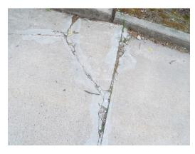
Building 8 - sidewalk trip hazard (Critical Repair)
