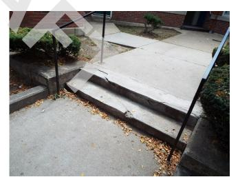
448. Building 12 - concrete steps trip hazard (Critical Repair)
