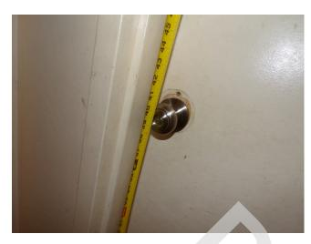
49. Building 4 - unit 412 - 3-bed/1.5-bath - UFAS - non-levered door hardware (Critical Repair)
