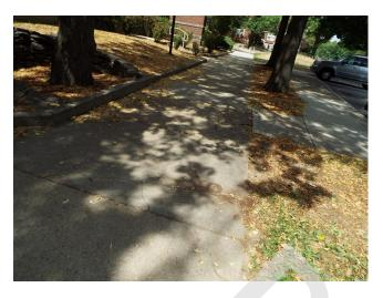
457. Building 12 - sidewalk trip hazards (Critical Repair)
