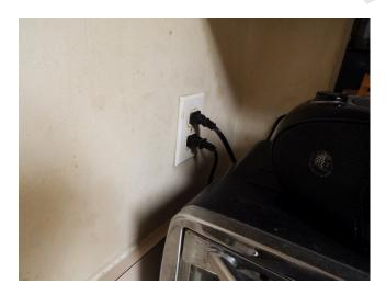
259. Building 11 - unit 1104 - 4-bed/2-bath - TH - unit 1104 - kitchen missing GFCI (Critical Repair)
