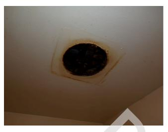
241. Building 8 - unit 822 - 2-bed/1.5-bath - TH - kitchen ventilation missing (Non-Critical Repair)
