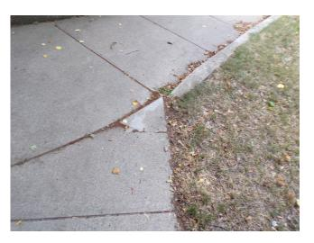
246. Building 5 - sidewalk trip hazard (Critical Repair)
