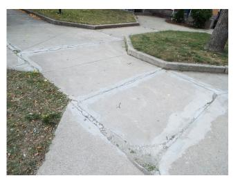
390. Building 8 - sidewalk trip hazard (Critical Repair)
