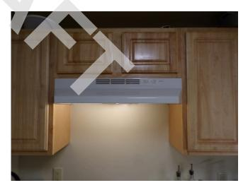
144. Building 4 - unit 437 - 4-bed/1.5-bath - UFAS - kitchen range hood missing front end controls (Critical Repair)
