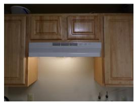
Building 4 - unit 437 - 4-bed/1.5-bath - UFAS - kitchen range hood missing front end controls (Critical Repair)
