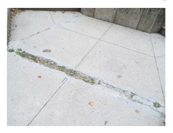
459. Building 12 - sidewalk trip hazard (Critical Repair)
