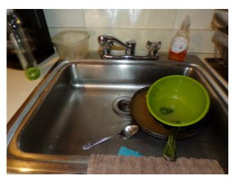
66. Building 4 - unit 422 - 3-bed/1.5-bath - UFAS - kitchen sink missing levered hardware (Critical Repair)
