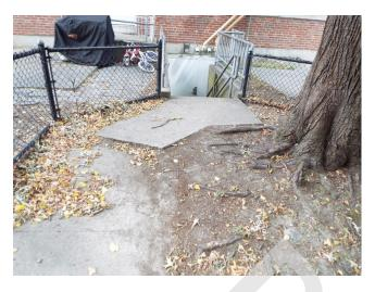
429. Building 10 - sidewalk trip hazard (Critical Repair)
