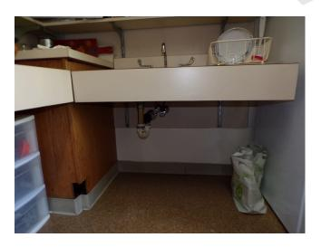
219. Building 7 - unit 731 - 2-bed/1-bath - UFAS - kitchen sink missing scald and abrasion protection (Critical Repair)
