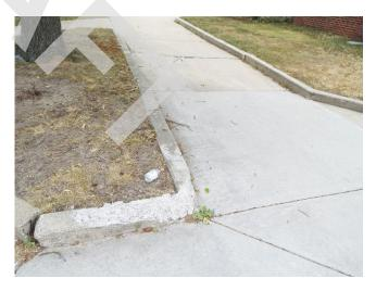
388. Building 8 - curb damage (Non-Critical Repair)
