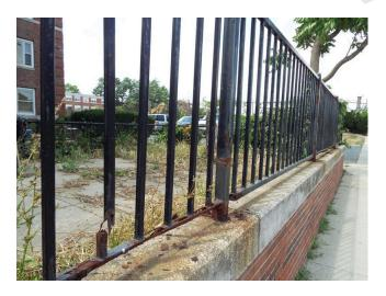
435. Building 11 - fence damage (Non-Critical Repair)
