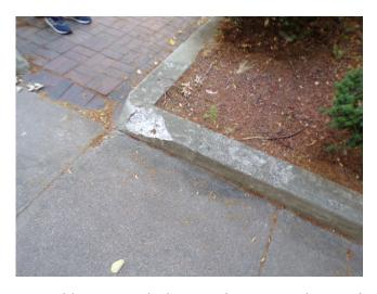
46. Building 4 - curb damage (Non-Critical Repair)
