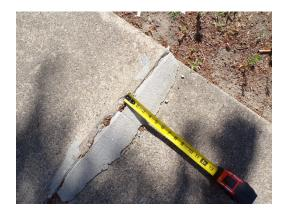
Building 4 - sidewalk trip hazard (Critical Repair)
