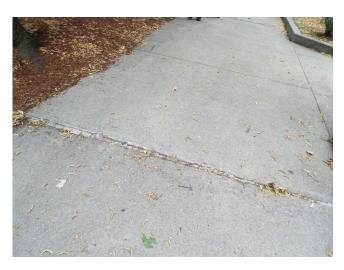
454. Building 12 - sidewalk trip hazard (Critical Repair)
