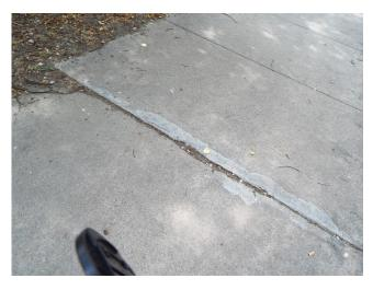
398. Building 8 - sidewalk trip hazard (Critical Repair)
