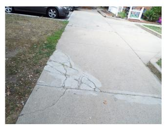
402. Building 9 - sidewalk trip hazard (Critical Repair)
