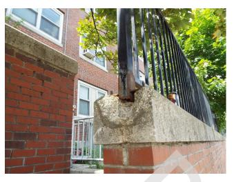
441. Building 11 - retaining wall damage by fence (Non-Critical Repair)
