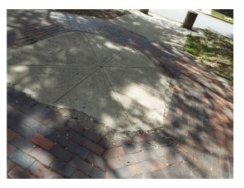
418. Building 9 - sidewalk trip hazard (Critical Repair)
