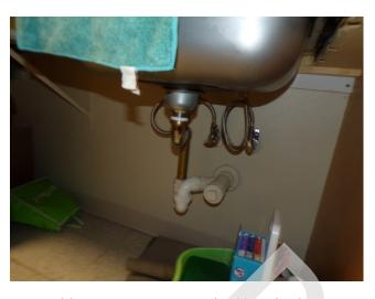
153. Building 4 - unit 417 - 3-bed/1.5-bath - UFAS - kitchen sink missing scald and abrasion protection (Critical Repair)
