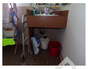
221. Building 7 - unit 731 - 2-bed/1-bath - UFAS - bathroom sink missing scald and abrasion protection (Critical Repair)
