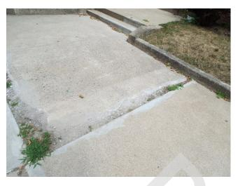
413. Building 9 - sidewalk trip hazard (Critical Repair)
