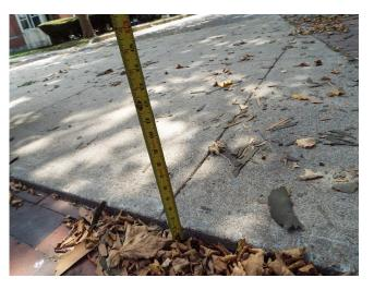
470. Building 13 - sidewalk trip hazard (Critical Repair)
