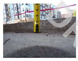
Building 5 - sidewalk trip hazard (Critical Repair)
