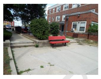
501. Building 10 and 11 - plaza access concrete stairs trip hazard (Critical Repair)
