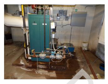
233. Community building - boiler, leak (Critical Repair)
