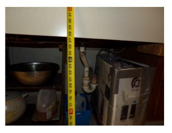
122. Building 4 - unit 415 - 3-bed/2-bath - TH - UFAS - kitchen sink missing scald and abrasion protection (Critical Repair)
