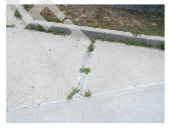
428. Building 10 - sidewalk trip hazard (Critical Repair)
