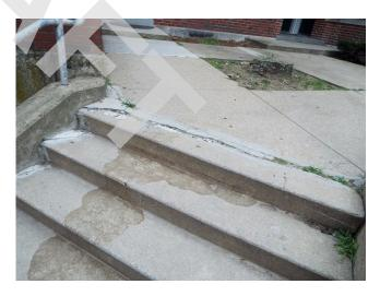
460. Building 12 - concrete stair trip hazard (Critical Repair)
