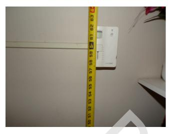
29. Building 4 - unit 414 - 3-bed/2-bath - TH - UFAS - lower thermostat (Critical Repair)
