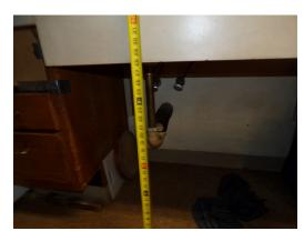
Building 4 - unit 414 - 3-bed/2-bath - TH - UFAS - kitchen sink pipes missing scald and abrasion protection (Critical Repair)
