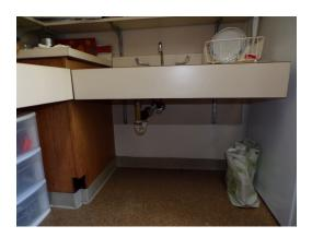
Building 7 - unit 731 - 2-bed/1-bath - UFAS - kitchen sink missing scald and abrasion protection (Critical Repair)
