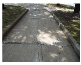
Building 9 - sidewalk trip hazard (Critical Repair)
