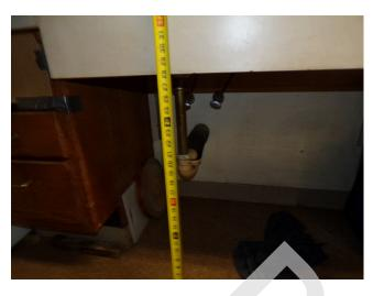
9. Building 4 - unit 414 - 3-bed/2-bath - TH - UFAS - 10. Building 4 - unit 414 - 3-bed/2-bath - TH - UFAS kitchen sink pipes missing scald and abrasion protection (Critical Repair)
