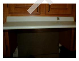
Building 4 - unit 427 - 3-bed/1.5-bath - UFAS - kitchen range hood missing front end controls (Critical Repair)
