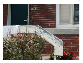
455. Building 12 - peeling paint on hand rail (Non-Critical Repair)
