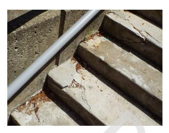
485. Building 13 - concrete stairs trip hazard (Critical Repair)
