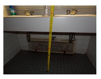
210. Community building - men's restroom missing scald and abrasion protection and levered sink hardware (Critical Repair)
