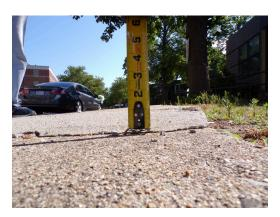
Building 4 - sidewalk trip hazard (Critical Repair)
