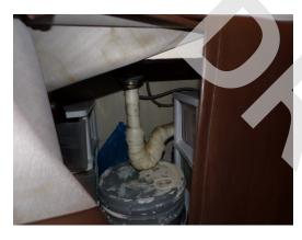
Building 7 - unit 735 - 2-bed/1-bath - UFAS - kitchen sink missing scald and abrasion protection (Critical Repair)
