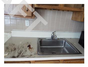
256. Building 11 - unit 1110 - 2-bed/1-bath - TH - kitchen missing GFCI (Critical Repair)
