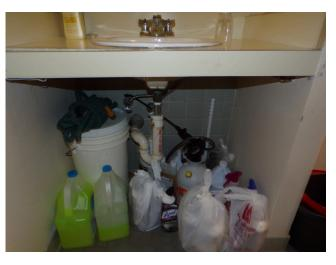
130. Building 4 - unit 415 - 3-bed/2-bath - TH - UFAS - bathroom sink missing scald and abrasion protection (Critical Repair)
