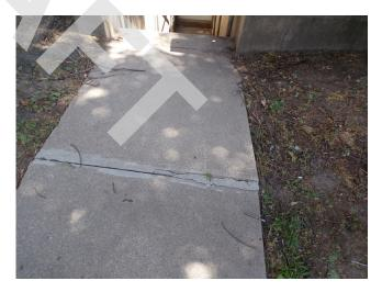
256. Building 5 - sidewalk trip hazard (Critical Repair)
