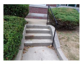
318. Building 7 - stairs missing railing (Critical Repair)
