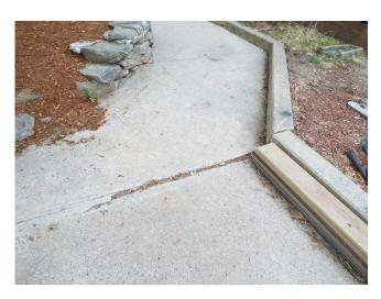
414. Building 9 - sidewalk trip hazard (Critical Repair)
