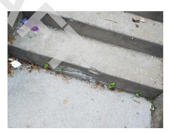
484. Building 13 - concrete stairs damaged (Critical Repair)
