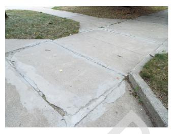
397. Building 8 - sidewalk trip hazard (Critical Repair)
