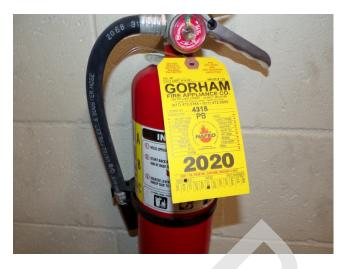
141. Building 4 - elevator room fire extinguisher expired (Non-Critical Repair)
