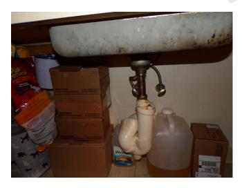
107. Building 4 - unit 432 - 4-bed/1.5-bath - UFAS - kitchen sink missing partial scald and abrasion protection (Critical Repair)
