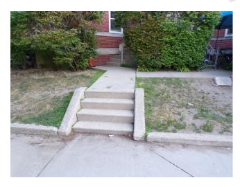
39. Building 4 - concrete stairs missing railing (Critical Repair)
