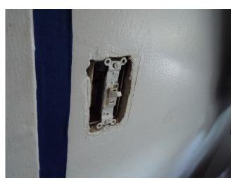
278. Building 12 - unit 1224 - 5-bed/2bath - TH - bathroom on second floor missing switch plate (Critical Repair)
