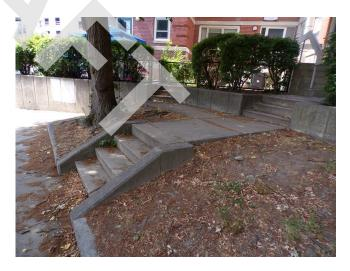
252. Building 5 - stairs missing railings (Critical Repair)
