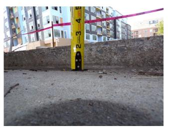
258. Building 5 - sidewalk trip hazard (Critical Repair)
