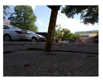
314. Building 7 - sidewalk trip hazard (Critical Repair)
