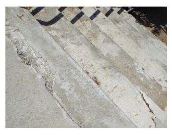
466. Building 13 - concrete stairs trip hazard (Critical Repair)
