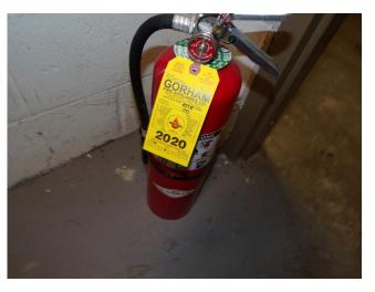
302. Building 7 - elevator room fire extinguisher expired (Non-Critical Repair)
