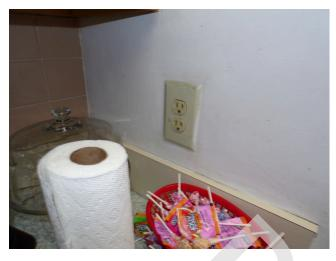
61. Building 4 - unit 418 - 3-bed/1.5-bath - TH - kitchen missing GFCI (Critical Repair)
