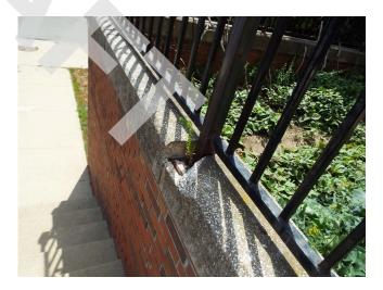
440. Building 11 - retaining wall damage (Non-Critical Repair)
