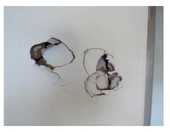
258. Building 11 - unit 1110 - 2-bed/1-bath -TH - living room wall damage (Non-Critical Repair)
