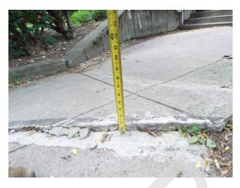
469. Building 13 - sidewalk trip hazard (Critical Repair)
