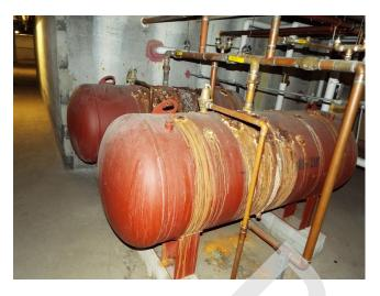
369. Building 11 - hot water storage tank corrosion (Non-Critical Repair)
