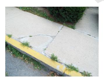
443. Building 11 - sidewalk trip hazard (Critical Repair)
