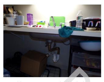
145. Building 4 - unit 437 - 4-bed/1.5-bath - UFAS kitchen sink missing scald and abrasion protection (Critical Repair)
