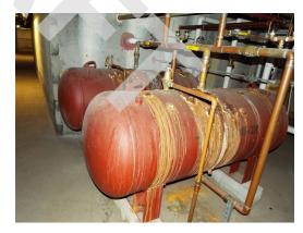
Building 11 - hot water storage tank corrosion (Non-Critical Repair)
