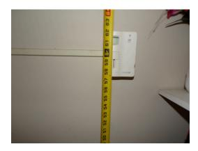
Building 4 - unit 414 - 3-bed/2-bath - TH - UFAS - lower thermostat (Critical Repair)
