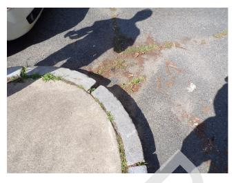
13. Building 4 - curb damage trip hazard (Critical Repair))
