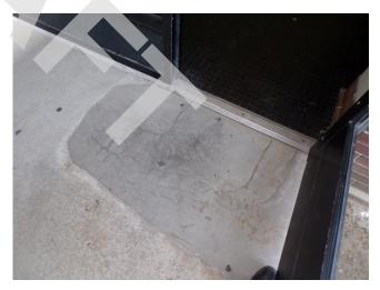
324. Building 7 - concrete ramp trip hazard (Critical Repair)
