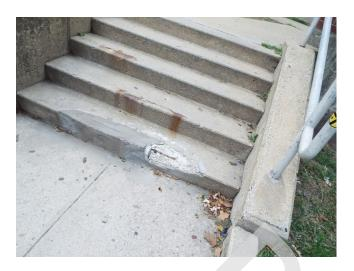
449. Building 12 - concrete steps trip hazard (Critical Repair)
