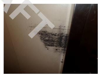
336. Building 7 - elevator cab door rubbing (Non-Critical Repair)
