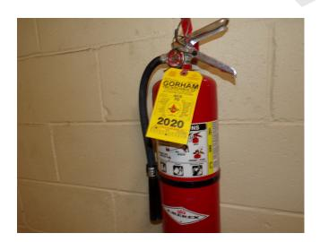
343. Building 7 - elevator room fire extinguisher expired (Non-Critical Repair)
