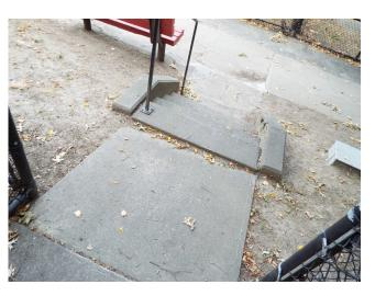
406. Building 9 - sidewalk trip hazard (Critical Repair)
