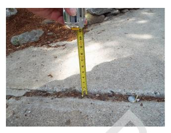
405. Building 9 - sidewalk trip hazard (Critical Repair)
