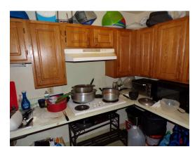
Building 4 - unit 412 - 3-bed/1.5-bath - UFAS - kitchen range hood missing front end controls (Critical Repair)
