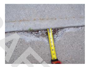
Building 4 - concrete trip hazard (Critical Repair)
