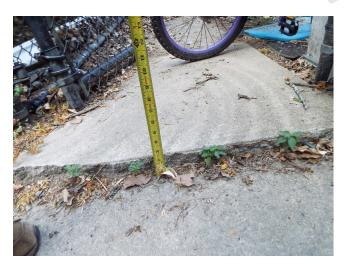
447. Building 12 - sidewalk trip hazard (Critical Repair)
