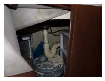
198. Building 7 - unit 735 - 2-bed/1-bath - UFAS - kitchen sink missing scald and abrasion protection (Critical Repair)
