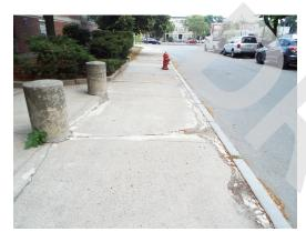
Building 10 - sidewalk trip hazard (Critical Repair)
