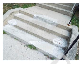
465. Building 13 - concrete stair trip hazard and missing railing (Critical Repair)
