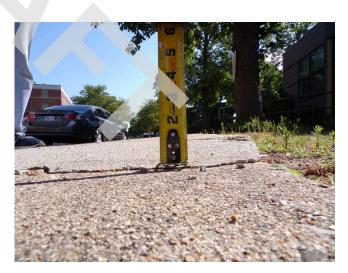
12. Building 4 - sidewalk trip hazard (Critical Repair)
