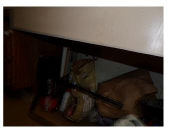
186. Building 5 - unit 515 - 3-bed/1.5-bath - TH - UFAS - kitchen sink missing scald and abrasion protection (Critical Repair)
