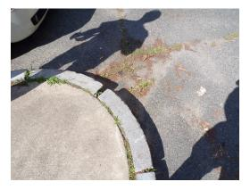
Building 4 - curb damage trip hazard (Critical Repair))
