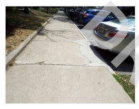
Building 9 - sidewalk trip hazard (Critical Repair)
