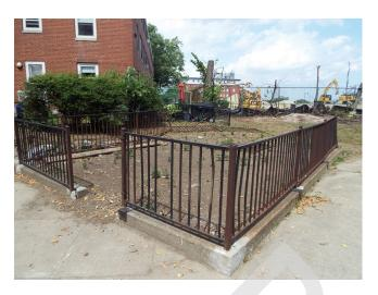
425. Building 10 - iron fence damage and bare ground (Non-Critical Repair)
