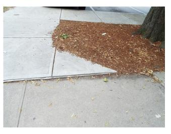
446. Building 12 - sidewalk trip hazard (Critical Repair)
