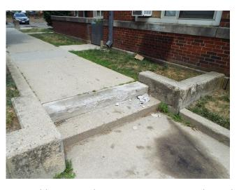
434. Building 10 and 11 - concrete step trip hazard (Critical Repair)
