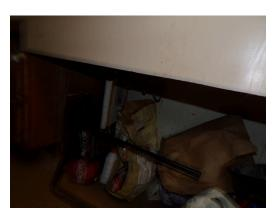
Building 5 - unit 515 - 3-bed/1.5-bath - TH - UFAS - kitchen sink missing scald and abrasion protection (Critical Repair)
