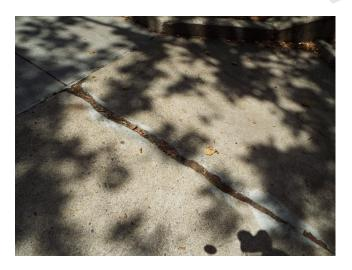
411. Building 9 - sidewalk trip hazard (Critical Repair)
