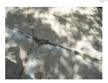
415. Building 9 - sidewalk trip hazard (Critical Repair)
