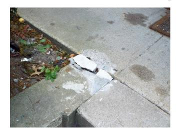
483. Building 13 - concrete stairs trip hazard (Critical Repair)
