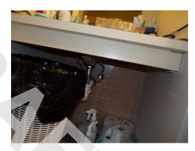
Apartment building 1 - Apartment 114 - 2-bed/1-bath - UFAS unit - bathroom sink missing scald and abrasion protection (Critical Repair)
