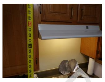
53. Apartment building 1 - Apartment 135 - 2-bed/ 1-bath - UFAS unit - Range hood not front end controls and upper cabinets over 48 inches (Critical Repair)
