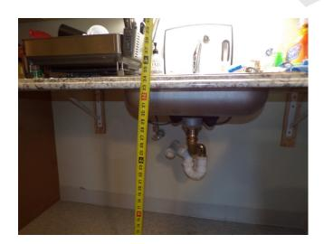
75. Apartment building 1 - Apartment 125 - 2-bed/ 1-bath - UFAS unit - kitchen sink missing scald and abrasion protection (Critical Repair)
