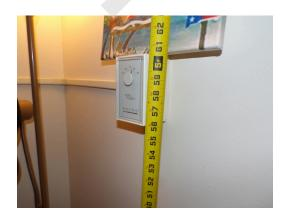
Apartment building 1 - Apartment 111 - 1-bed/1-bath - UFAS unit - heat control thermostat over 48 inches (Critical Repair)
