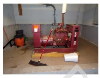
109. Apartment buildings 1 and 2 inoperable fire sprinkler system generator (Critical Repair)
