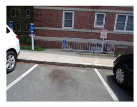
Apartment building 1 handicap parking signage less than 60 inches above ground (Critical Repair)
