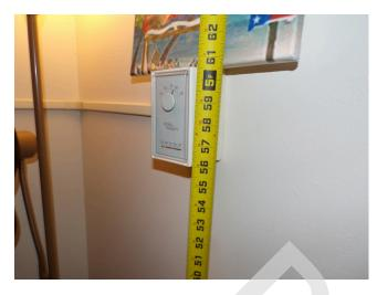
113. Apartment building 1 - Apartment 111 - 1-bed/ 1-bath - UFAS unit - heat control thermostat over 48 inches (Critical Repair)
