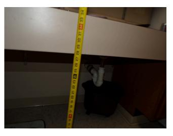
122. Apartment building 2 - Apartment 212 - 1-bed/ 1-bath - UFAS unit - kitchen sink missing scald and abrasion protection (Critical Repair)
