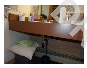
Apartment building 2 - Apartment 212 - 1-bed/1-bath - UFAS unit - bathroom sink missing scald and abrasion protection (Critical Repair)
