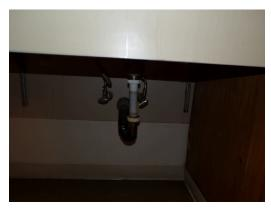
Apartment building 1 - Apartment 111 - 1-bed/1-bath - UFAS unit - kitchen sink missing scald and abrasion protection (Critical Repair)
