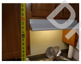
Apartment building 1 - Apartment 135 -2-bed/1-bath - UFAS unit - Range hood not front end controls and upper cabinets over 48 inches (Critical Repair)
