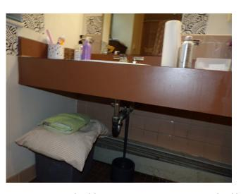
130. Apartment building 2 - Apartment 212 - 1-bed/ 1-bath - UFAS unit - bathroom sink missing scald and abrasion protection (Critical Repair)
