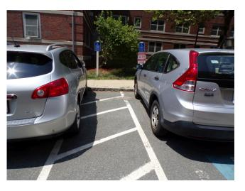
30. Apartment building 1 handicap parking signage and missing curb cutout (Critical Repair)
