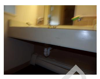
117. Apartment building 1 - Apartment 111 - 1-bed/1-bath - UFAS unit - bathroom sink missing scald and abrasion protection (Critical Repair)
