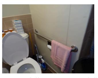
102. Apartment building 1 - Apartment 114 - 2-bed/1-bath - UFAS unit - bathroom toilet missing rear toilet grab bar (Critical Repair)
