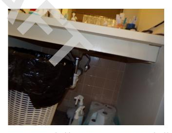
100. Apartment building 1 - Apartment 114 - 2-bed/1-bath - UFAS unit - bathroom sink missing scald and abrasion protection (Critical Repair)
