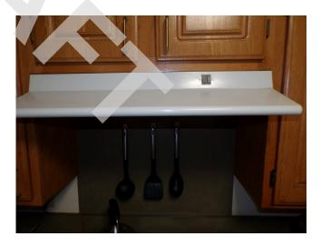
188. Apartment building 2 - Apartment 214 - 2-bed/1-bath - UFAS unit - Range hood missing front end controls and over 48 inches (Critical Repair)
