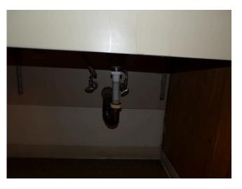
110. Apartment building 1 - Apartment 111 - 1-bed/ 1-bath - UFAS unit - kitchen sink missing scald and abrasion protection (Critical Repair)
