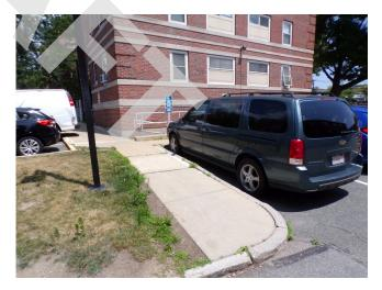
16. Apartment building 1 parking lot handicap parking missing curb cutout (Critical Repair)
