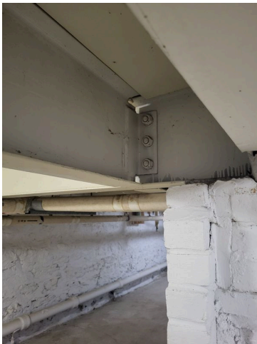
123. Basement support beam
