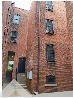
Court yard ingress/egress door and stairs
