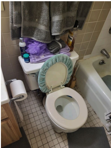
43. Apartment 56-3 bathroom toilet
