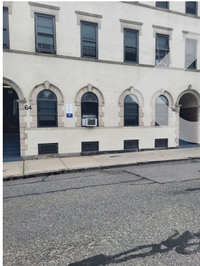
Window-mounted air conditioning, window screens and basement windows
