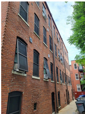
East elevation windows
