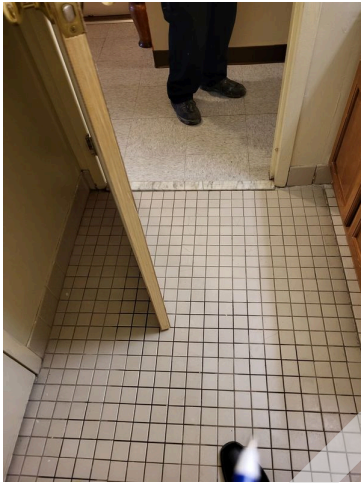
93. Apartment 52-3 bathroom ceramic tile flooring
