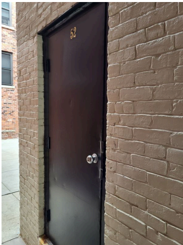
55. Exterior door ingress/egress
