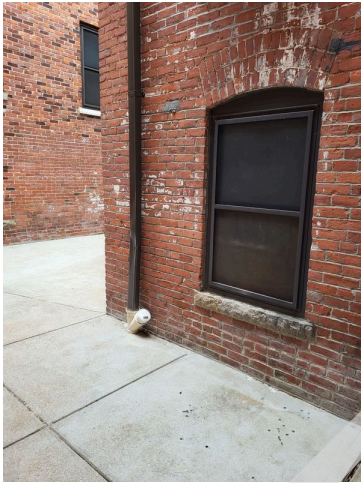
57. Building downspout and drainage
