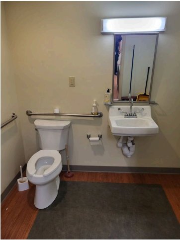
90. Community room restroom toilet, grab bars and sink
