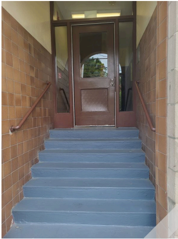
41. Building ingress/egress painted ingress/egress stairs, handrails and door hardware
