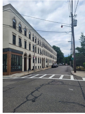
Pole electric transformer
