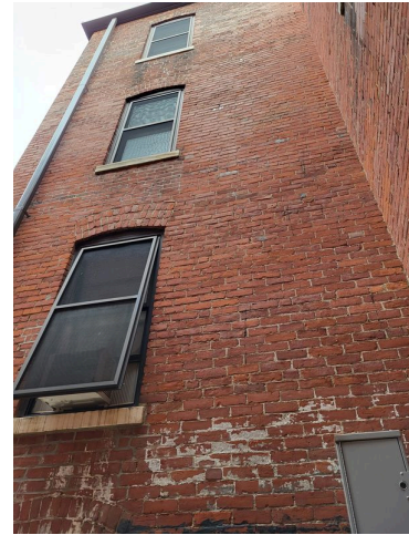
58. Southeast elevation brick façade
