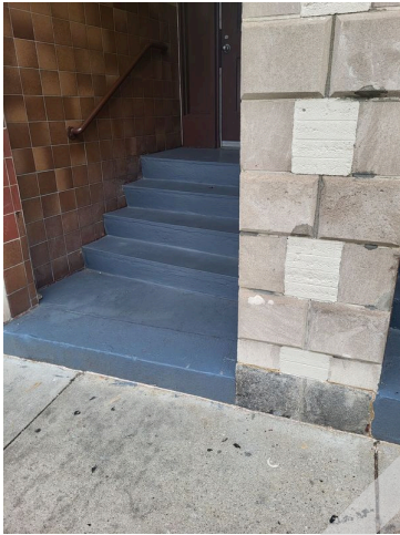
45. Building ingress/egress painted concrete stairs
