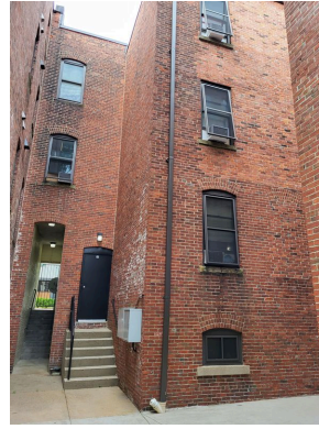
Court yard ingress/egress door and stairs
