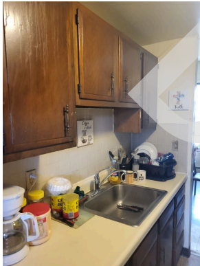
Apartment 56-3 kitchen cabinets, countertop and sink
