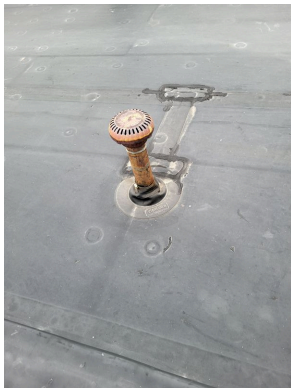
Roof ventilation and flashing
