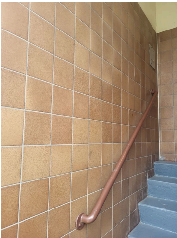
23. Building ingress/egress stairs railing and intercom
