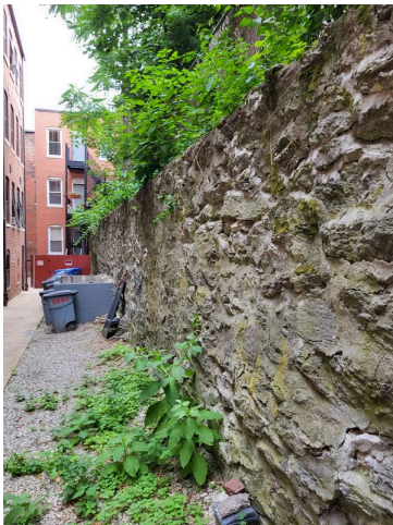
67. East elevation retaining wall and alley wood fence ingress/egress
