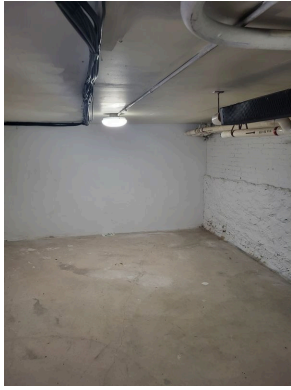
Basement light fixture
