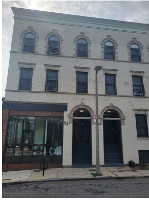
West elevation pole light
