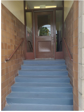
Building ingress/egress painted ingress/egress stairs, handrails and door hardware
