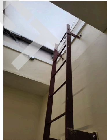
4. Building roof ingress/egress roof hatch
