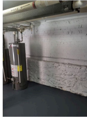
Basement concrete and brick wall
