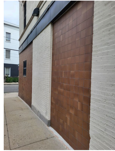
50. South elevation façade painted brick and ceramic tile
