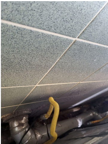
95. Laundry room acoustical ceiling tile
