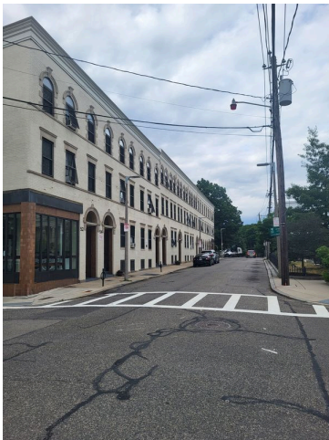
15. Pole electric transformer
