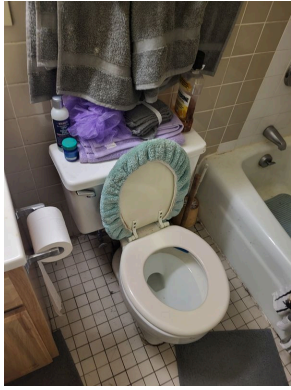
Apartment 56-3 bathroom toilet
