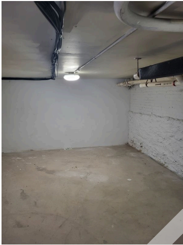
117. Basement light fixture
