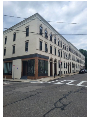
West elevation painted brick façade
