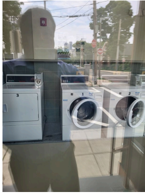
Common area laundry room leased front end loader washers and dryers
