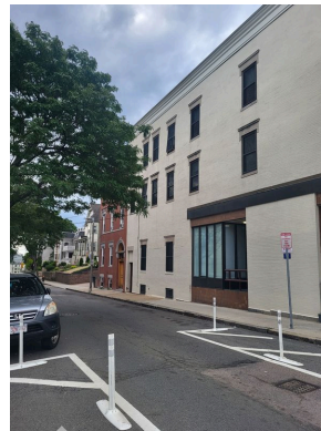
North elevation painted brick façade
