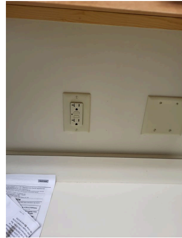
86. Community room kitchen area GFCI
