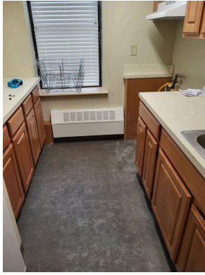
Community room kitchen area flooring, cabinets, countertops, range hood and hydronic baseboard
