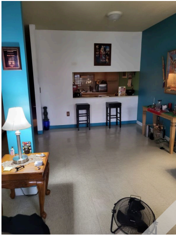
61. Apartment 58-3 living room area light fixture and vinyl tile flooring
