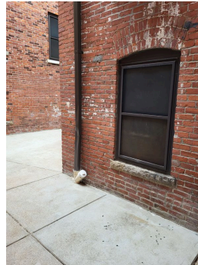
Building downspout and drainage
