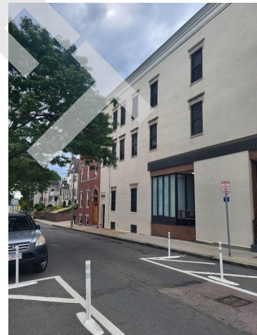
12. North elevation painted brick façade
