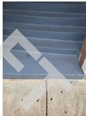
Building ingress/egress painted concrete stairs
