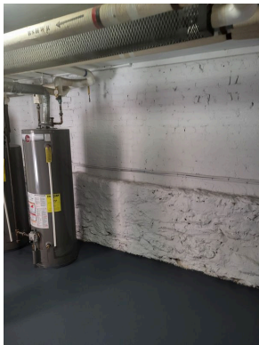
Basement concrete and brick wall
