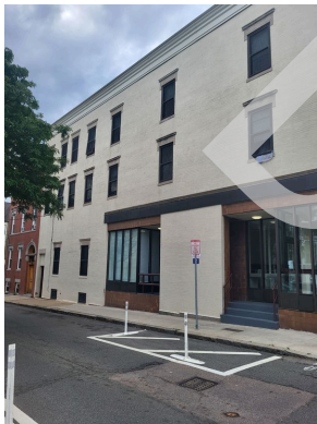
North elevation painted brick façade
