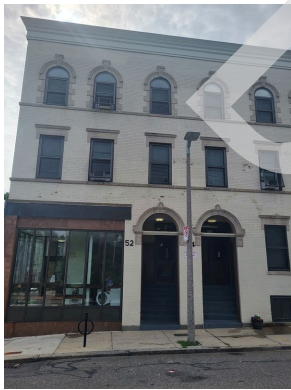
West elevation pole light
