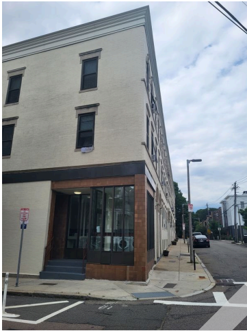
13. North elevation painted brick façade and common area ingress/egress
