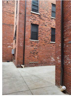
Building downspout and drainage
