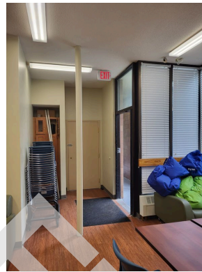
Community room and kitchen area emergency exit sign and emergency lighting
