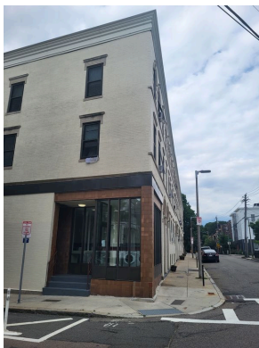
North elevation painted brick façade and common area ingress/egress
