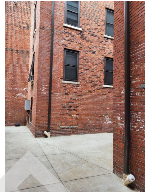
Building downspout and drainage
