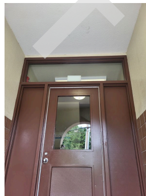
Building ingress/egress door
