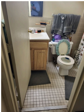
Apartment 56-3 bathroom vanity, sink, toilet and flooring
