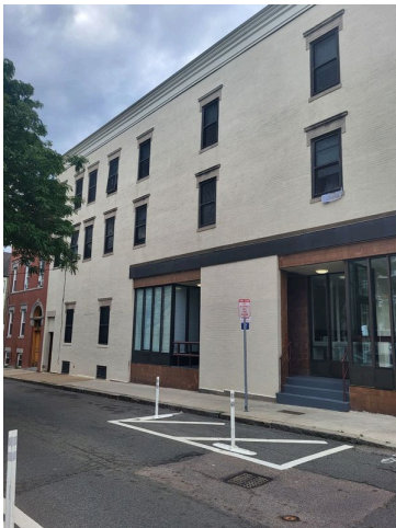
11. North elevation painted brick façade
