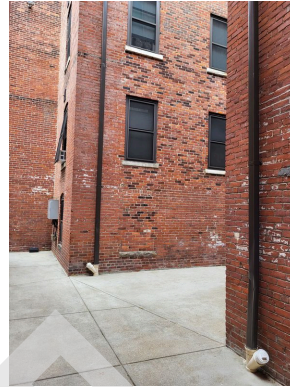
Building downspout and drainage
