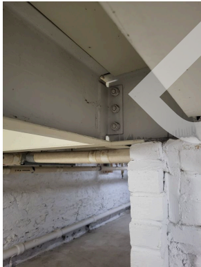
Basement support beam
