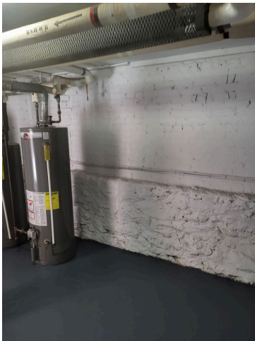
99. Basement concrete and brick wall
