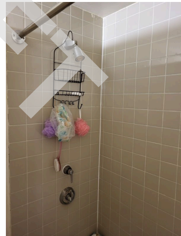
100. Apartment 52-3 bathroom bathtub hardware
