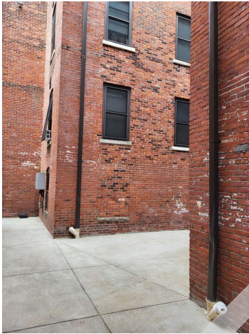
61. Building downspout and drainage
