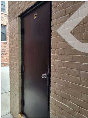
Exterior door ingress/egress
