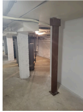
Basement support columns
