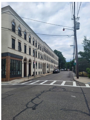
Pole electric transformer
