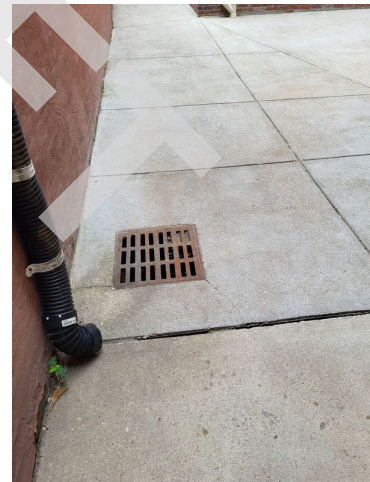
56. Building downspout and drainage
