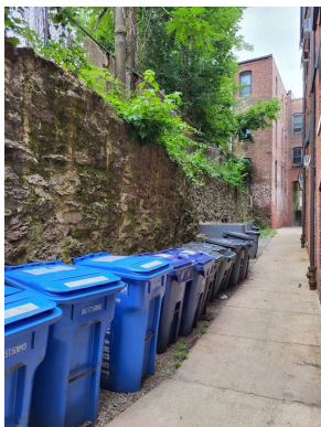
East elevation trash containers
