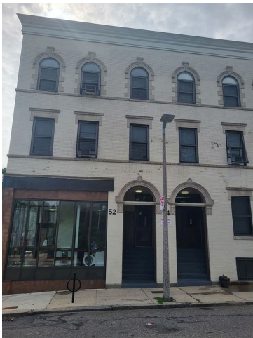
35. West elevation pole light
