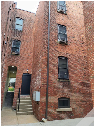
65. Court yard ingress/egress door and stairs
