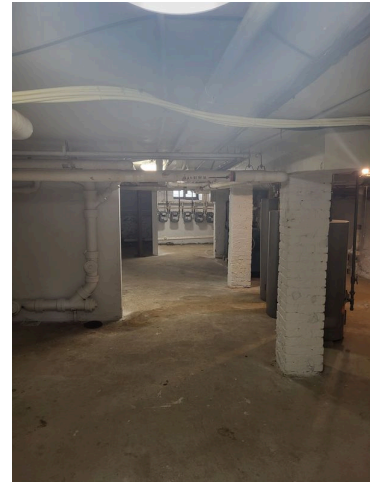
118. Basement support columns
