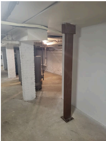
119. Basement support columns
