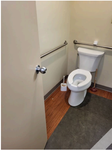
89. Community room restroom door hardware
