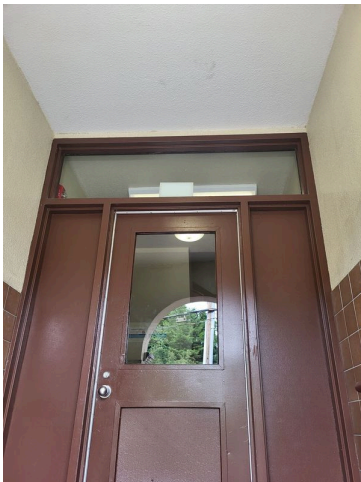
39. Building ingress/egress door
