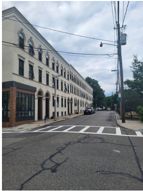
Pole electric transformer
