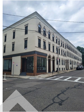
West elevation painted brick façade
