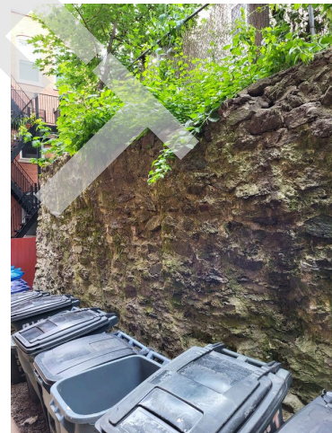
64. East elevation stone retaining wall
