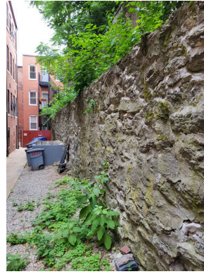
East elevation retaining wall and alley wood fence ingress/egress
