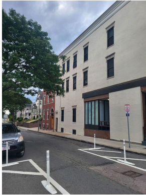
North elevation painted brick façade
