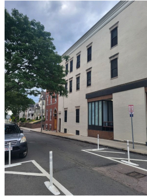
North elevation painted brick façade
