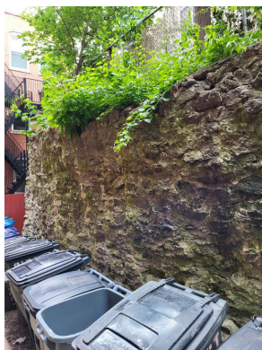
East elevation stone retaining wall
