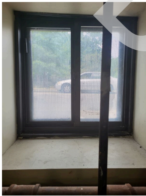
Basement concrete window sill and small window
