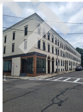
West elevation painted brick façade
