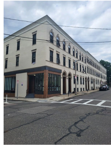
14. West elevation painted brick façade
