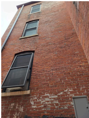
Southeast elevation brick façade
