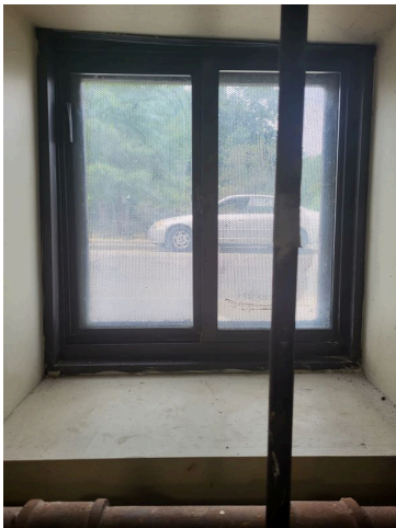
107. Basement concrete window sill and small window
