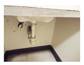
Bathroom sink lacks pipe protection - UFAS - unit 213 (Critical Repair)
