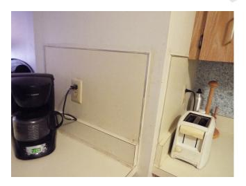
335. 1-bed-1-bath - unit 514 - kitchen lacks GFCI receptacle (Critical Repair)
