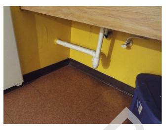
25. Kitchen sink lacks pipe protection - UFAS - unit 211 (Critical Repair)
