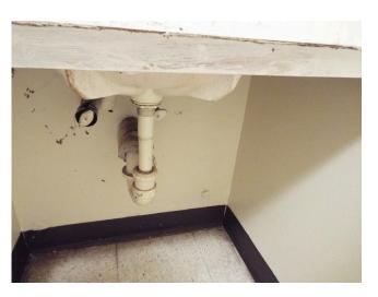
86. Bathroom sink lacks pipe protection - UFAS - unit 213 (Critical Repair)
