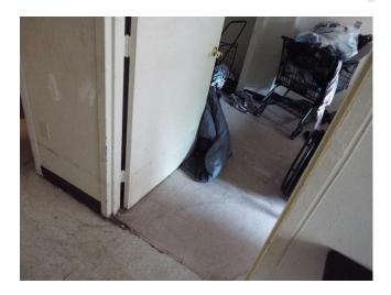
91. Doors lack lever hardware - UFAS - unit 213 (Critical Repair)
