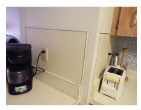
1-bed-1-bath - unit 514 - kitchen lacks GFCI receptacle (Critical Repair)
