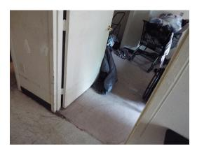
Doors lack lever hardware - UFAS - unit 213 (Critical Repair)
