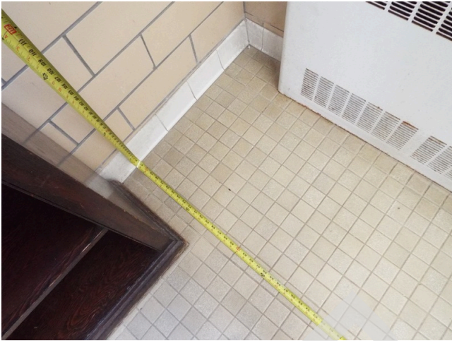
217. Common area - building 12 - women's restroom
