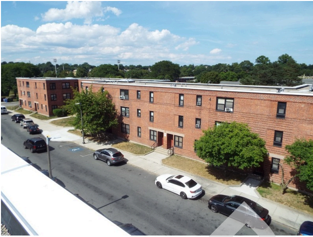
17. Typical asphalt street paving - Stratton Street Extension
