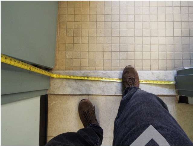
213. Common area - building 12 - women's restroom
