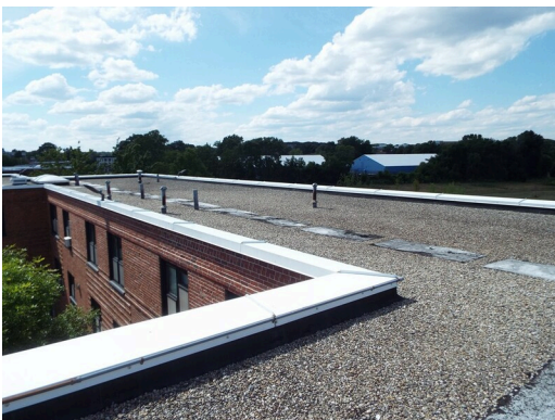
Roof overview - building 14
