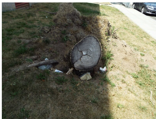
Hole at stump - building 4 (Critical Repair)
