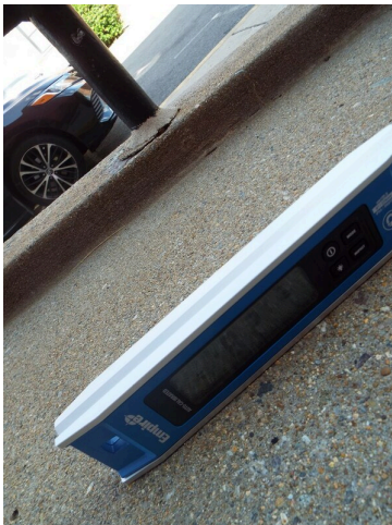
199. Ramp - Ames Way - building 6
