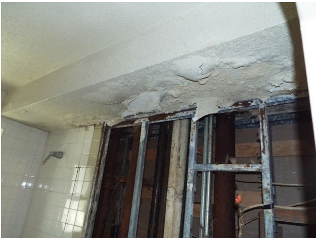
107. 2-bed-1-bath- unit 230A - building 1 - bathroom ceiling repairs (Non-Critical Repair)
