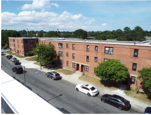
Typical asphalt street paving - Stratton Street Extension
