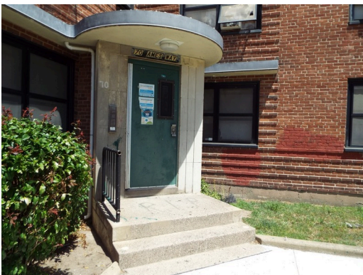
Typical building entry steps
