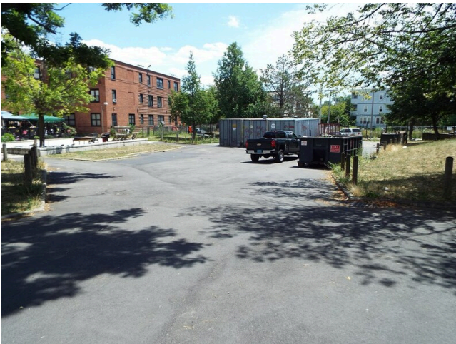
23. Asphalt paving - rear building 12
