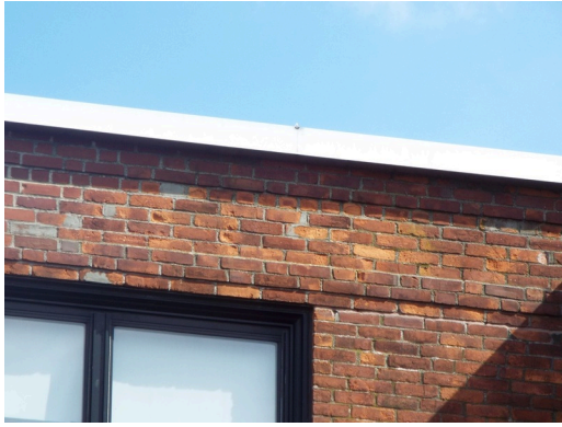
Brick masonry condition - building 17 (Non-Critical Repair)
