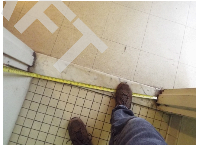
244. 3-bed-1-bath-UFAS - unit 13 - building 4
