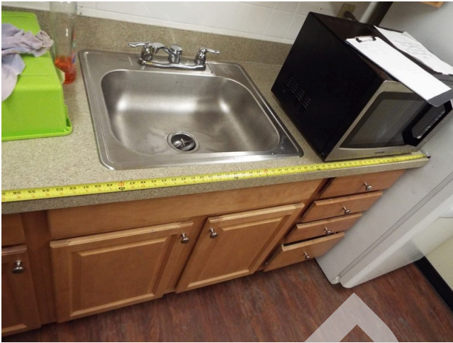
241. Common area - building 18 - teen center - kitchen
