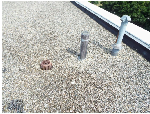
Roof penetrations - building 14
