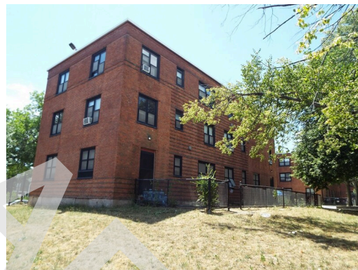
Typical elevation - side - building 11
