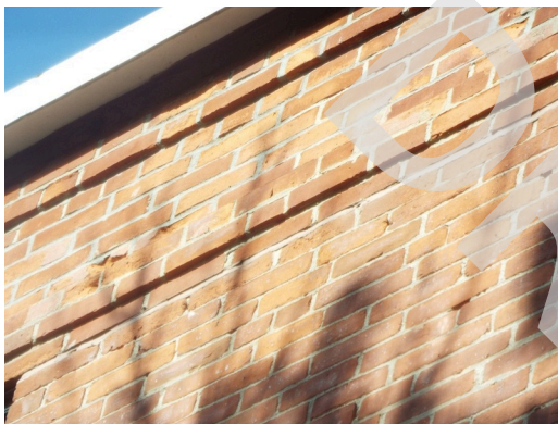
Brick masonry condition - building 6 (Non-Critical Repair)
