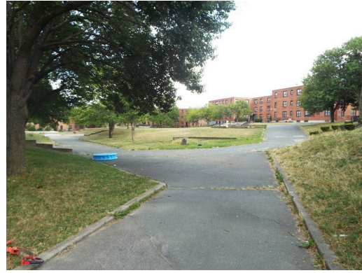
Asphalt paving - buildings 14 thru 19 (Non-Critical Repair)
