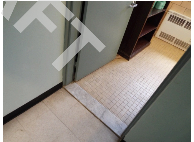
212. Common area - building 12 - women's restroom
