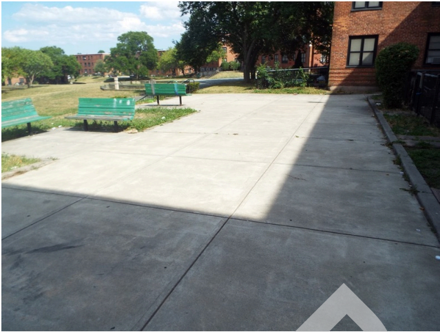
89. Concrete terrace seating area - building 17 rear
