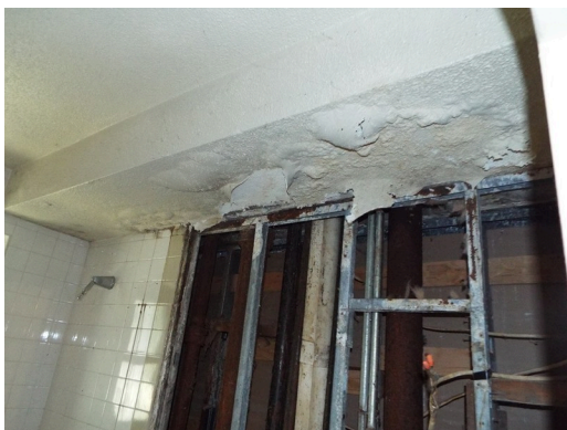
2-bed-1-bath- unit 230A - building 1 - bathroom ceiling repairs (Non-Critical Repair)
