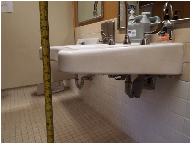
251. Common area - building 18 - teen center - women's restroom
