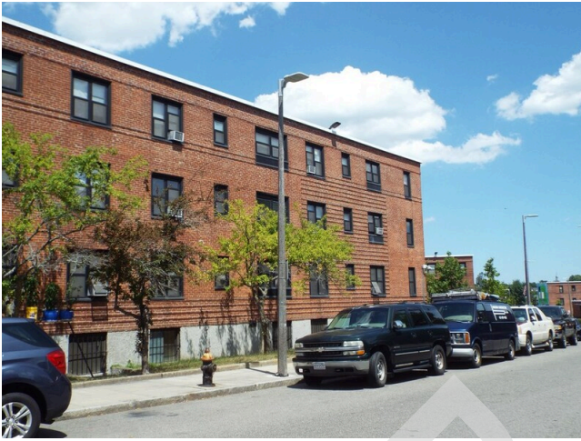
197. Municipal pole mounted lighting
