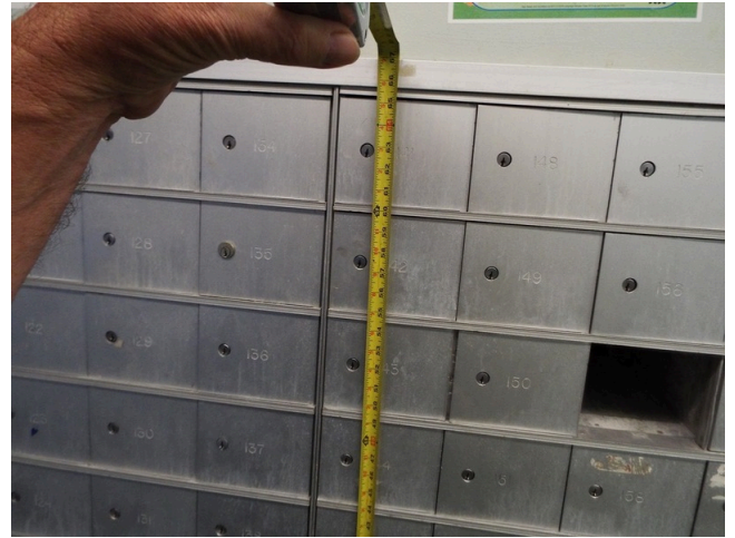
206. Common area - building 12 - mailboxes
