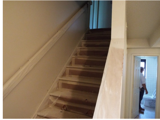
4-bed-2-bath-TH - unit 50A - building 5 - stair
