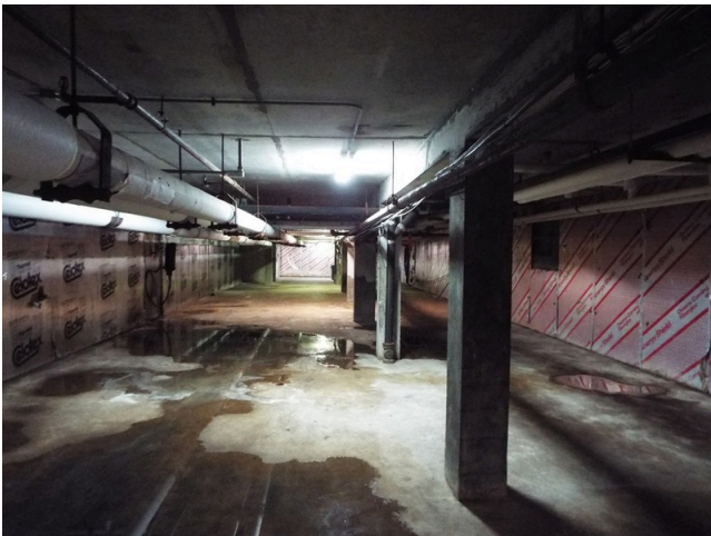
79. Framing - basement - building 17
