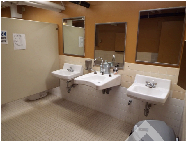
177. Common area - building 18 - teen center - women's restroom
