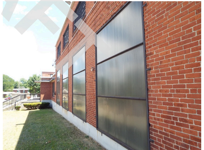
124. Steel framed fixed windows - building 12
