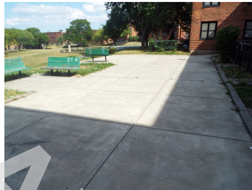
Concrete terrace seating area - building 17 rear
