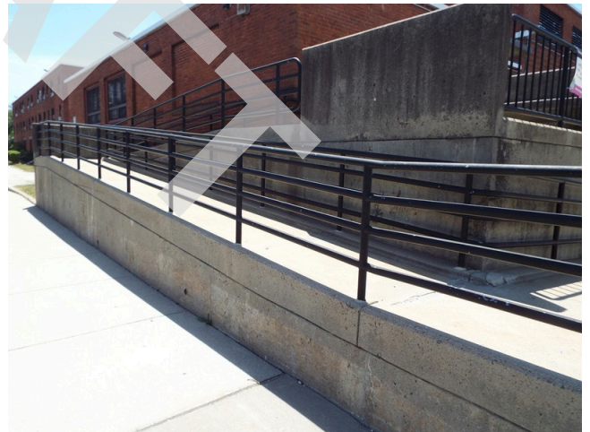
200. Ramp access - building 12 leasing office
