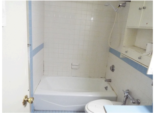
34. 1-bed-1-bath - unit 90D - building 19 - tub shower
