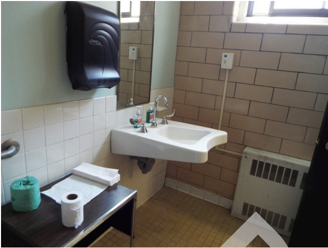
209. Common area - building 12 - men's restroom
