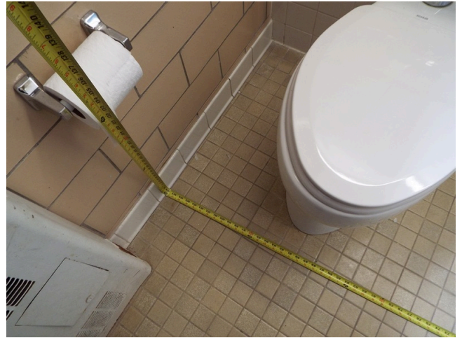
218. Common area - building 12 - women's restroom
