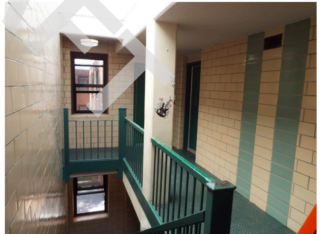
180. Typical upper level stair hall - building 7
