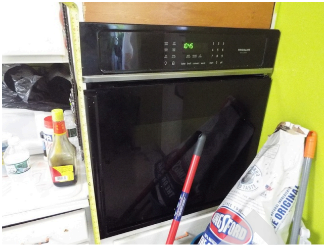
185. UFAS wall oven - unit 53 - building 8
