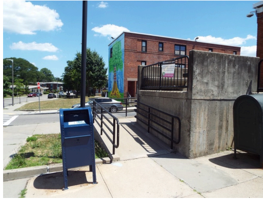
Ramp access - building 12 leasing office
