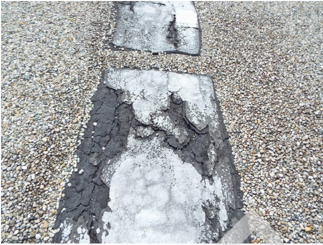
133. Roof traffic surface condition (Non-Critical Repair)
