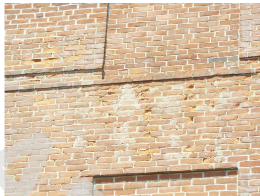
Brick masonry condition - building 7 (Non-Critical Repair)
