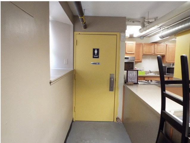
247. Common area - building 18 - teen center - women's restroom
