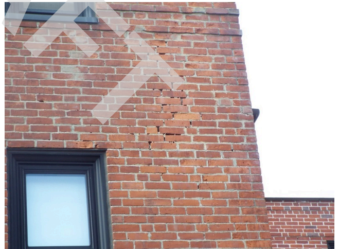
116. Brick masonry condition - building 14 (Non-Critical Repair)
