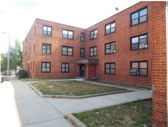
35. Typical sidewalk - building 6
