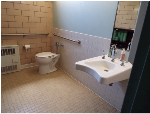
Common area - building 12 - women's restroom
