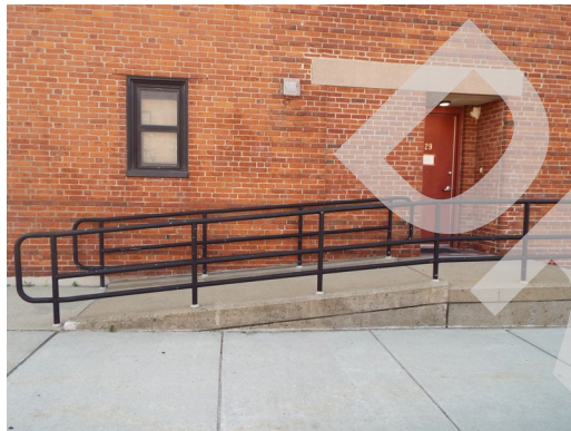
Ramp - Ames Way - building 6
