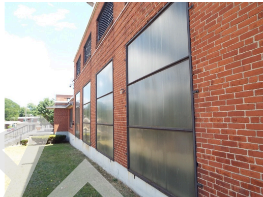
Steel framed fixed windows - building 12
