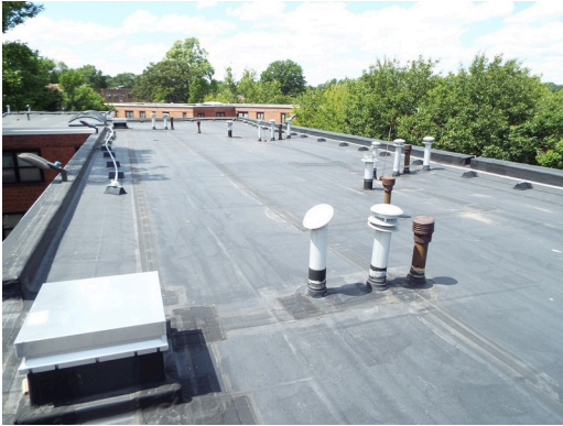
Roof overview - building 2
