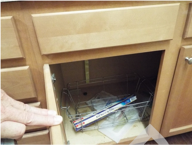
237. Common area - building 18 - teen center - kitchen
