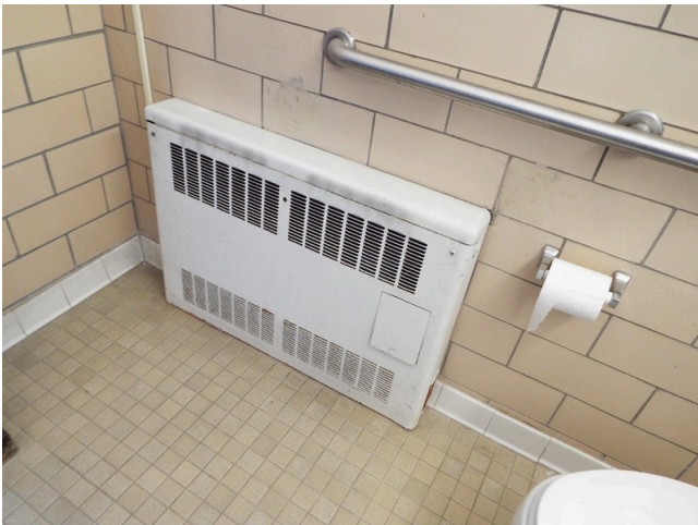
219. Common area - building 12 - women's restroom
