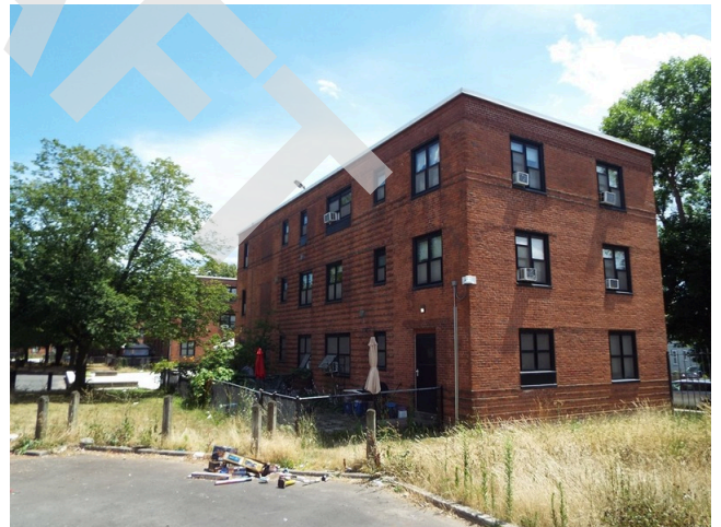
56. Overgrown vegetation - building 10 (Non-Critical Repair)
