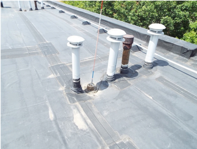
127. Roof penetrations- building 2
