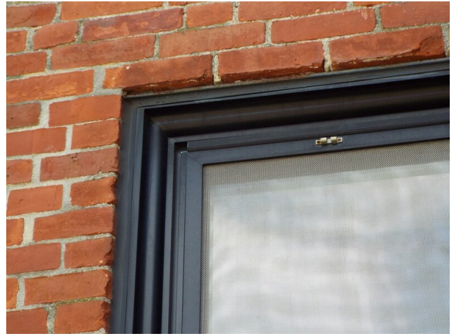
122. Typical window frame
