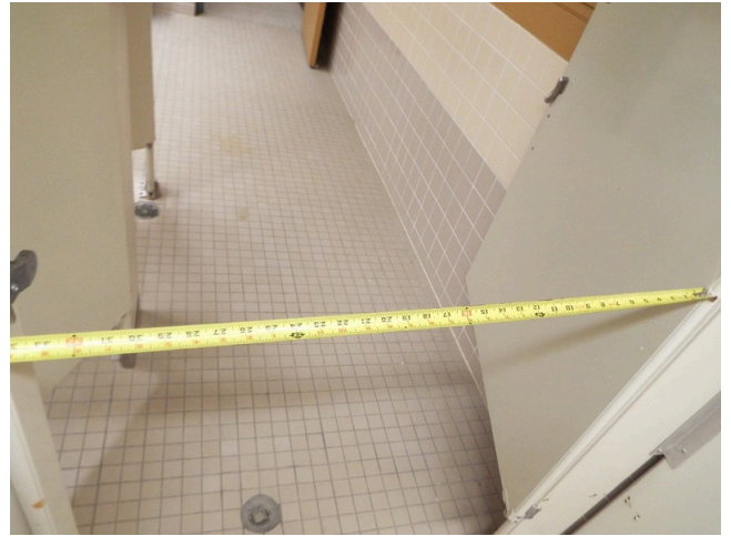
254. Common area - building 18 - teen center - women's restroom
