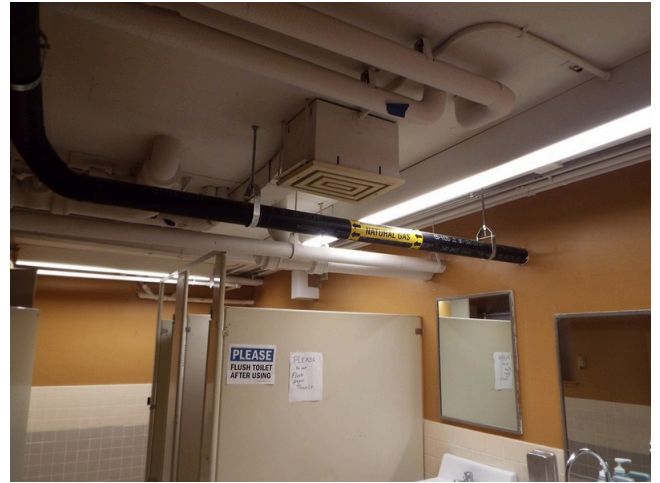
250. Common area - building 18 - teen center - women's restroom
