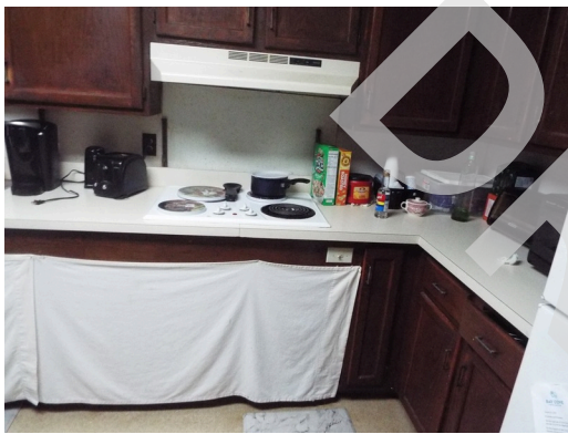
UFAS kitchen cabinets - 3-bed-1-bath-UFAS - unit 13 - building 4
