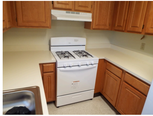
2-bed-1-bath - unit 140E - building 12 - kitchen cabinets (newer)
