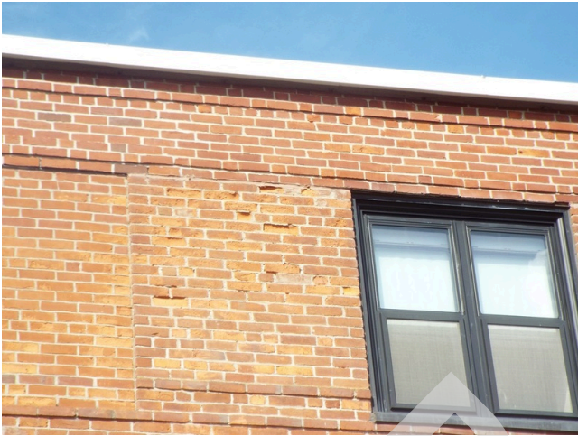
201. Brick masonry condition - building 17 (Non-Critical Repair)
