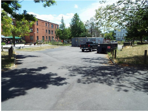
Asphalt paving - rear building 12
