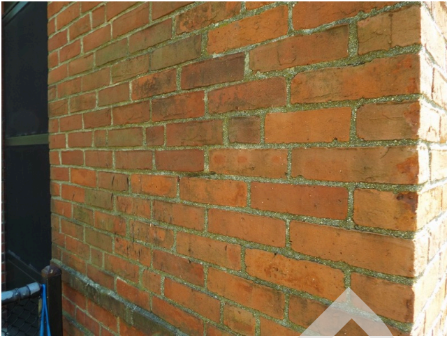
113. Brick masonry condition - building 11 (Non-Critical Repair)
