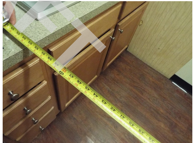
244. Common area - building 18 - teen center - kitchen
