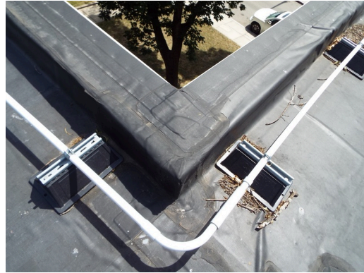
Roof flashing - building 2
