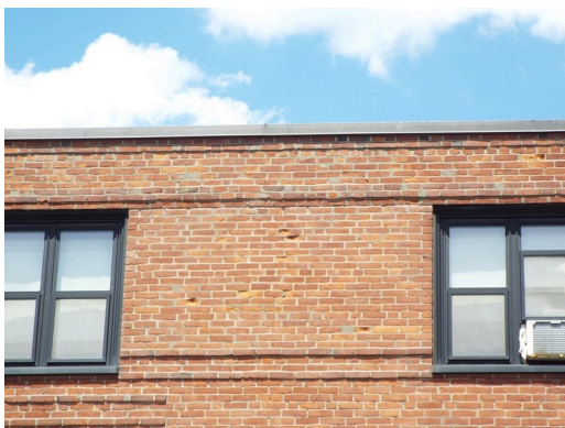
Brick masonry condition - building 8 (Non-Critical Repair)
