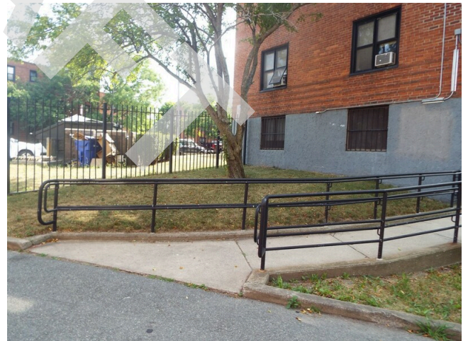
192. Ramp - teen center entry - building 18
