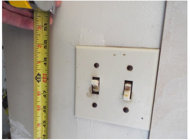
230. 3-bed-1-bath-UFAS - unit 13 - building 4
