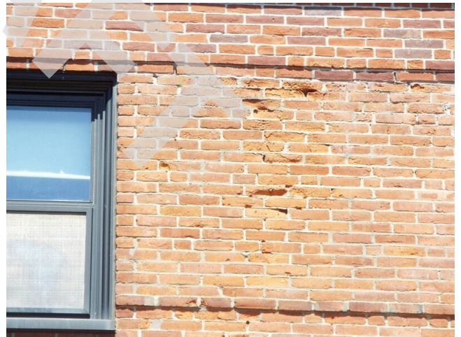
112. Brick masonry condition - building 10 (Non-Critical Repair)
