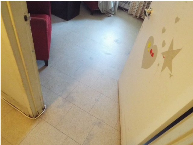
191. 4-bed-2-bath-UFAS - unit 53 - building 8
