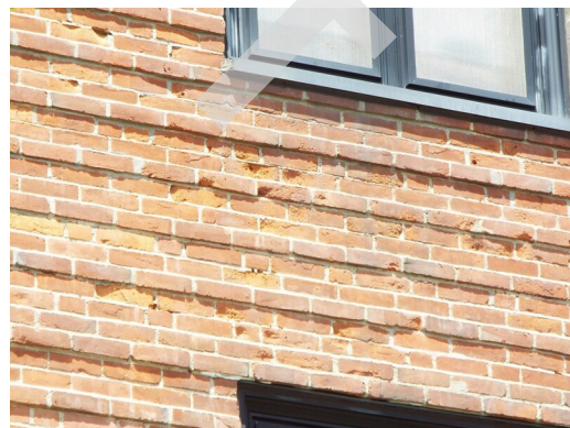
Brick masonry condition - building 9 (Non-Critical Repair)
