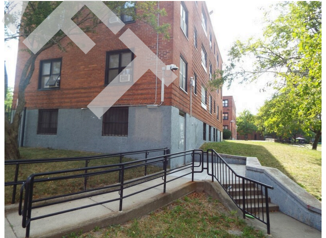
48. Ramp - teen center entry - building 18
