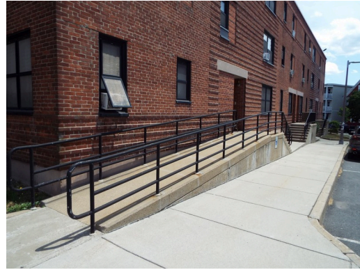
Ramp - building 7 unit 82
