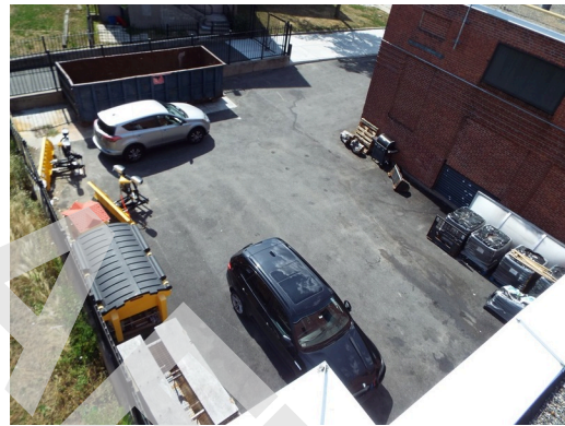
Asphalt paving service area - building 19
