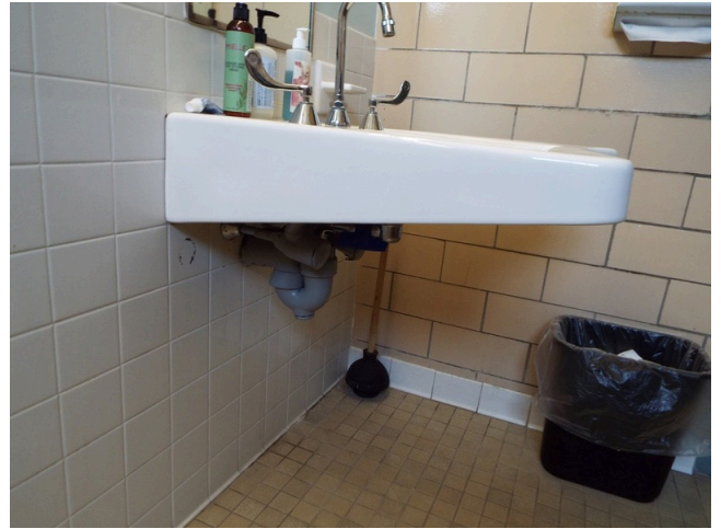
214. Common area - building 12 - women's restroom
