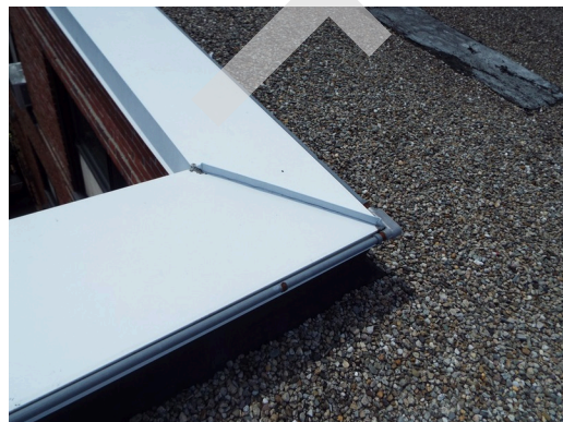
Roof coping - building 14
