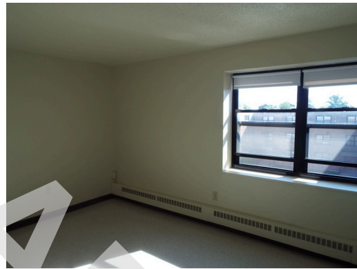
2-bed-1-bath - unit 140E - building 12- living room
