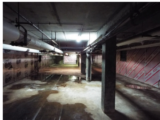
Framing - basement - building 17
