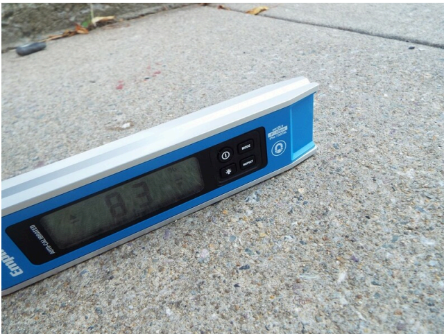
195. Ramp - teen center entry - building 18
