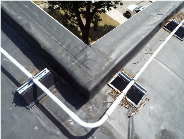
126. Roof flashing - building 2
