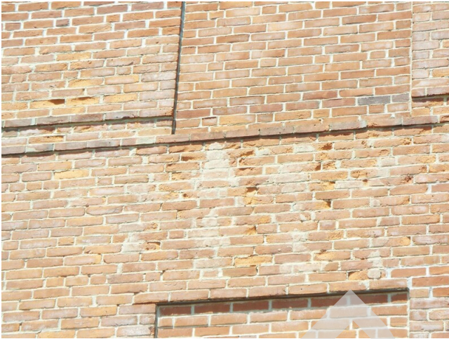
109. Brick masonry condition - building 7 (Non-Critical Repair)
