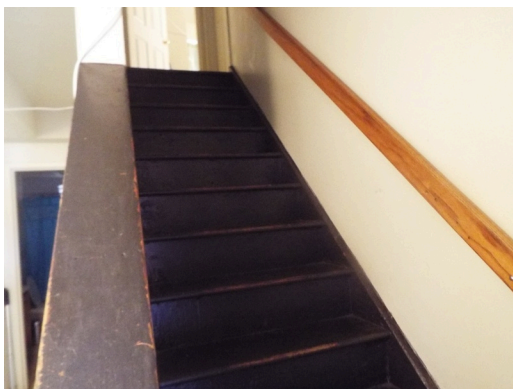
5-bed-2-bath-TH - unit 190A - building 14 - stair
