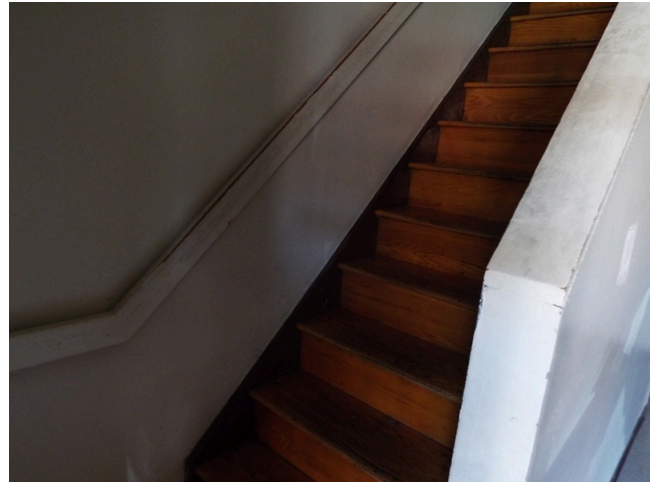
146. 3-bed-1.5-bath-TH - unit 160B - building 13 - stair
