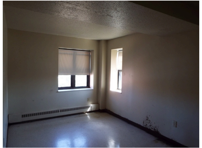
150. 3-bed-1.5-bath-TH - unit 160B - building 13
