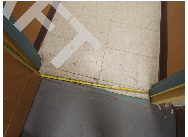
248. Common area - building 18 - teen center - women's restroom
