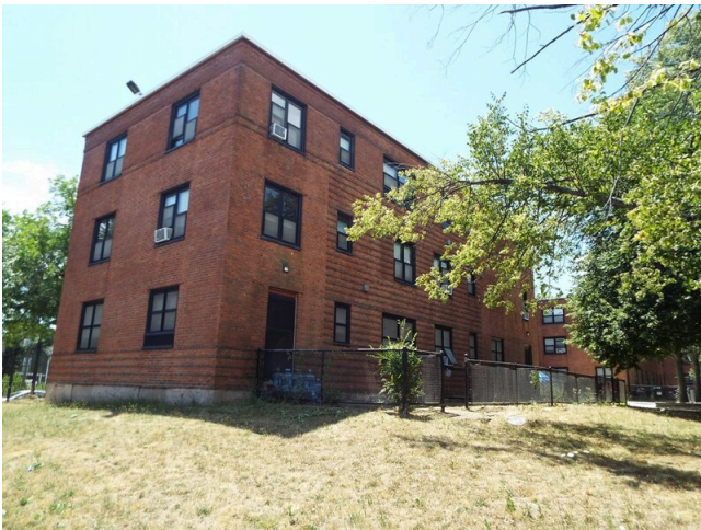
103. Typical elevation - side - building 11
