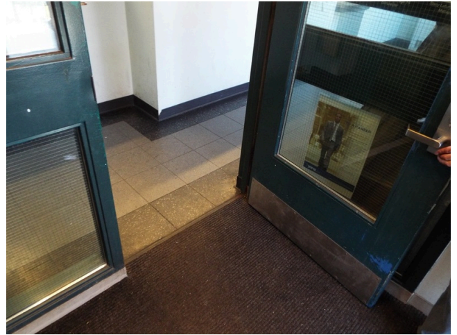
226. Common area - building 12 - leasing area interior entry door
