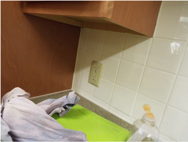
245. Common area - building 18 - teen center - kitchen
