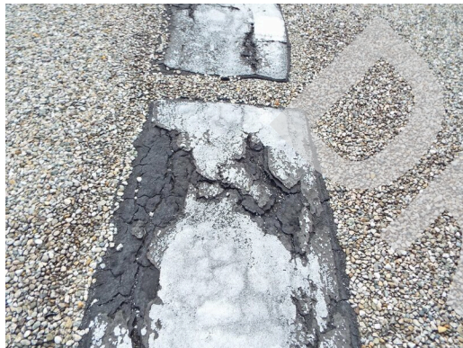
Roof traffic surface condition (Non-Critical Repair)
