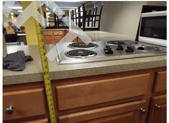
236. Common area - building 18 - teen center - kitchen
