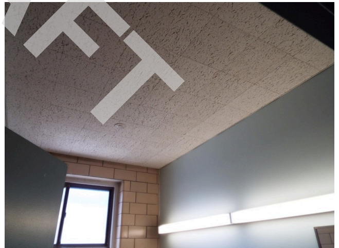
220. Common area - building 12 - women's restroom
