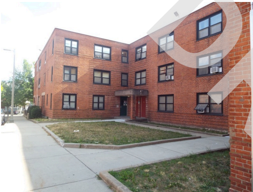
Typical sidewalk - building 6
