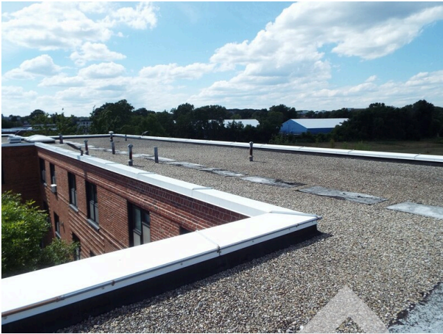
129. Roof overview - building 14
