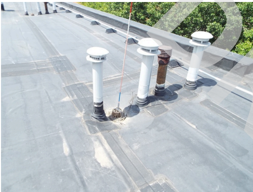
Roof penetrations- building 2
