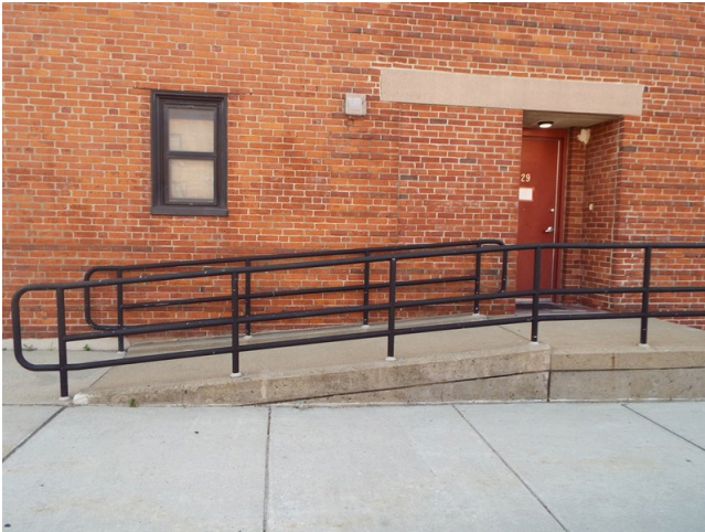
47. Ramp - Ames Way - building 6
