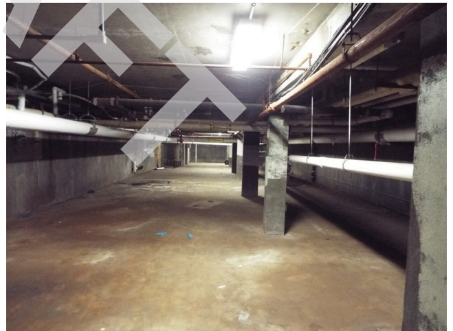
80. Framing - basement - building 19
