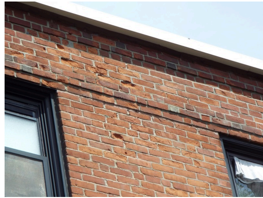
Brick masonry condition - building 4 (Non-Critical Repair)
