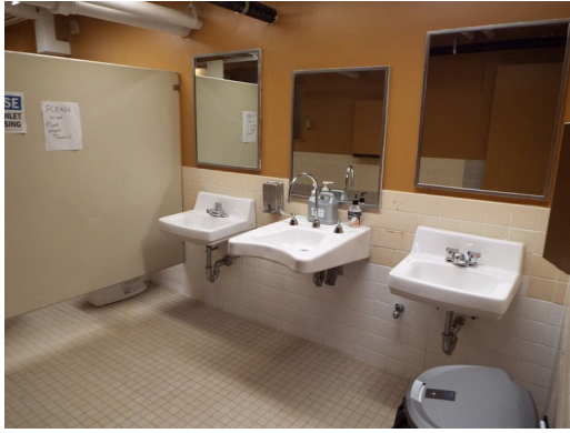
Common area - building 18 - teen center - women's restroom
