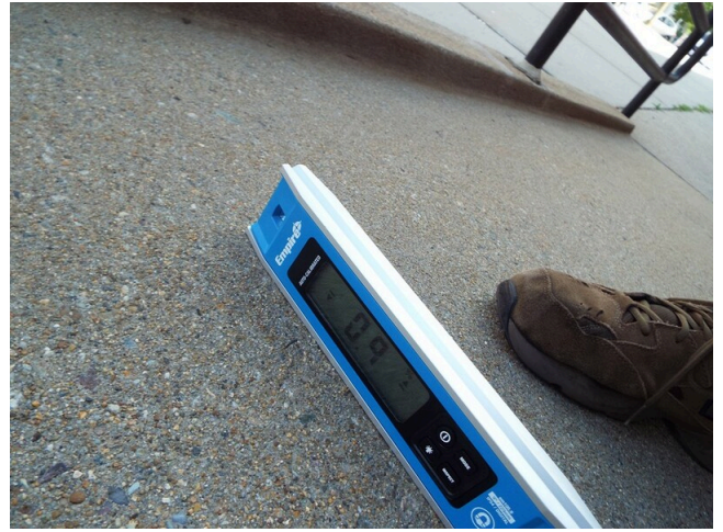
198. Ramp - Ames Way - building 6
