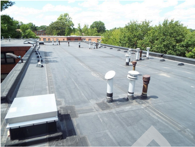
125. Roof overview - building 2
