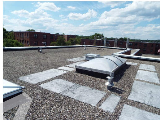
Roof overview - building 12
