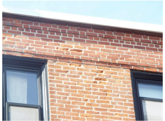
202. Brick masonry condition - building 18 (Non-Critical Repair)
