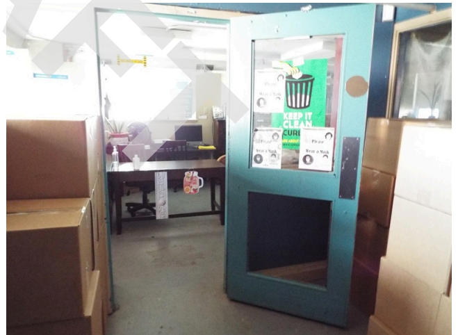
228. Common area - building 18 - teen center - interior entry door
