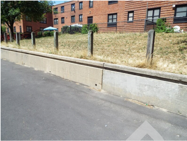
5. Concrete retaining wall
