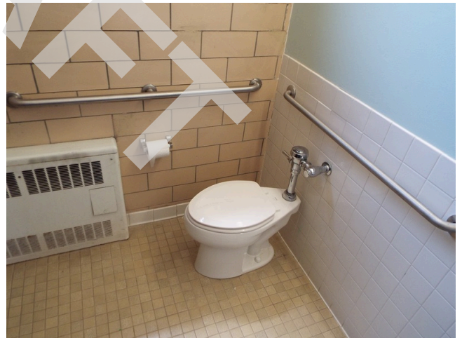
216. Common area - building 12 - women's restroom
