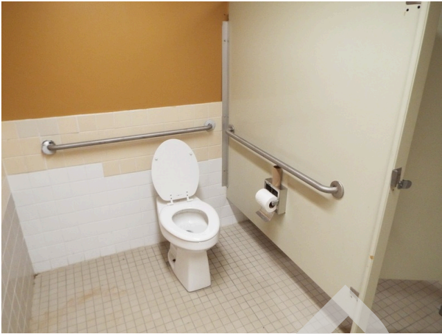
253. Common area - building 18 - teen center - women's restroom
