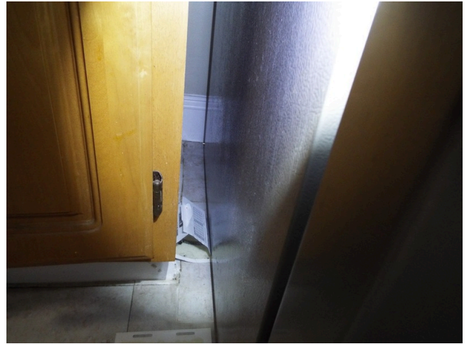
78. 2-bed-1-bath - unit 160C - building 15 - rodents reported - kitchen (Critical Repair)
