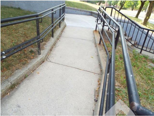
193. Ramp - teen center entry - building 18
