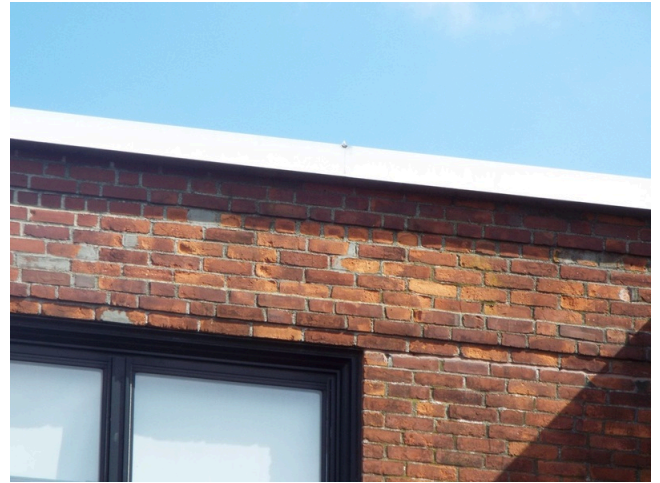
118. Brick masonry condition - building 17 (Non-Critical Repair)
