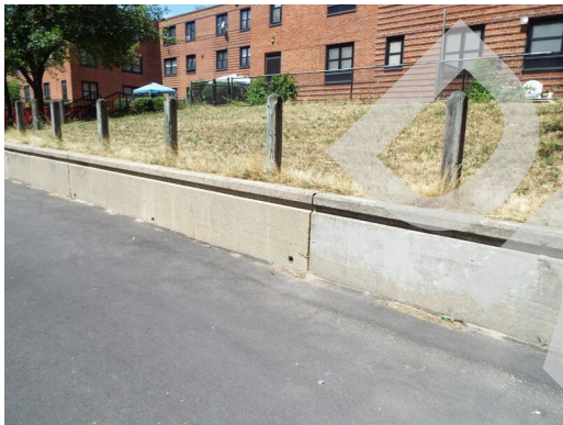
Concrete retaining wall
