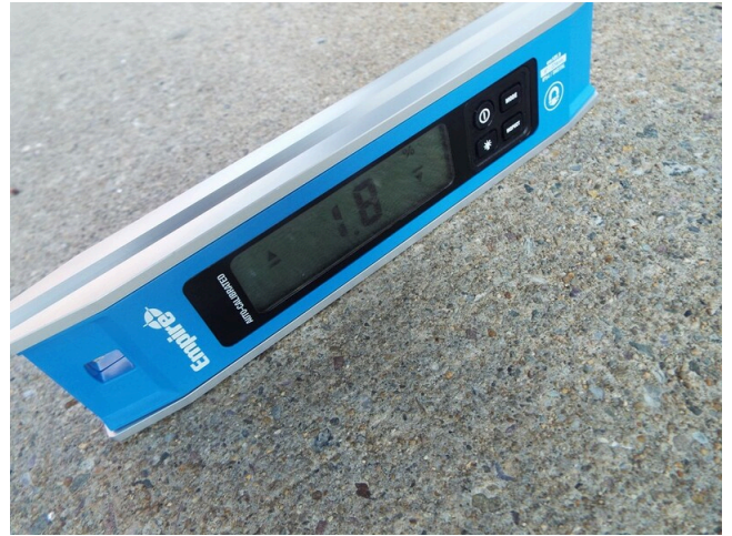
194. Ramp - teen center entry - building 18
