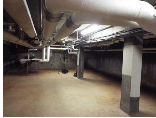
Framing - basement - building 19
