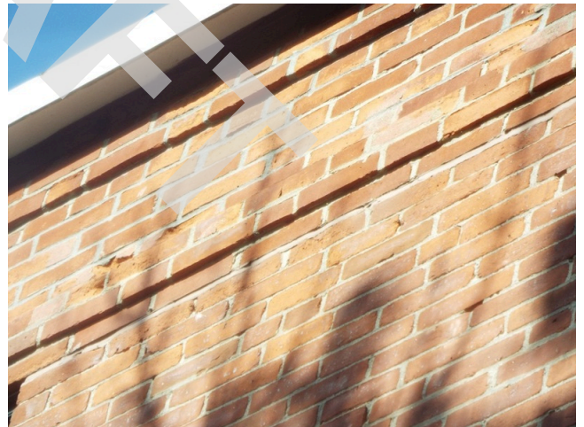
108. Brick masonry condition - building 6 (Non-Critical Repair)
