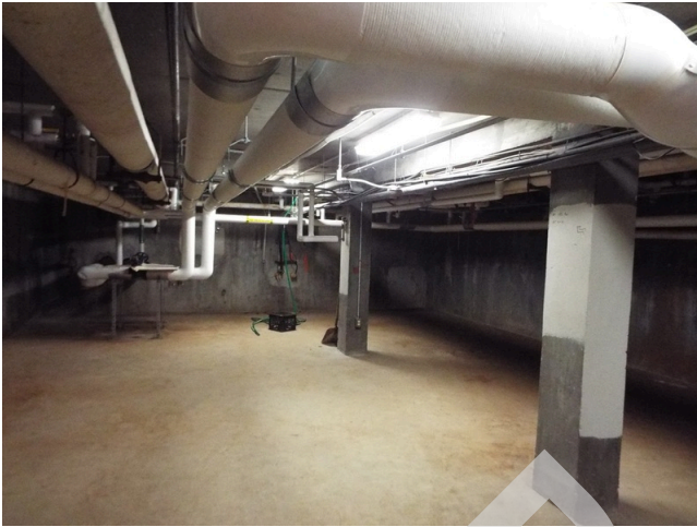
81. Framing - basement - building 19
