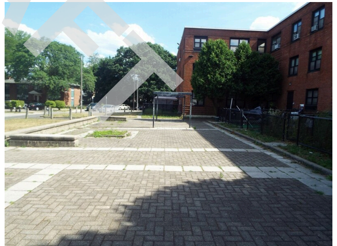
88. Concrete paver terrace - building 19
