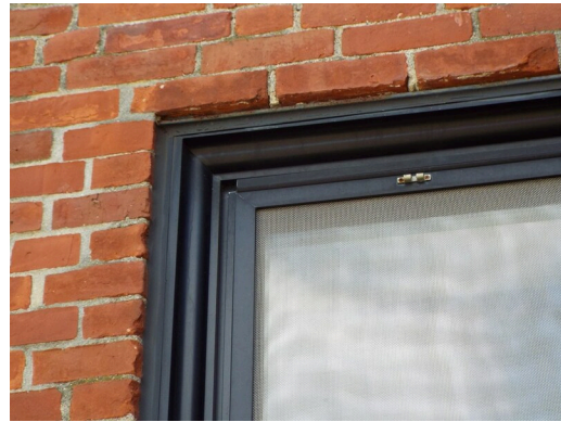
Typical window frame
