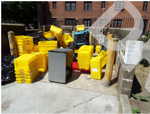
Dumpster pad condition - building 1 (Non-Critical Repair)
