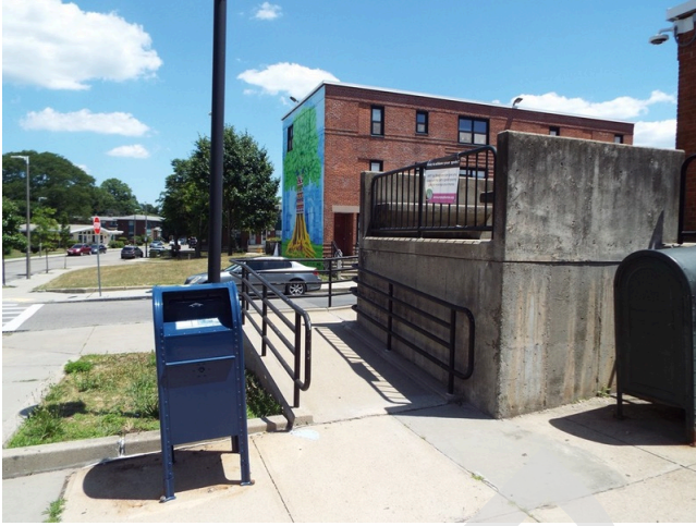
45. Ramp access - building 12 leasing office
