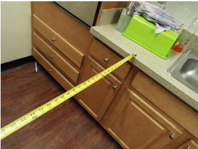
243. Common area - building 18 - teen center - kitchen
