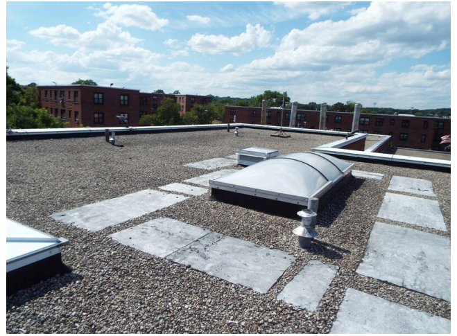
134. Roof overview - building 12
