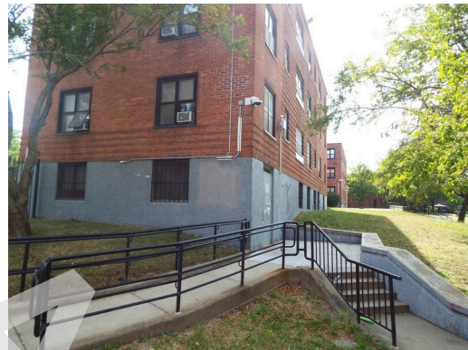
Ramp - teen center entry - building 18
