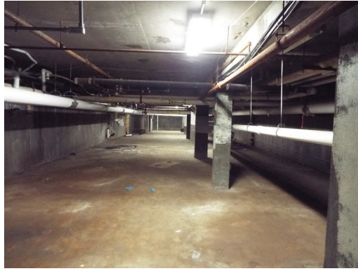
Framing - basement - building 19
