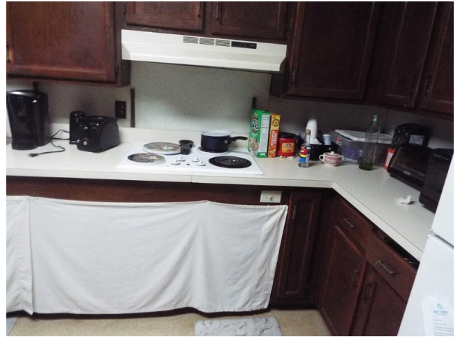
234. UFAS kitchen cabinets - 3-bed-1-bath-UFAS - unit 13 - building 4
