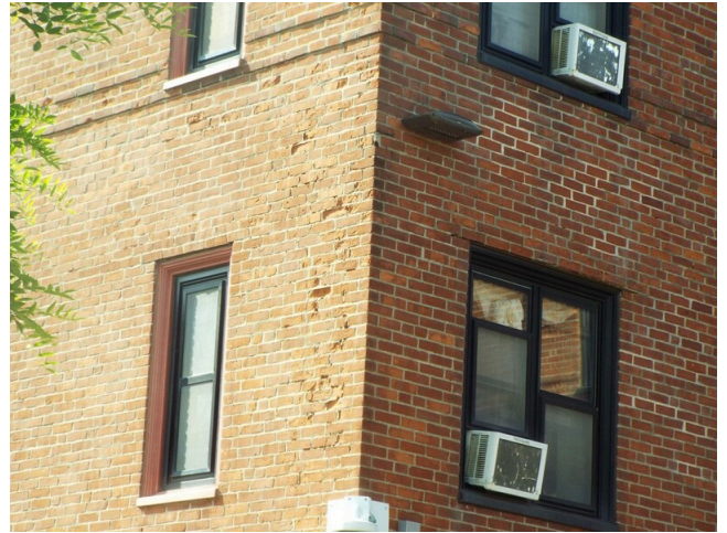
106. Brick masonry condition - building 3 (Non-Critical Repair)
