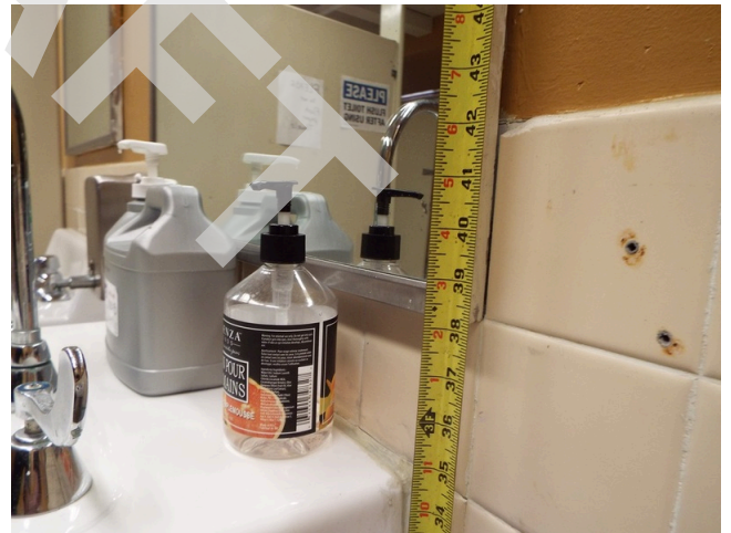
252. Common area - building 18 - teen center - women's restroom
