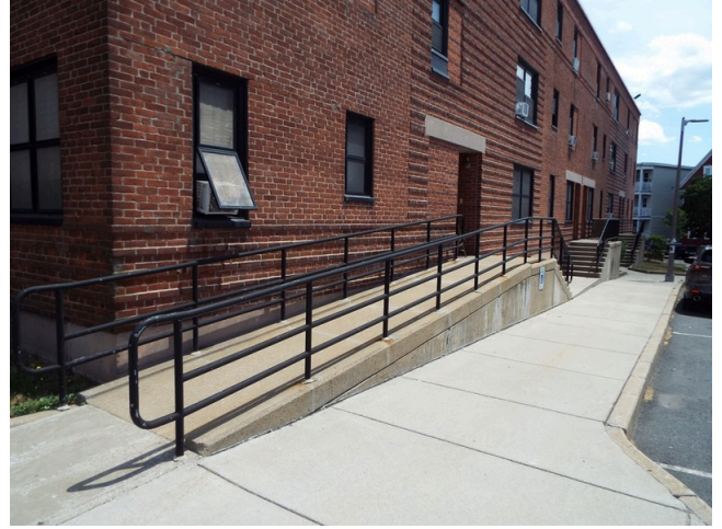
46. Ramp - building 7 unit 82
