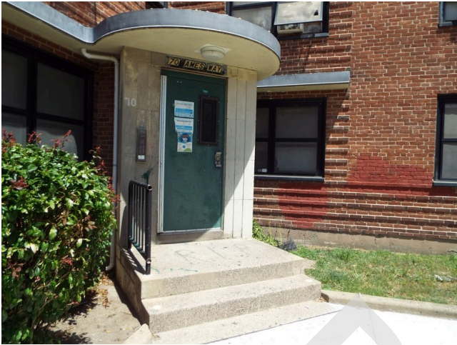
37. Typical building entry steps
