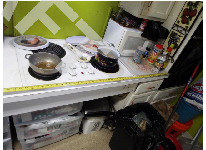
184. UFAS cooktop - unit 53 - building 8
