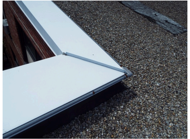
130. Roof coping - building 14
