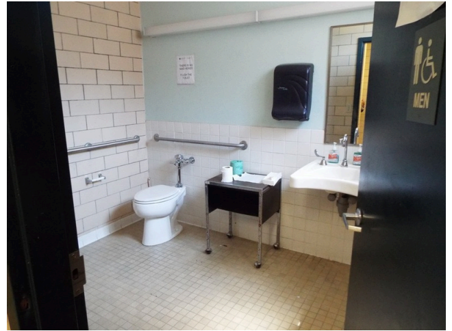
170. Common area - building 12 - men's restroom
